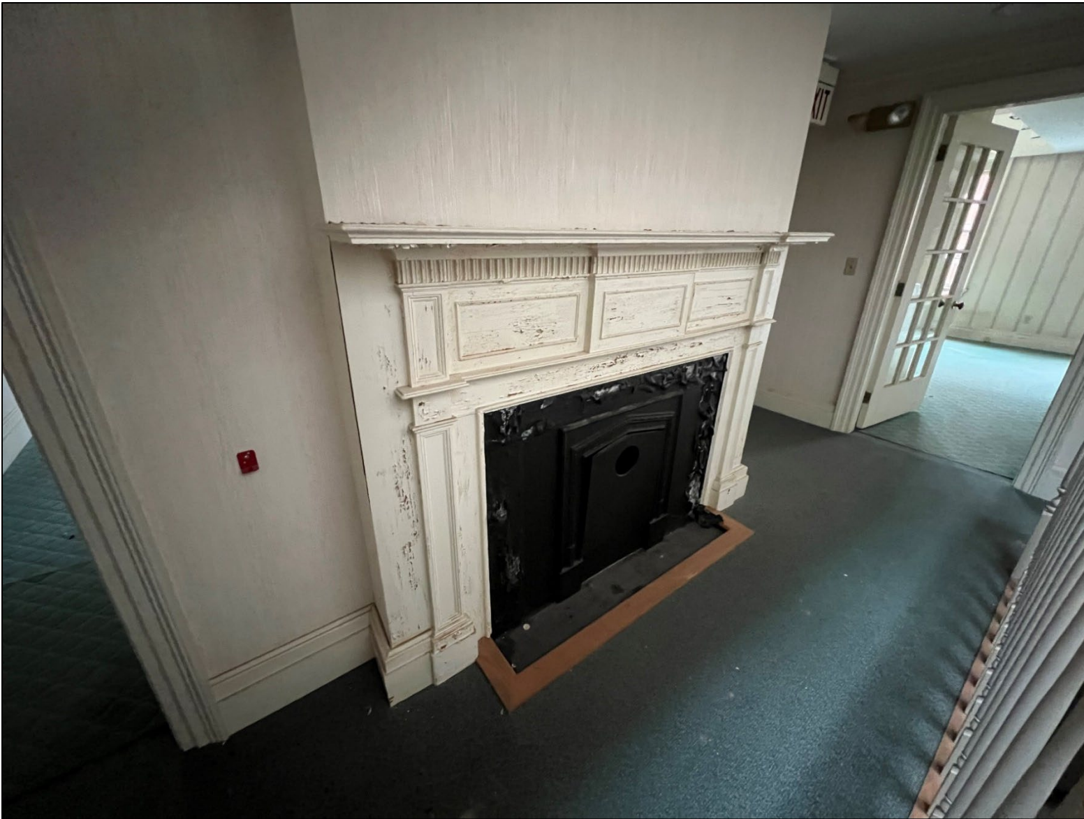
Photograph 12. Interior elevation, south wall second story central room, camera facing west. This room is now the location of the new central stairs..
