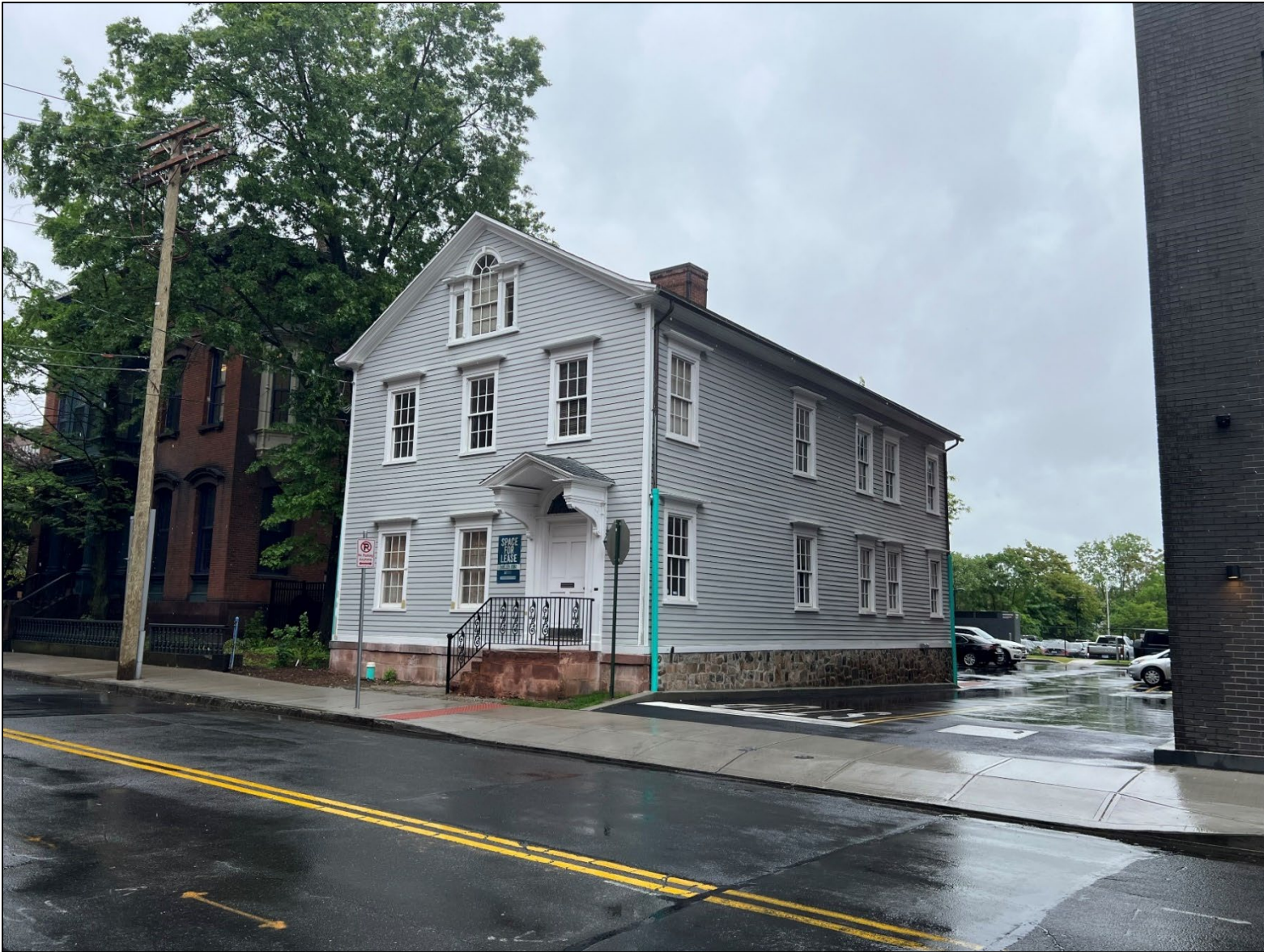
Photograph 1. Front (western) and southern elevations, camera facing east.
