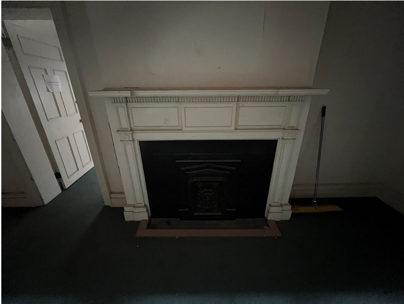
Photograph 8. Fireplace in south central room of original portion of building, first floor (north wall), camera facing north.
