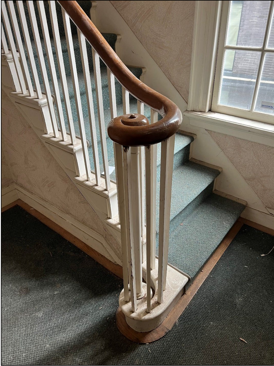
Photograph 6. Front stairway from the first floor hallway, camera facing southeast.
