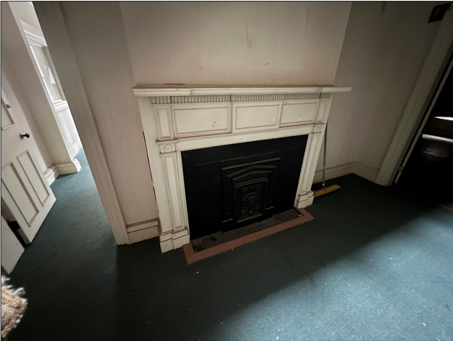
Photograph 9. Fireplace (south) wall in central room, north side of first floor in original main block, camera facing south.
