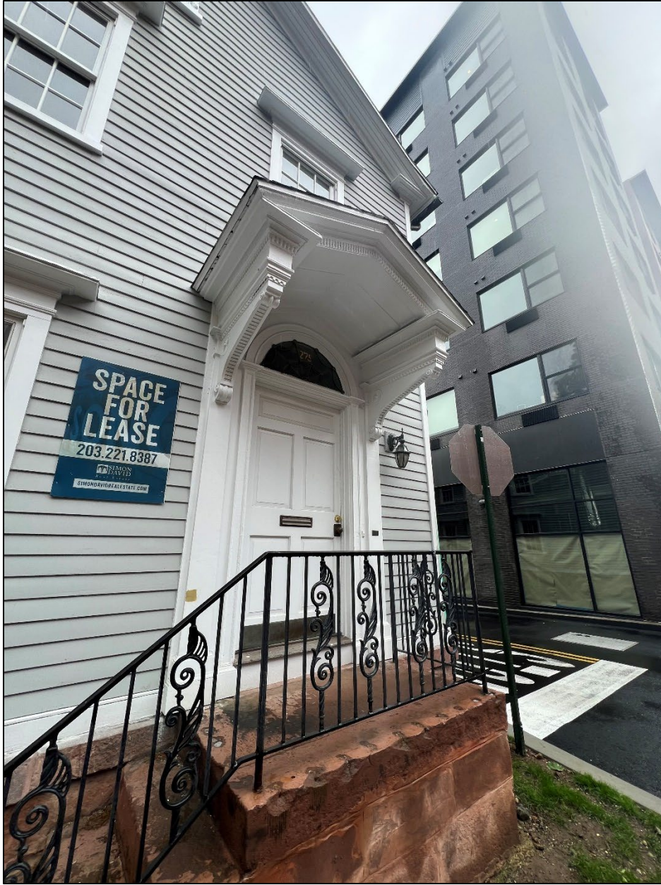
Photograph 5. Front entry, camera facing southeast.
