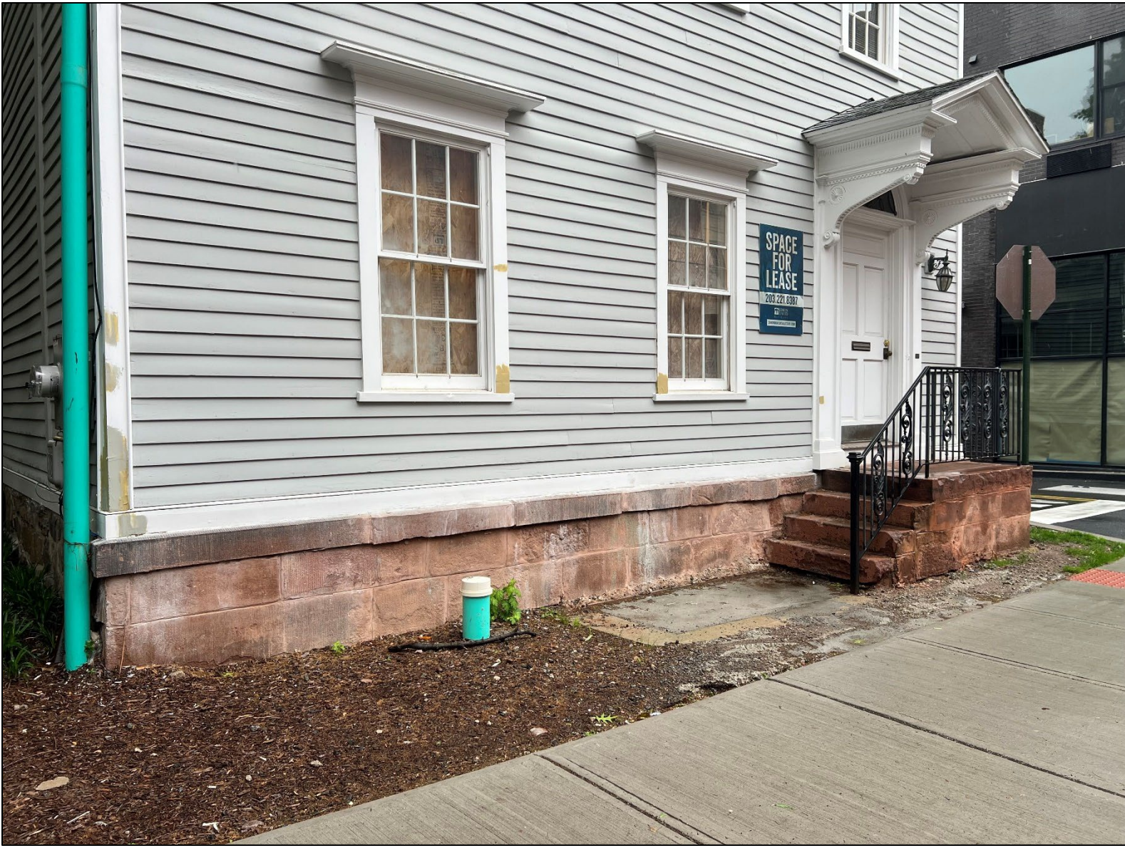
Photograph 4. The new foundation and stoop, camera facing south.
