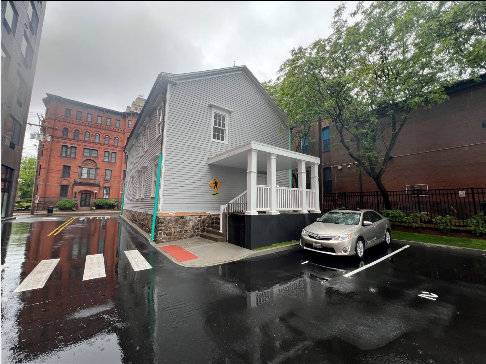
Photograph 3. Rear (eastern) and southern elevations, camera facing northwest.
