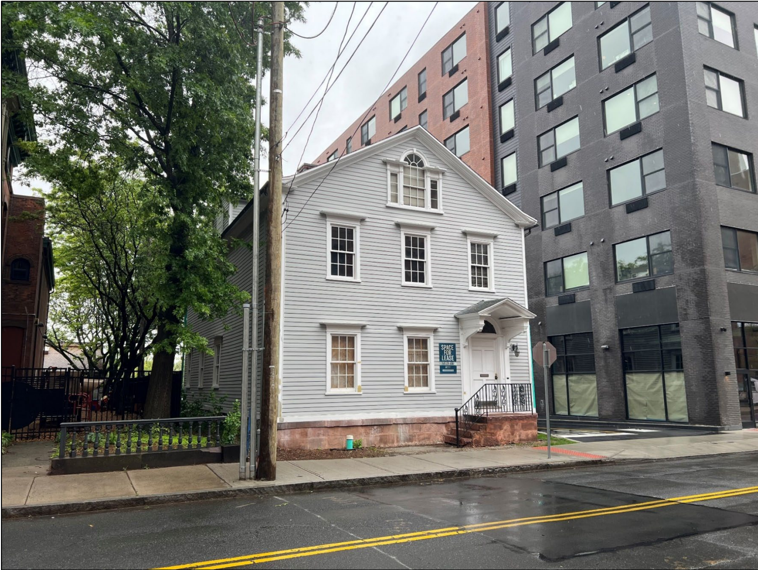
Photograph 2. Front (western) and northern elevations as viewed from the west.
