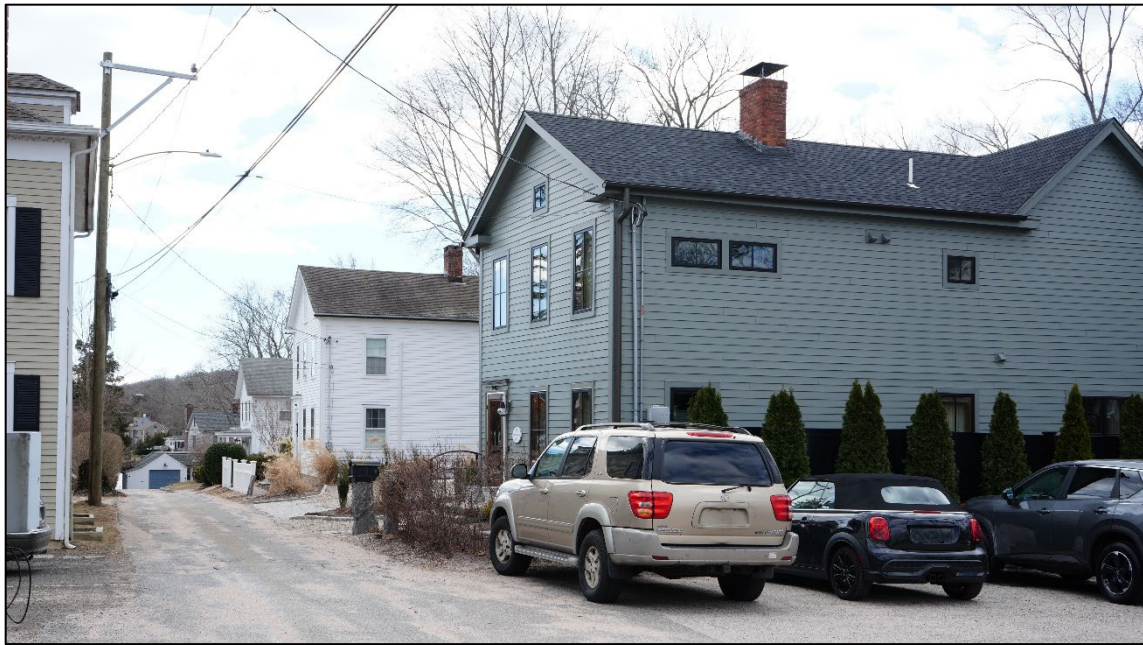
1 of 25. View of upper Bank Lane, facing south and west, showing intact and modified nineteenth and early twentieth century structures.
