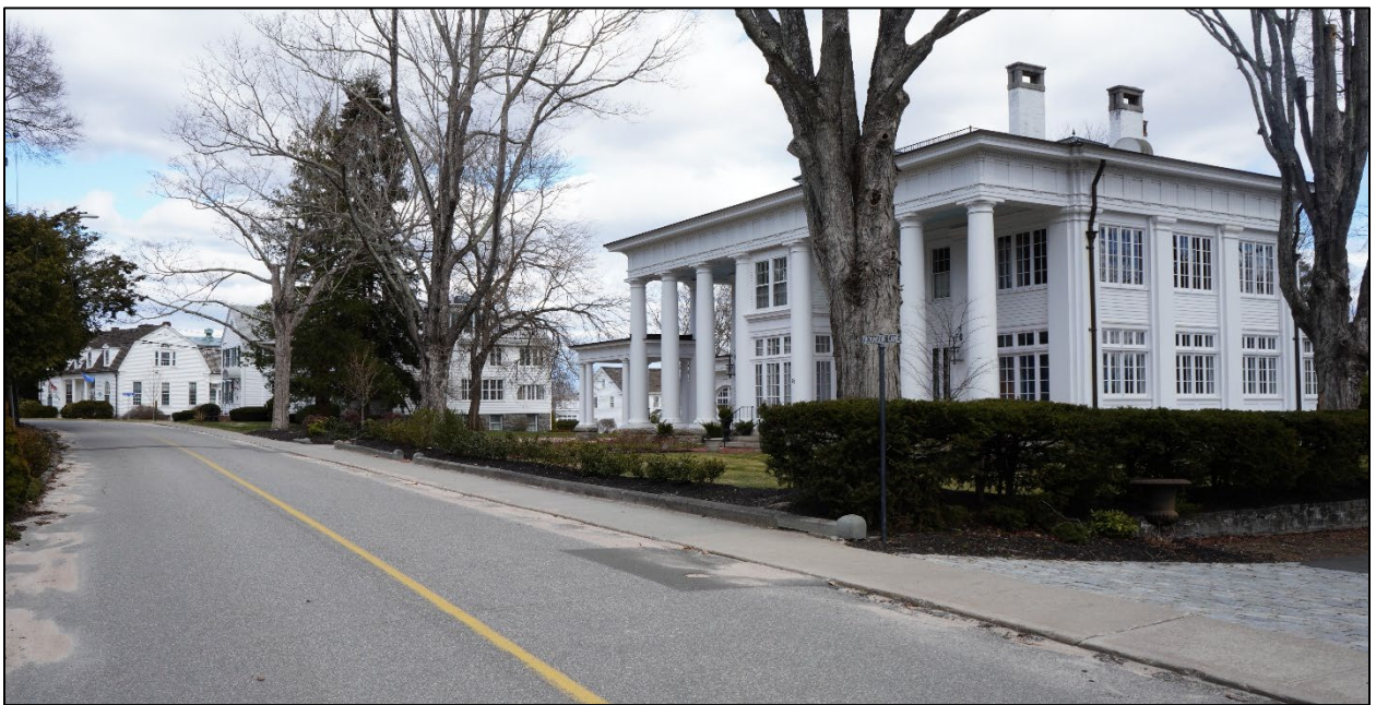
12 of 25. View of lower North Main Street residential area, facing northeast, showing 21 North Main Street through 31 Main Street.
