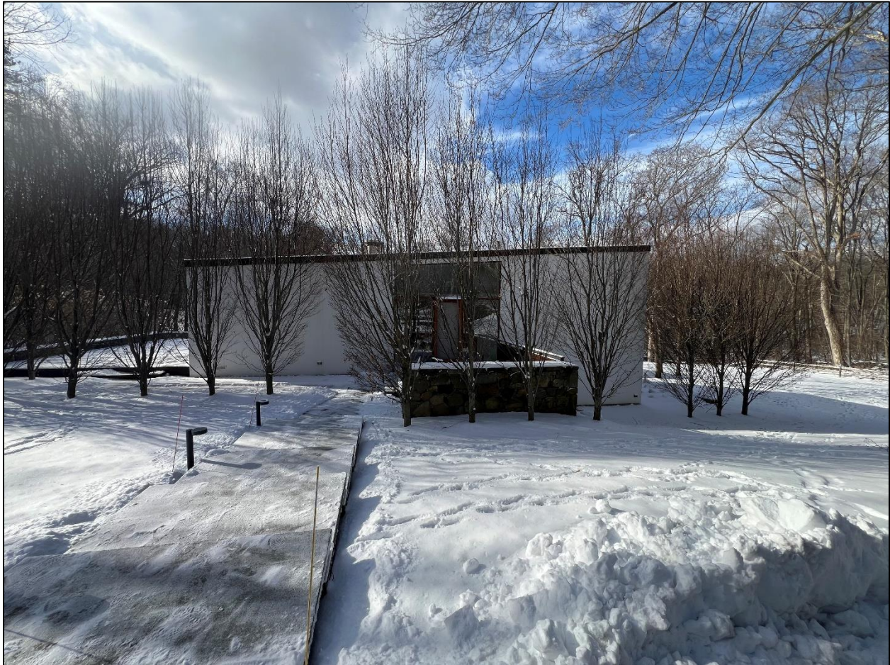
Photograph 11 of 26. Looking east at the façade of 160 Chichester Road.
