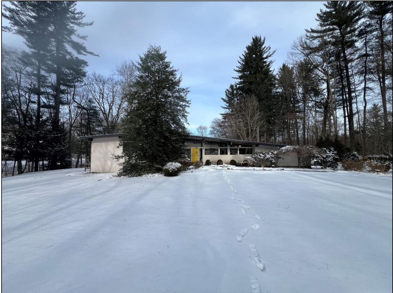
Photograph 1 of 26. Looking north at the façade of 126 Chichester Road.
