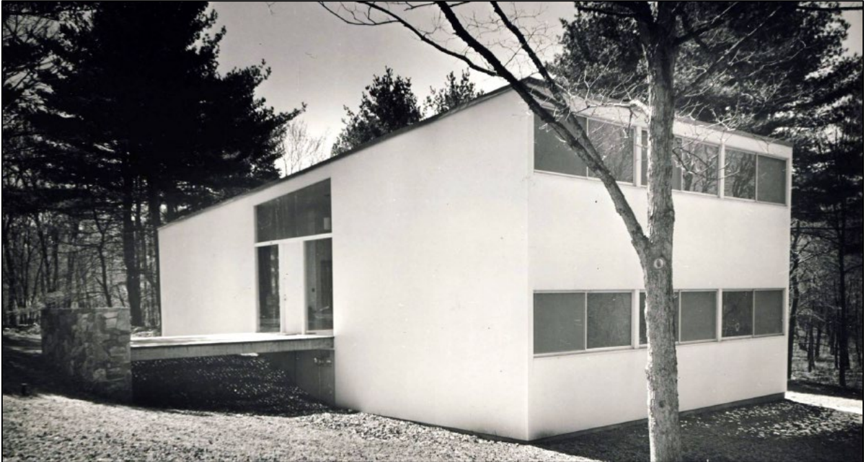
Figure 14. The Smallen House (160 Chichester Road) in 1969 (Collections of the New Canaan Historical Society)
