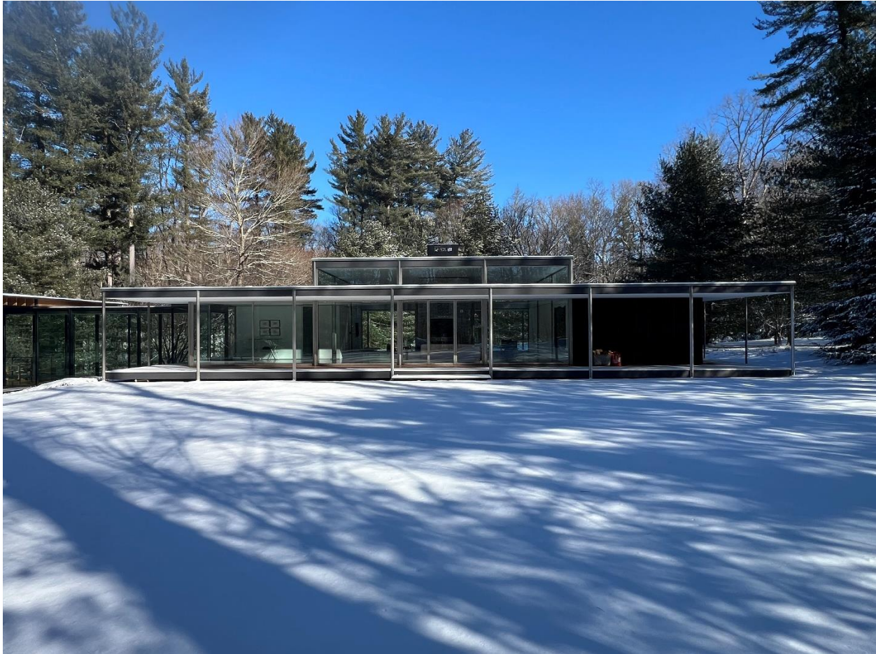
Photograph 22 of 26. Looking north at the Lee II House at 202 Chichester Road. The new addition is at the left edge of the photograph.
