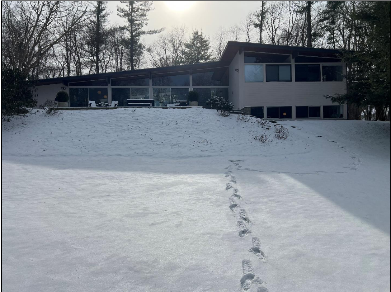
Photograph 2 of 26. Looking south at the rear of 126 Chichester Road.
