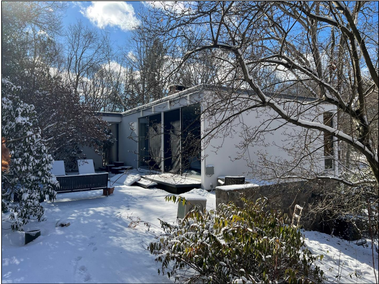
Photograph 8 of 26. Looking southwest at the north and east sides of 136 Chichester Road.
