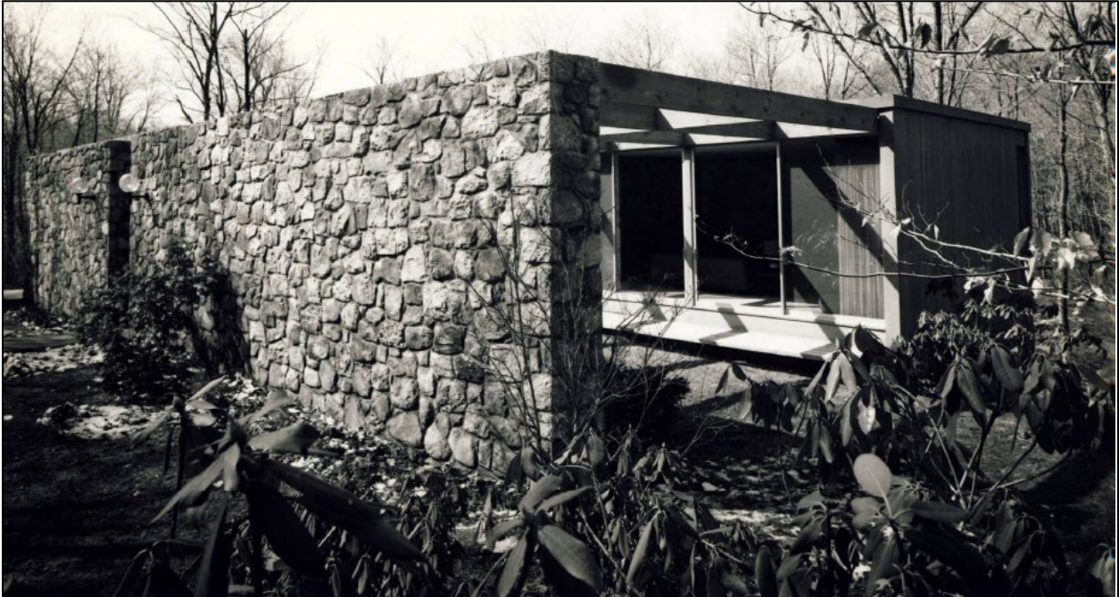
Figure 12. The Becker House in 1967 (collections of the New Canaan Historical Society).
