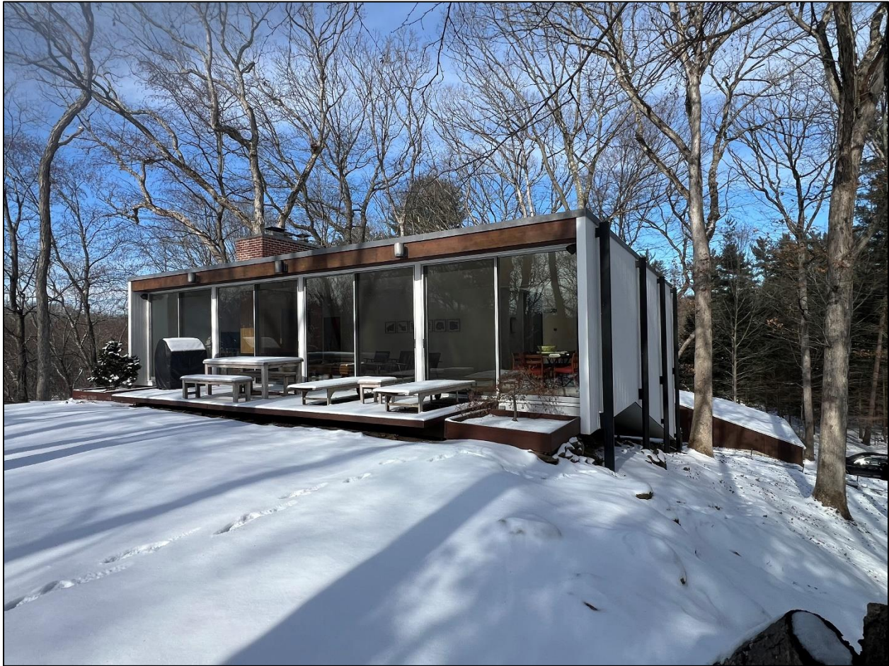
Photograph 18 of 26. Looking northeast at the Parsons House at 188 Chichester Road.
