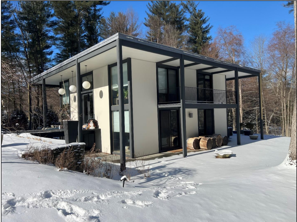
Photograph 5 of 26. Looking northwest at the System House.
