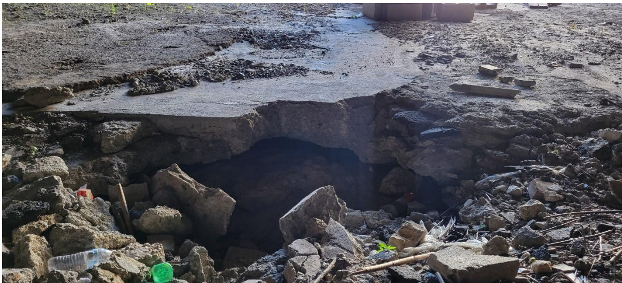
Photo 74: Photo showing the opening of the canal at the Rolling Mill (Building 34/223).
