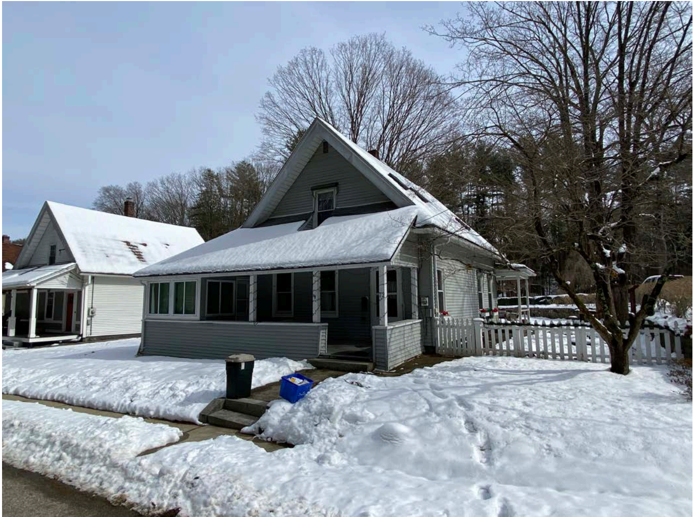
Photo 78 of 99. View of 72 Highland Terrace, looking east.
