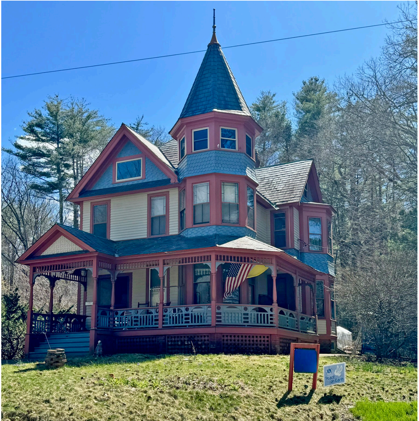
Photo 79 of 99. View of 78 Highland Terrace, looking south.
