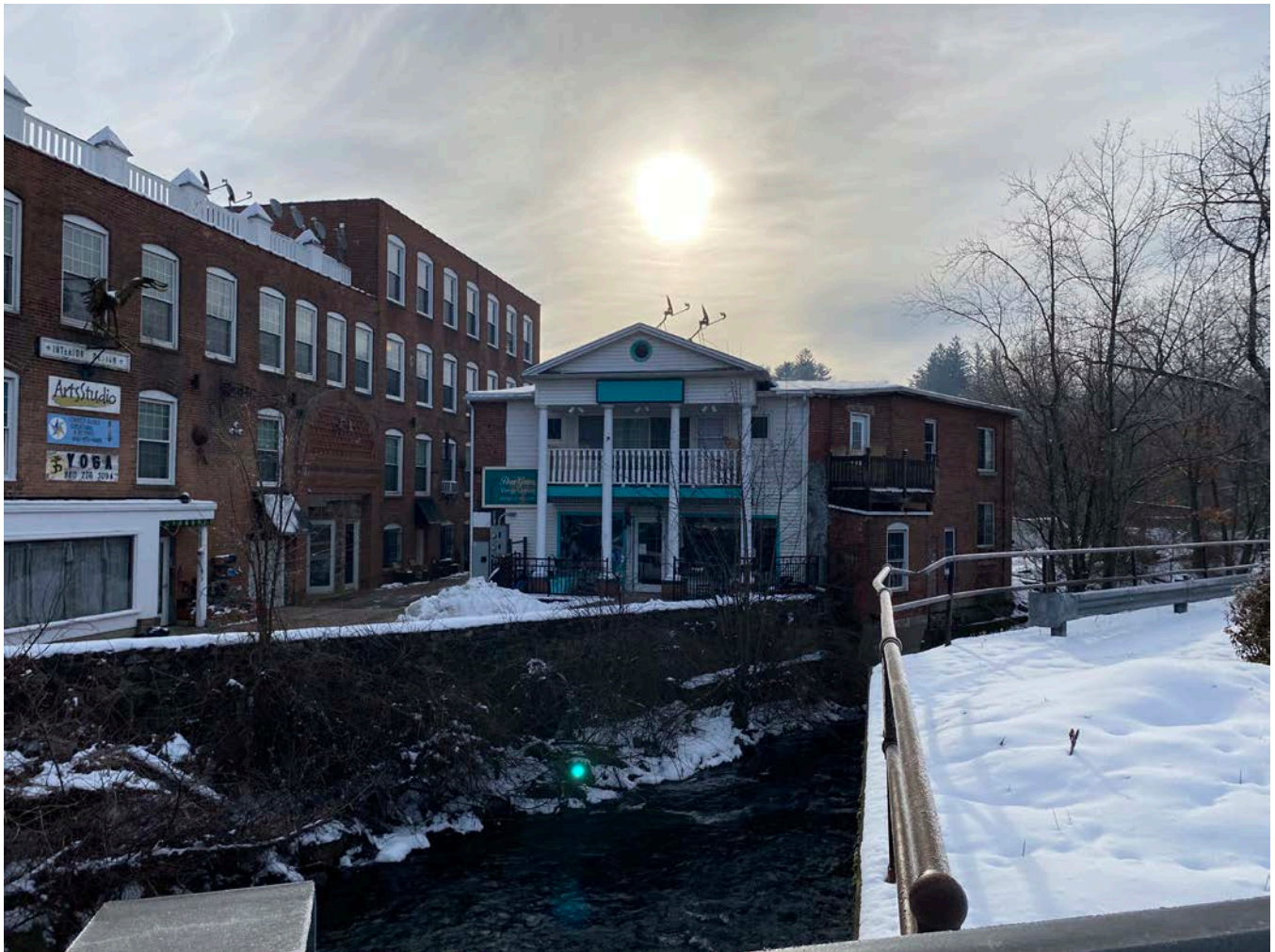
Photo 57 of 99. View of 2 River Road, looking west.
