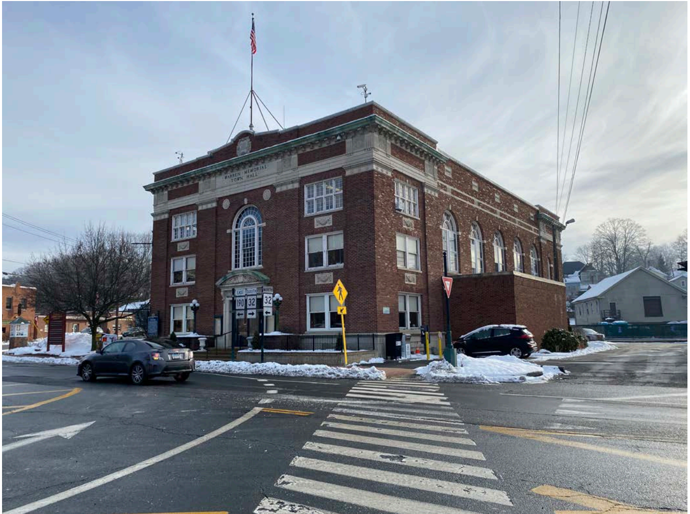
Photo 54 of 99. View of 1 Main Street, looking northeast.
