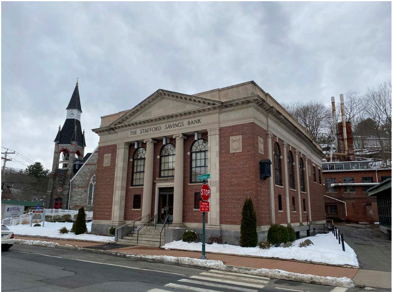
Photo 18 of 99. View of 2 Furnace Avenue, looking east.
