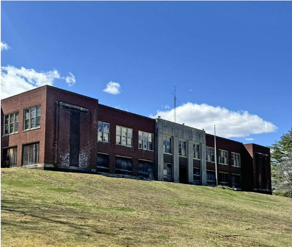
Photo 85 of 99. View of the Earl M. Witt School, looking west.
