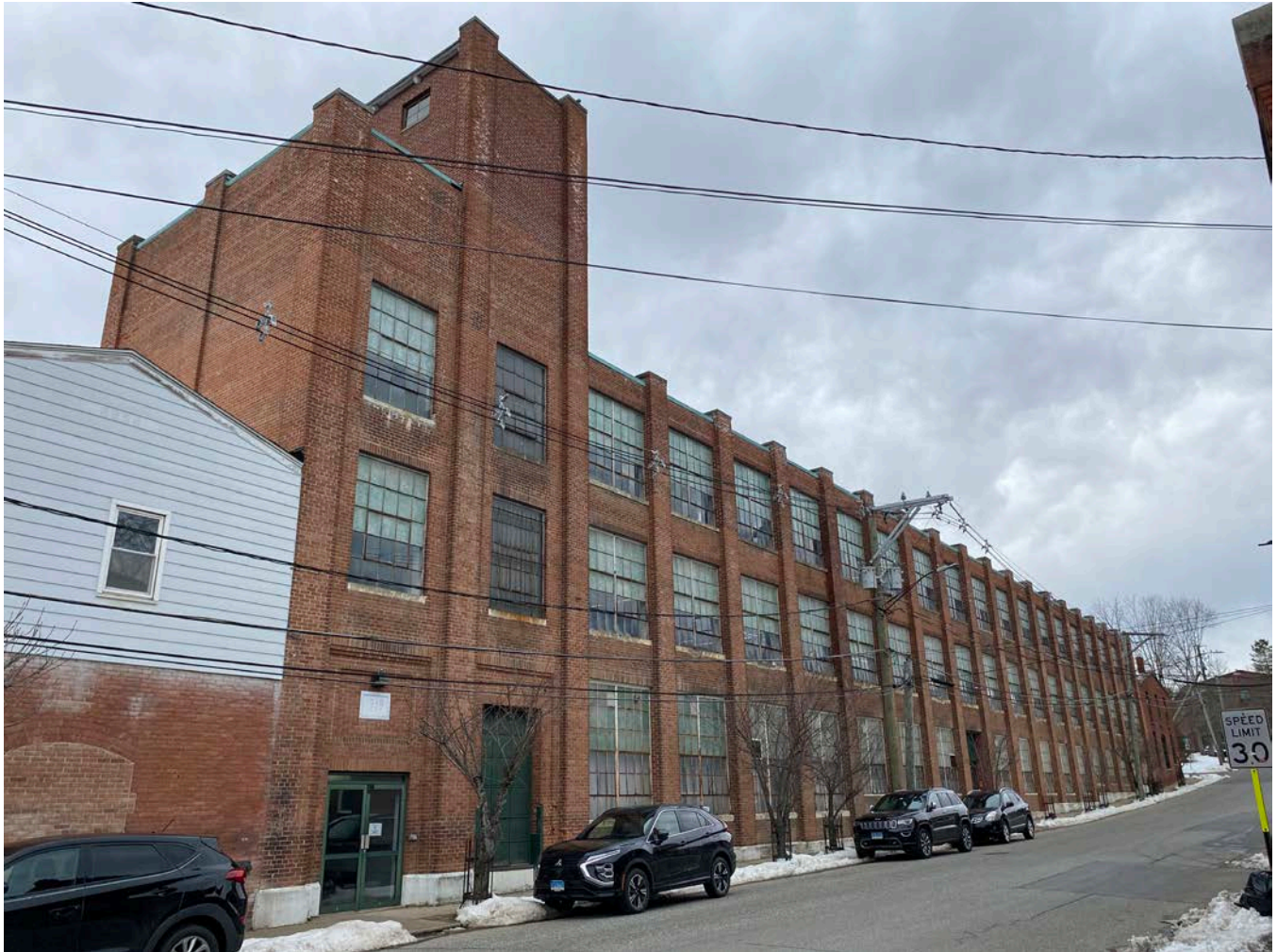
Photo 15 of 99. View of 8 Furnace Avenue (Weave Mill), looking northwest.
