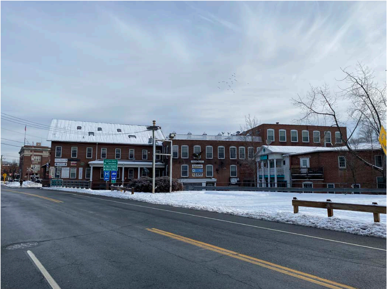
Photo 58 of 99. View of the complex at 2 River Road, looking north-northeast.
