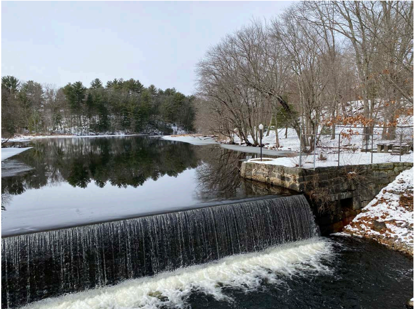
Photo 93 of 99. View of the Chelsea Dam and Pond, looking northwest.
