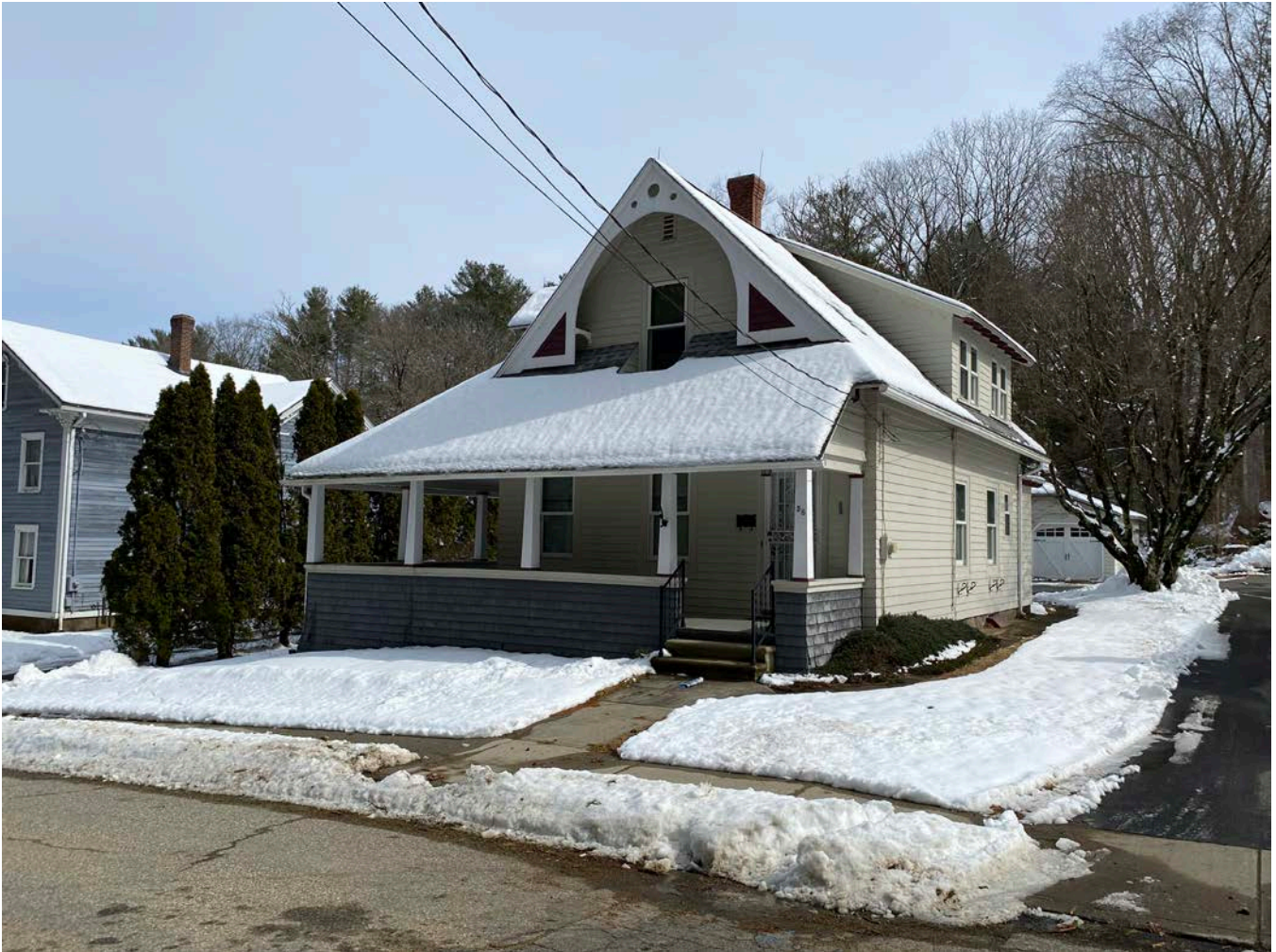
Photo 74 of 99. View of 56 Highland Terrace, looking east.
