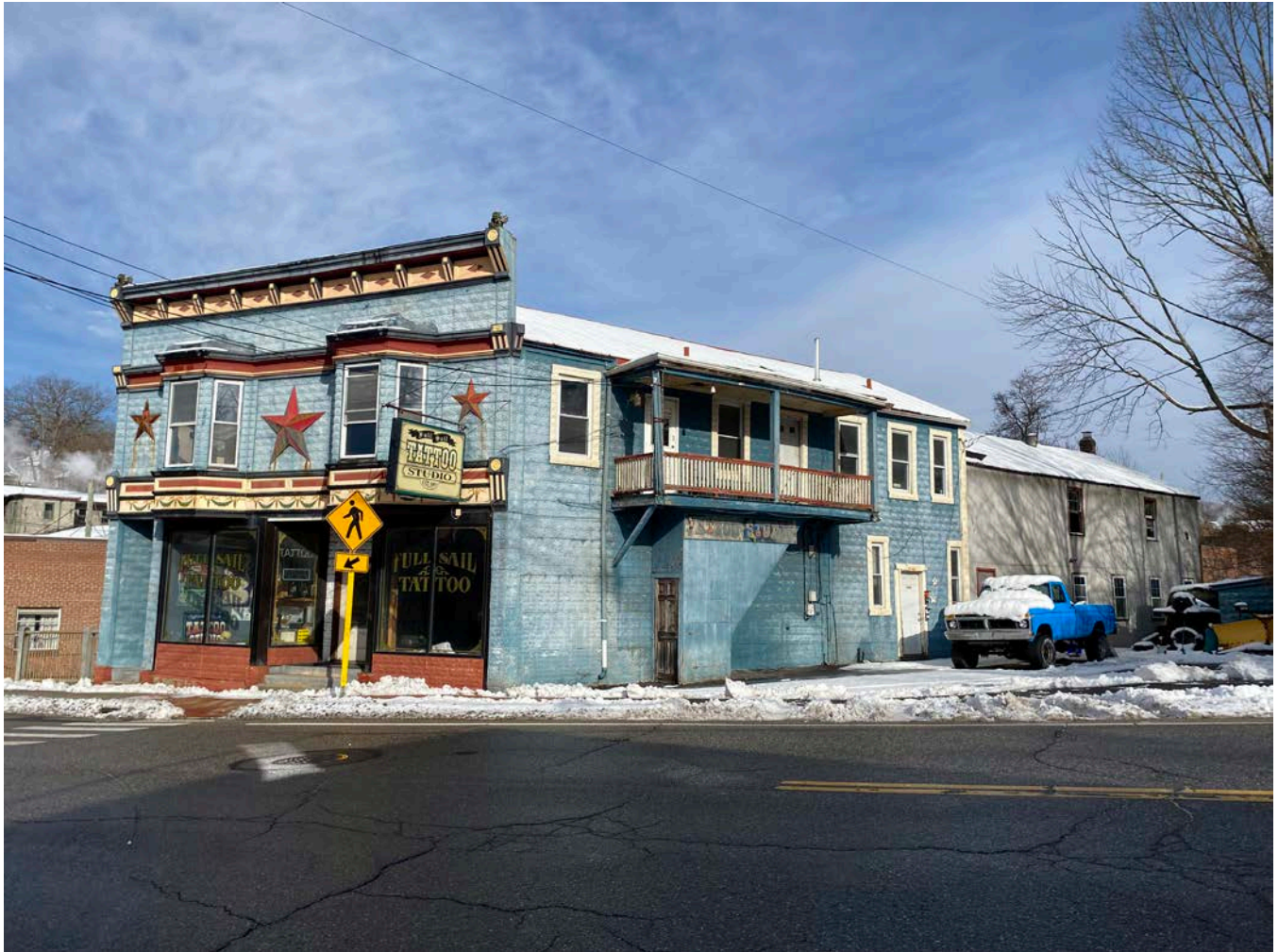
Photo 21 of 99. View of 30 East Main Street, looking north-northwest.
