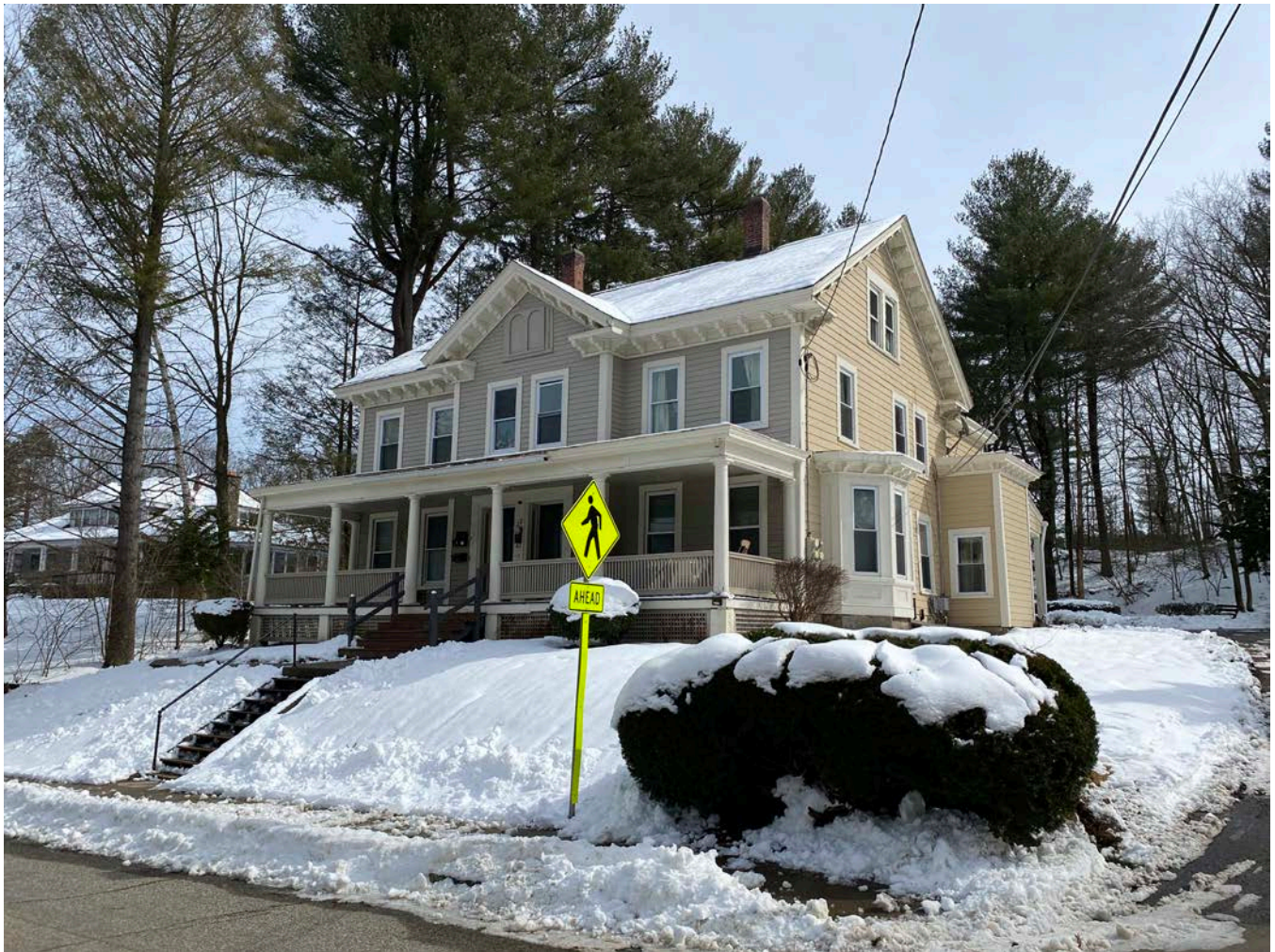
Photo 68 of 99. View of 28 Highland Terrace, looking east.
