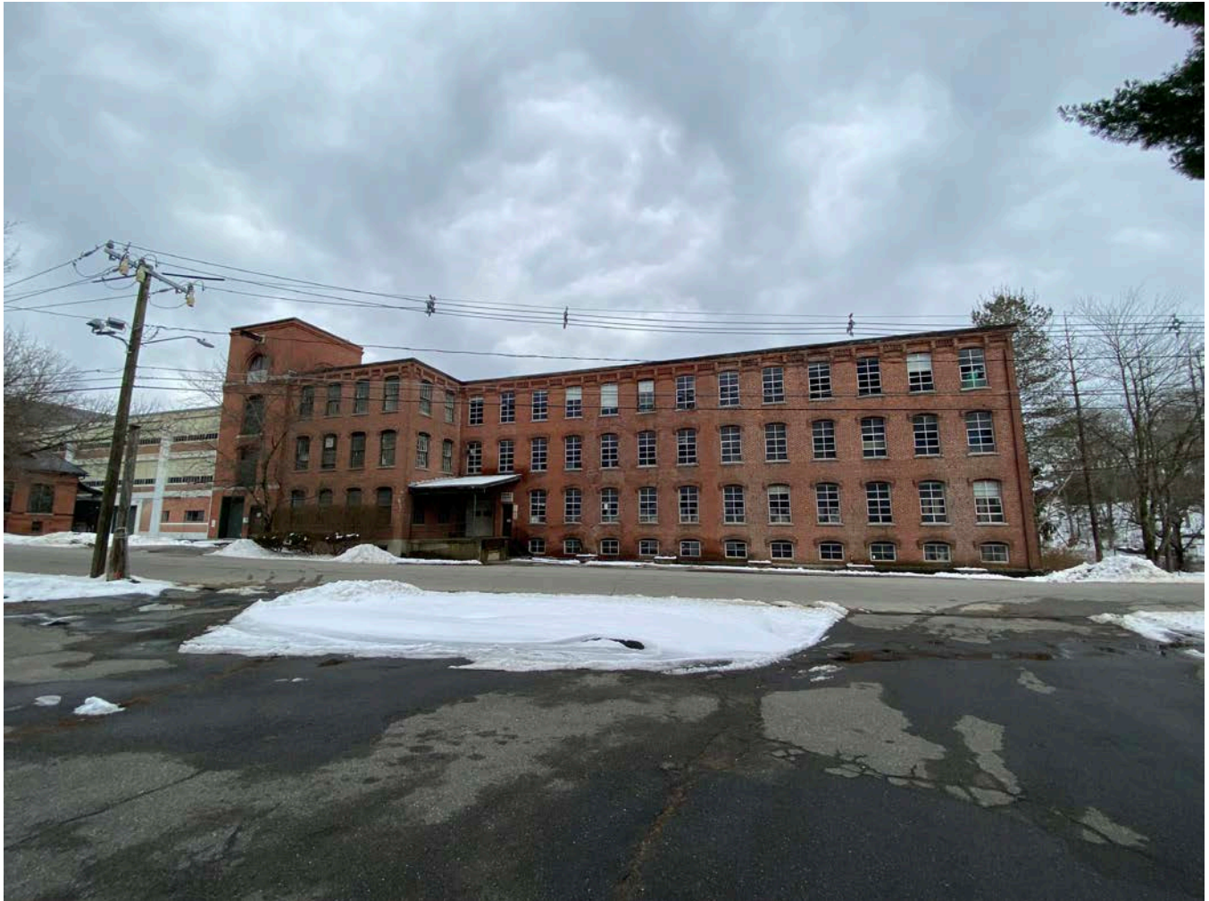
Photo 5 of 99. View of 29 Furnace Avenue, looking east.
