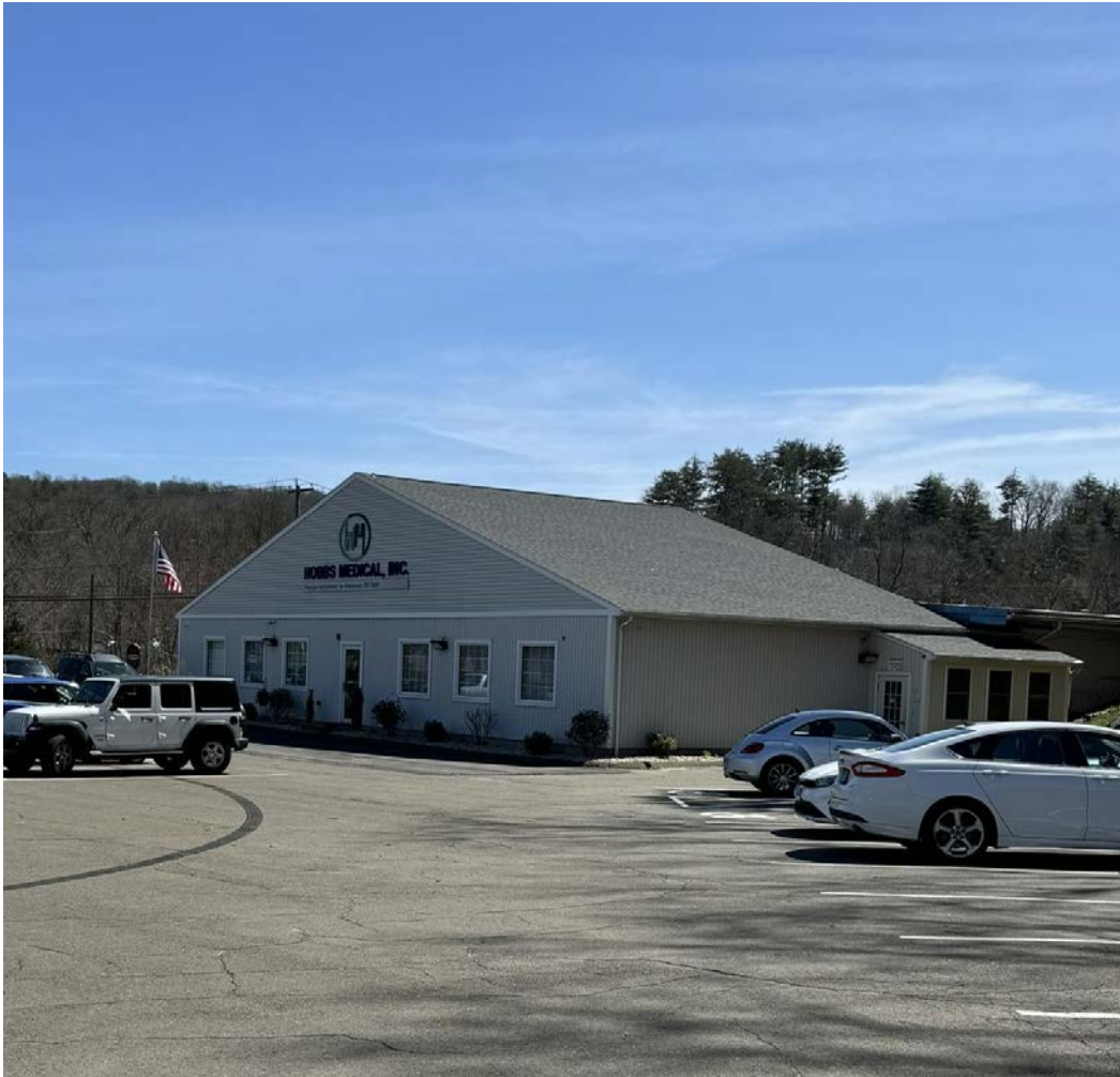
Photo 96 of 99. View of 8 Spring Street, looking south-southeast.
