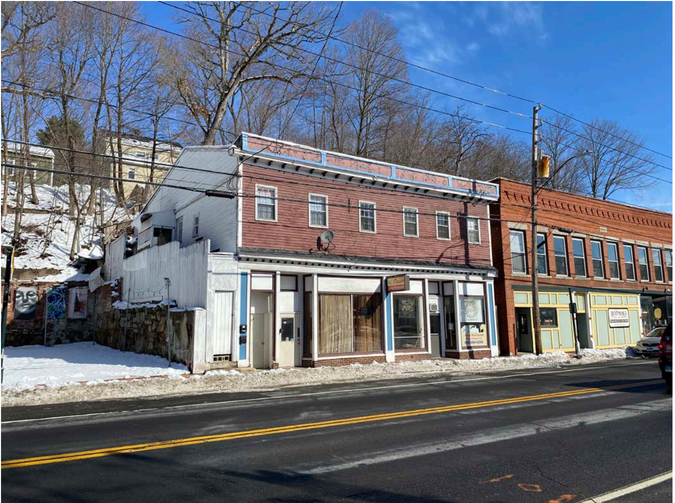
Photo 44 of 99. View of 29 Main Street, looking northeast.
