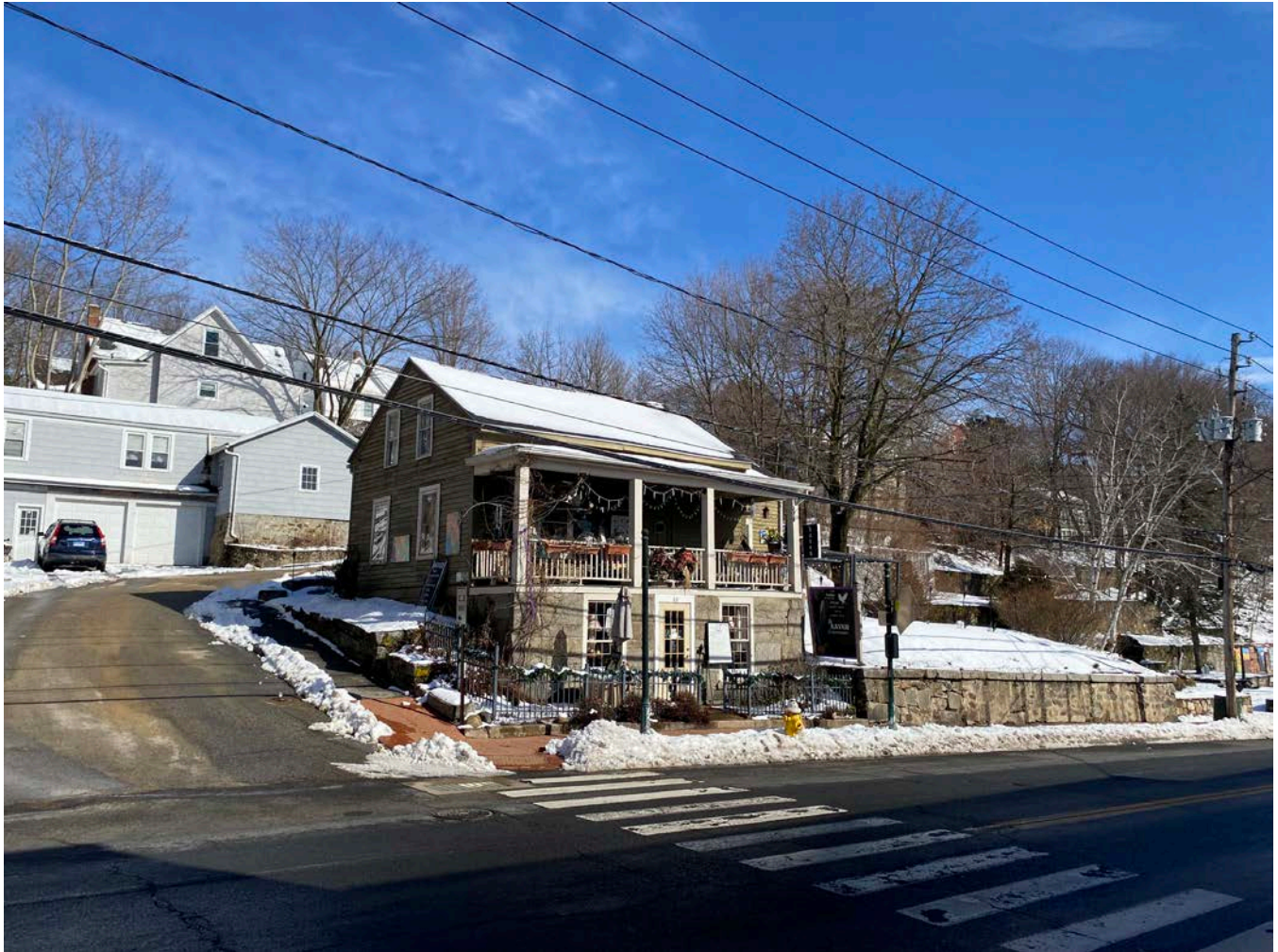
Photo 38 of 99. View of 63 Main Street, looking northeast.
