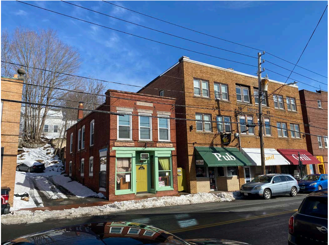
Photo 33 of 99. View of 81-83 Main Street, looking north-northeast.
