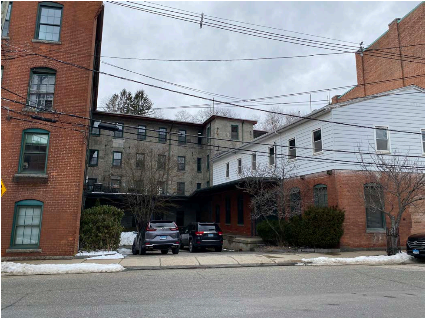
Photo 16 of 99. View of 8 Furnace Avenue (Original "Main" Mill), looking west.
