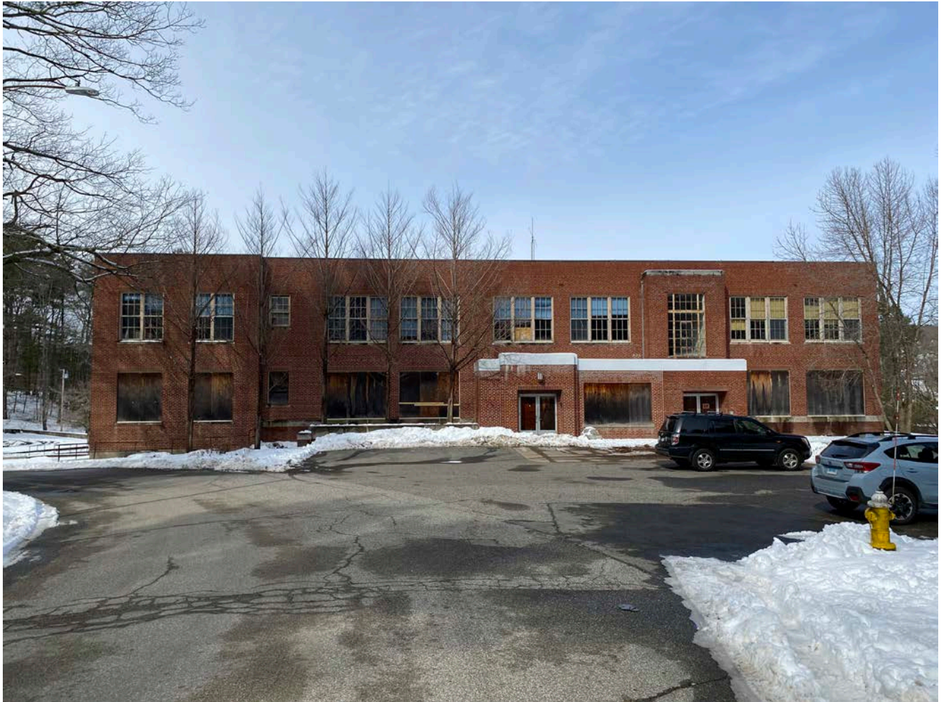
Photo 88 of 99. View of the Earl M. Witt School, looking east-northeast.
