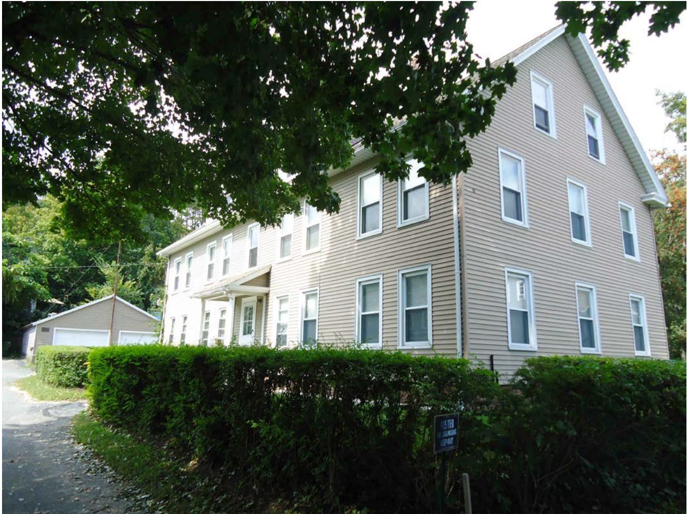
Photo 9 of 99. View of 18 Furnace Avenue, looking northwest.
