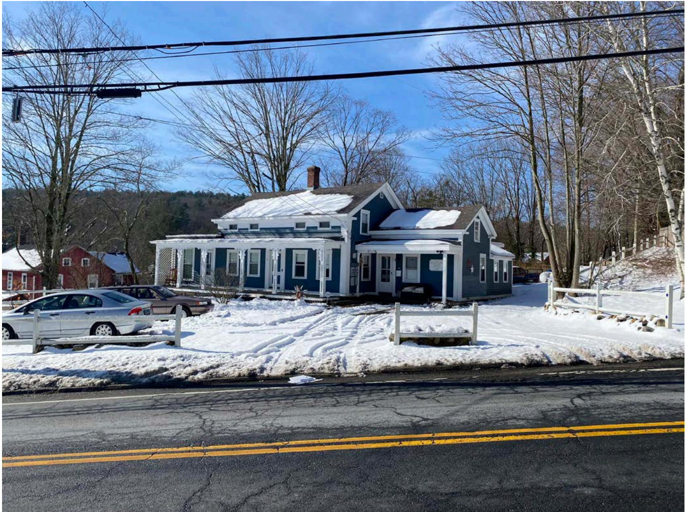
Photo 24 of 99. View of 6 West Main Street, looking west-southwest.
