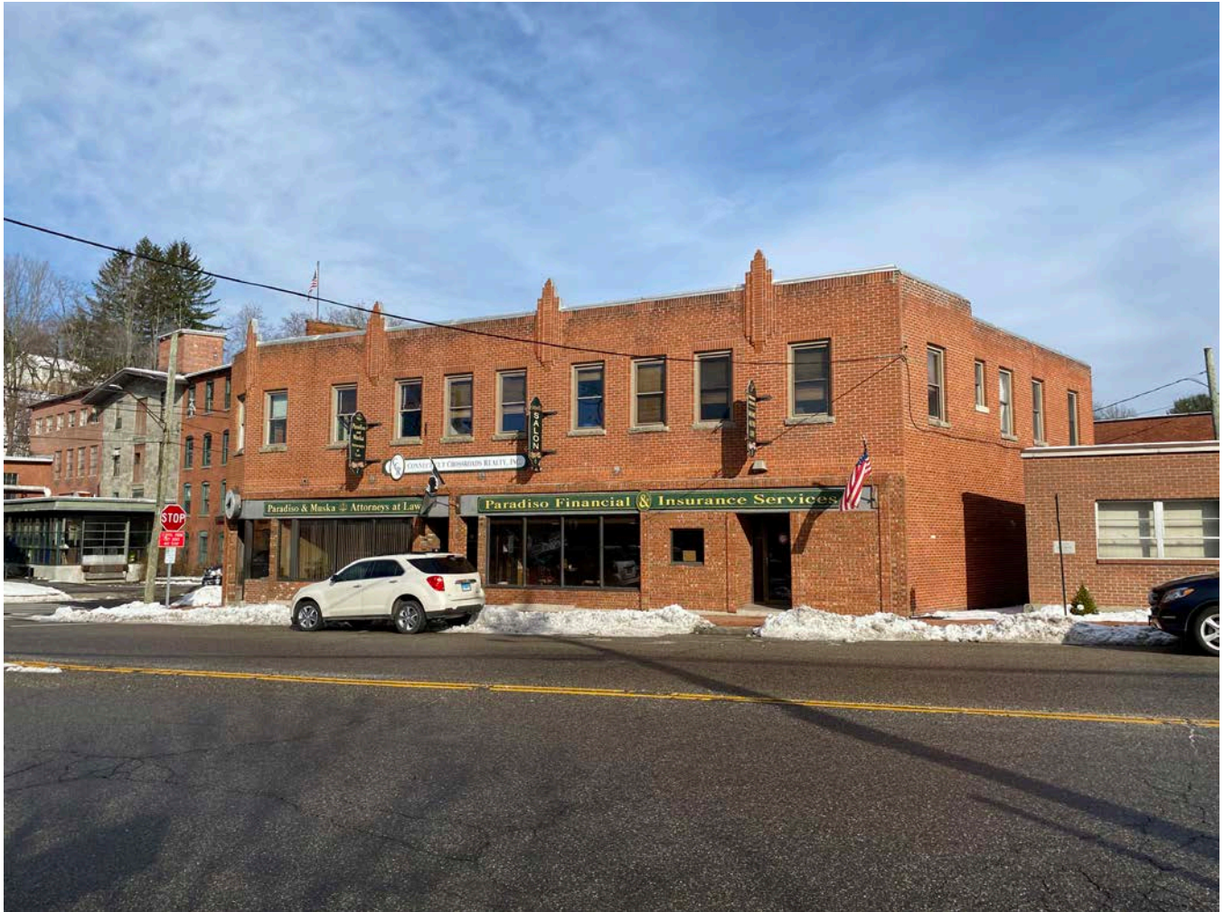
Photo 19 of 99. View of 2-8 East Main Street, looking north-northwest.
