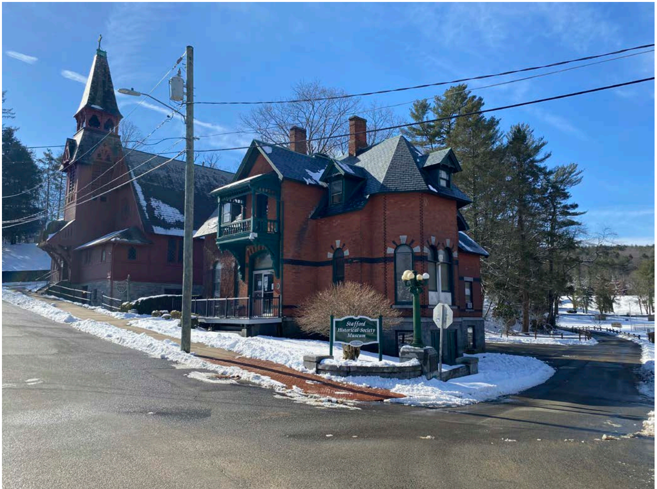
Photo 61 of 99. View of 5 Spring Street, looking southwest.
