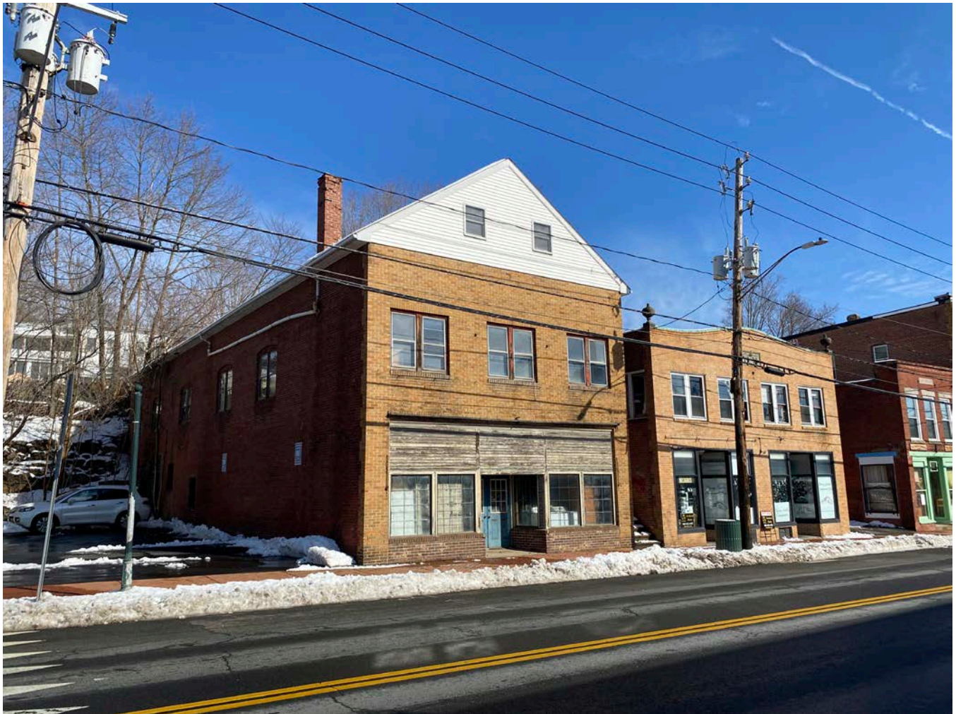
Photo 29 of 99. View of 87 Main Street, looking north-northeast.
