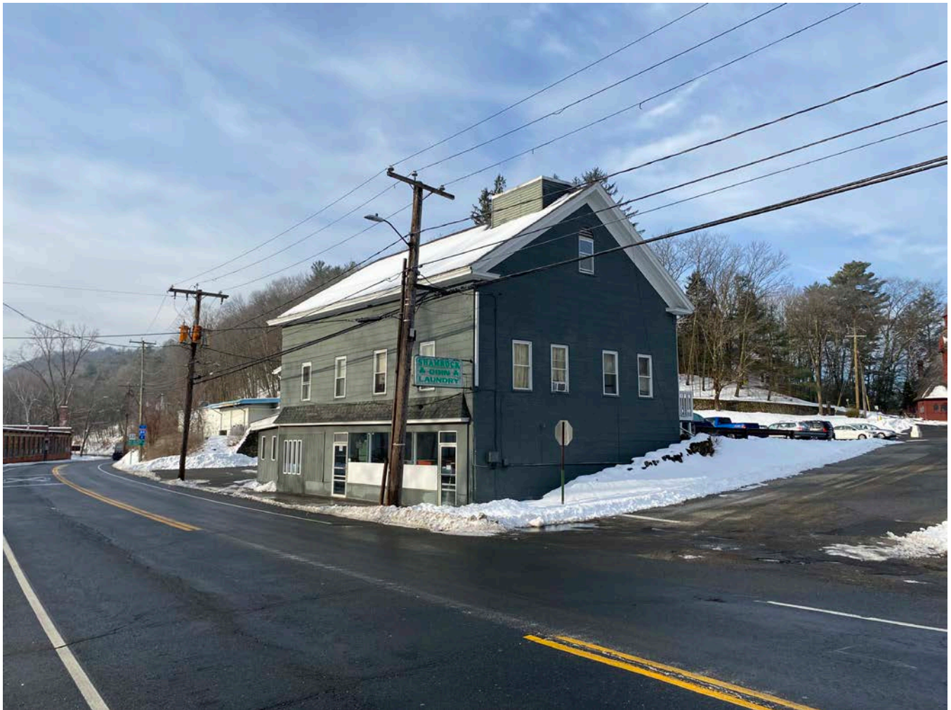
Photo 94 of 99. View of 9 River Road, looking southwest.
