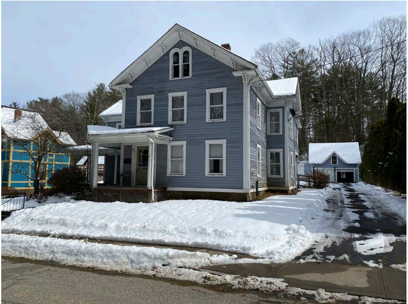
Photo 73 of 99. View of 52 Highland Terrace, looking east.
