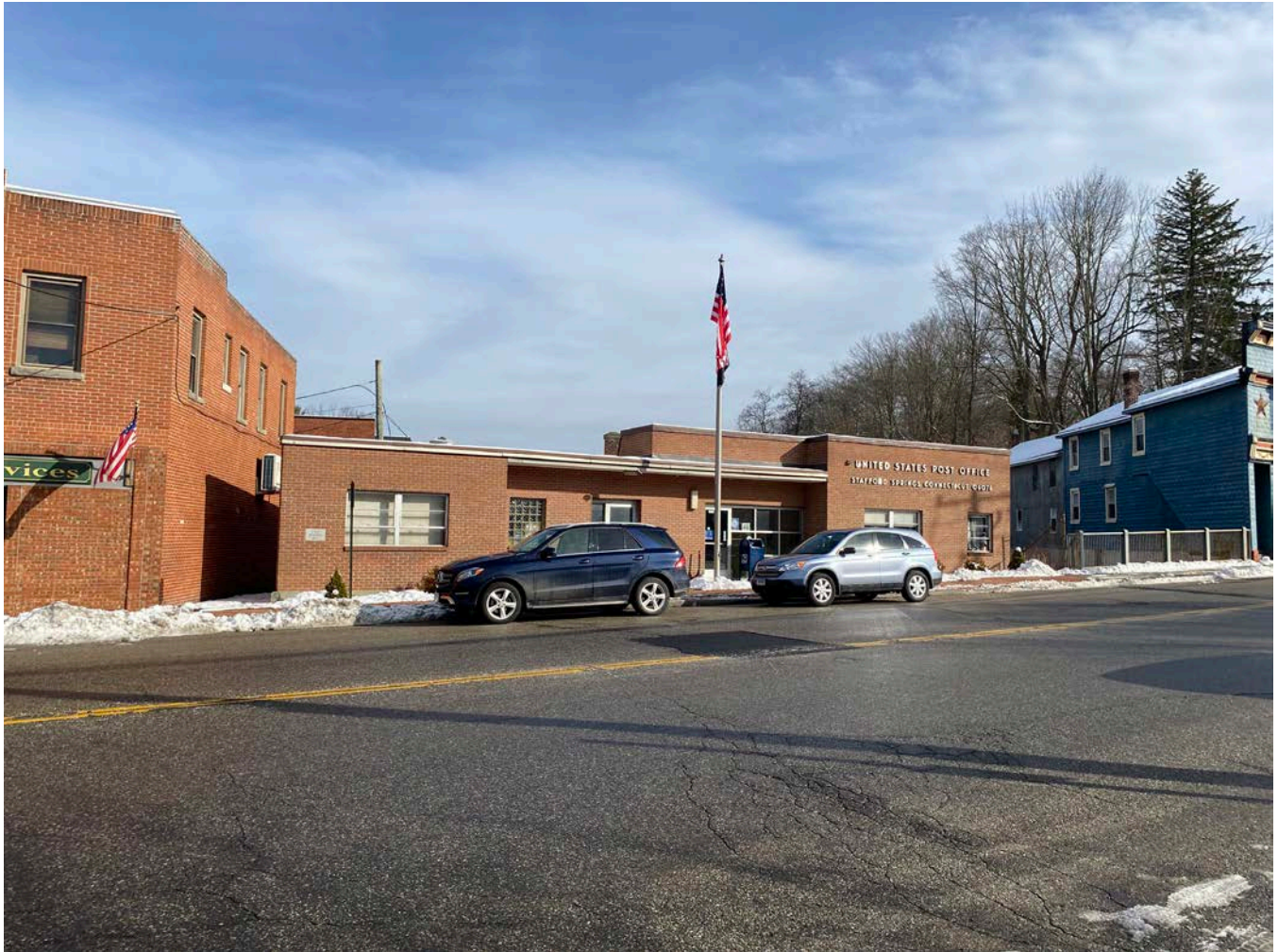
Photo 20 of 99. View of 14 East Main Street, looking north-northeast.
