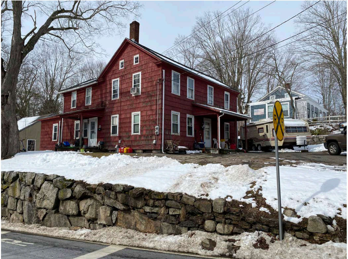
Photo 26 of 99. View of 1 Tolland Avenue, looking northwest.
