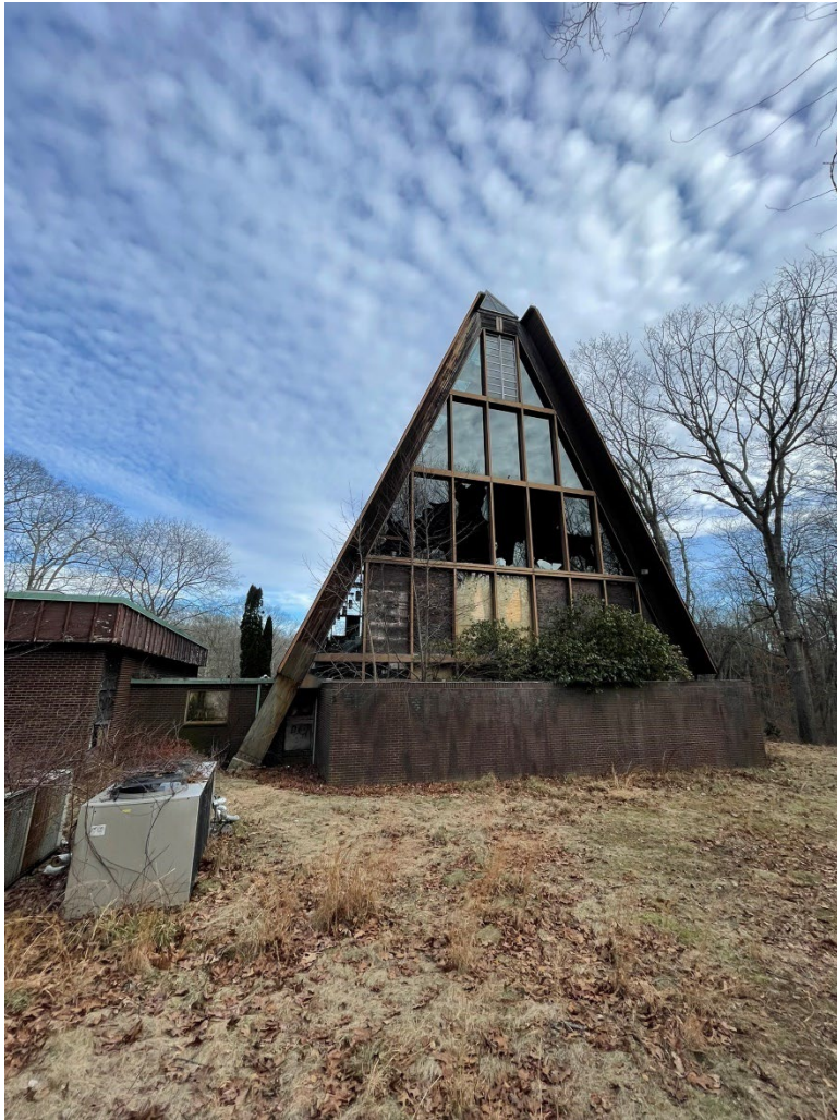
Photograph 8. Western elevation, view east.
