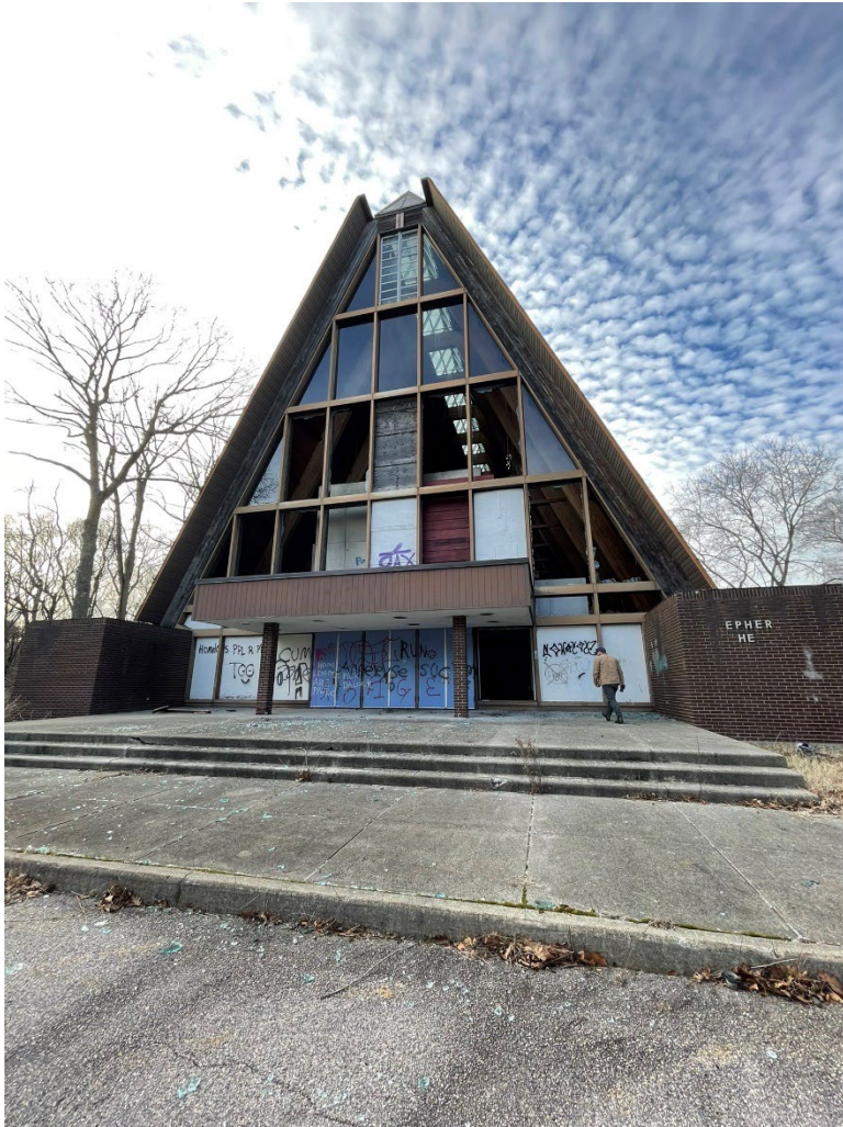
Photograph 5. Façade (eastern elevation of Chapel, view west.
