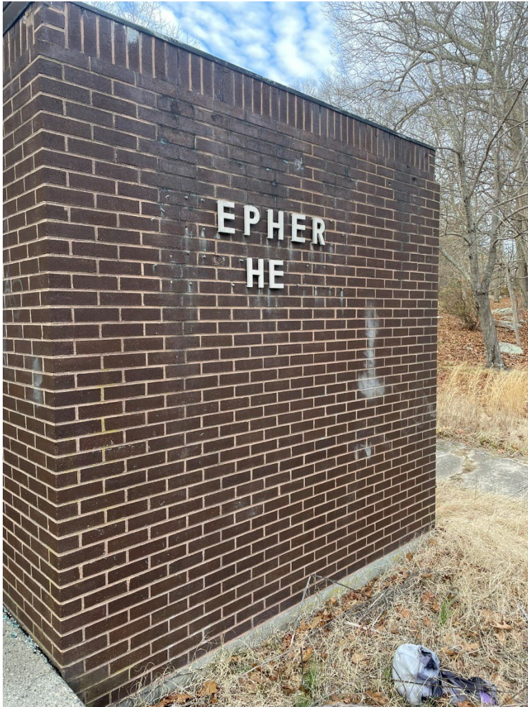
Photograph 6. Brick end wall on north side of entrance, view northwest.
