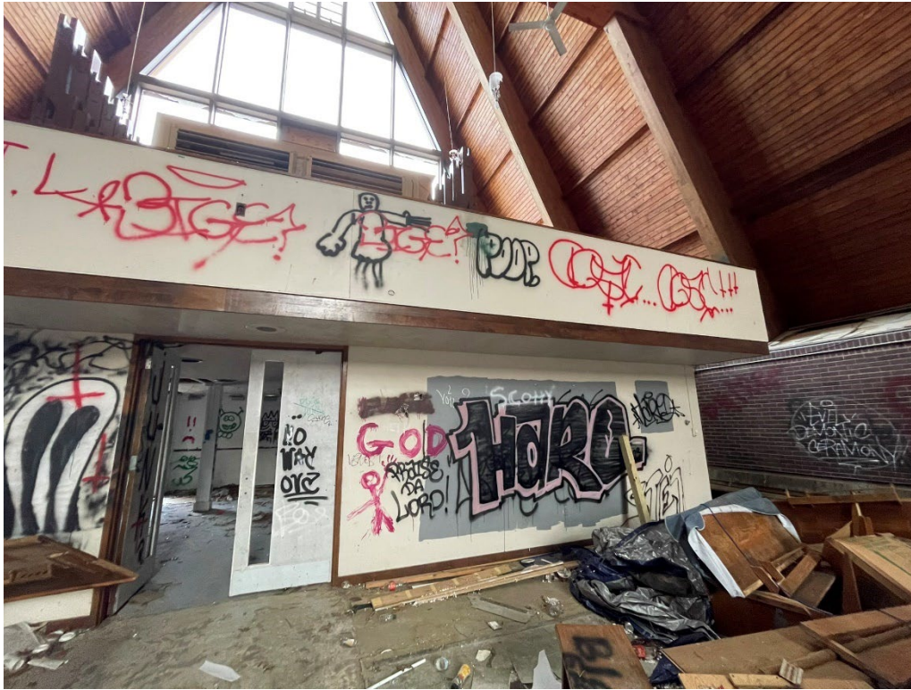
Photograph 15. Detail of the balcony and narthex/entry, view southwest.
