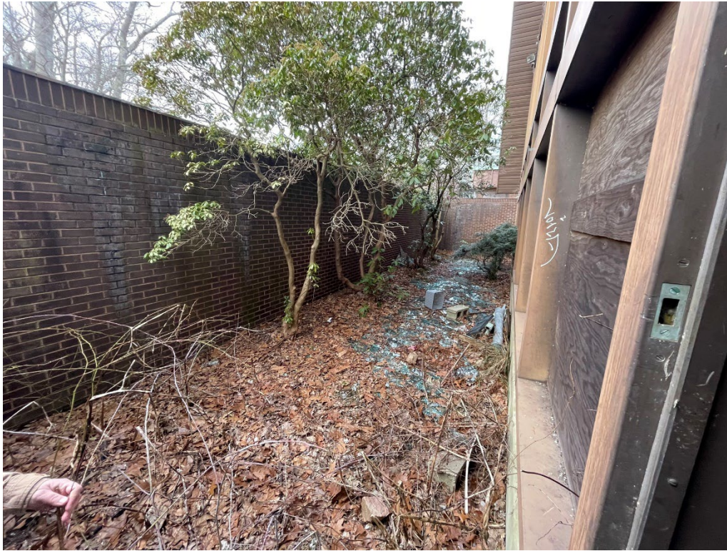
Photograph 7. Walled garden at the rear (west) of the building, view north.
