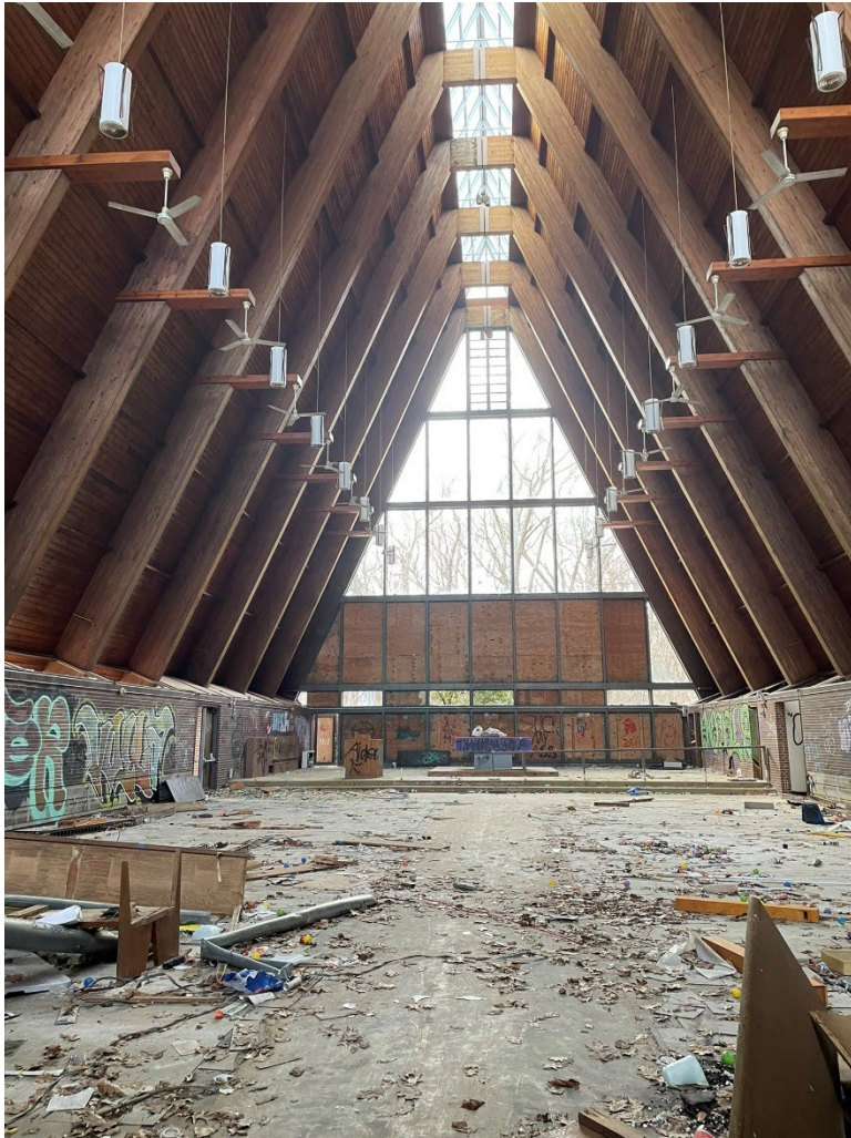
Photograph 12. Interior of the building facing the alter, view west.
