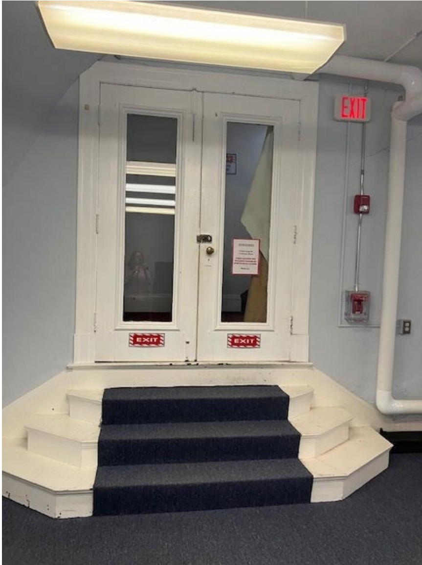
Photograph 33. Steps leading to stairwell, view southwest.
