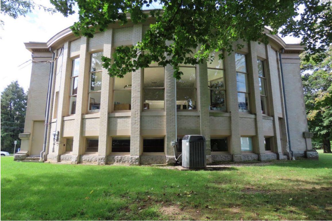
Photograph 7. Rear of the building, view west.
