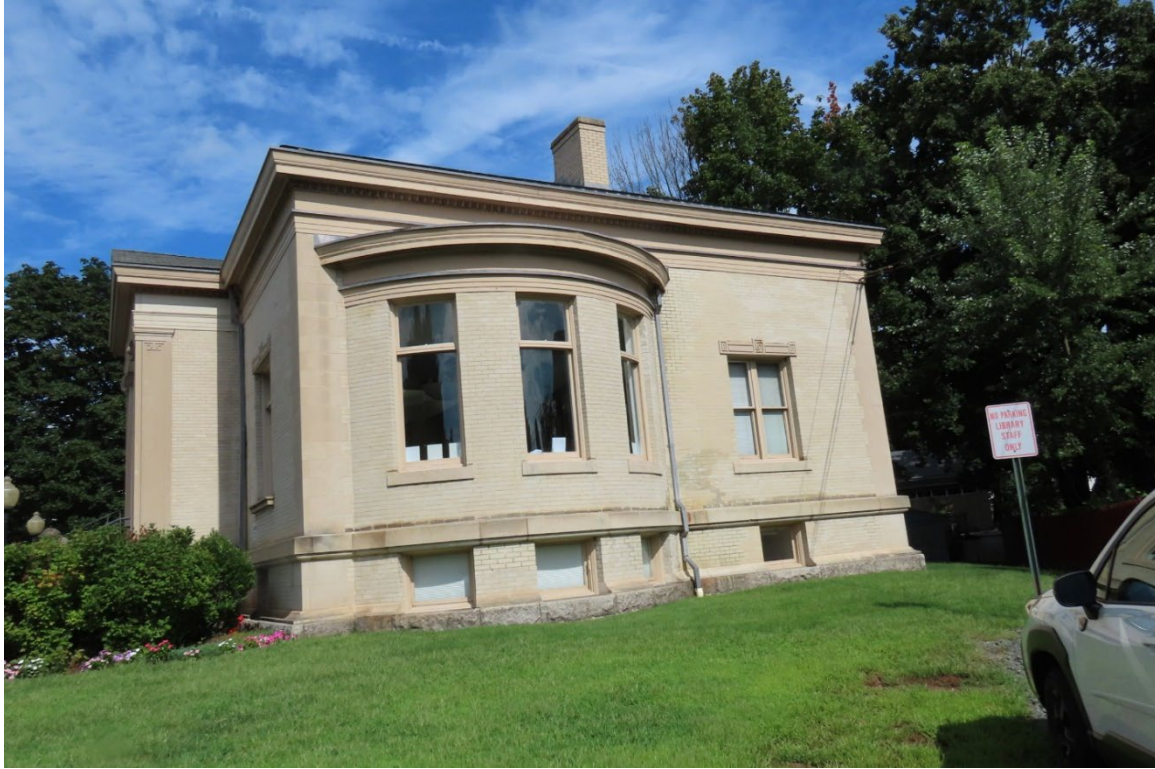
Photograph 5. Southern elevation, view north/northeast.
