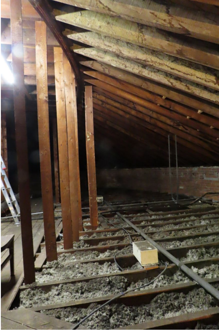
Photograph 25. View in attic looking east.
