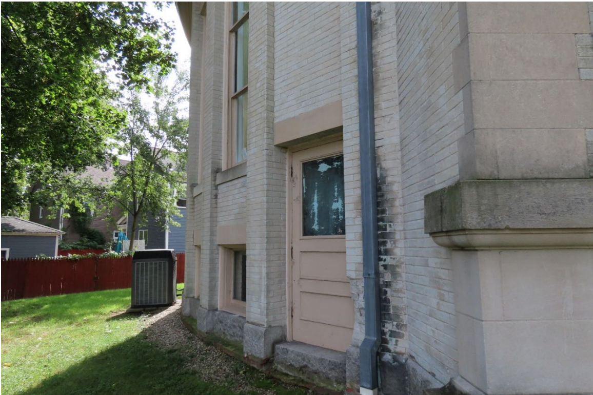
Photograph 8. Entrance to ground level on northwest corner, view south.
