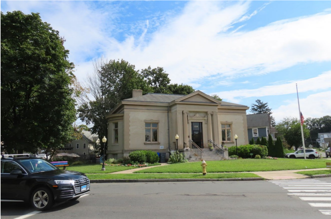
Photograph 1. Enfield Carnegie Library, view east.
