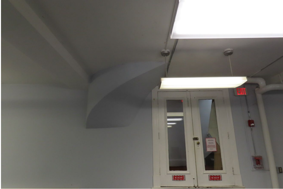
Photograph 34. View southwest showing the curved stairway leading to the second story.
