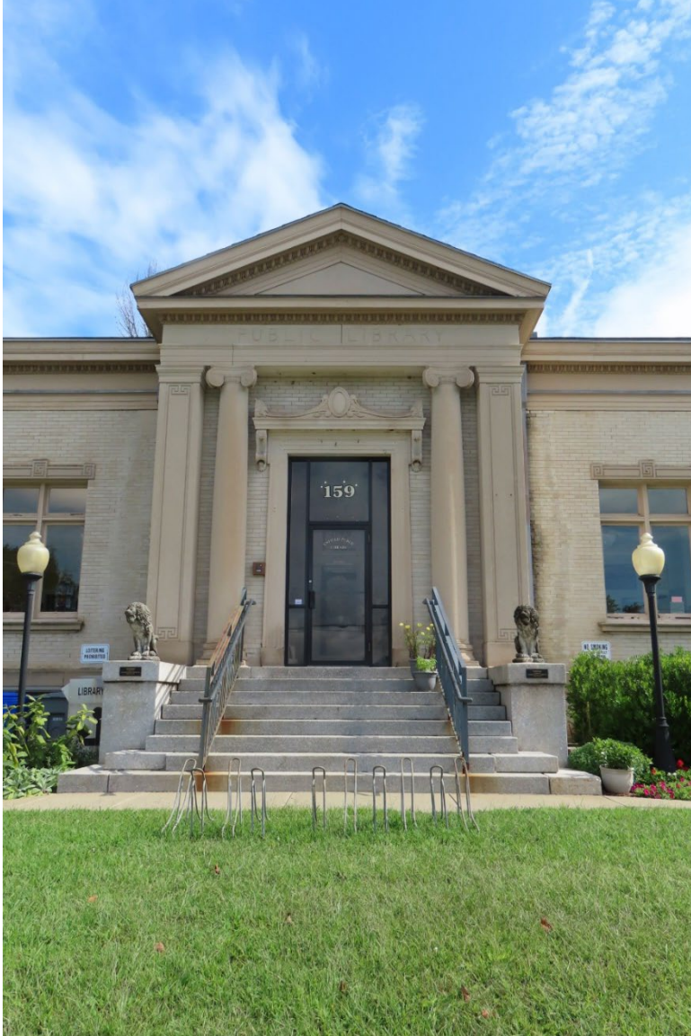
Photograph 3. Detail of portico, view northeast.
