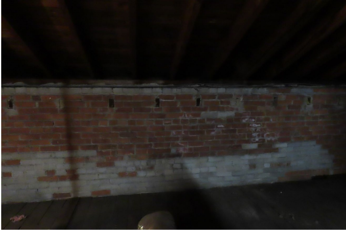
Photograph 26. View southwest in attic of knee wall.
