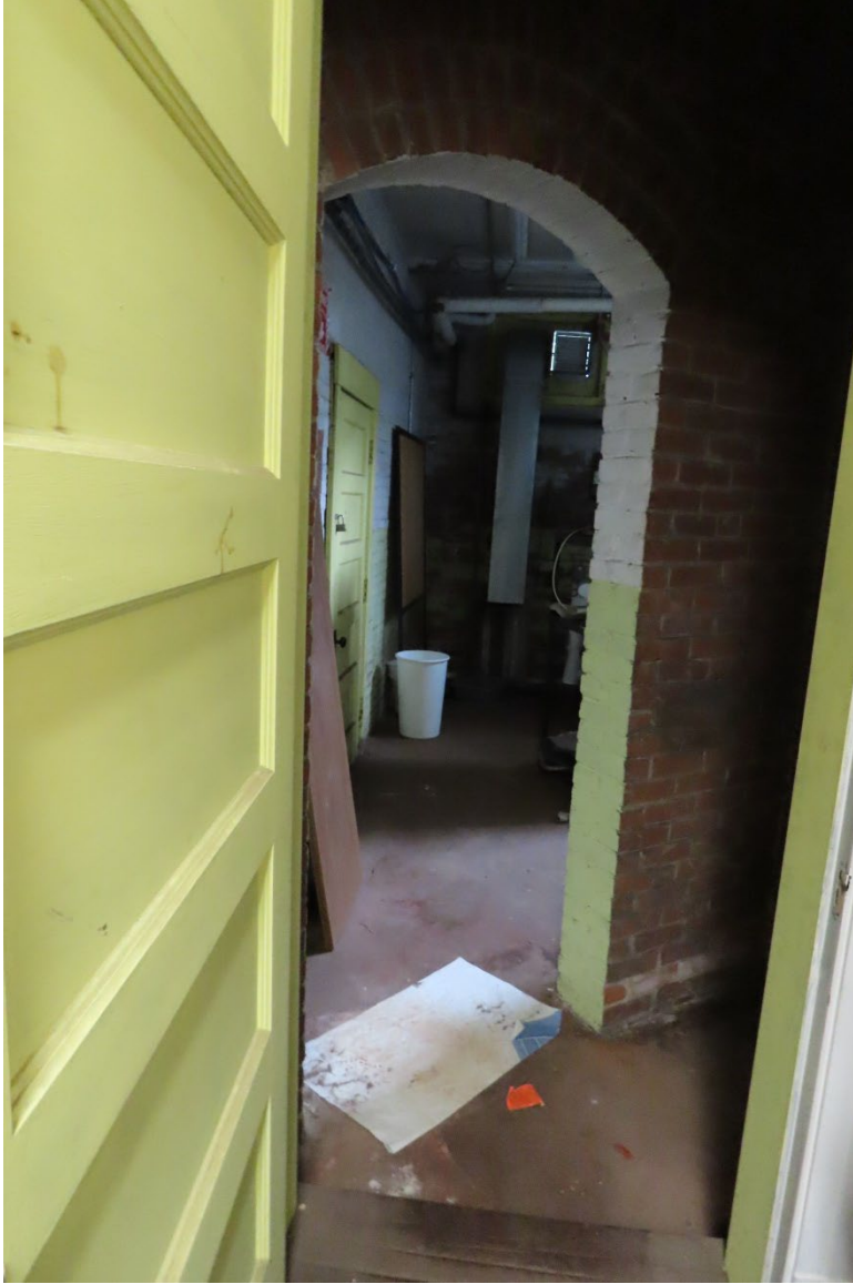
Photograph 29. Arched opening leading to storage, view northeast.
