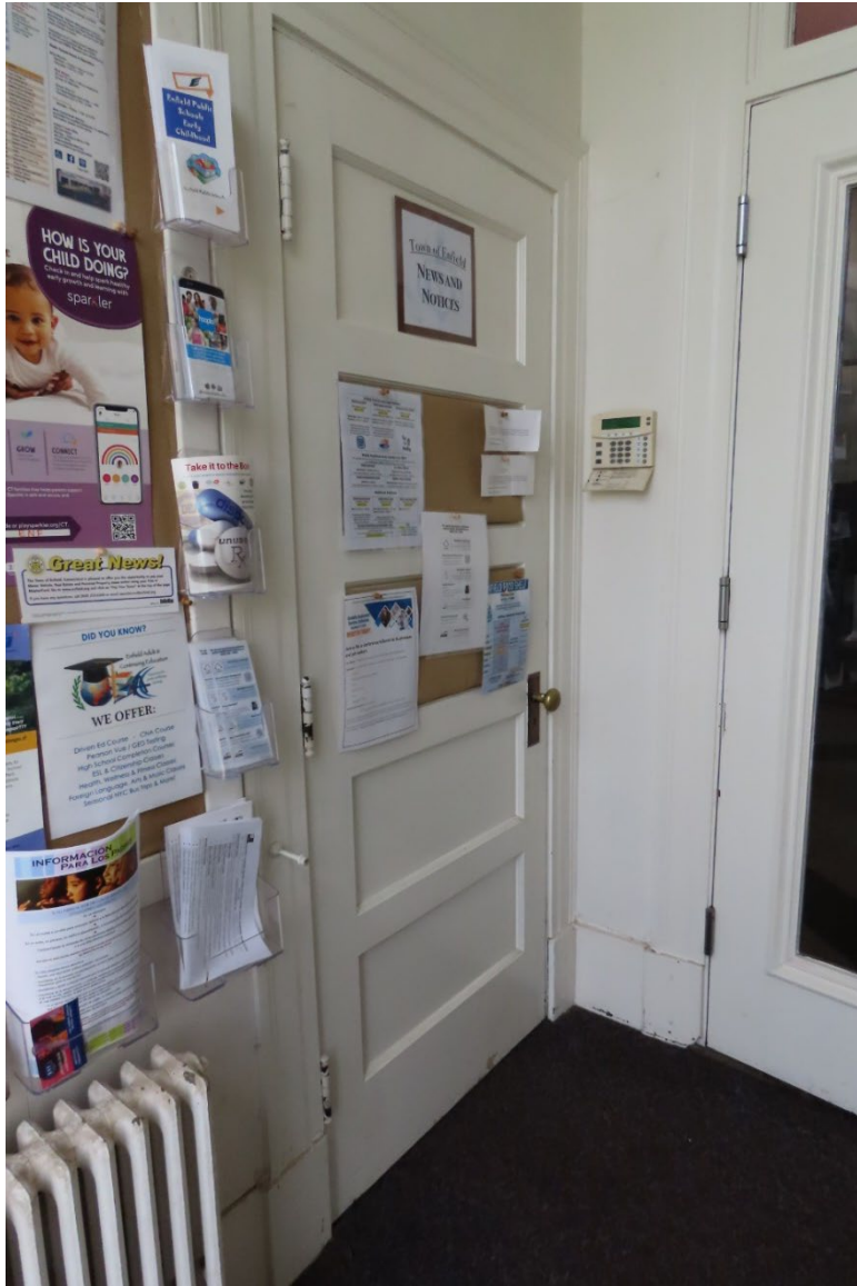
Photograph 12. Door leading to basement, northwest.
