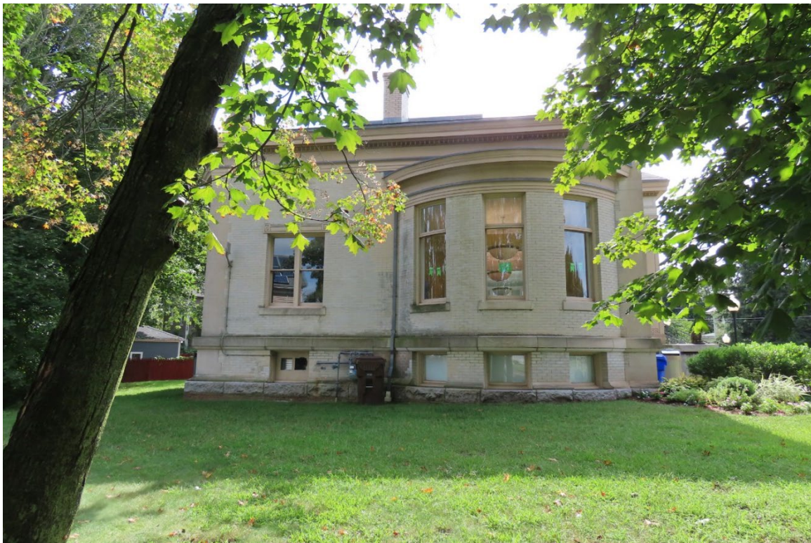
Photograph 6. Northern elevation, view south.
