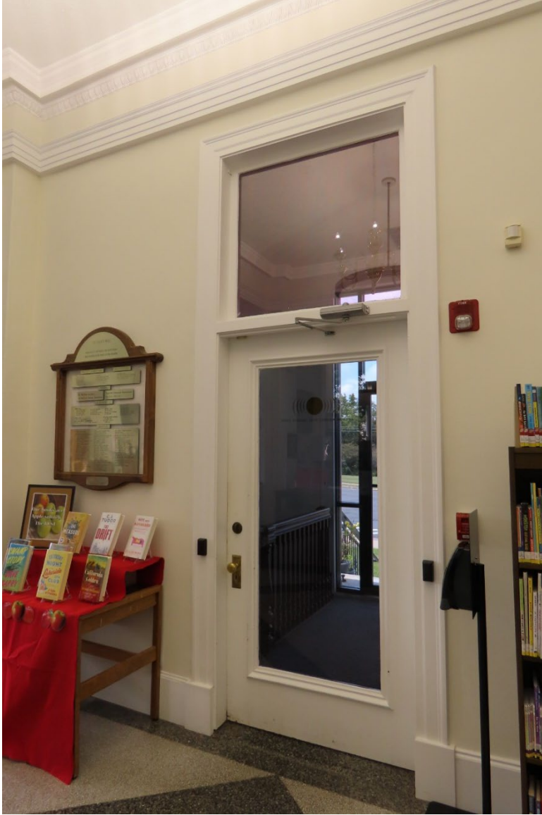
Photograph 14. Door to vestibule, view southwest.
