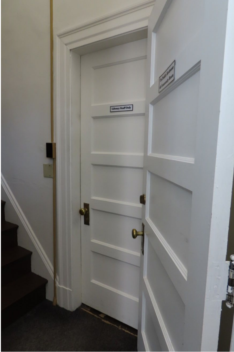
Photograph 23. Stairwell leading to attic, view southwest.
