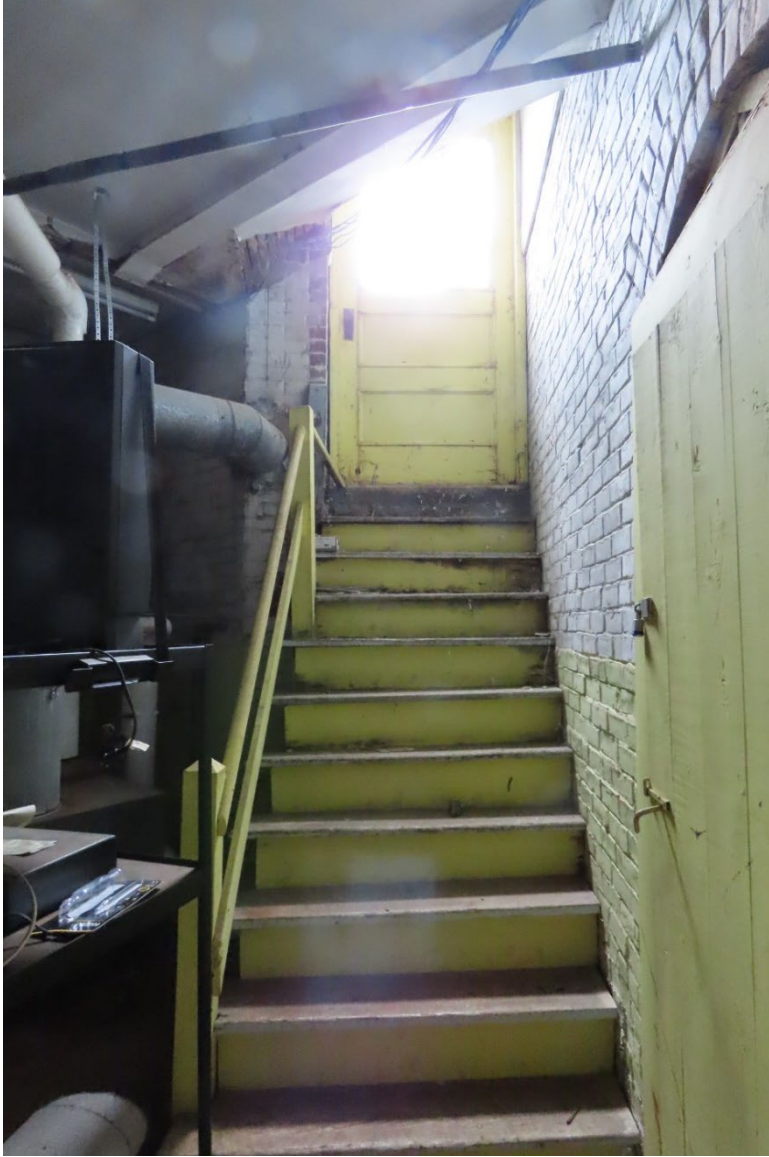
Photograph 32. Stair leading to exterior, view northeast.
