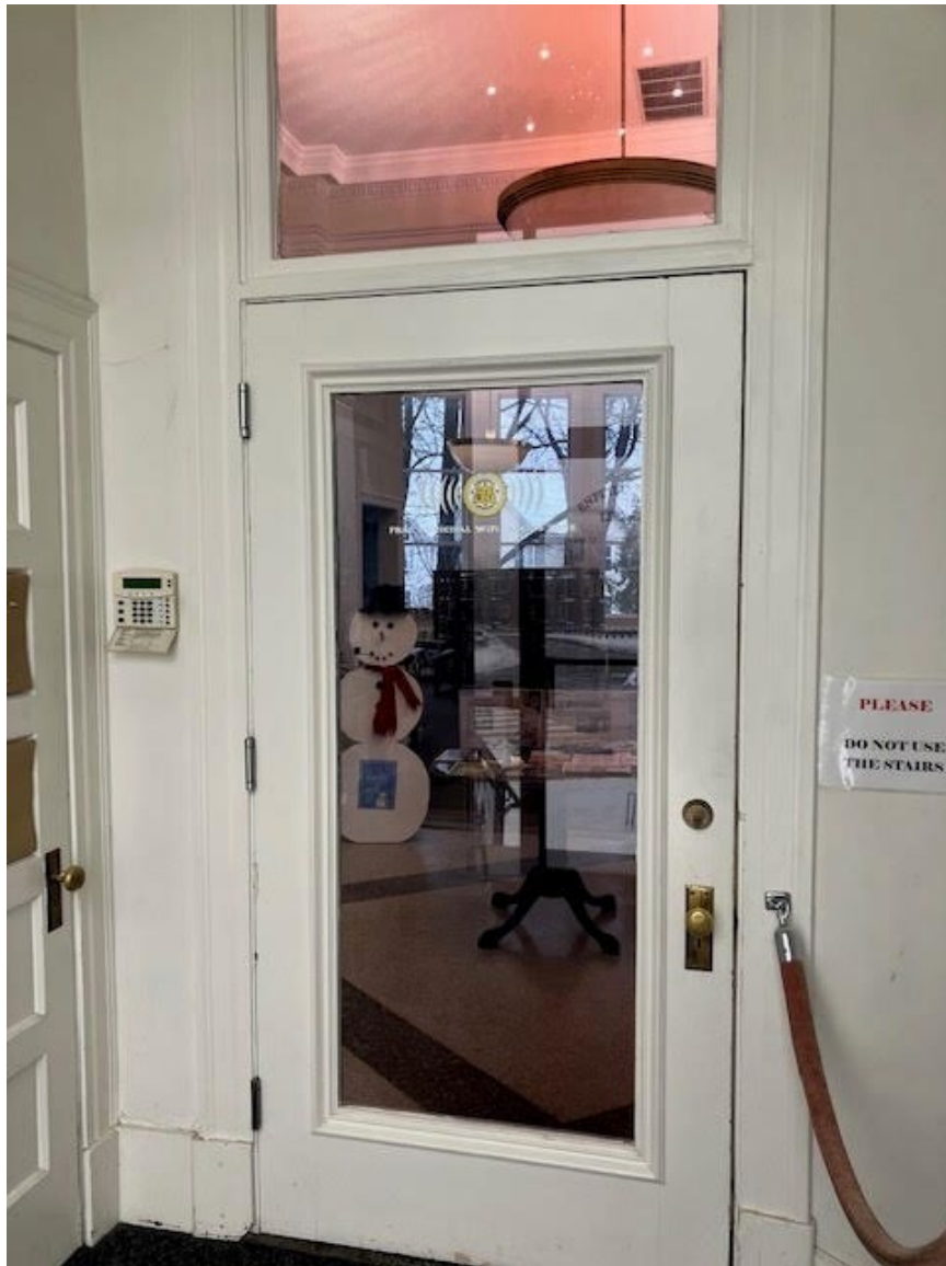
Photograph 13. Door leading to circulation room, view northeast.
