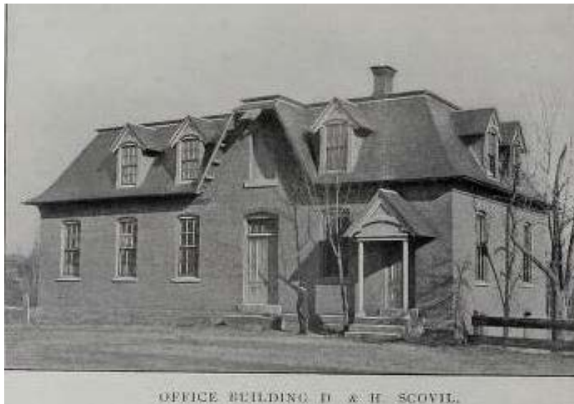
Figure 24. Photograph illustration of Office/Storage building in The Middletown Tribune Souvenir Edition , 1896.
