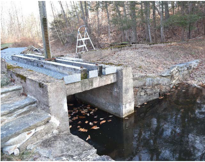
Photographs 35 & 36. Modern headgate for reservoir canal within stone wall structure; camera facing northeast (L), downstream side of headgate; camera facing southwest (R).
