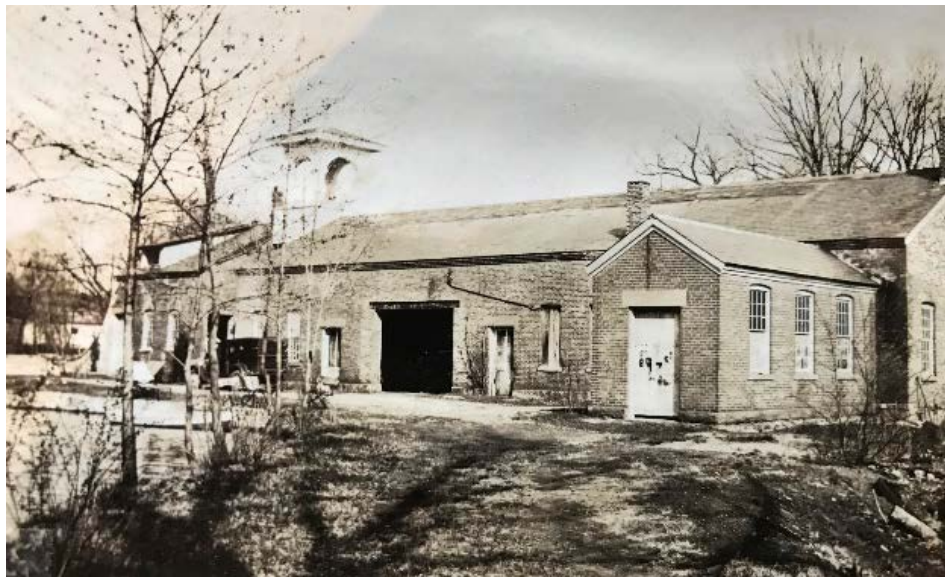
Figure 20. Photograph of north elevation of Mill #2, after demolition of most of eastern block, c.1935-40. Benham photo album.
