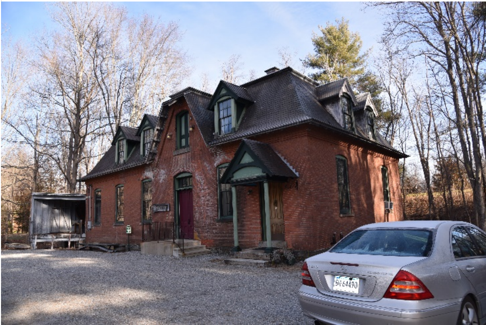
Photograph 66. West elevation with entrance to storage and loft door at center and office entry at right; camera facing east.
