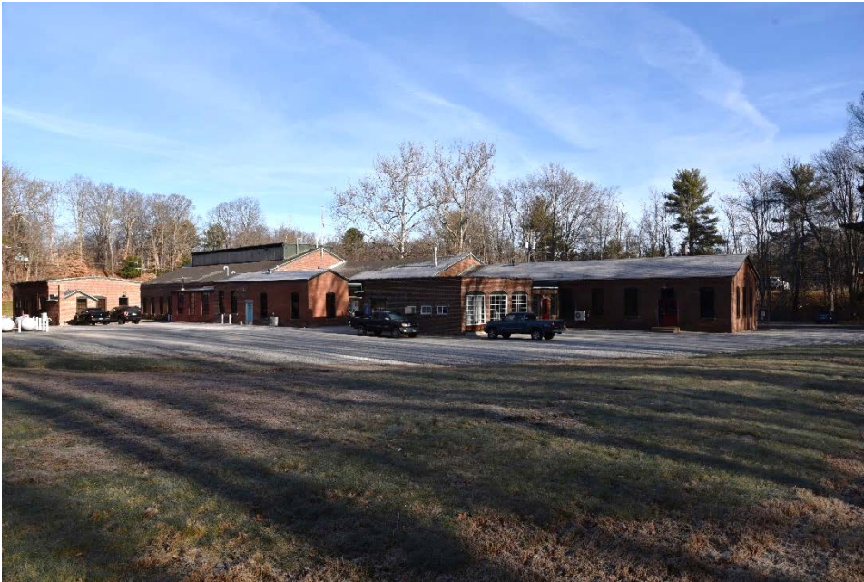
Photograph 43. Rear/west elevation of complex; camera facing northeast.
