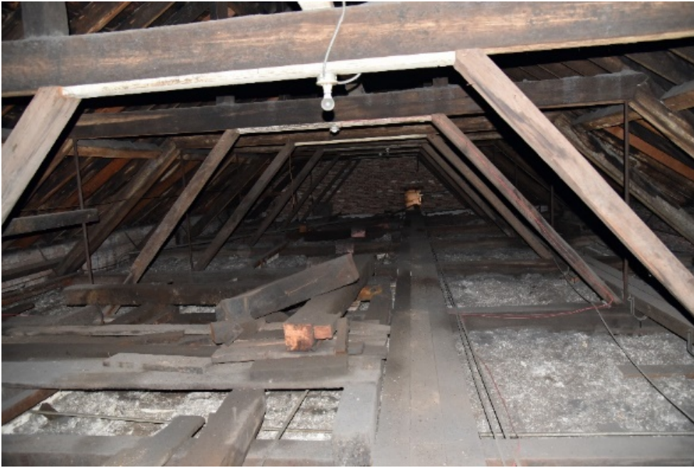
Photographs 108 & 109. Truss system and brick fire wall in background (L), and monitor truss (R).
