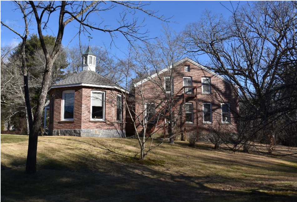
Photograph 17. West elevation with chapel addition off ell at left; camera facing northeast.
