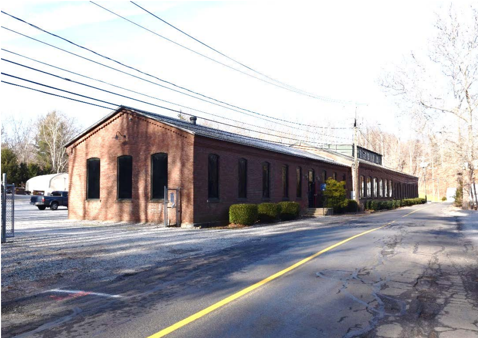
Photograph 42. South and front/east elevations of Mill #3 complex along Scovil Road; camera facing north/northwest.
