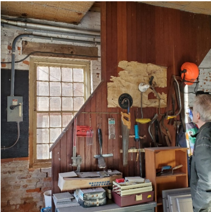
Photograph 26. A vertical bead board stair leads to second level.
