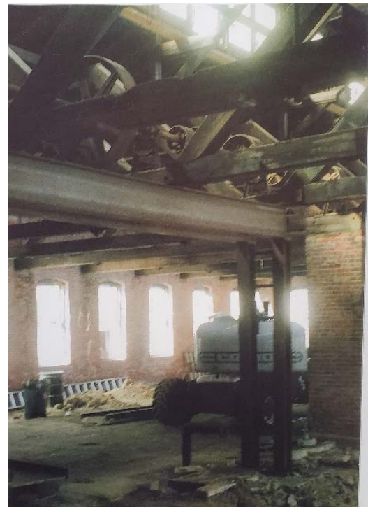
Figure 30 a & b. a. Interior of Polish Room showing the metal truss system in c.1905 extension. b. belt and pulley system in forge block. Photographs taken by Ronald Denmam c.2005 after purchase Mill #3 and the Office/Storage properties.
