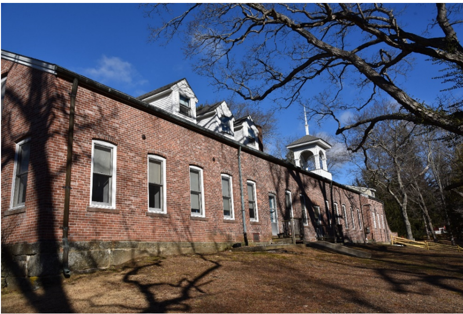
Photograph 18. South elevation; camera facing northeast.
