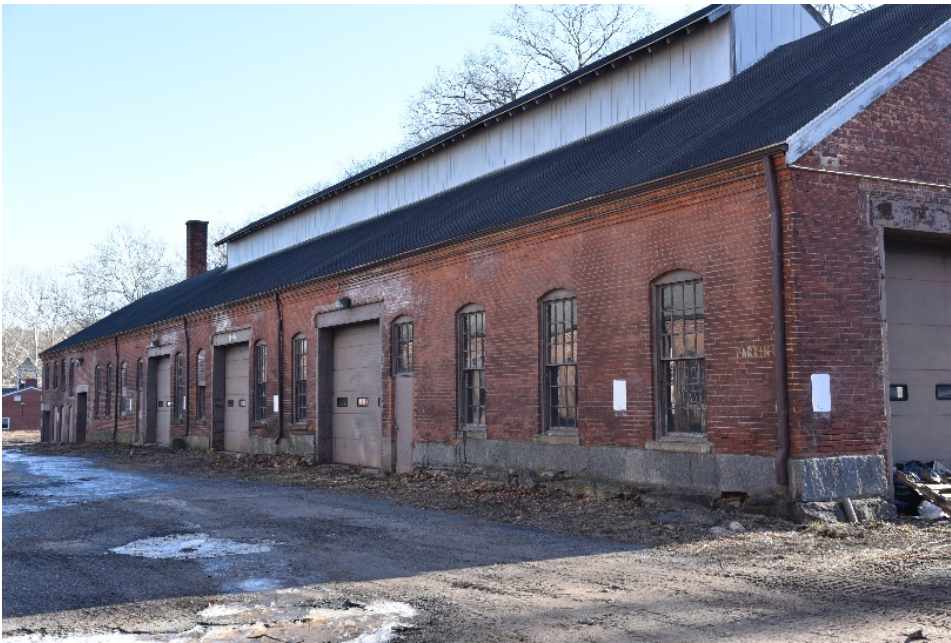
Photograph 80. North elevation of c.1889 forge shop, camera facing east.
