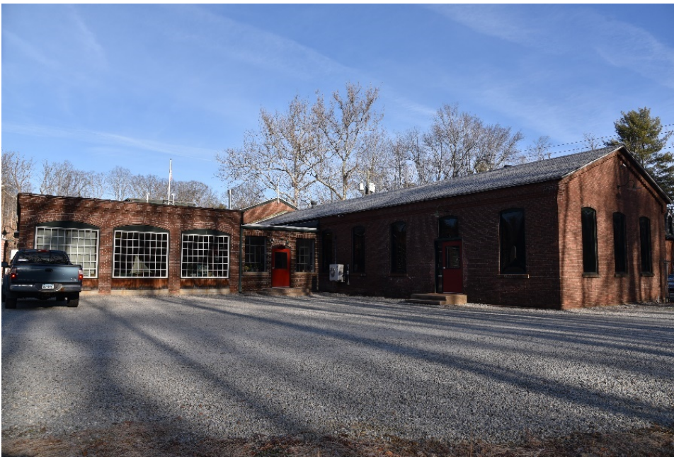
Photograph 44. From left: south elevation of auto house, connector to japan house, west and south elevations of japan house.
