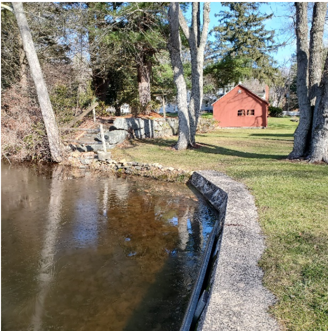
Photograph 14. Concrete wall section generally corresponds to the location of the former head race intake for the turbine. Granite block retaining wall runs from the pond to the barn, which sits on the granite foundation of a former horse shed.
