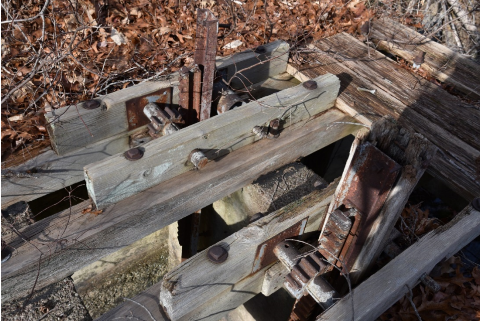
Photograph 2. Close-up of headgate mechanism.
