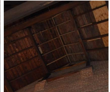
Photographs 90 & 91. Former engine room with elevated concrete floor and firewall at right (L). Detail showing extant monitor framing supported by brick corbels on fire wall (R).
