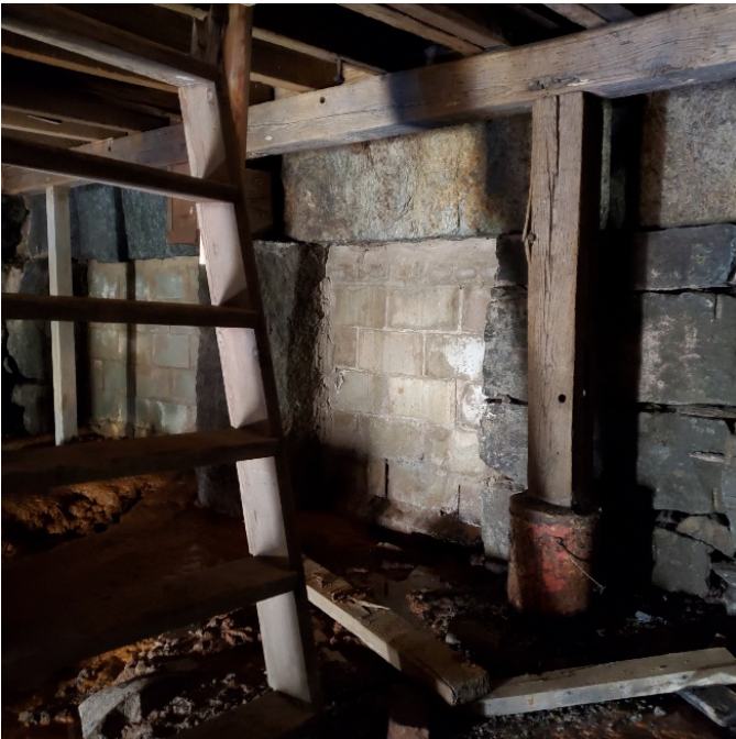
Photograph 31. Concrete block in north wall closing off head race; note large granite blocks to carry building across head race.
