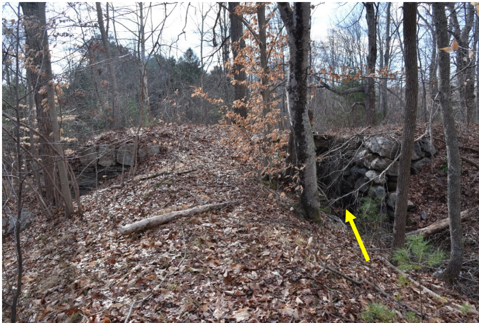
Photograph 1 of 109. Looking southwest from canal berm toward dam; canal and headgate at right. The dam wall, though shallow extends northward (to the right) some 60-70 feet; the wall to the south/left was the main face, some 50 feet above the brook bed and approximately 100 feet to the south/southeast. See also Figure 13.
