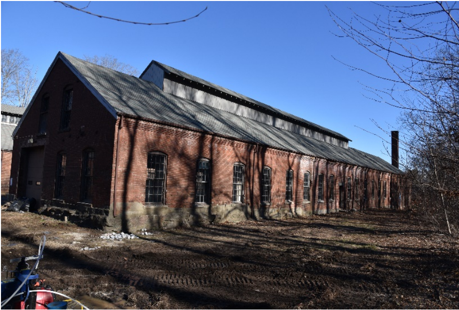
Photograph 82. West and south elevations of c.1889 forge shop; camera facing east. Openings on south wall, along brook, have not been altered.
