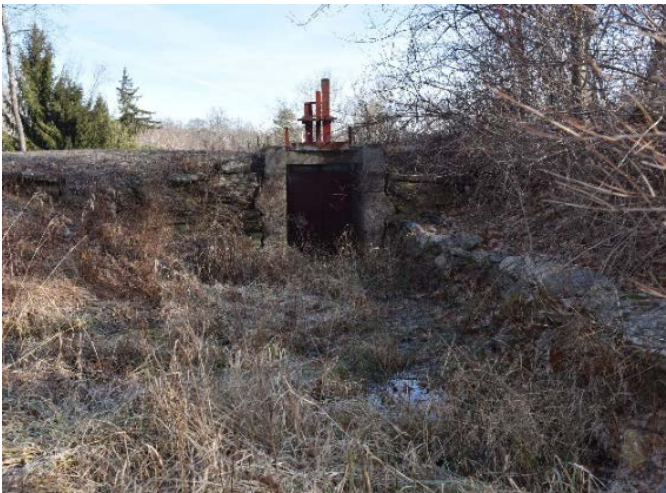
Photographs 39 & 40. Interior view of reservoir canal stone retaining walls and sluce gate at its east end (L), exterior of reservoir canal stone retaining walls; camera facing southwest (R).
