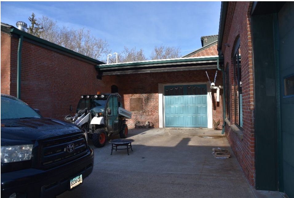
Photograph 46. From left: east elevation of engine block, south elevation of boiler block (with modern garage door), with west wall of polish room at R; camera facing north.
