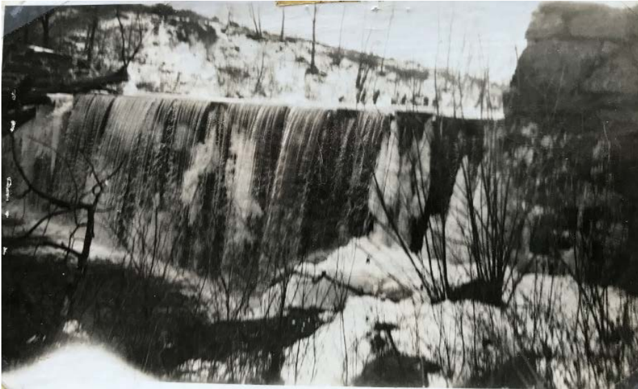
Figure 13. Photograph of dam at upper pond for Mill #1, c.1940. Benham photo album.
