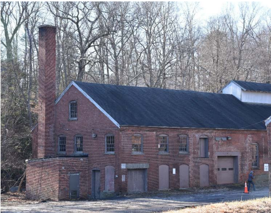
Photograph 81. East and south elevations of c.1889 forge shop; camera facing southwest. Garage door opens into former engine room.
