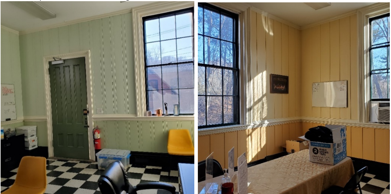
Photographs 68 & 69. Front office room and rear of paneled entry door (L); rear office room.
