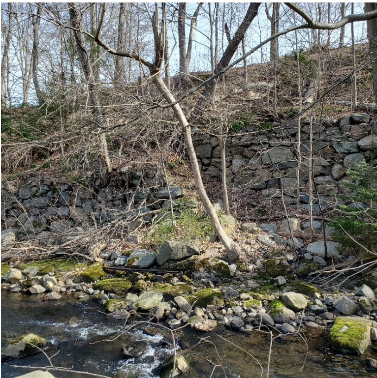
Photographs 76 & 77. Stone embankment wall on south side of brook where flume traveled (L) and stone pillars that carried the flume across the brook from the south bank to the 1886 mill (R) at non-contributing archaeological site at Mill #4.
