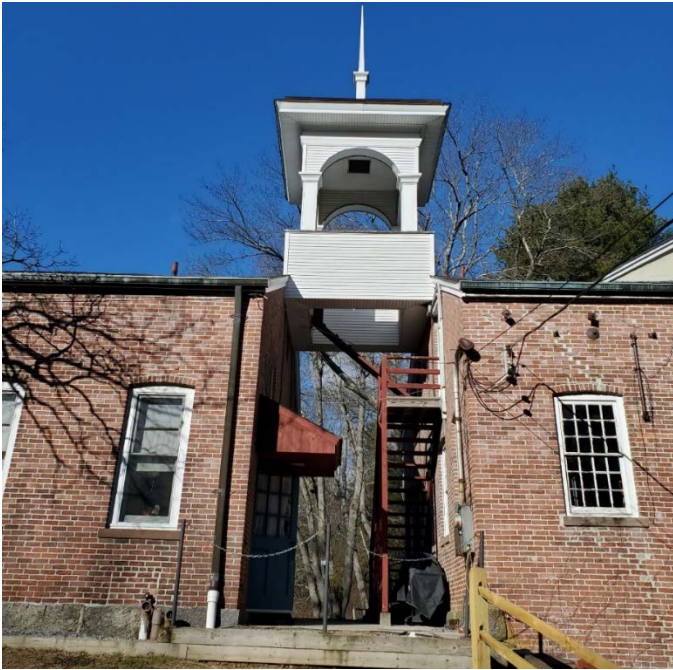
Photograph 19. Bell tower connection between blocks as seen on south elevation.
