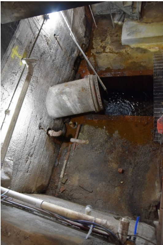
Photographs 55 & 56. Inside the engine block: partial view of turbine pit and outflow flume toward street (L), and power shaft coming off turbine (R).
