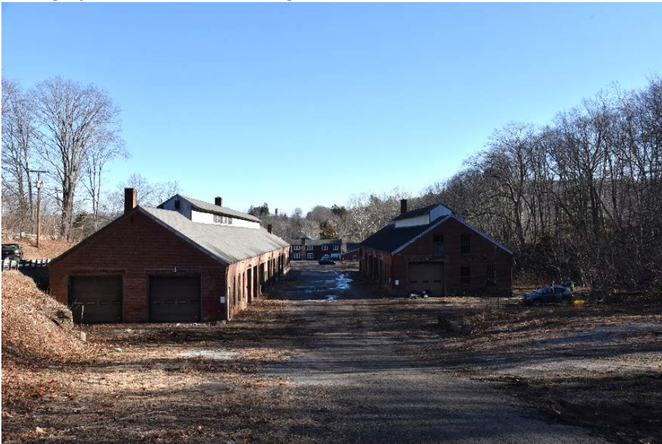
Photograph 79. The two forge buildings between Candlewood Hill Road to the left and the brook to the right; camera facing east from the location of former mill pond.
