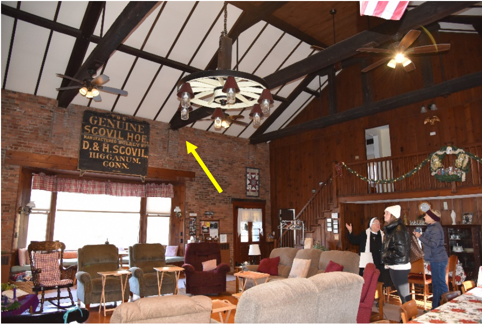
Photograph 21. Interior of center space in western block; note how trusses sits on brick corbels in the load bearing brick walls.
