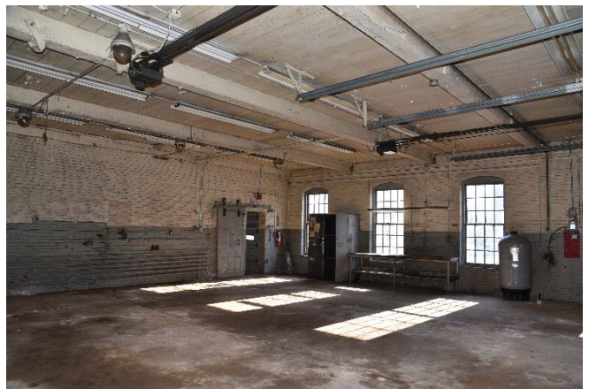
Photographs 102 & 103. Open workspace adjacent to office: camera facing west (L) with another brick firewall in background, and camera facing east (R) with non-structural mid-20 th century wall creating added office space at east end adjacent to office. Ceiling has same treatment as office.
