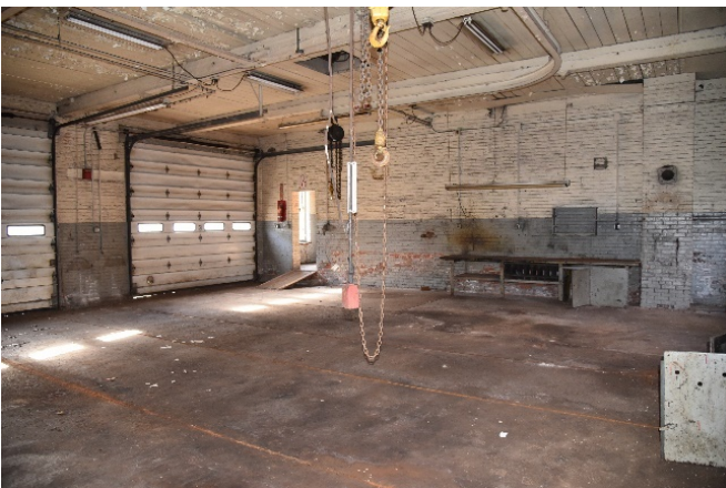
Photographs 102 & 103. Open workspace adjacent to office: camera facing west (L) with another brick firewall in background, and camera facing east (R) with non-structural mid-20 th century wall creating added office space at east end adjacent to office. Ceiling has same treatment as office.
