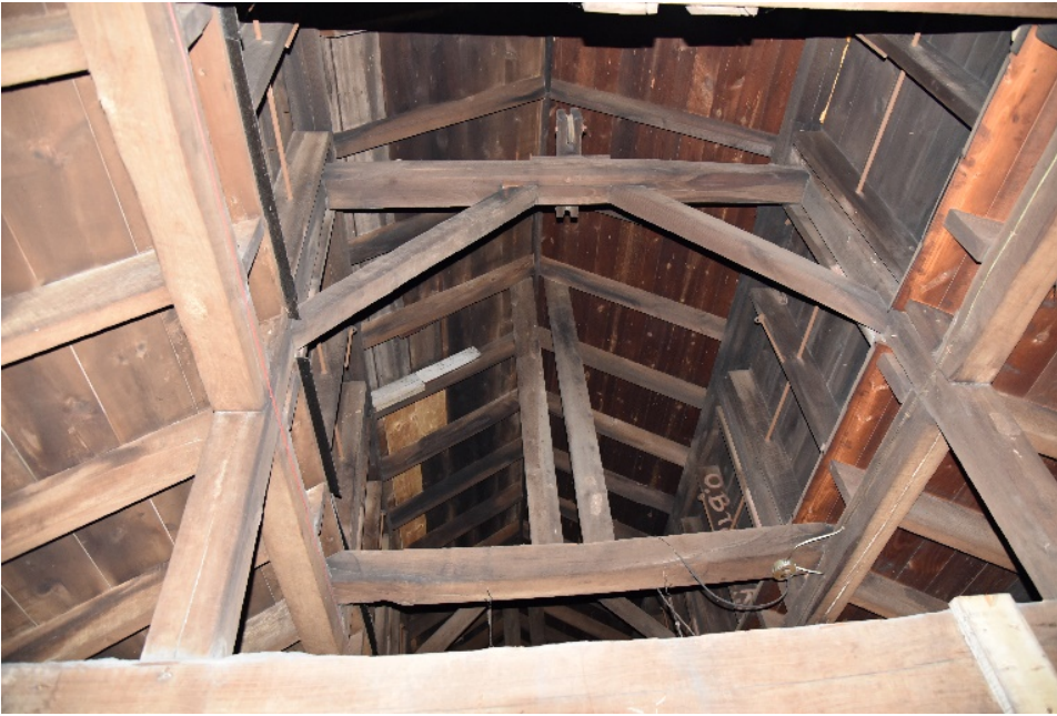
Photograph 89. Monitor framing above upper storage area.
