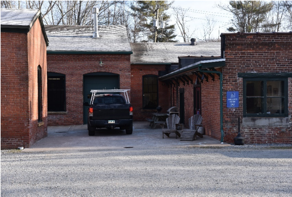
Photograph 45. From left: south end of boiler block, south end of polish room, northernmost bay of japan house, north and west elevations of auto house; camera facing east.
