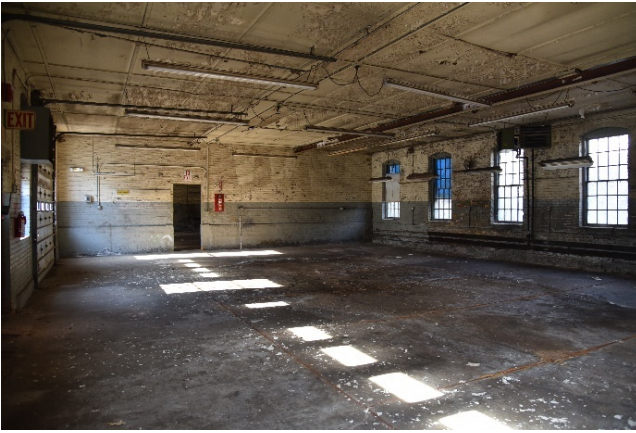
Photographs 102 & 103. Open workspace adjacent to office: camera facing west (L) with another brick firewall in background, and camera facing east (R) with non-structural mid-20 th century wall creating added office space at east end adjacent to office. Ceiling has same treatment as office.
