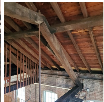
Photographs 87 & 88. Upper storage area at west end of building (L); truss and detail of framing sitting in load bearing brick wall (R).
