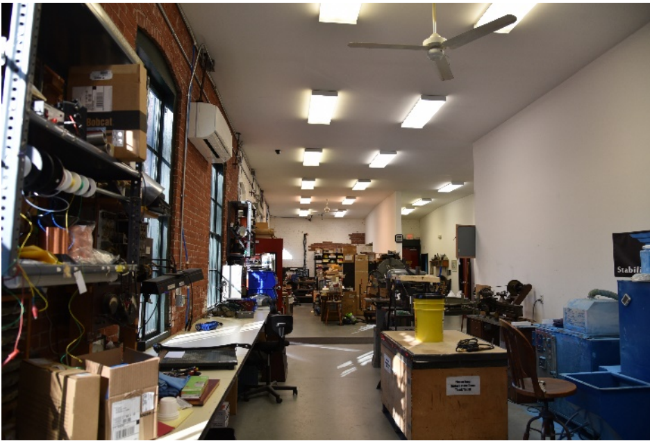
Photograph 52. Japan house interior with exposed brick perimeter walls and non-structural partition walls.
