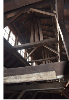
Photographs 108 & 109. Truss system and brick fire wall in background (L), and monitor truss (R).
