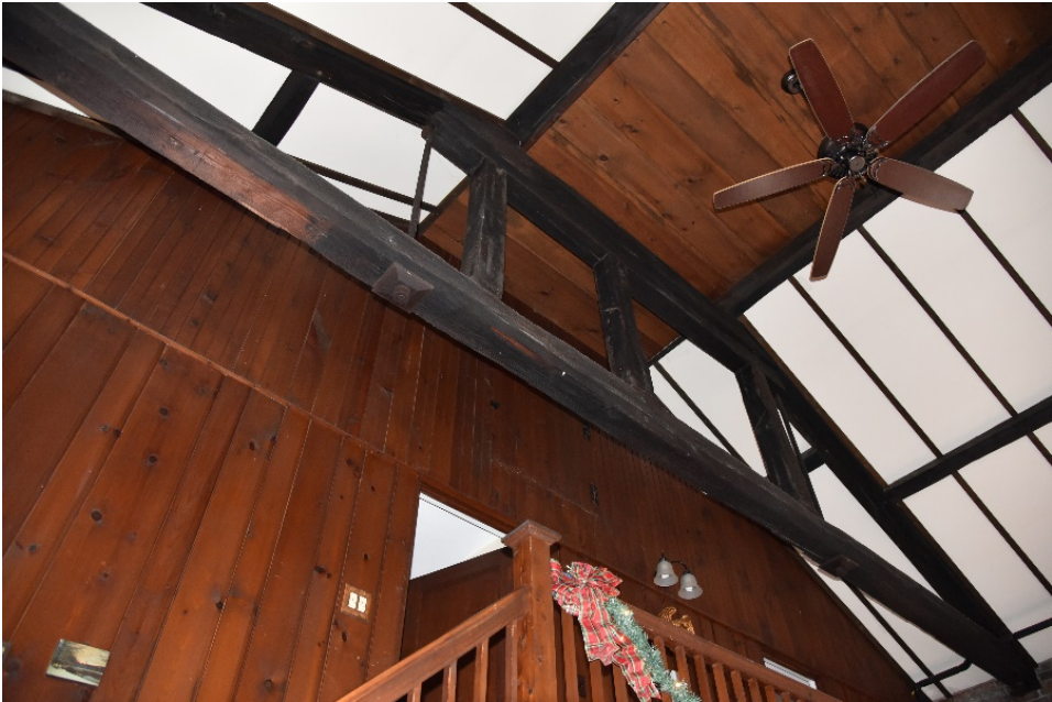
Photograph 22. Truss configuration and plank ceiling originally open to clerestory.
