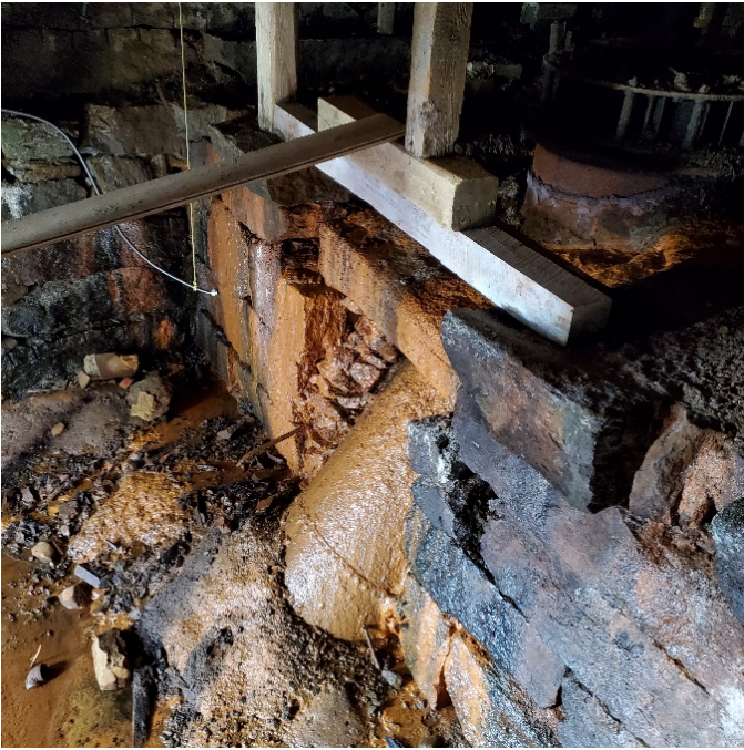
Photograph 32. Flume discharge for water exiting turbine.
