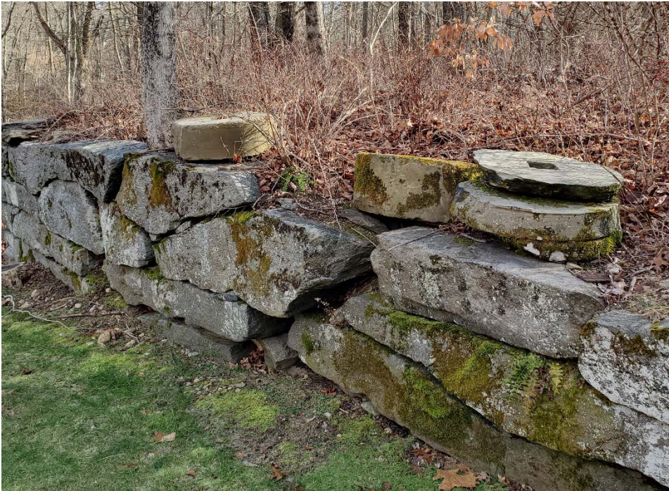
Photograph 8. Several of many small grindstones throughout the site used in working iron into hoes; these sit atop the north foundation wall of the north/south forge shop. They were approximately 6 feet in diameter when first used and changed out when reduced to 2-3 feet in diameter.
