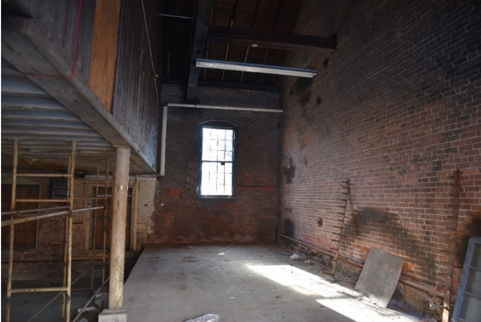
Photographs 90 & 91. Former engine room with elevated concrete floor and firewall at right (L). Detail showing extant monitor framing supported by brick corbels on fire wall (R).
