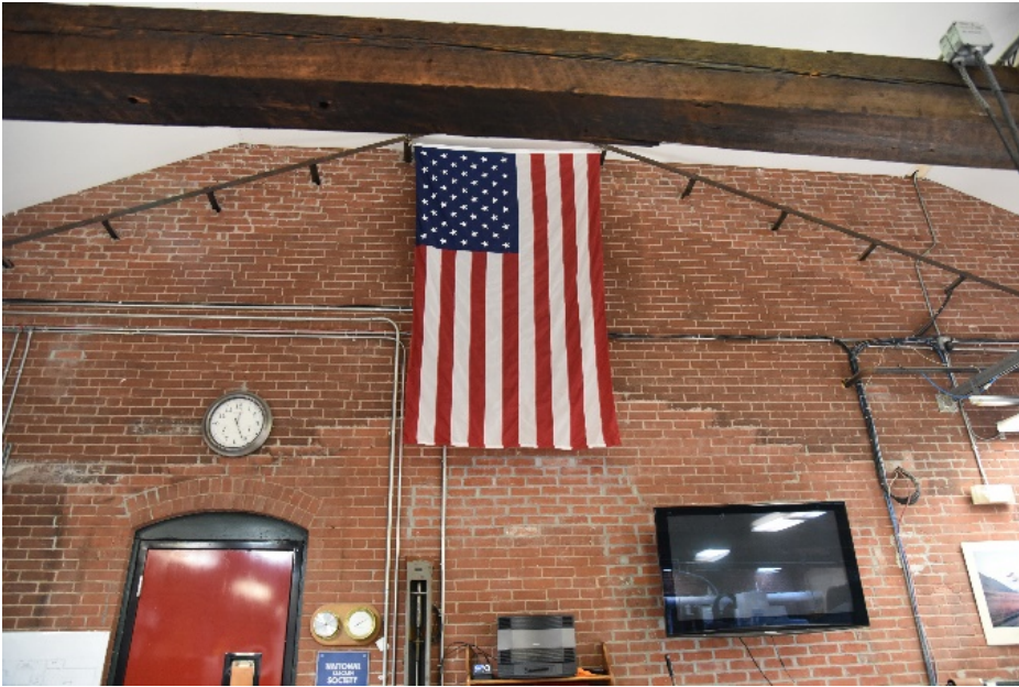
Photograph 54. Common wall between the japan house and polish room, taken from inside the latter; camera facing south. Note shadow line of prior building configuration as well as exposed ends of steel truss framing in Japan house.
