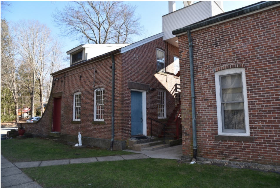
Photograph 16. North and west elevations of eastern block; camera facing east.
