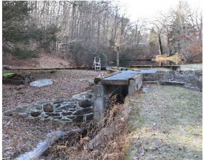
Photographs 35 & 36. Modern headgate for reservoir canal within stone wall structure; camera facing northeast (L), downstream side of headgate; camera facing southwest (R).
