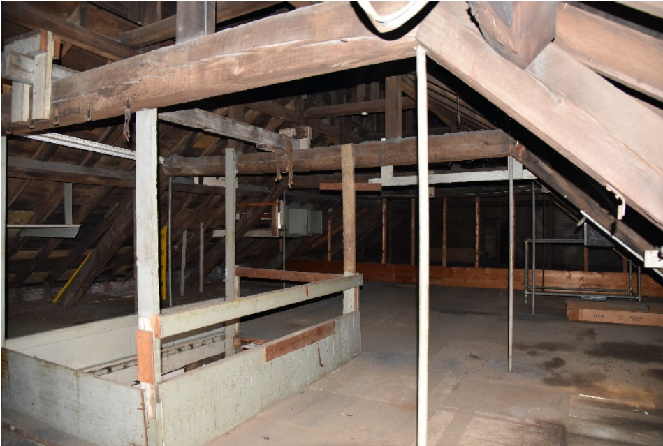
Photographs 87 & 88. Upper storage area at west end of building (L); truss and detail of framing sitting in load bearing brick wall (R).
