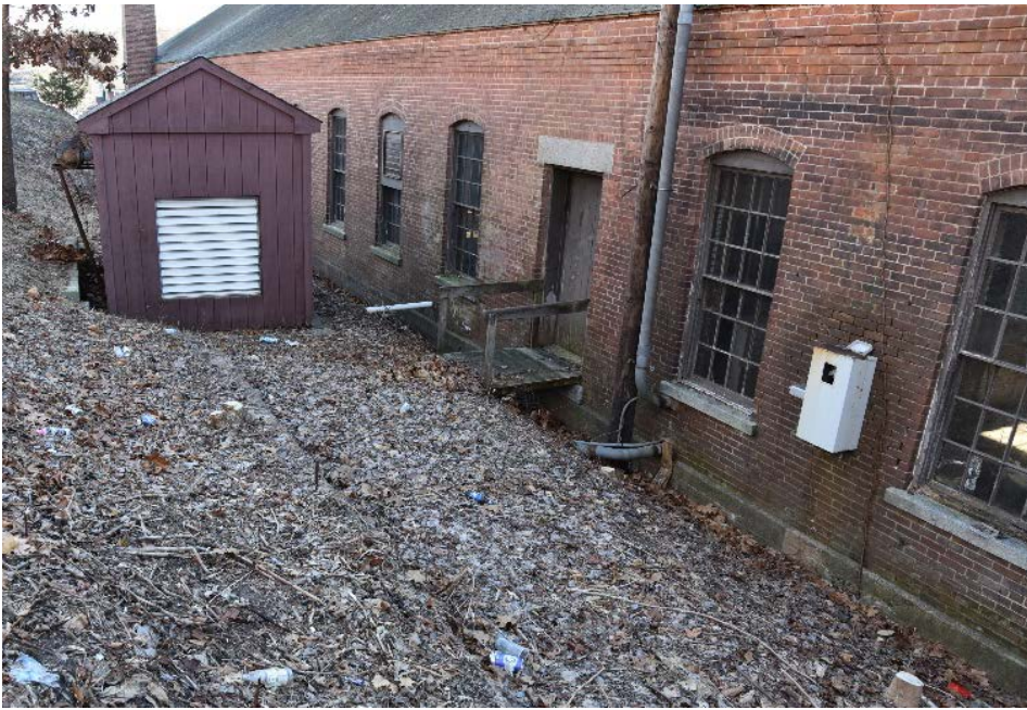
Photograph 98. Door and window openings on north elevation; camera facing east.
