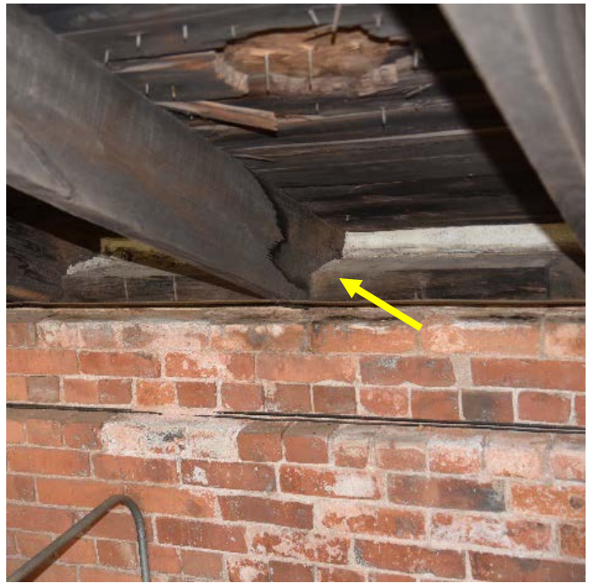
Photographs 62 & 63. Truss detail showing at least two periods of construction, from top, mortise and tenon joints, later toe-nailed supports, and notched joints with tie rods (L); main roof rafters seated on plate atop brick bearing wall with bird's mouth joint (R).
