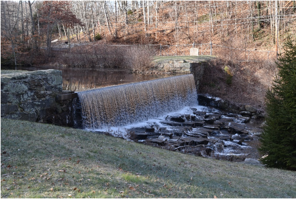
Photograph 34. Dam at mill pond for Mill #3; camera facing west. The headgate to the canal is to its left. Candlewood Hill Road is on the north (back) side of the pond.
