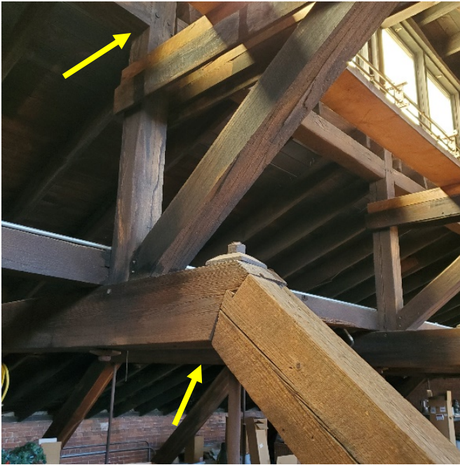
Photographs 62 & 63. Truss detail showing at least two periods of construction, from top, mortise and tenon joints, later toe-nailed supports, and notched joints with tie rods (L); main roof rafters seated on plate atop brick bearing wall with bird's mouth joint (R).
