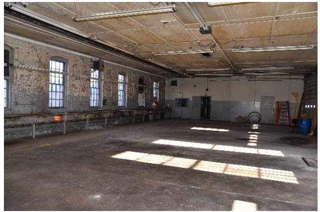
Photographs 102 & 103. Open workspace adjacent to office: camera facing west (L) with another brick firewall in background, and camera facing east (R) with non-structural mid-20 th century wall creating added office space at east end adjacent to office. Ceiling has same treatment as office.
