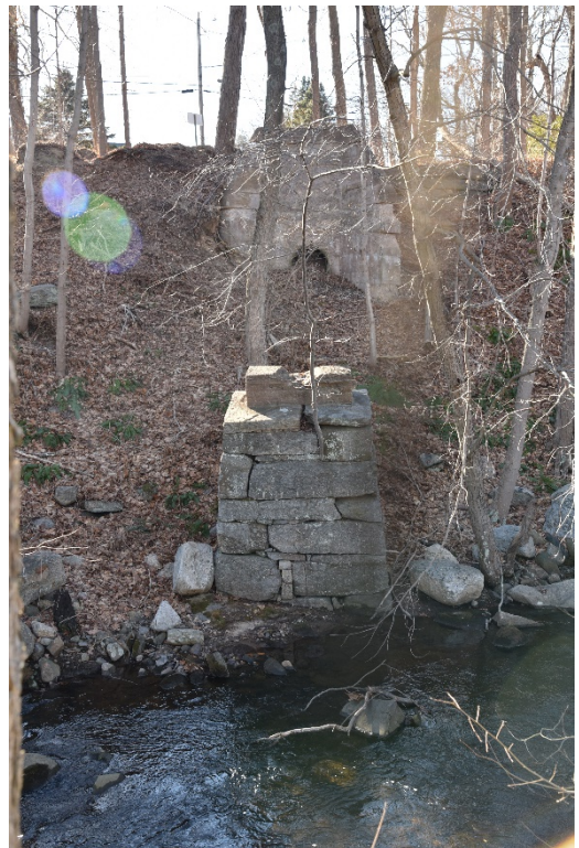
Photographs 76 & 77. Stone embankment wall on south side of brook where flume traveled (L) and stone pillars that carried the flume across the brook from the south bank to the 1886 mill (R) at non-contributing archaeological site at Mill #4.
