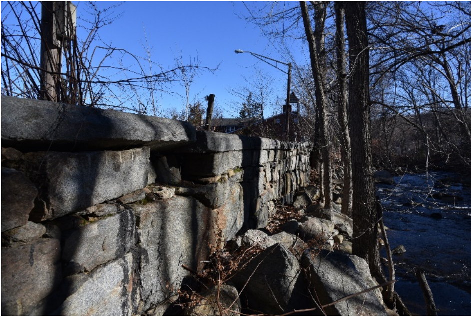
Photograph 78. Cut stone retaining wall on mill/north side of brook near flume crossing.
