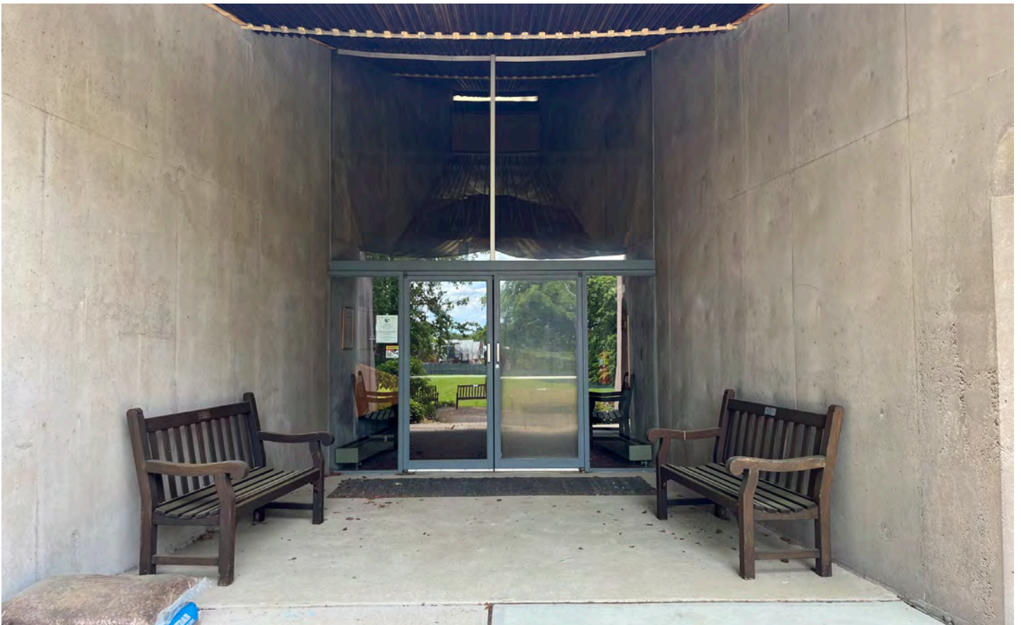
Photograph 8 of 29. Detail of secondary entrance at southeast building corner.
