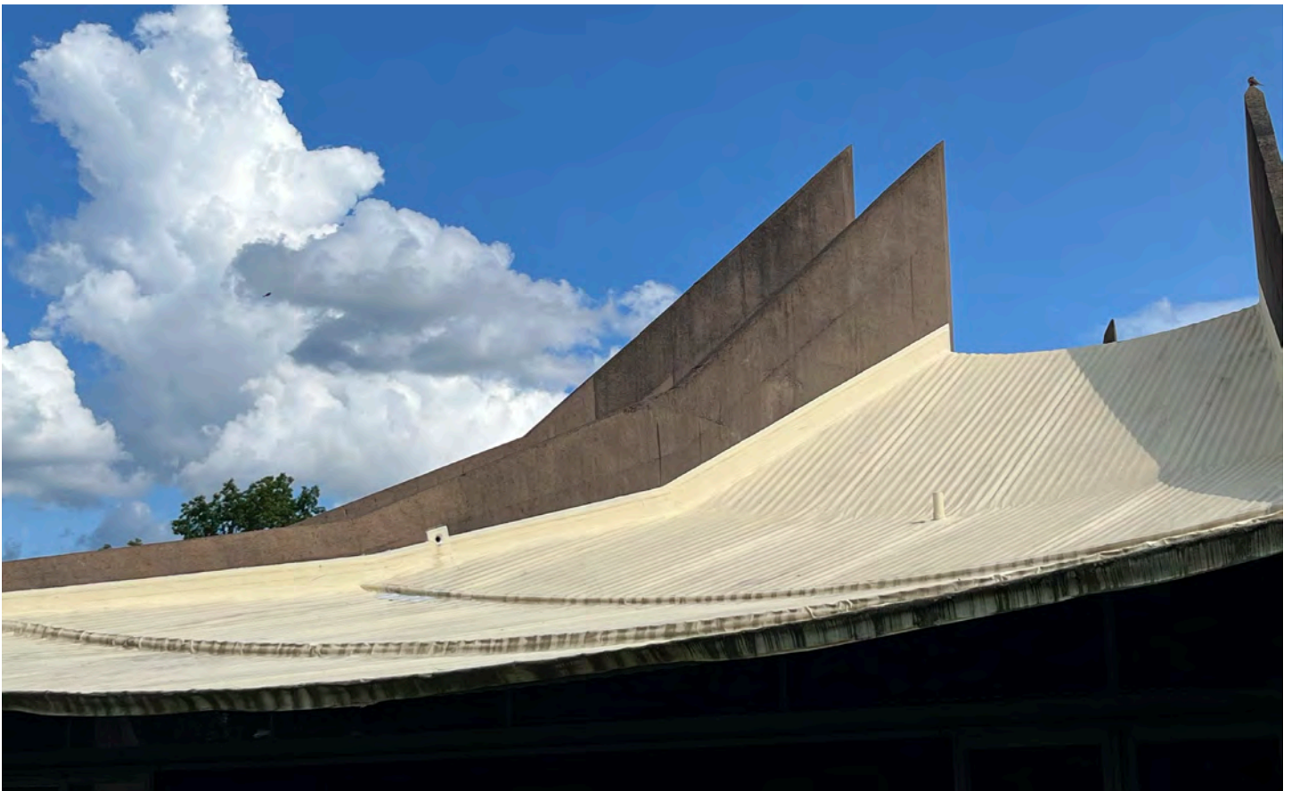
Photograph 6 of 29. Roof scupper in concrete peripheral wall.
