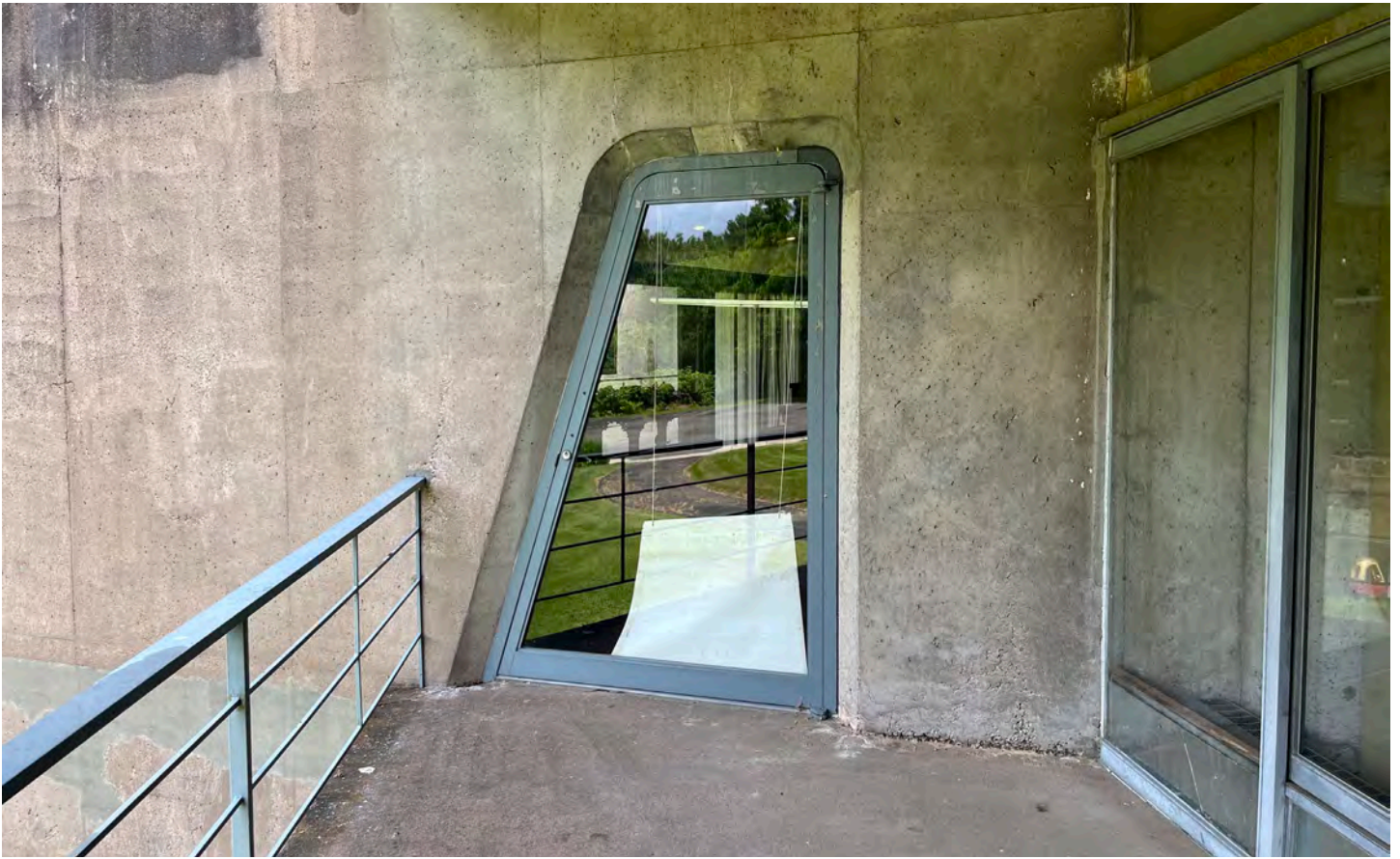
Photograph 11 of 29. Trapezoidal glass-and-metal doors to balcony from the chapel.
