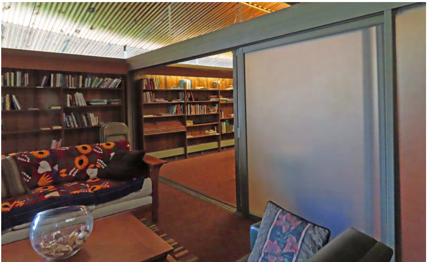
Photograph 22 of 29. Aluminum-and-glass sliding partitions between main-level peripheral meeting rooms.
