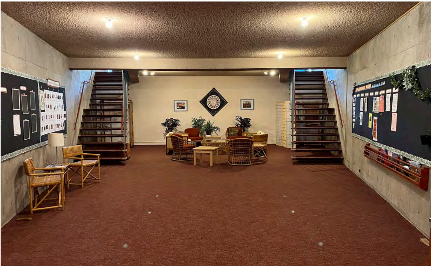
Photograph 26 of 29. Metal-and-wood open-riser stairs at basement level.
