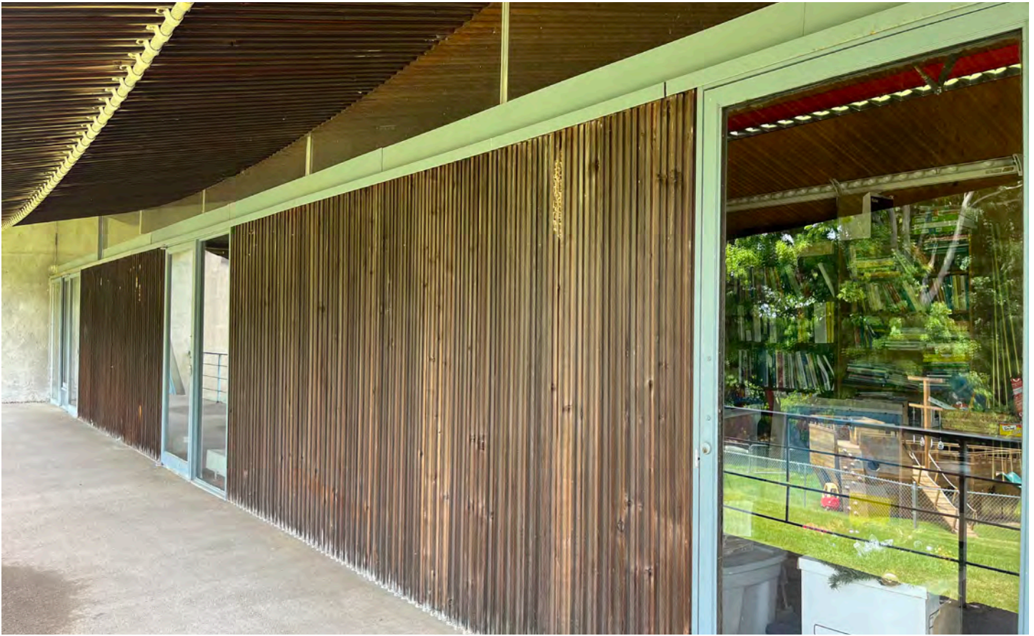
Photograph 9 of 29. Exterior wall composition at main-level peripheral meeting rooms.
