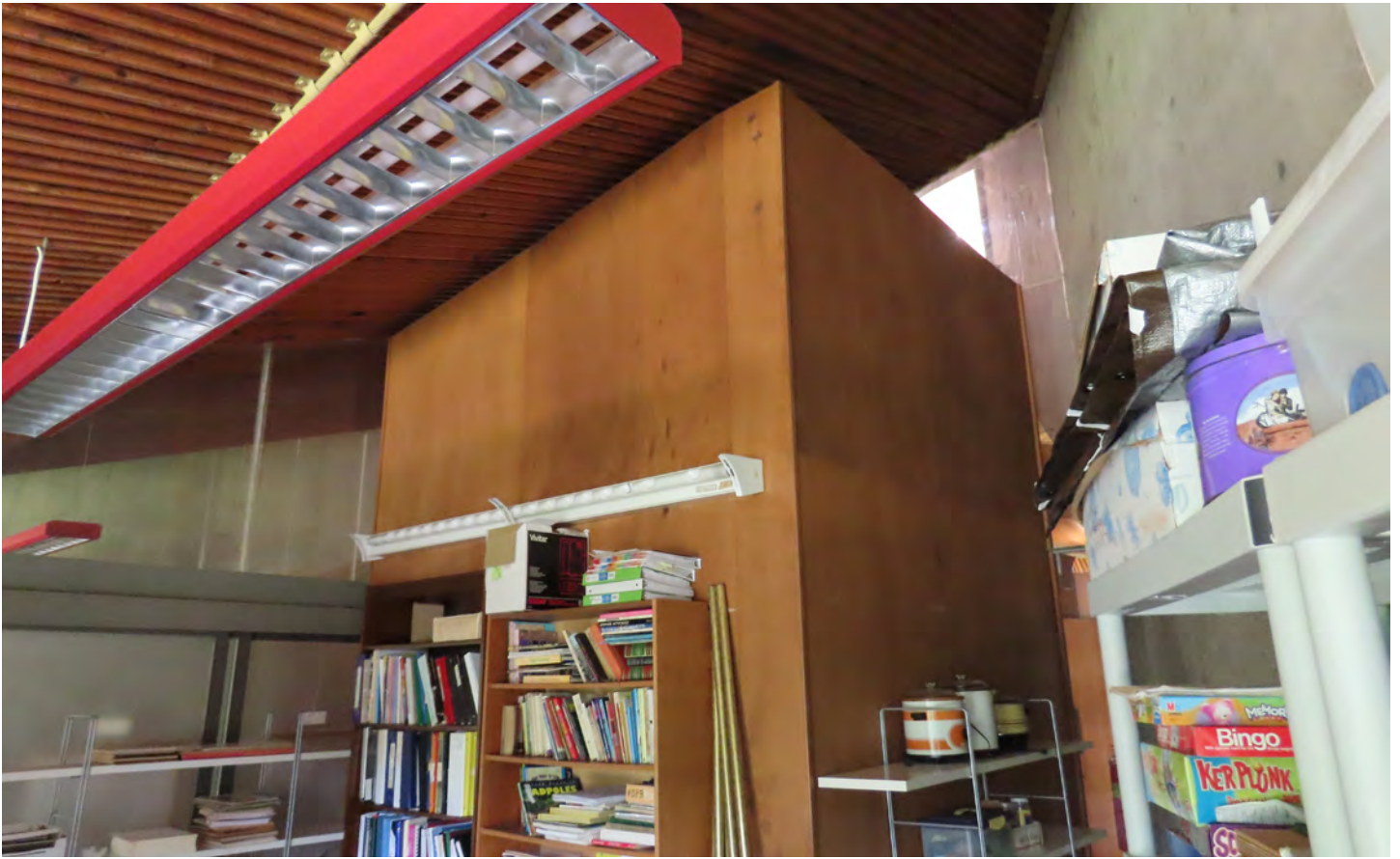
Photograph 25 of 29. Elevator shaft added at main-level peripheral meeting room in 1993.
