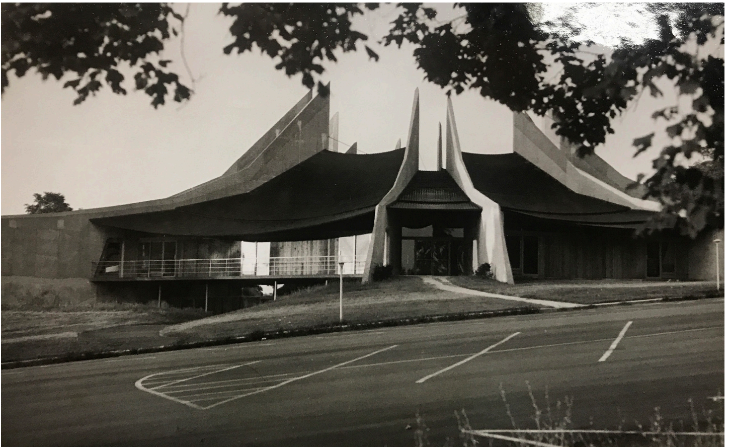
Figure 5 of 13. Building exterior, looking north, showing original dark-colored nylon roof membrane, c. 1964. Unitarian Society of Hartford Archives.
