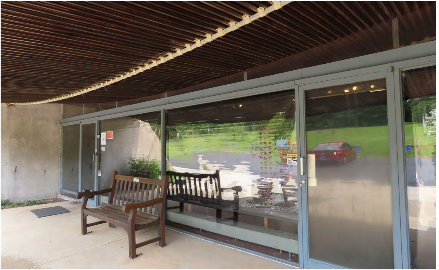
Photograph 7 of 29. Detail of primary entrance at west façade.
