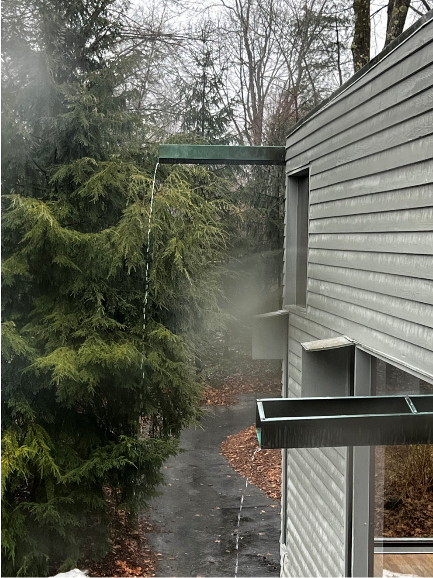
7 of 21. Copper rainspouts off living room, looking south.
