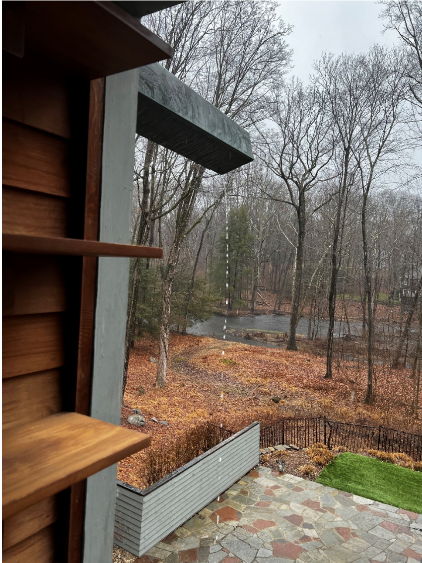
8 of 21. Copper rainspouts on rear (east) elevation, looking east.
