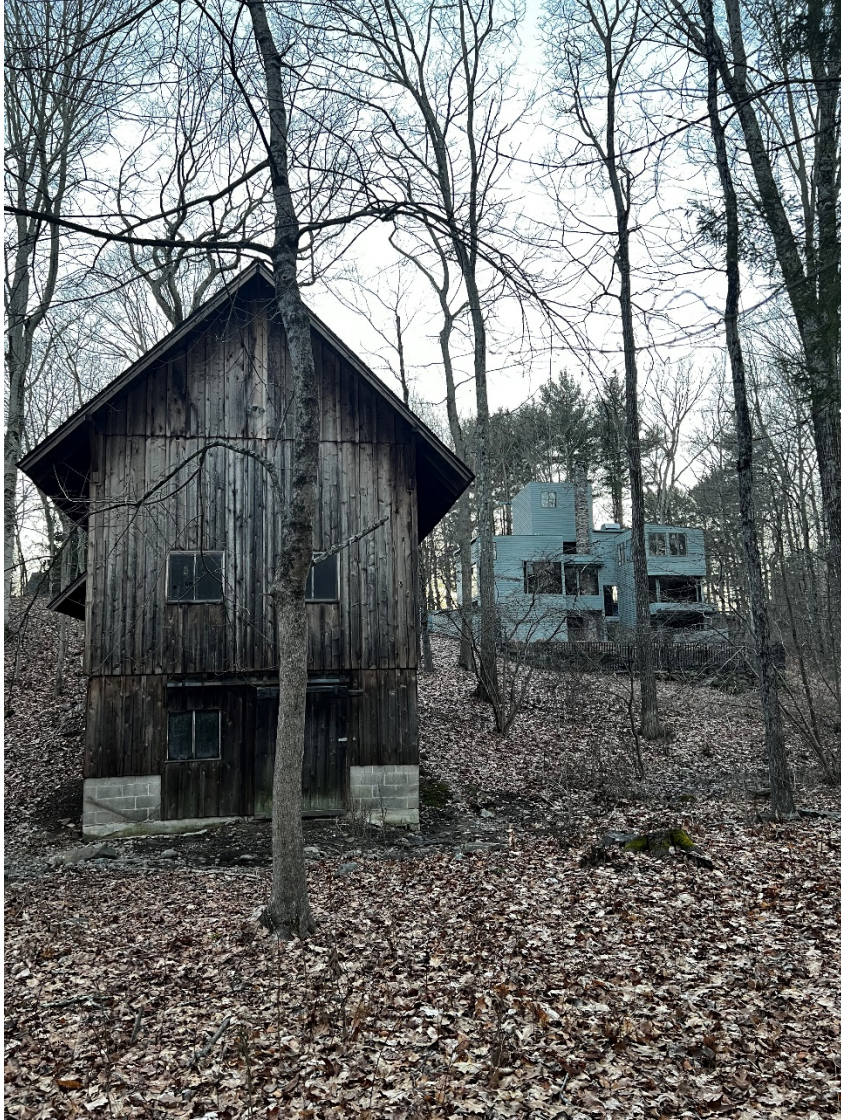
21 of 21. Non-contributing bank barn, in wetlands, with house in background, looking west.
