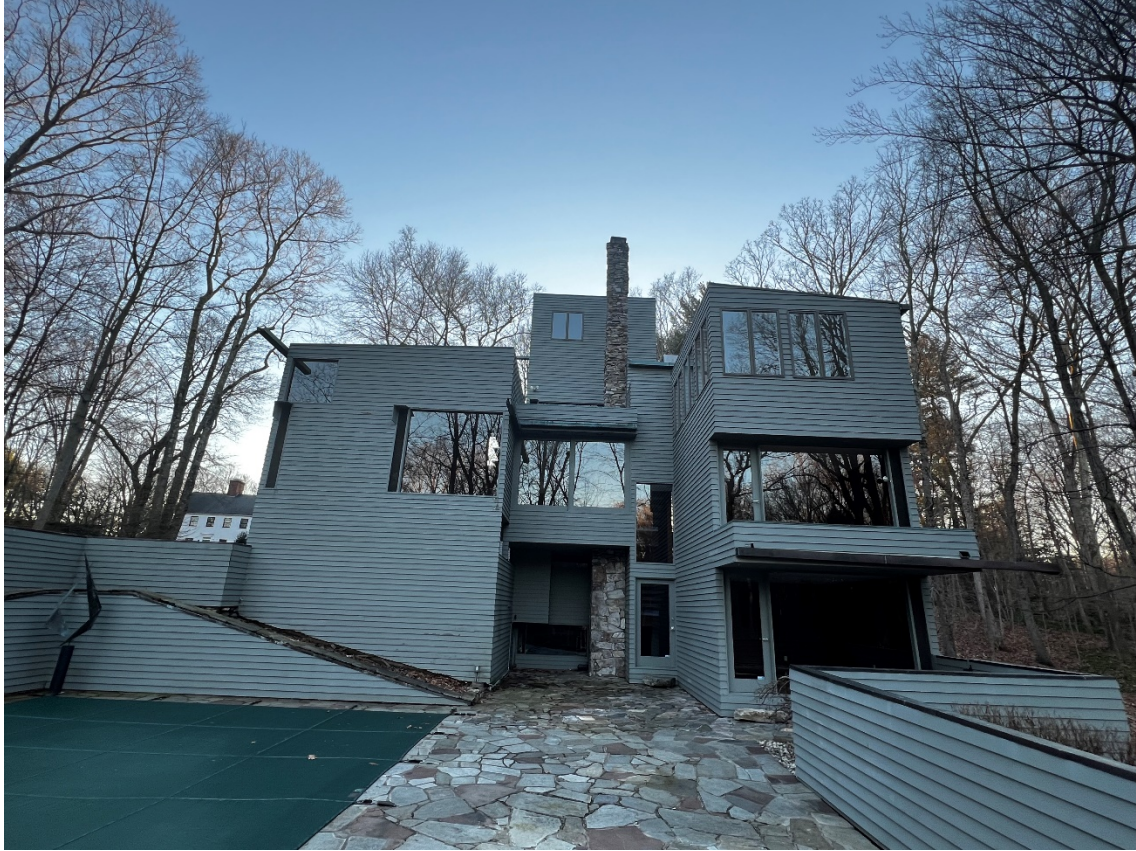
6 of 21. Rear (east) elevation showing three towers and new pool and patio, looking west.
