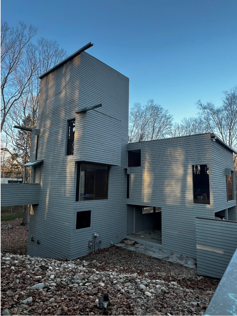
4 of 21. Southwest corner, looking northeast.
