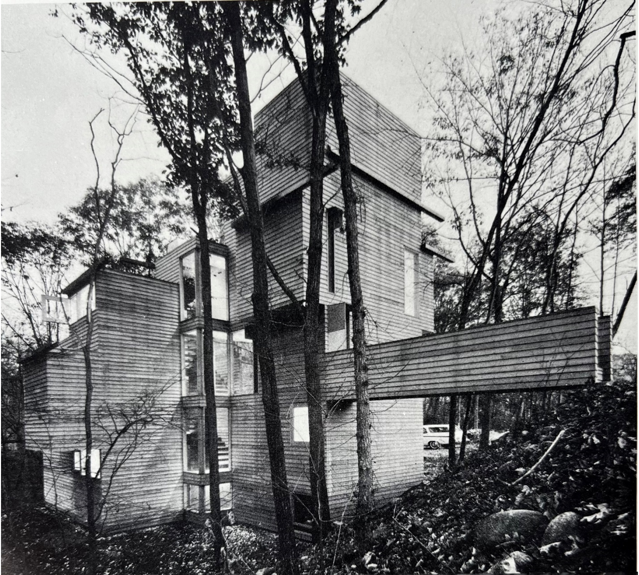
Figure 8. View of northwest elevation showing bridge entry looking southeast. Source: David Hirsch, Progressive Architecture , May 1965.
