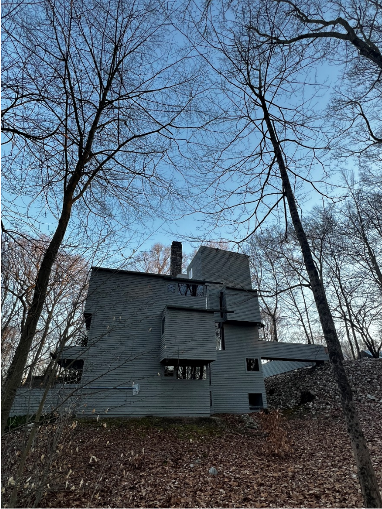
2 of 21. North (side) elevation showing cantilevered kitchen and primary bedroom closet, looking south.
