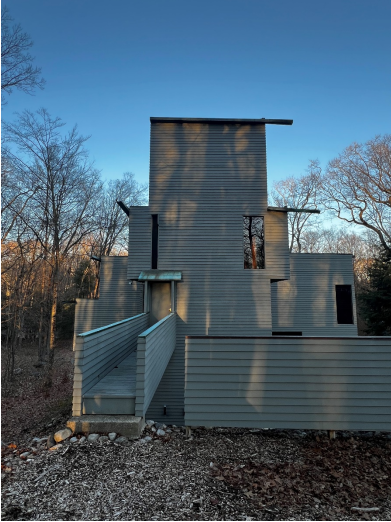
3 of 21. Front bridge entrance, looking east at façade (west elevation).
