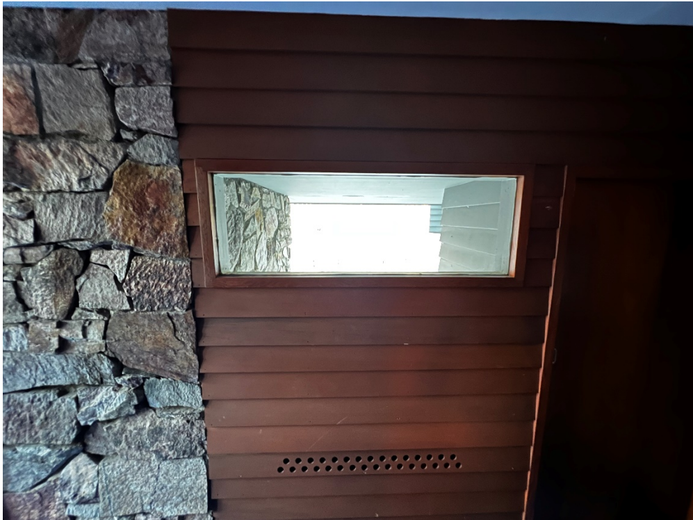
11 of 21. Detail of chimney and interior cedar siding with vented radiator, facing south. Level 2.
