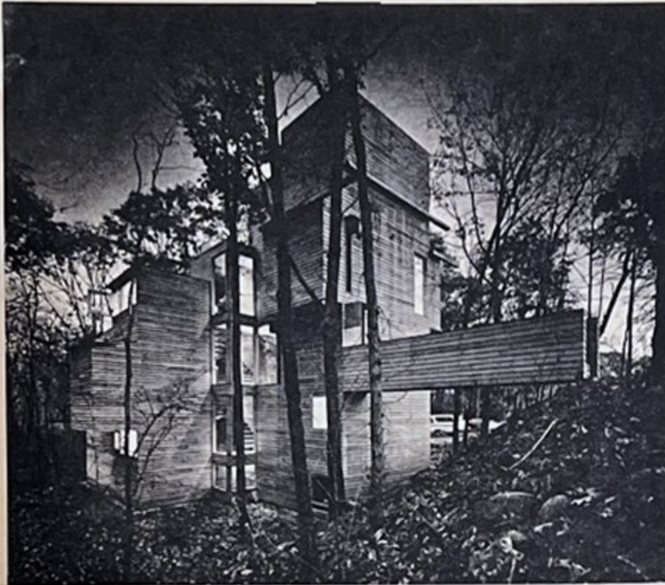
MULTILEVEL HOUSE —Central core is the staircase (seen through the vertical shaft of glass, center). Bridge, built over a dip in the land, leads to study and living room. Projections from the facade solve functional problems of kitchen and closets and provide terraces.
