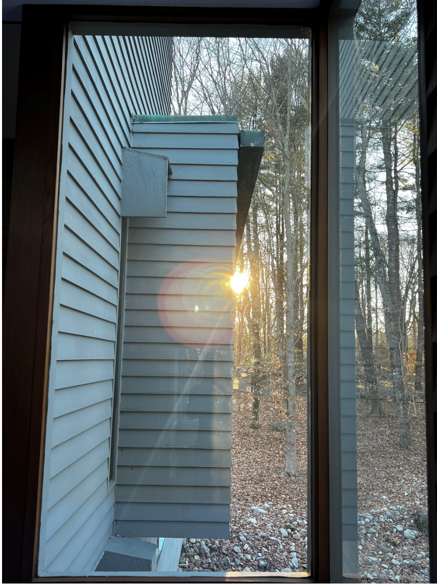
19 of 21. Cantilevered primary bedroom closet, looking west. Level 6.
