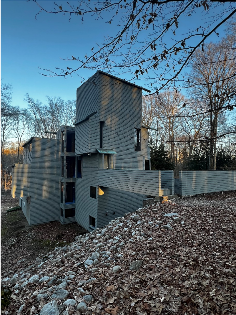
1 of 21. Main tower and central staircase with glass landings, looking southeast.
