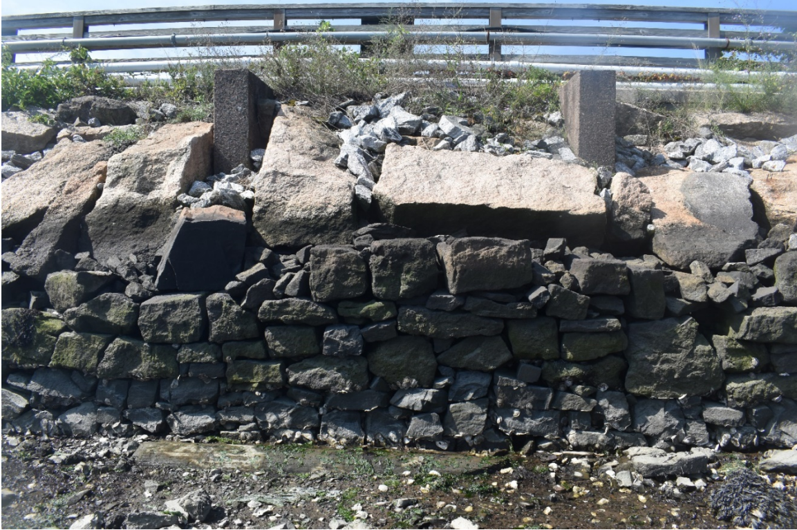
Photograph 5. Long Wharf Pier, looking southwest toward 1810 masonry underneath modern rip-rap.
