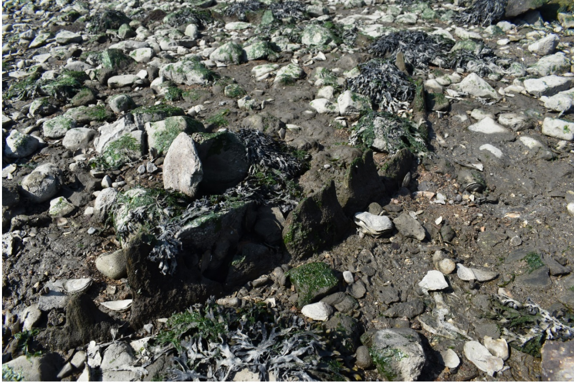
Photograph 11. Detail of wood structural remains within Long Wharf Pier footprint south of modern tidal marker, looking southwest.
