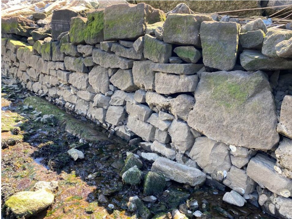
Figure 10. Long Wharf Pier structure, looking south (2021, New Haven Preservation Trust).
