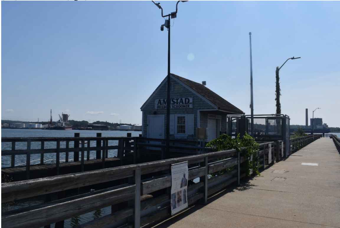
Photograph 16. Long Wharf Pier and Amistad Freedom Schooner Ticket Booth, looking east.
