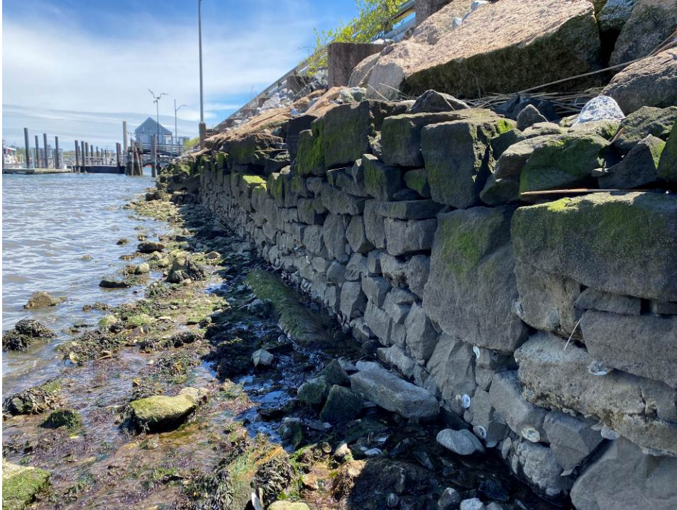
Figure 9. Long Wharf Pier structure, looking south (2021, New Haven Preservation Trust).
