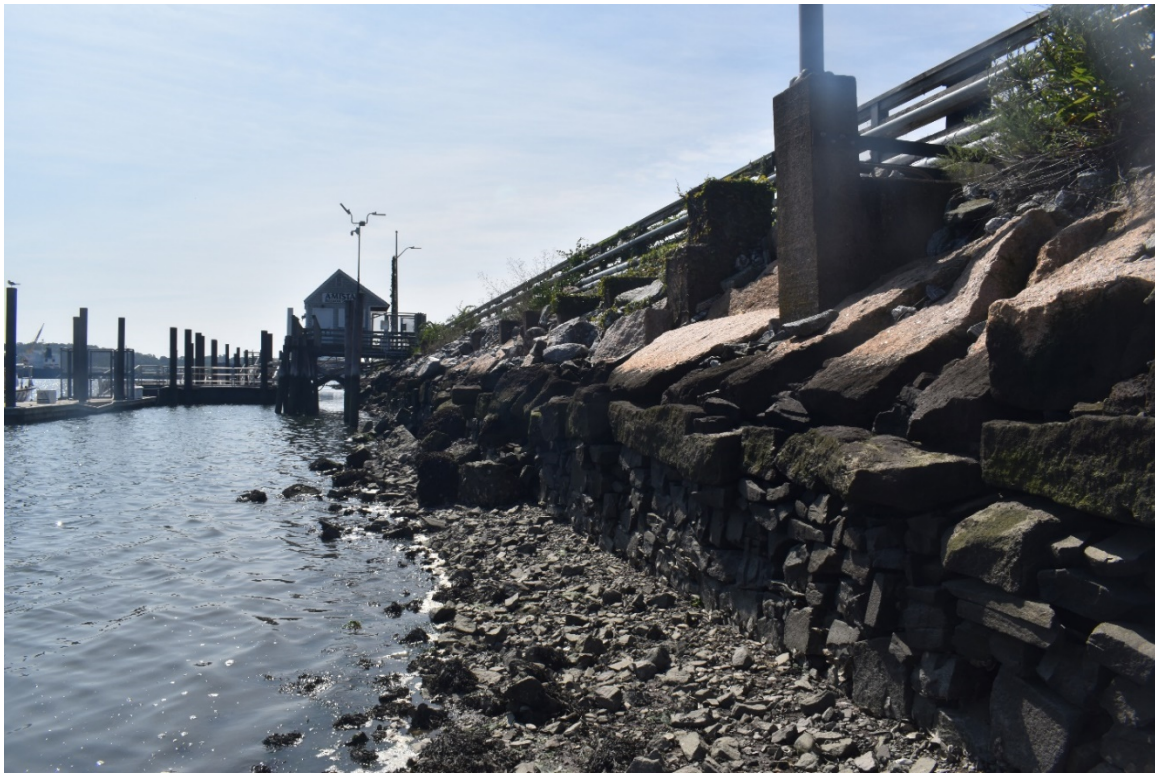
Photograph 4. Long Wharf Pier, looking southeast toward 1810 masonry underneath modern rip-rap.
