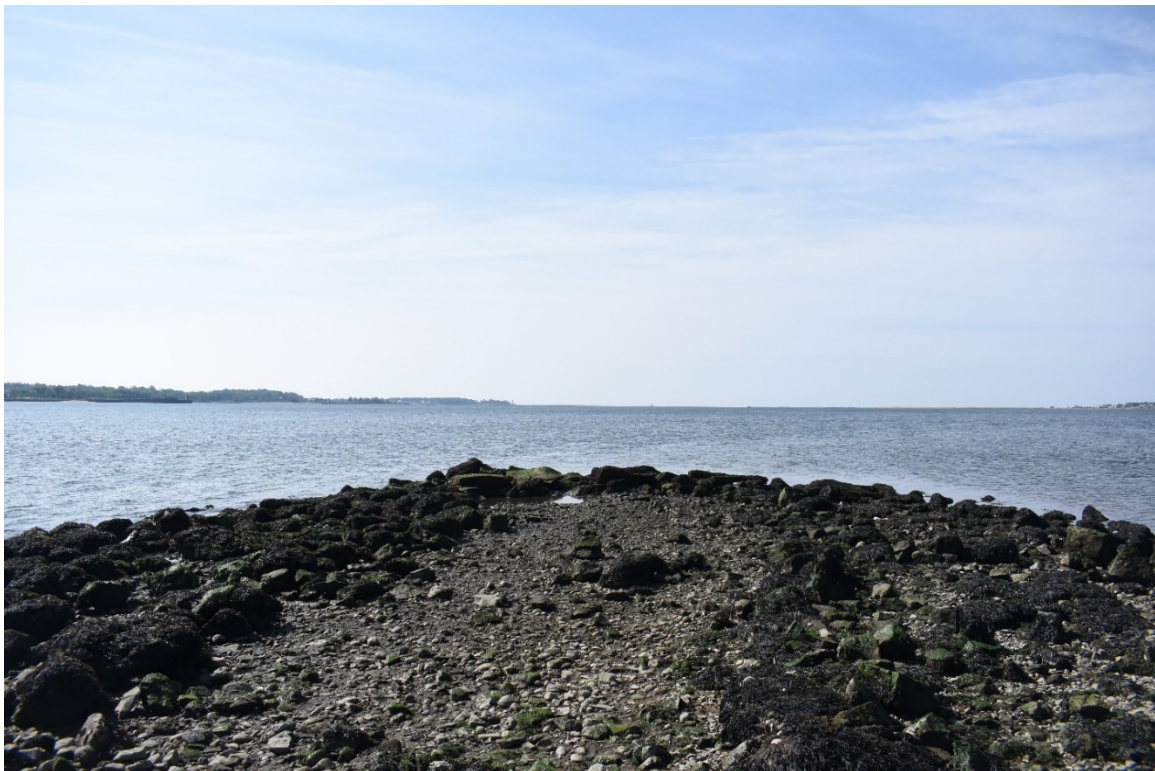
Photograph 12. Long Wharf Pier remnants, looking south.
