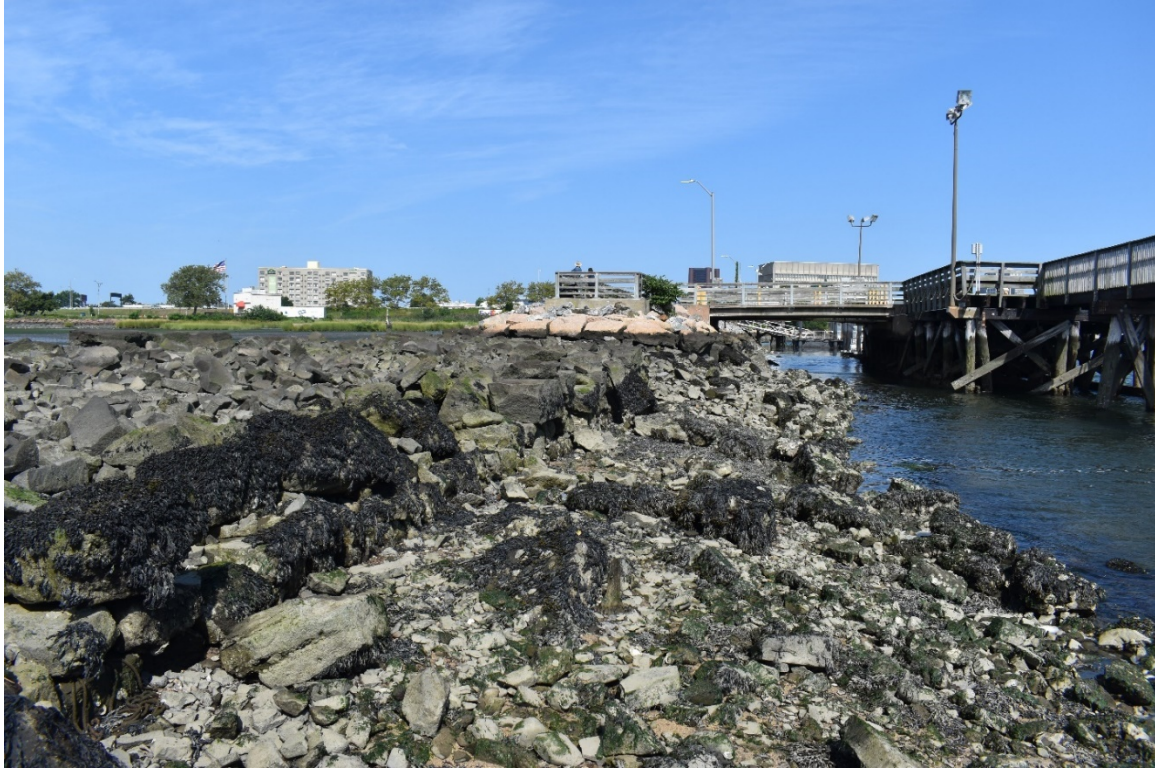
Photograph 9. Masonry remains from 1810 extension of Long Wharf Pier, looking northwest.
