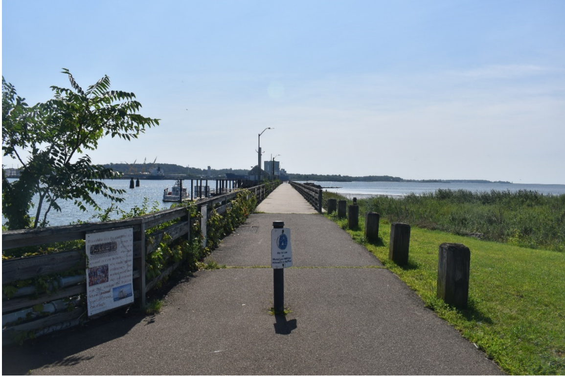
Photograph 3. Long Wharf Pier, looking southeast from head of the pier.
