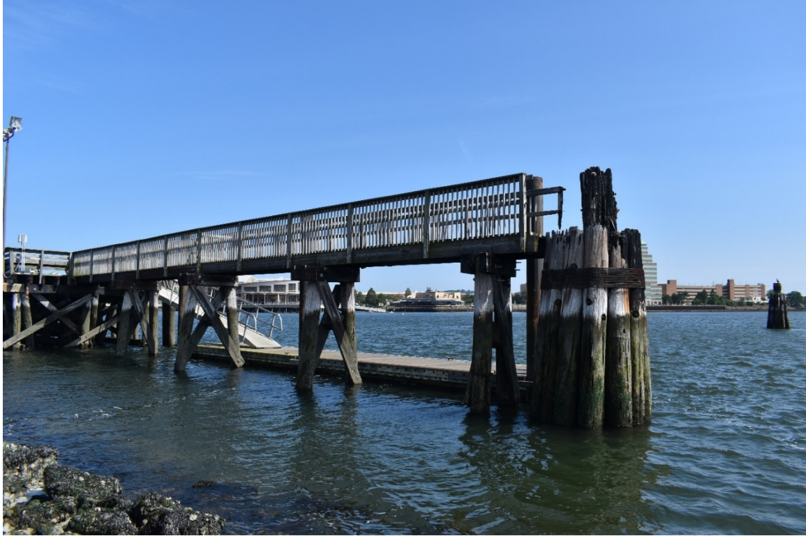
Photograph 7. Long Wharf Pier wood pier and floating platforms, looking north.
