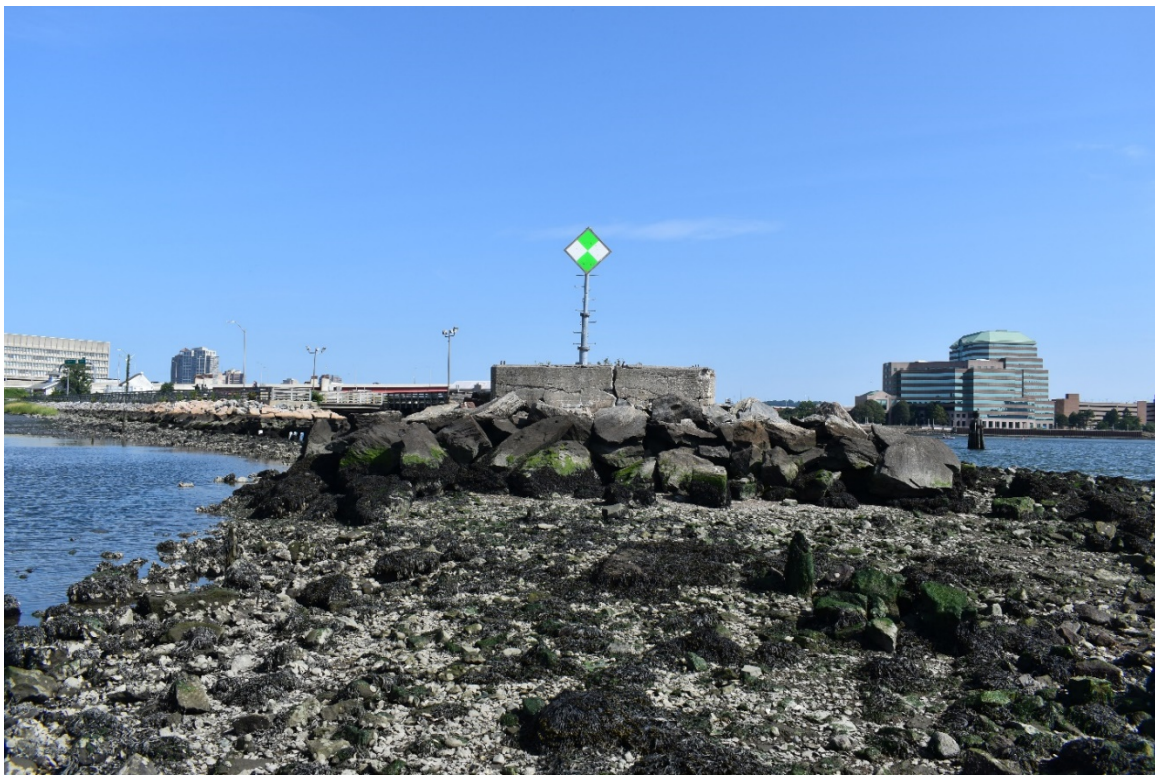
Photograph 10. Modern tidal marker constructed on top of Long Wharf Pier remnants, looking north.
