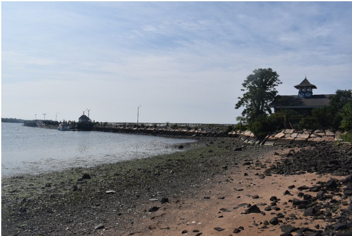
Photograph 2. Long Wharf Pier, looking southwest from beach east of pier.
