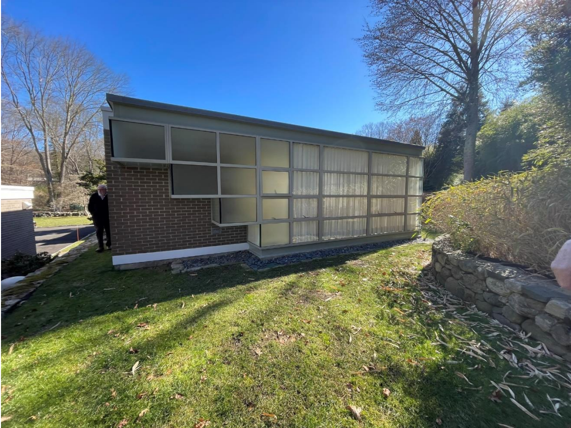
Photograph 10. North elevation of addition, view southeast.
