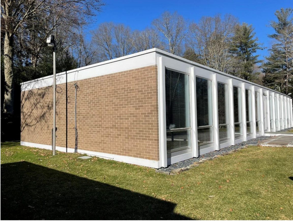
Photograph 11. Southern elevation, view northwest.
