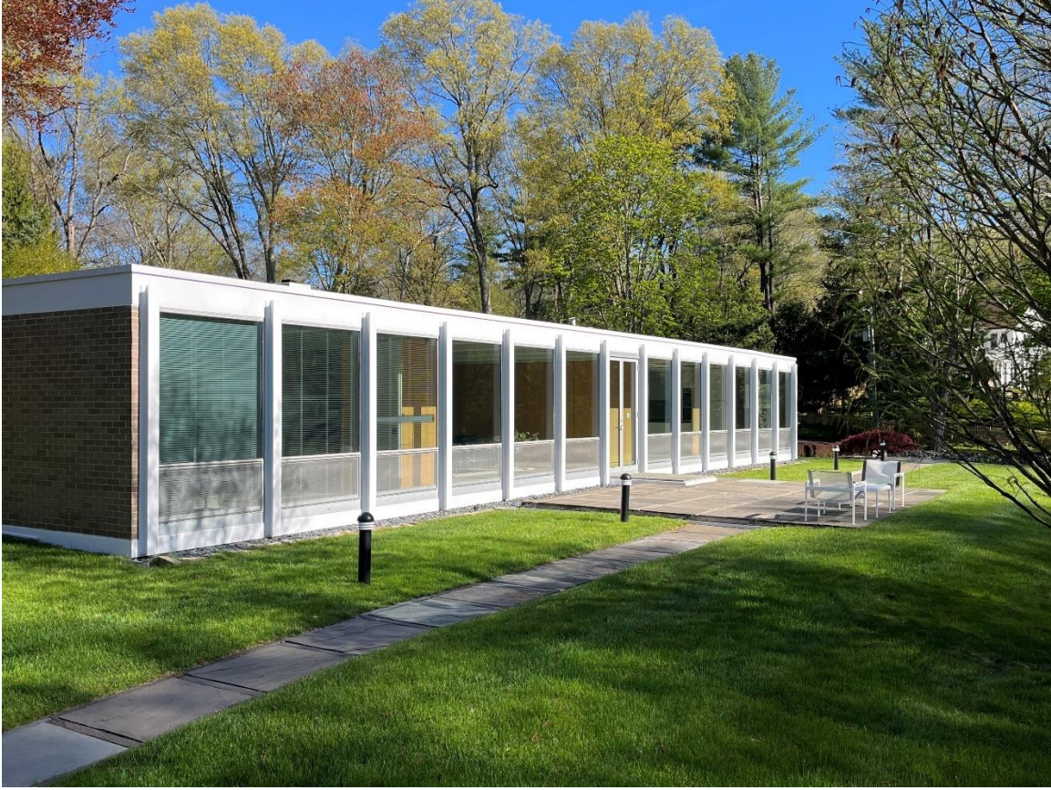
Photograph 1. View of the east elevation (façade), view north.
