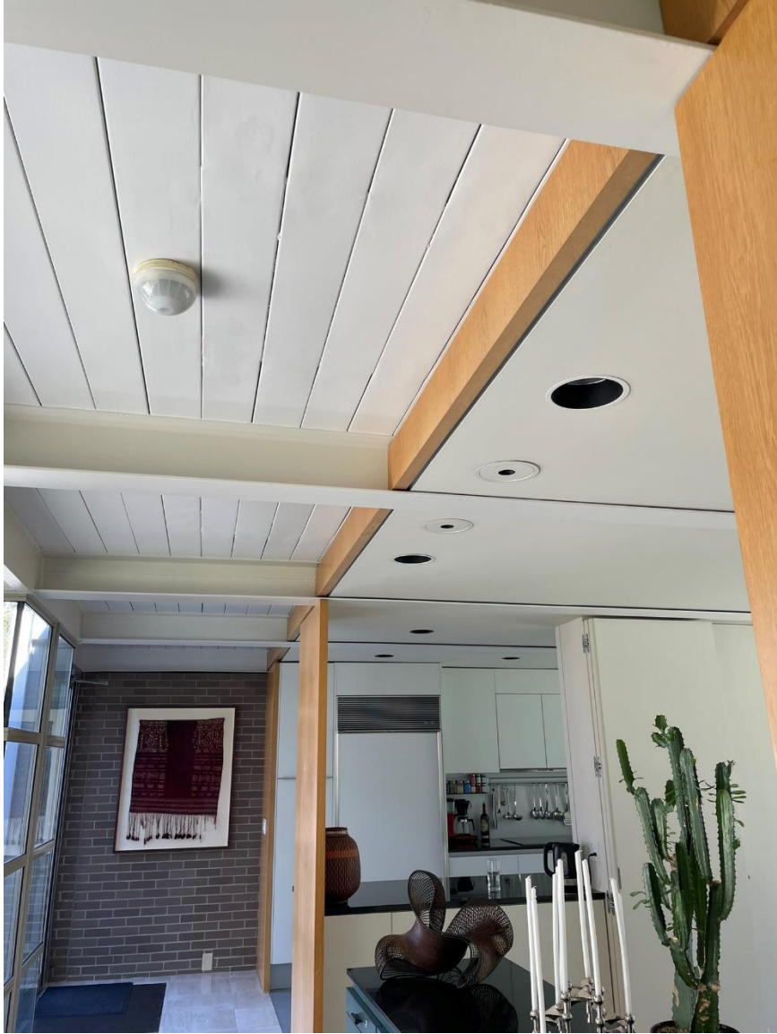
Photograph 13. Ceiling showing I-beams and metal roof deck, view south.
