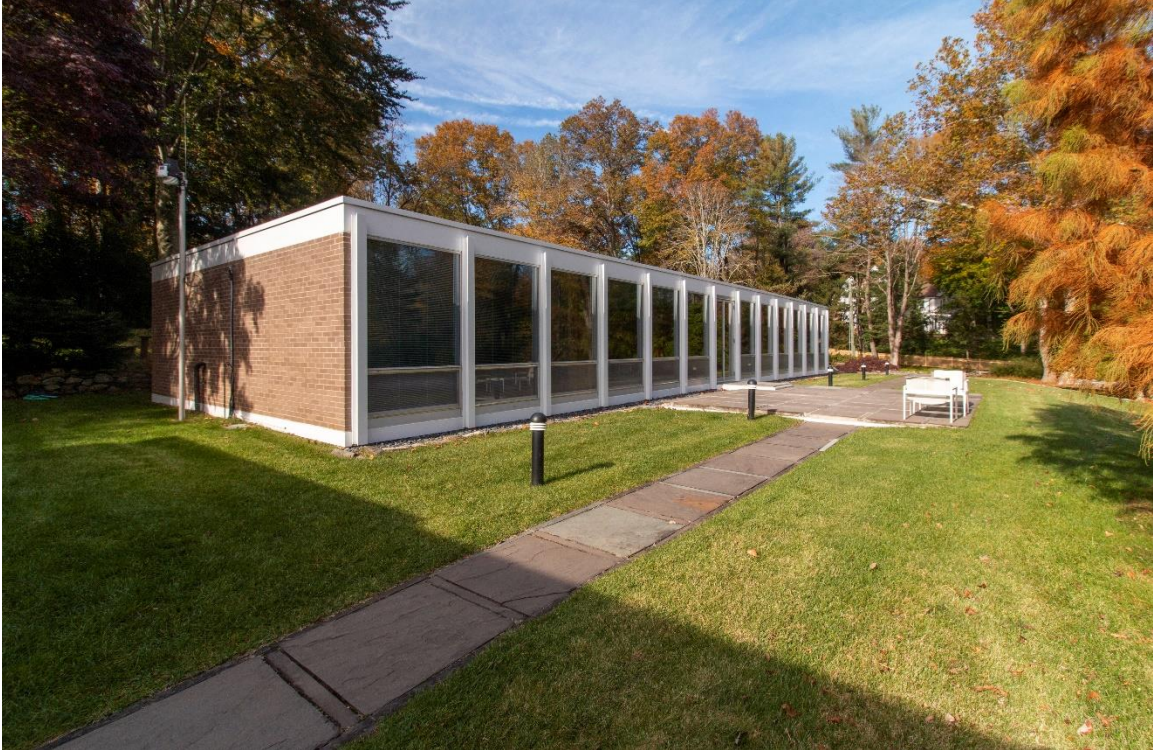
Photograph 6. South and east elevations, view northwest (Photo from Bob Gregson).
