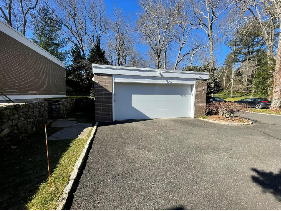
Photograph 28. Garage (1960), view west.
