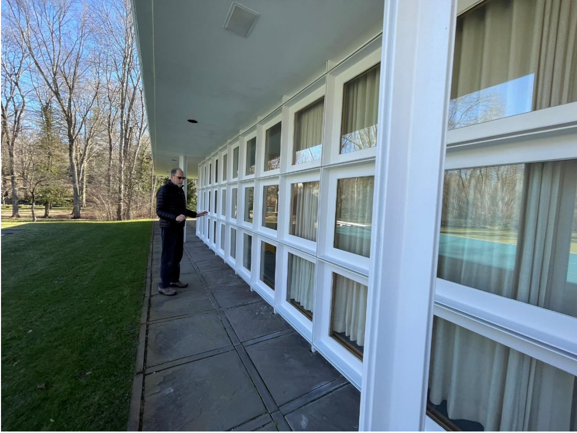
Photograph 33. Steel screen connecting pool and guest pavilions, view south.
