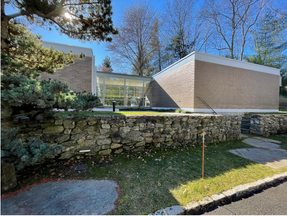
Photograph 12. Eastern elevation showing main block, corridor and second addition, view south.
