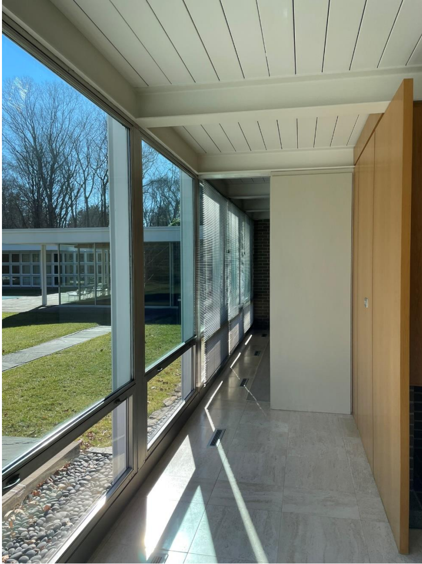
Photograph 16. Partition walls separating public and private spaces, looking south.
