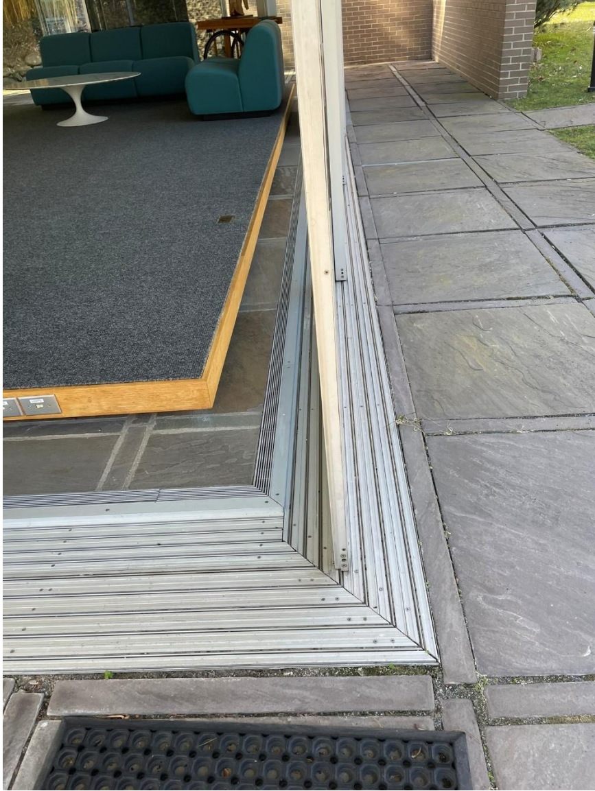
Photograph 31. Steel tracks in pavilion walls, view west.
