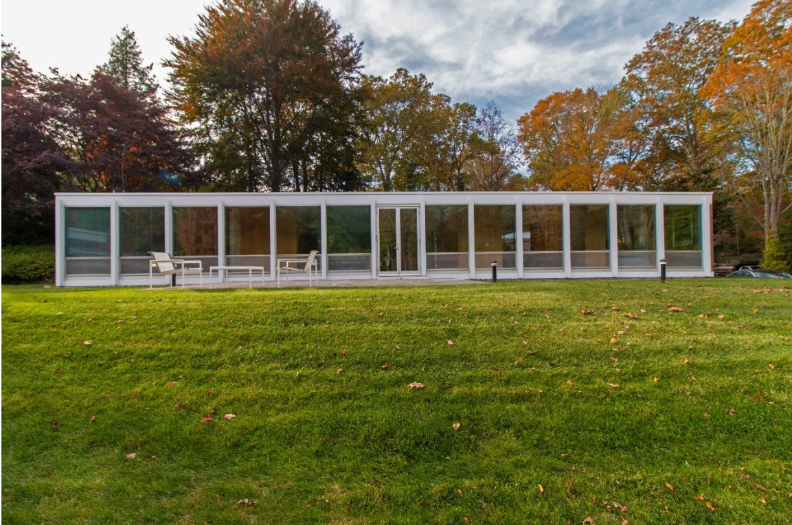
Photograph 2. East elevation, view west (Photo by Bob Gregson).
