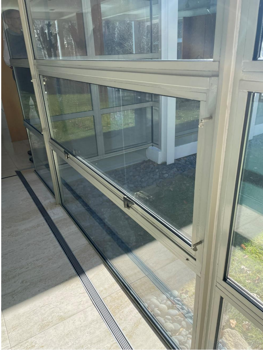
Photograph 9. Hopper windows on second addition, view southwest.
