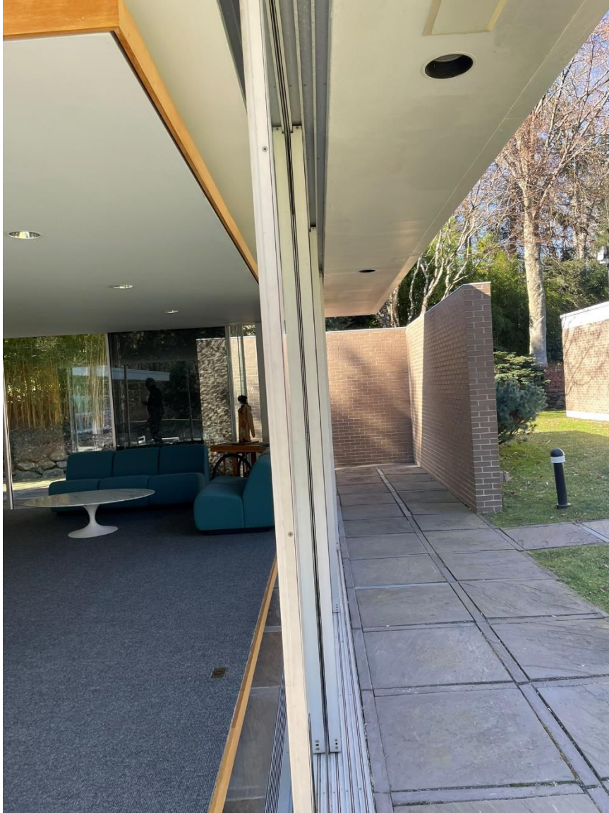
Photograph 32. Walls and surrounding brick walls of pool pavilion, view west.
