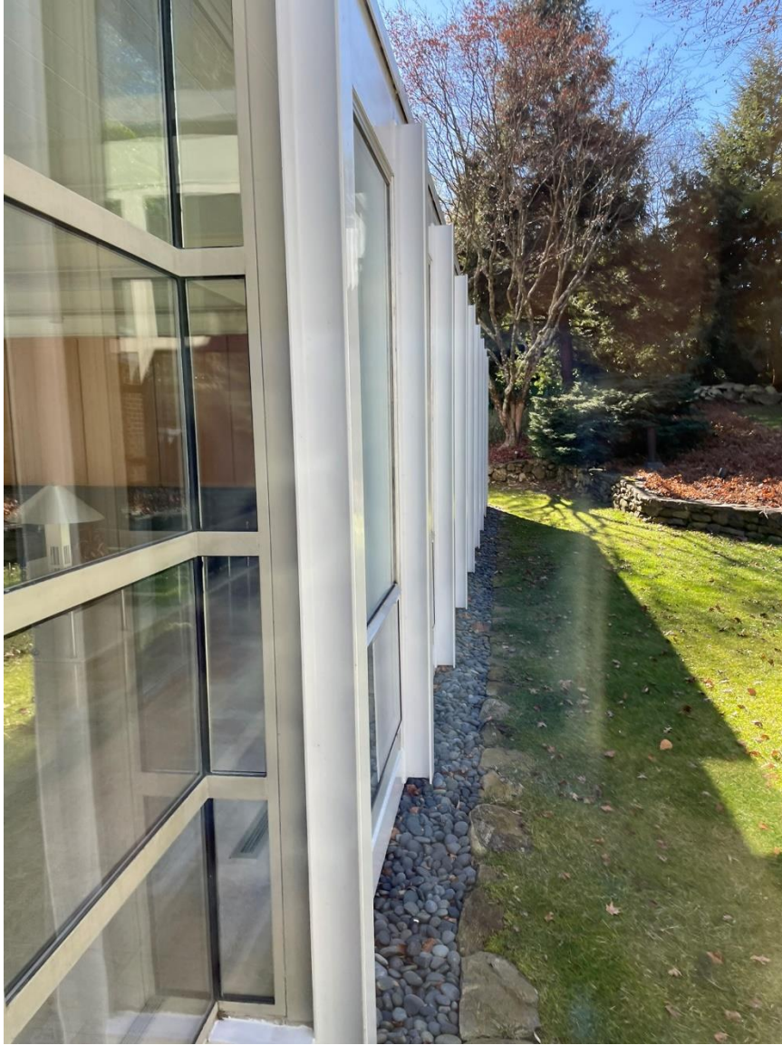
Photograph 8. Connection between second addition and main block, view south.
