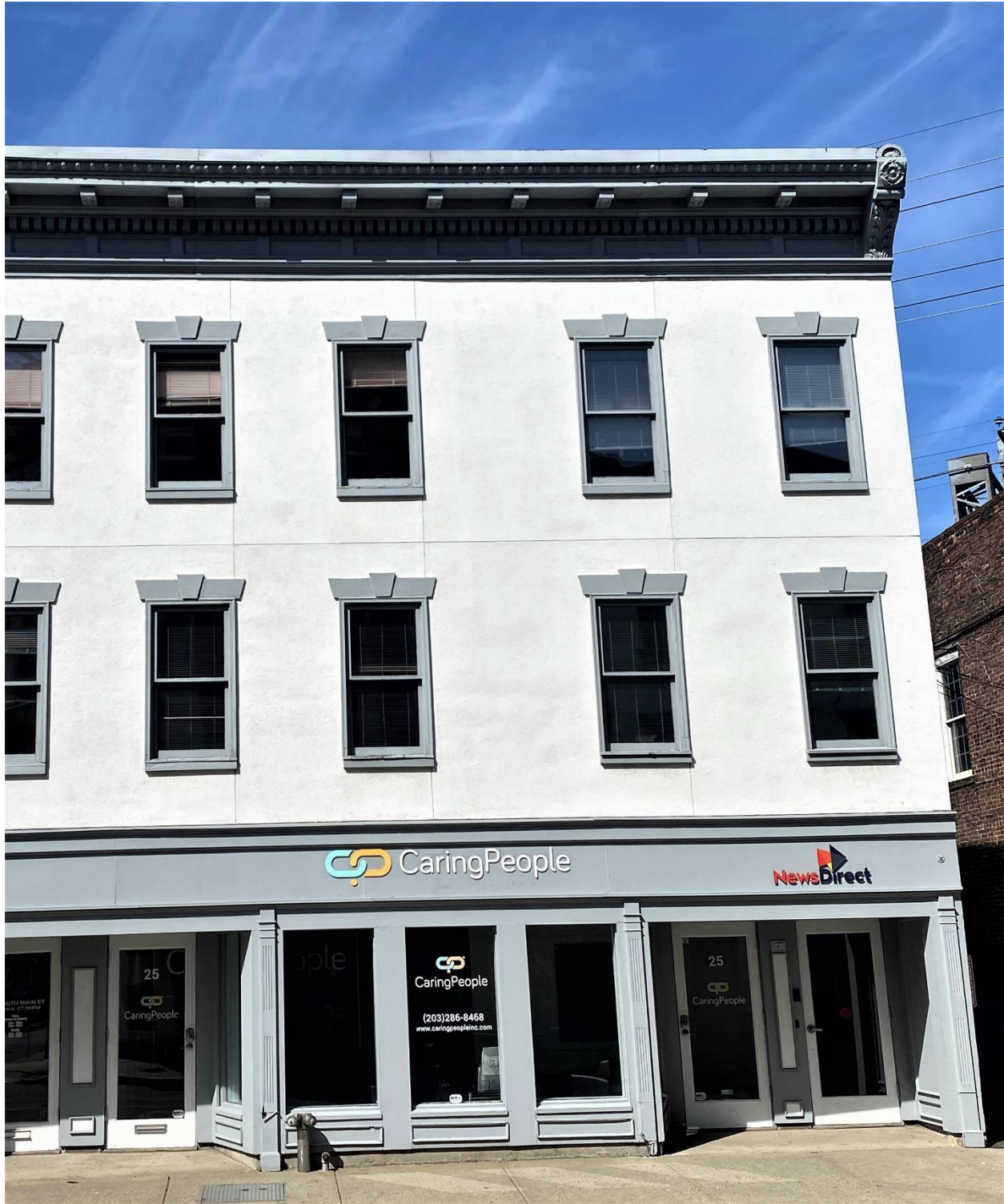
Photo 2 Expansion joints in the newer stucco application are not concealed, presenting an awkward grid appearance; the stucco is textured, unlike the original treatment.
