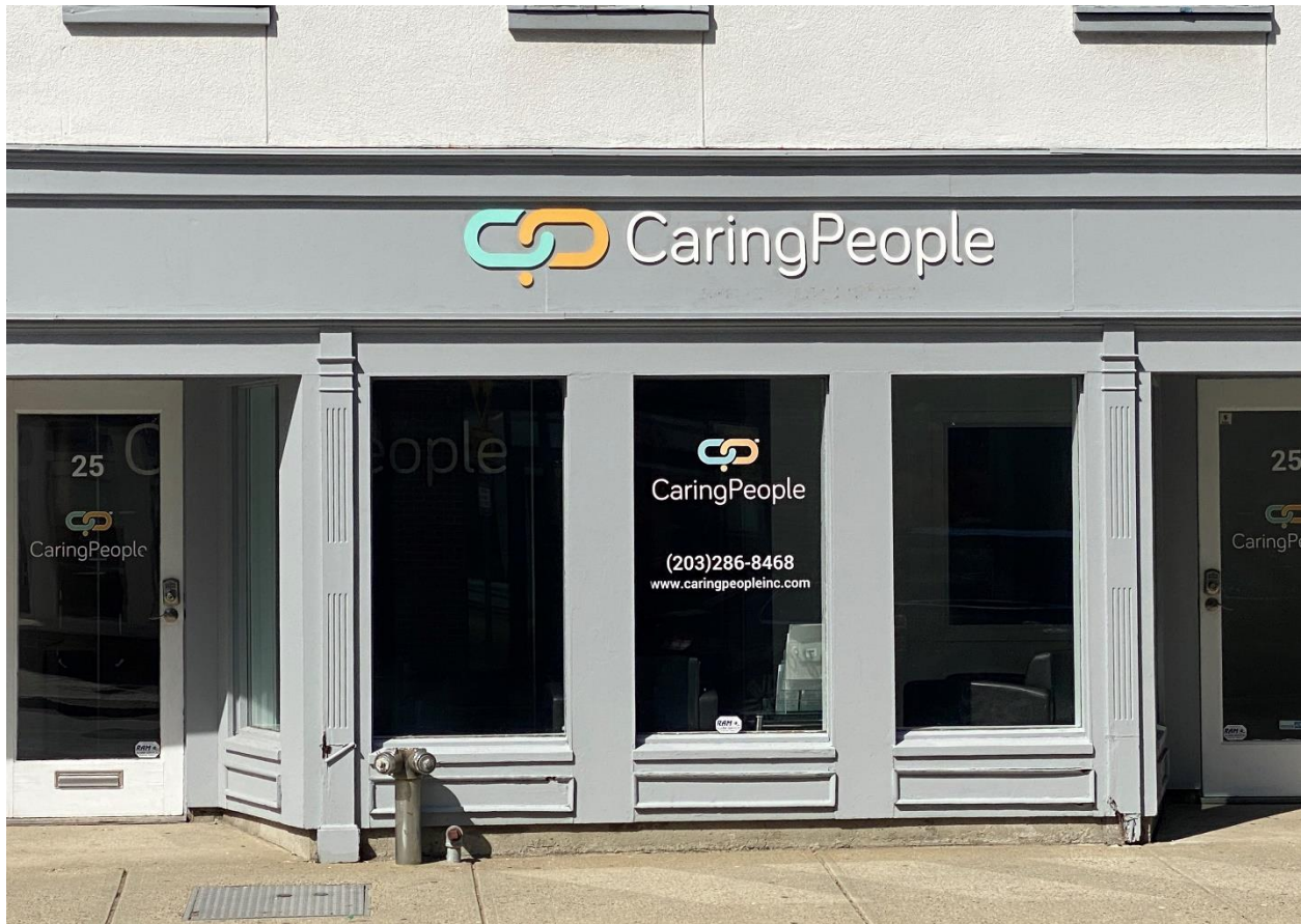
Photo 5 The ground floor commercial storefronts have been replaced, and do not match the originals.
