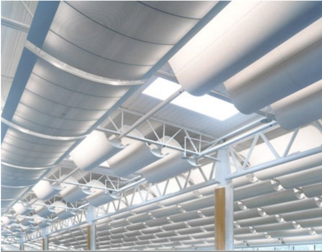
Photograph 15. View of ceiling detail, main floor, facing southwest.
