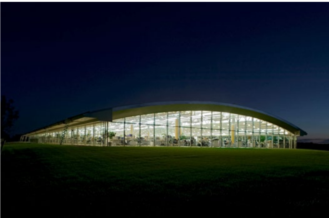
Photograph 6. View of east and north elevations at night, facing southwest.
