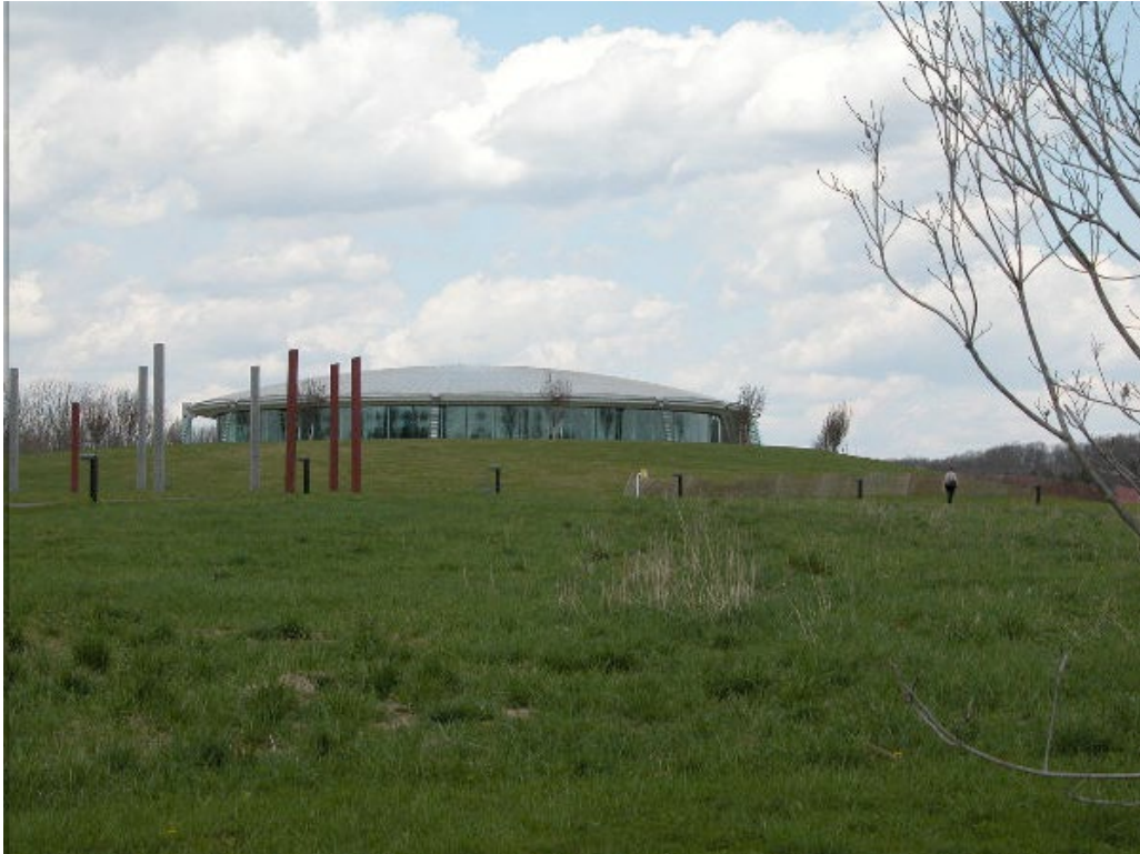
Photograph 3. View of south elevation, facing north.
