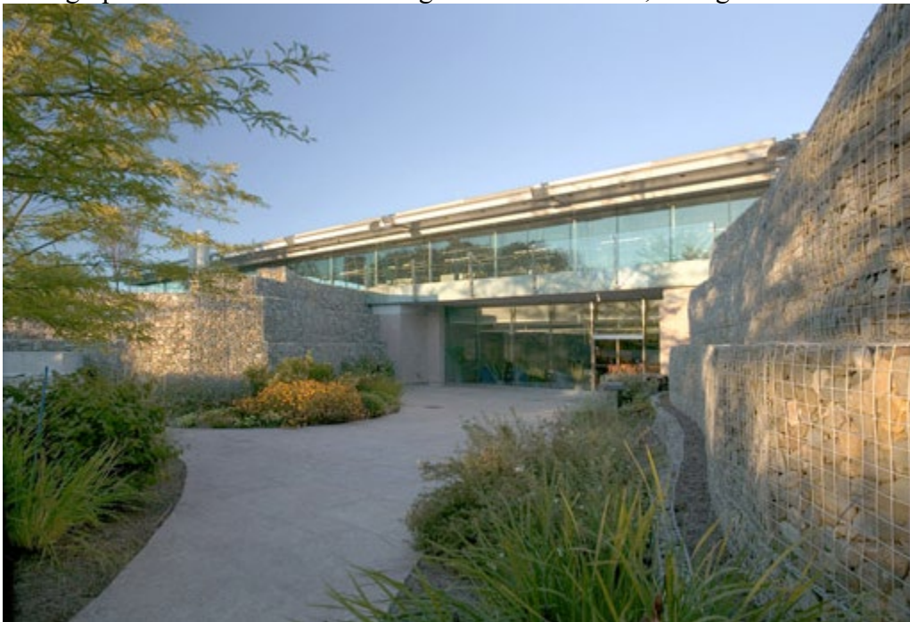
Photograph 8. View of entrance on east elevation, facing southwest.
