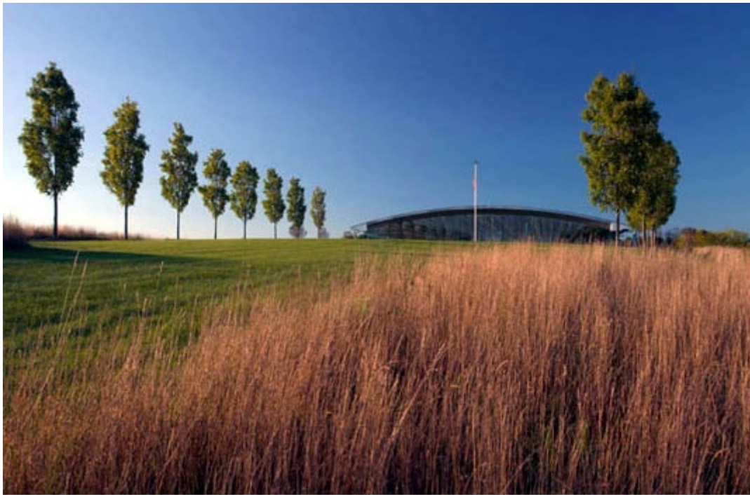
Photograph 4. View of north elevation and meadow, facing south.
