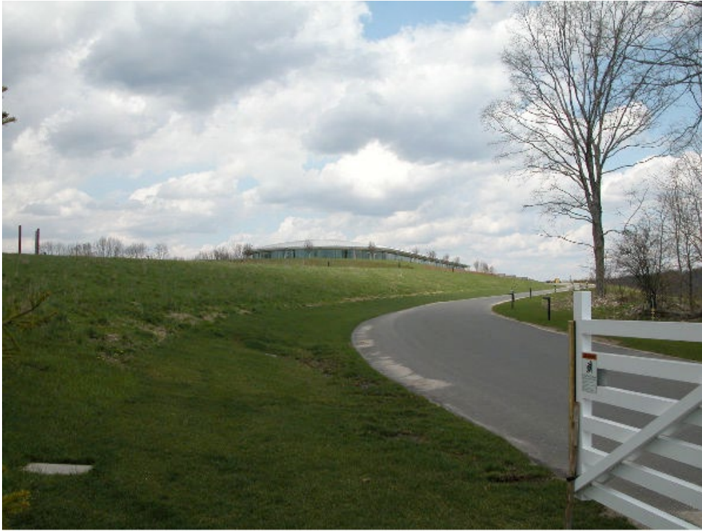
Photograph 1. View of setting from Timex Road, facing northwest.
