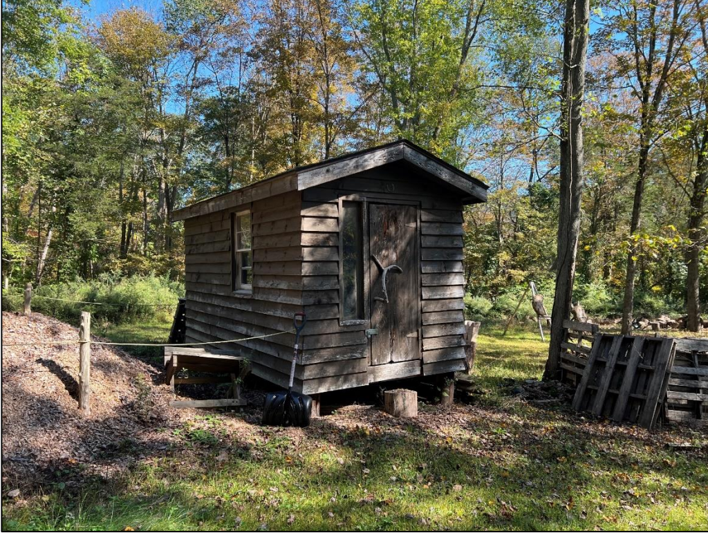
Photograph 31 – Looking northeast at the small cabin on the grounds of the Scout camp.
