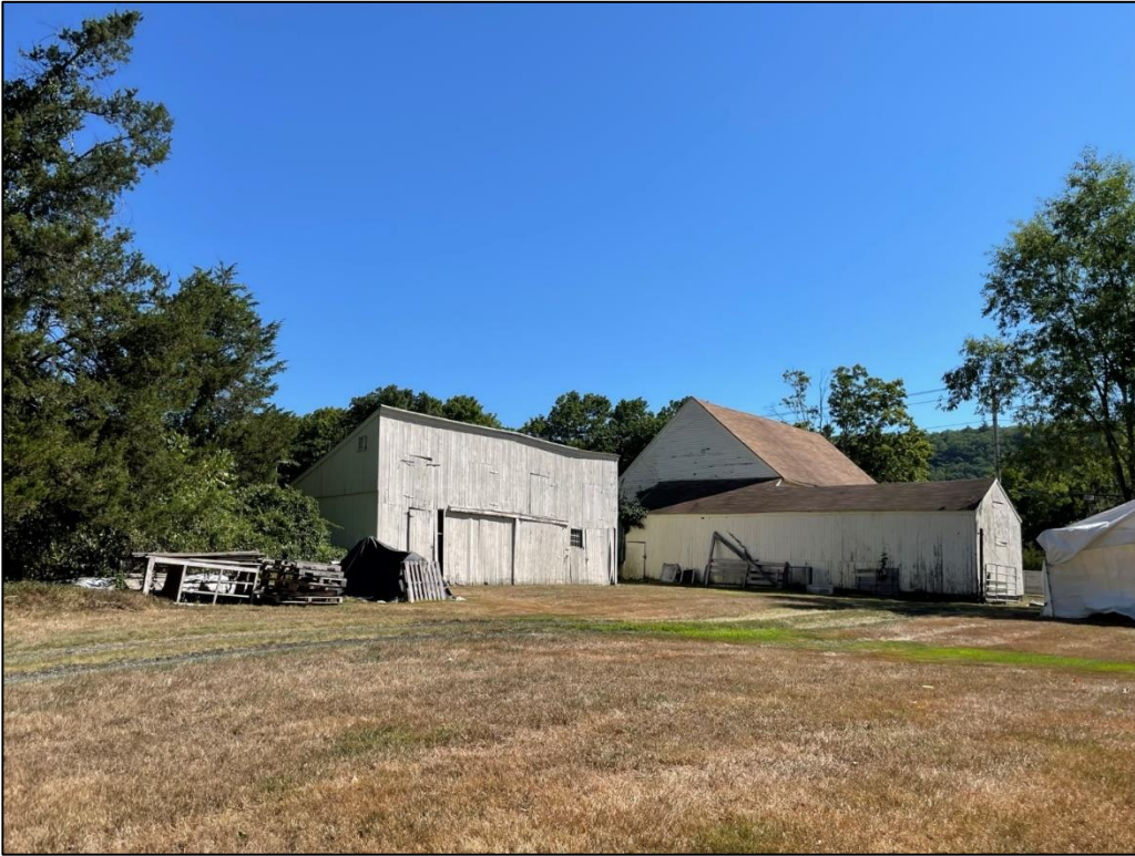
Photograph 14 – Looking northeast at the west barn with the cow barn and carriage shed behind it. (5412)
