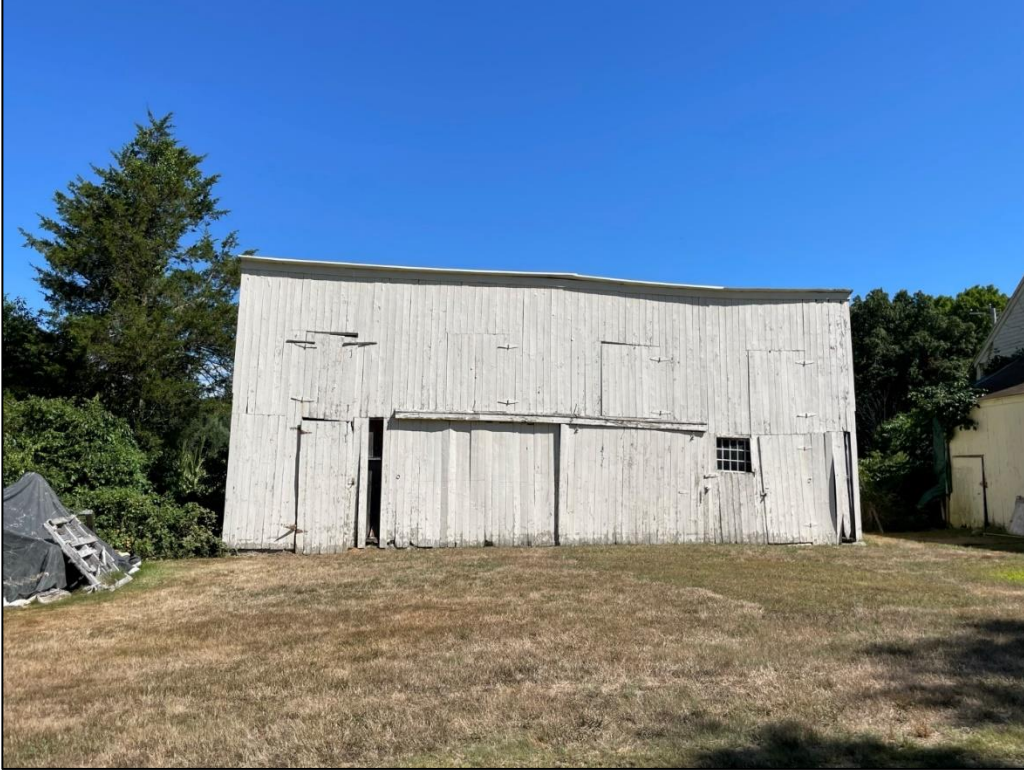
Photograph 13—Looking north at the south façade of the west barn. (5409)
