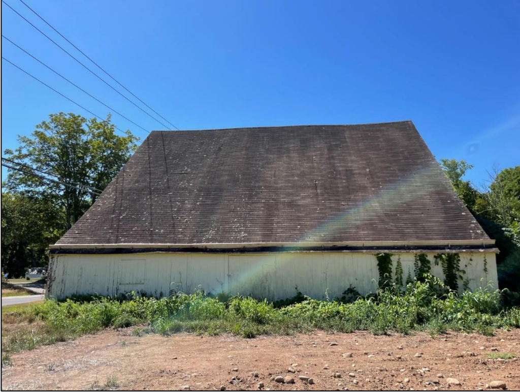
Photograph 7 – Looking south at the north side of the barn (5456)
