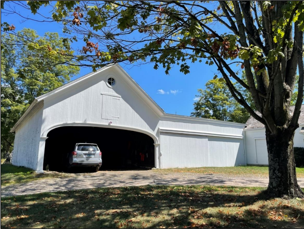
Photograph 10 – Looking northeast at the carriage barn (5464)
