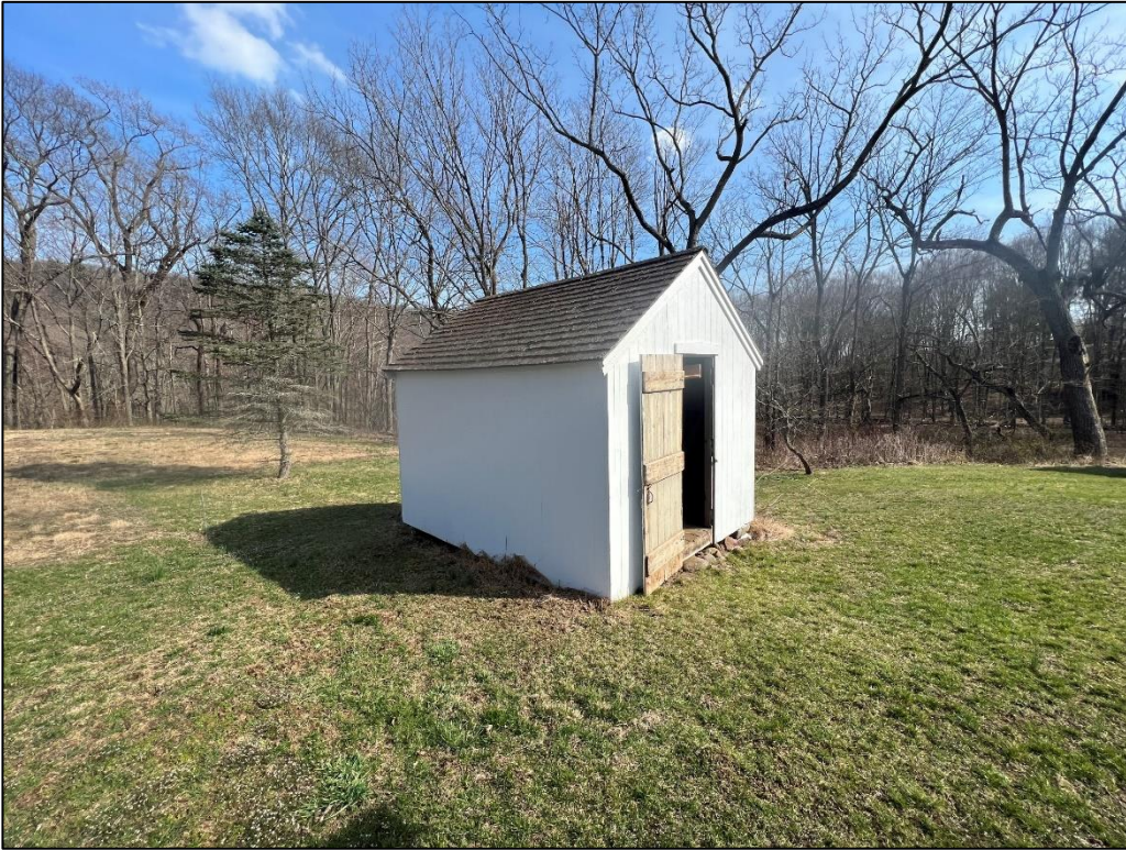
Photograph 19 – Looking southwest at the granary (5377)
