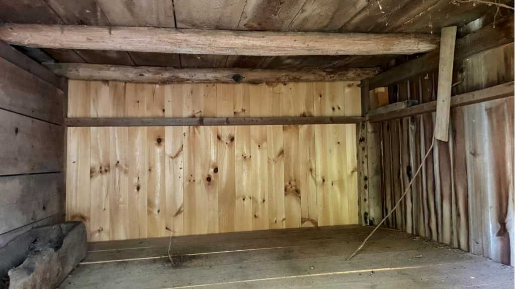
Photograph 21 – Looking north in the interior of the eastern section of the granary. (5381)
