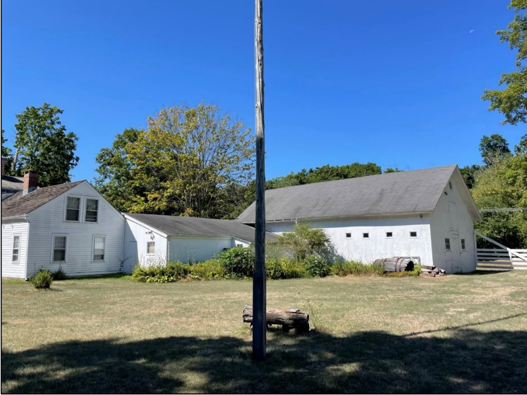
Photograph 11 – Looking southwest at the Stable (5399)
