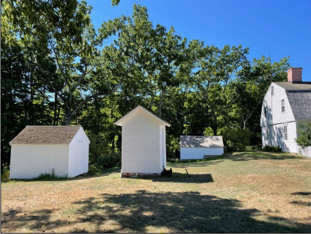
Photograph 23 – Looking south at the privy and other outbuildings behind the house. (5370)
