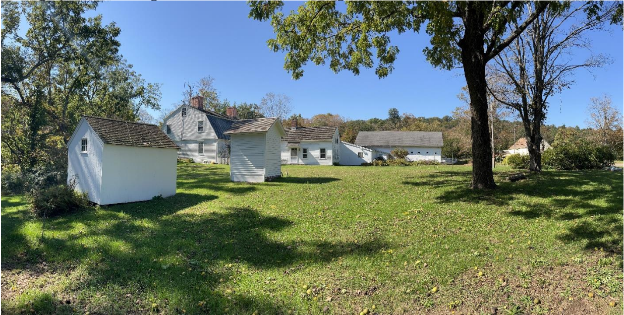
Photograph 2 – Looking west across the property. The granary is in the foreground left and the cow barn can be seen behind the trees in the background right.
