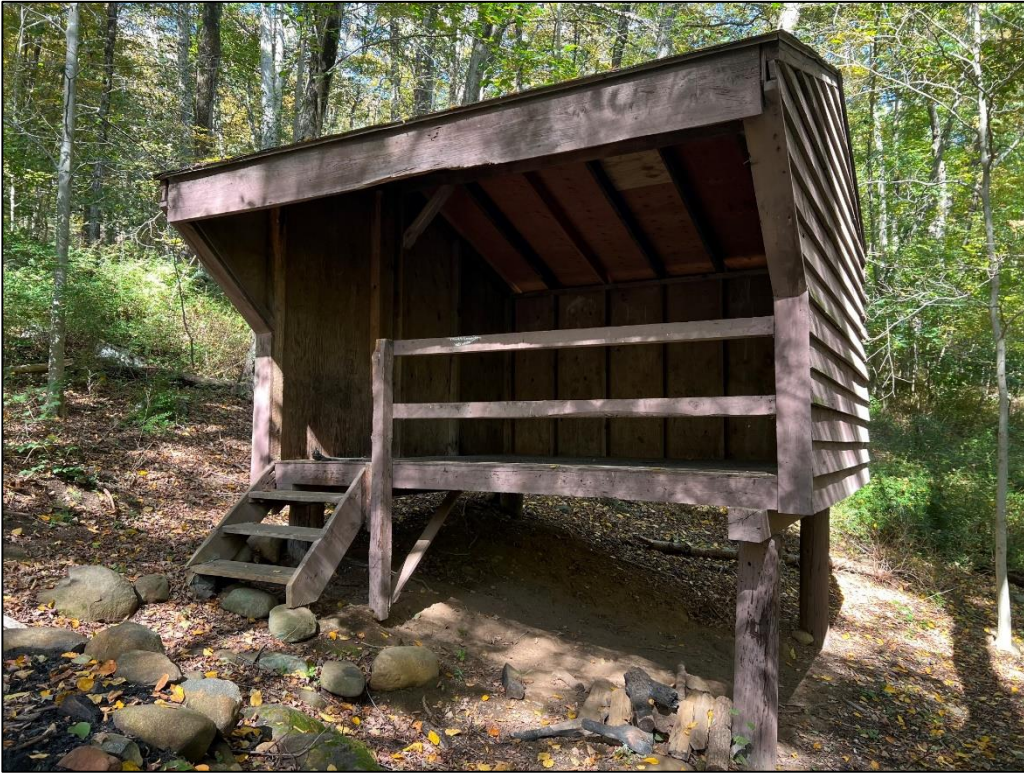
Photograph 30 – Looking northwest at the leanto on the grounds of the Scout camp. (9335)
