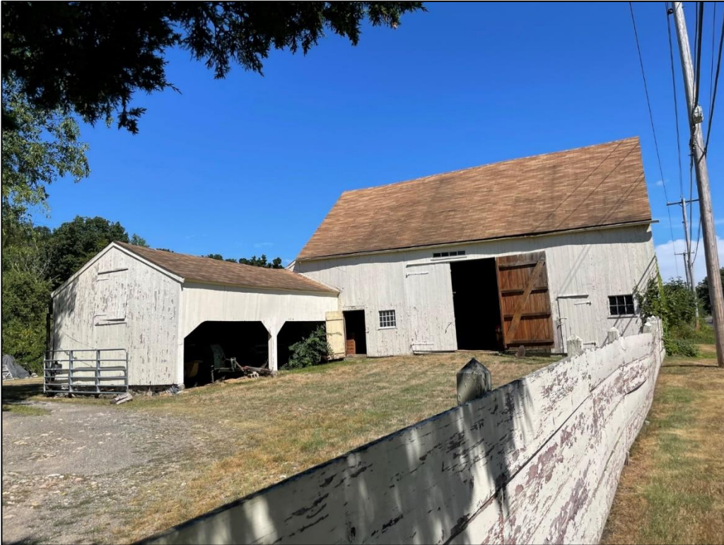
Photograph 6 – Looking north at the Cow Barn and attached wagon shed (5454)
