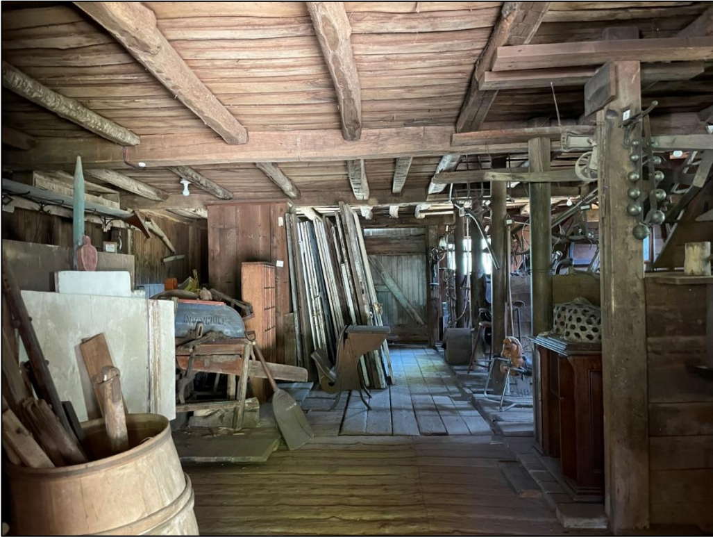
Photograph 12 – Looking north towards the north gable wall of the stable.
