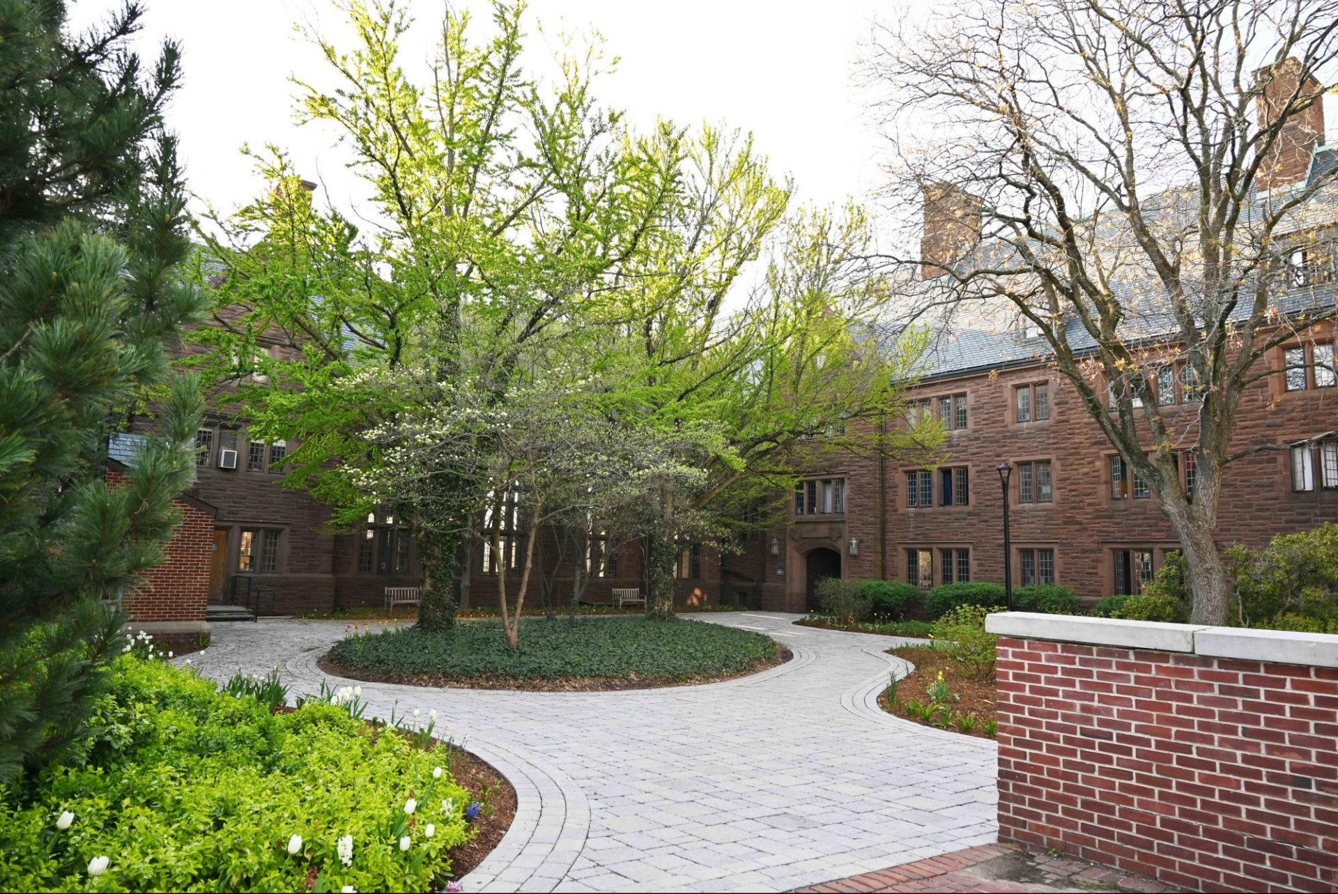
Mather Hall (far left), Hamlin Hall (center), and Cook Hall (right), camera facing northwest. Trinity College Long Walk Historic District Hartford County, Connecticut
