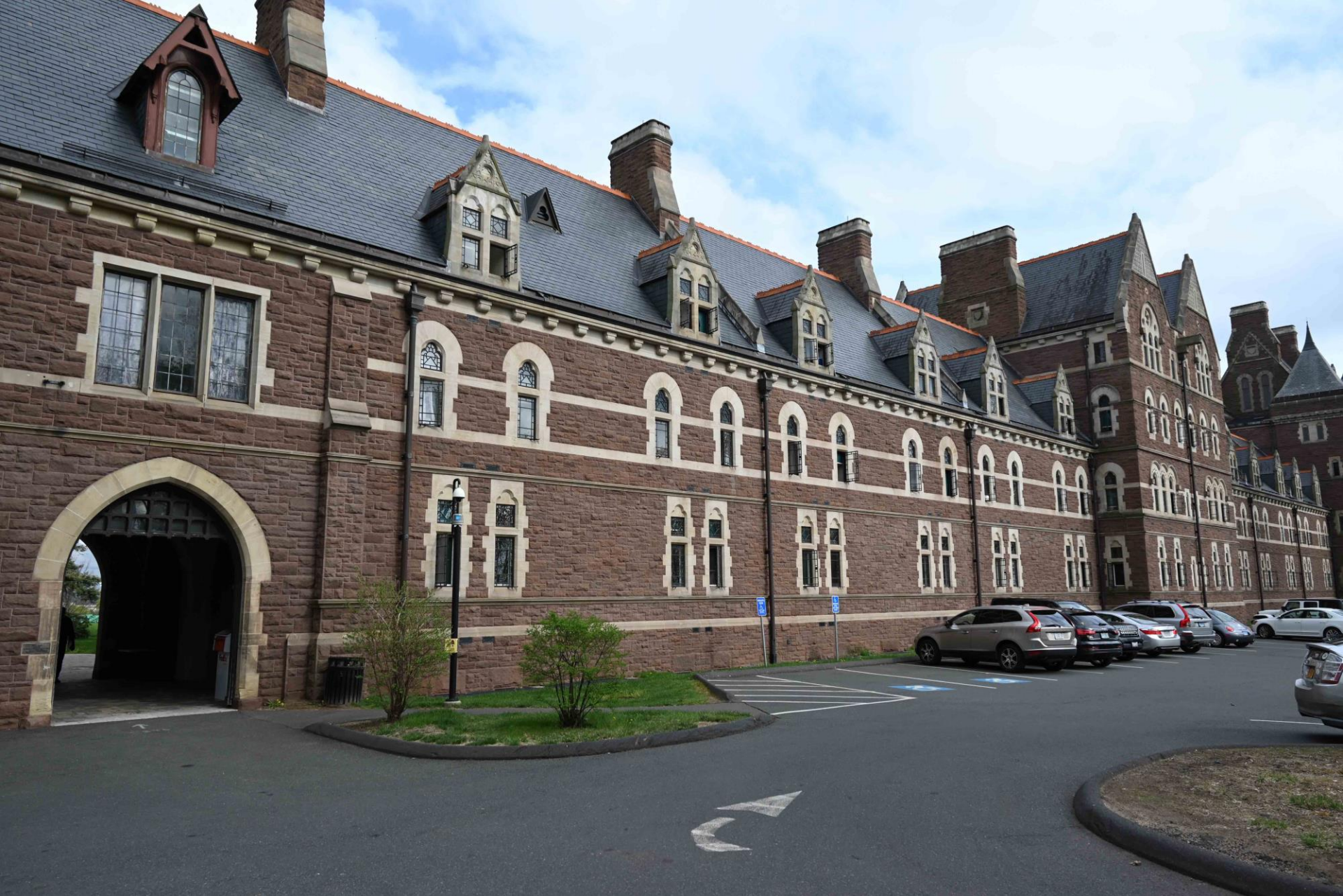
Jarvis Hall, camera facing southeast. Trinity College Long Walk Historic District Hartford County, Connecticut
