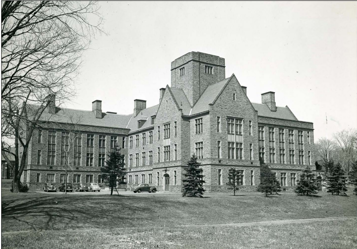
Figure 16. View of the Martin W. Clement Chemistry Laboratory, ca. 1945, camera facing northwest (from Trinity College Watkinson Library and College Archives).
