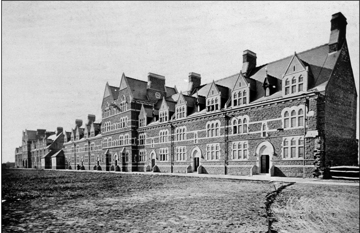
Figure 7. Long Walk view of east (Quad) side, camera facing southwest. Left to right: Seabury Hall and Jarvis Hall in 1878, before construction of Northam Towers (from Trinity College Watkinson Library and College Archives).
