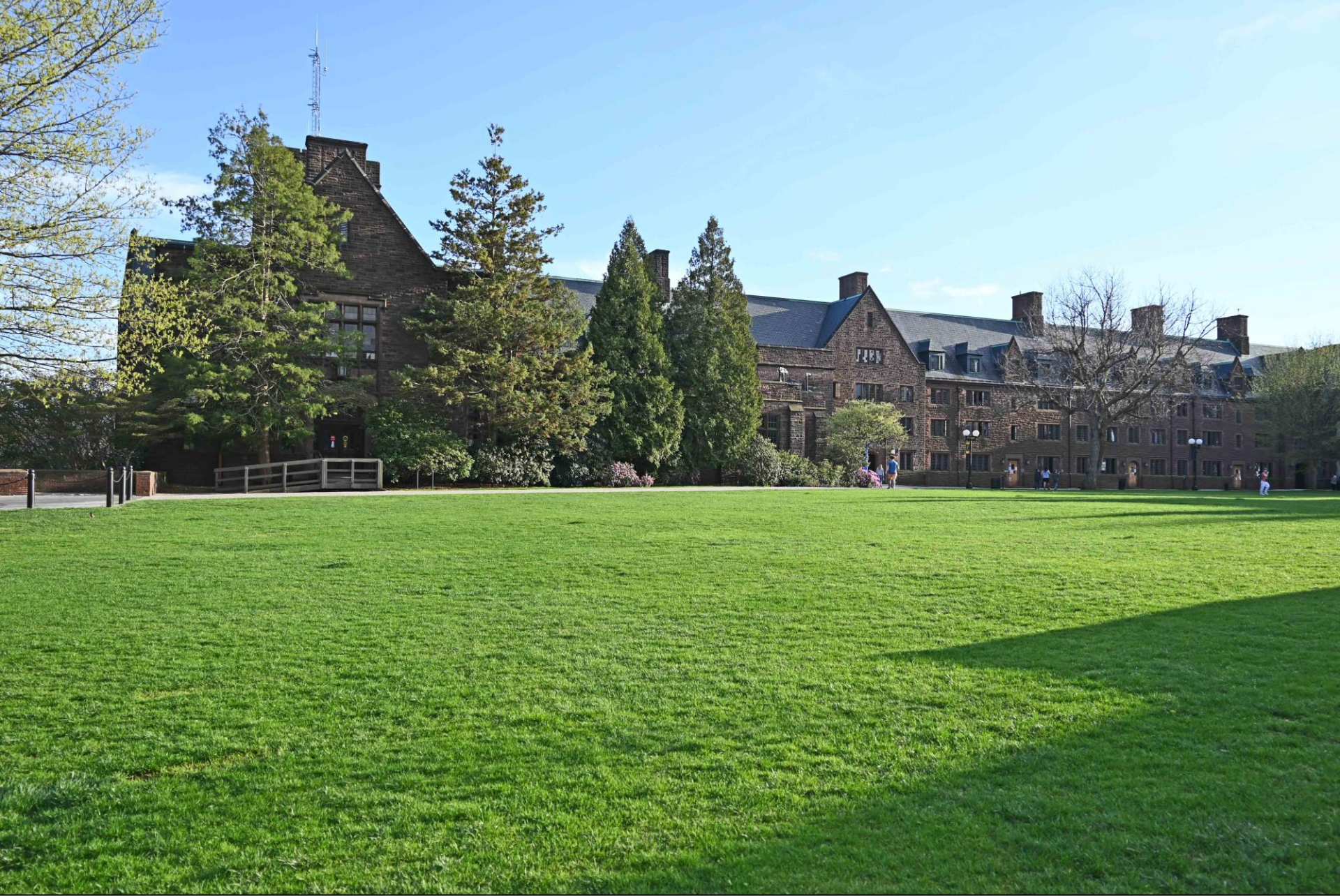
Martin W. Clement Chemistry Laboratory (left), Goodwin-Woodward Hall, and Cook Hall (right), camera facing south. Trinity College Long Walk Historic District Hartford County, Connecticut
