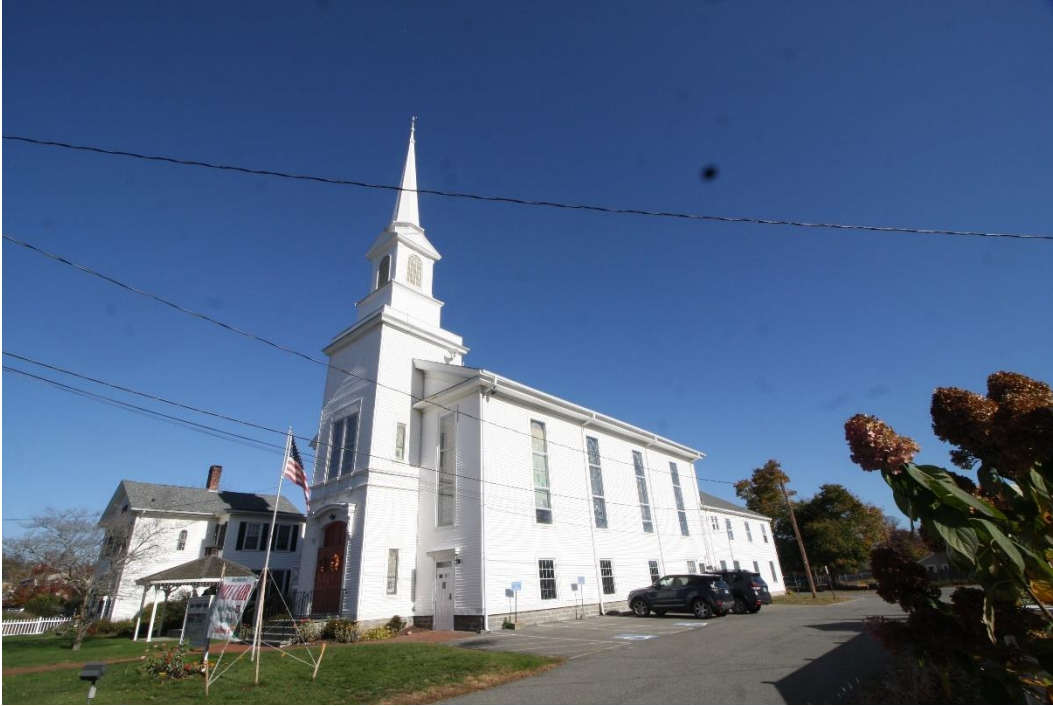
Photograph 11 of 14. Looking east at 10 Commerce Street (1855), the Clinton United Methodist Church.
