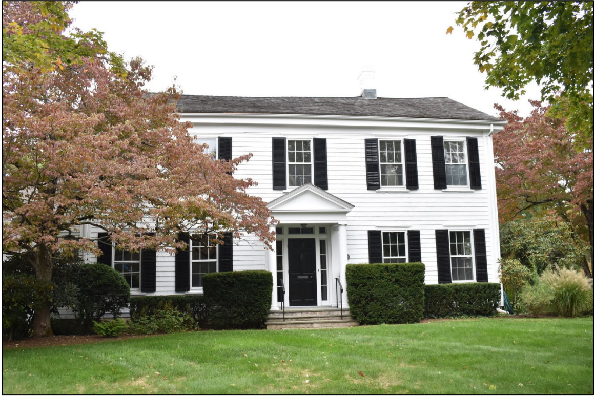
11 of 30. Town House, 13 Oenoke Ridge, facing north.
