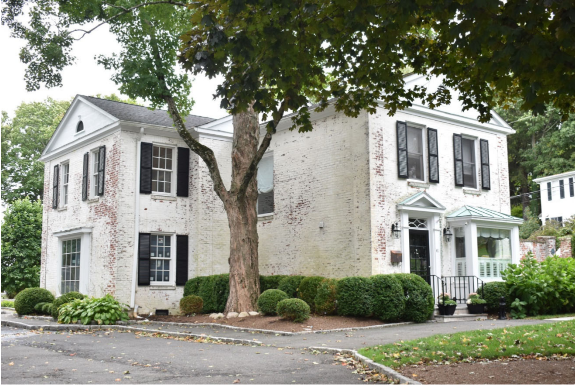
17 of 30. 41 Park Street, facing northwest.
