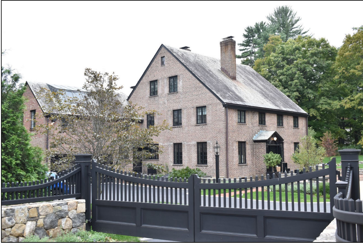
7 of 30. Frederick F. Fisher House, 40 Oenoke Ridge, facing southwest.
