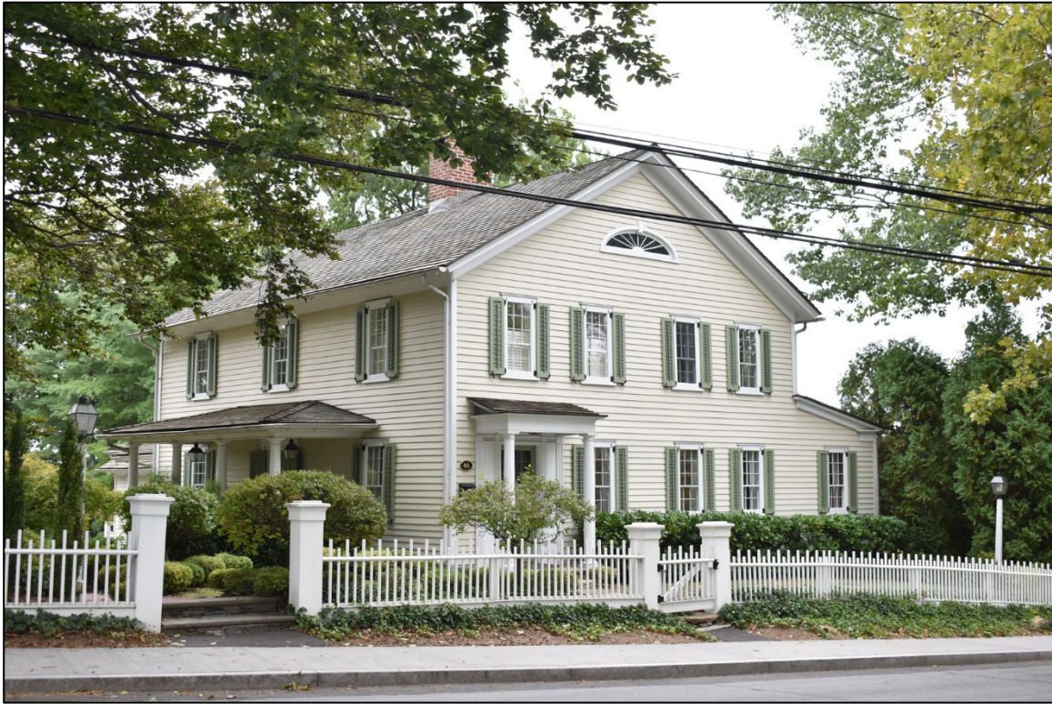
4 of 30. Husted-St. John House, 46-48 Park Street, facing southeast.
