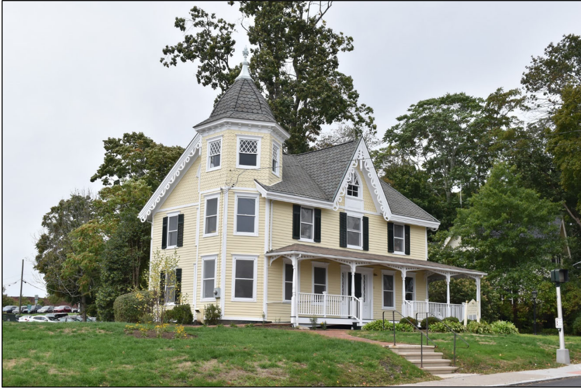
19 of 30. Vine Cottage, 61 Main Street, facing southwest.
