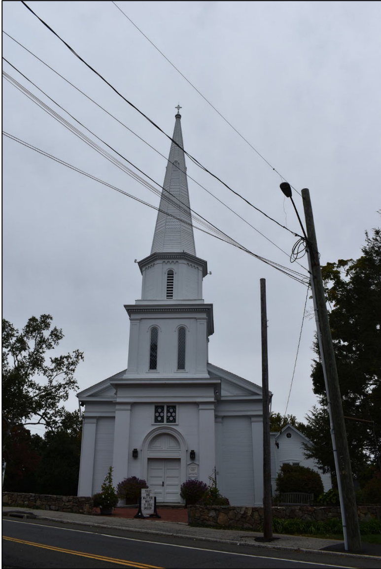
12 of 30. St. Mark's Episcopal Church/St. Michaels Lutheran Church, 5 Oenoke Ridge, facing north.
