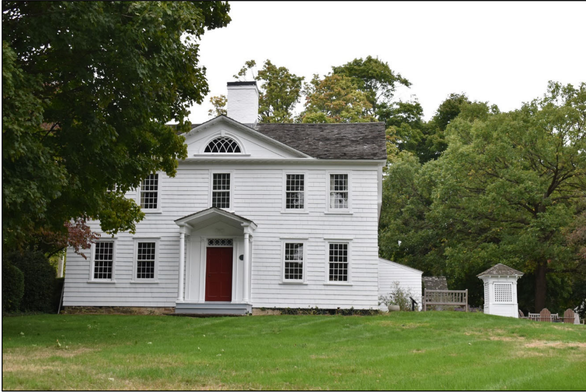
9 of 30. Hanford-Silliman House and Wellhouse, 13 Oenoke Ridge, facing north.
