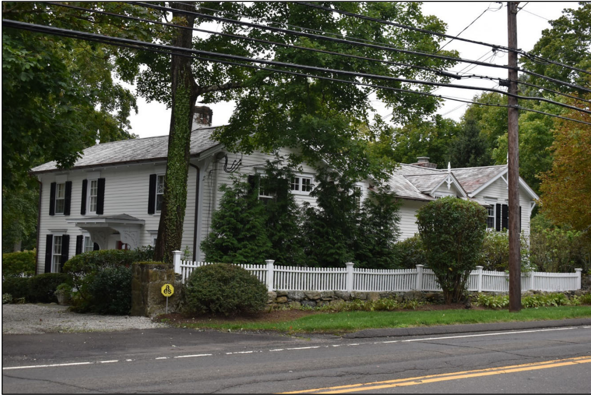
8 of 30. Second Episcopal Manse, 24–30 Oenoke Ridge, facing southwest.
