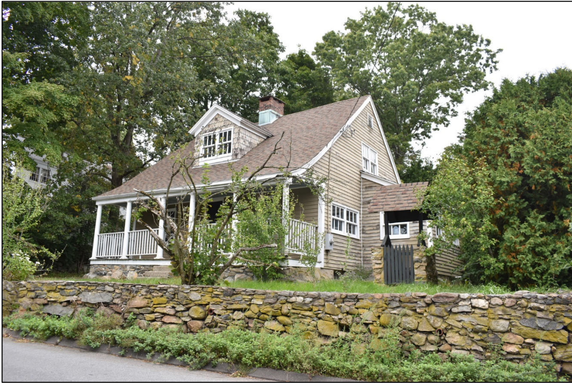
28 of 30. Eleazer Bouton House and Wellhouse, 97 Seminary Street, facing northwest.
