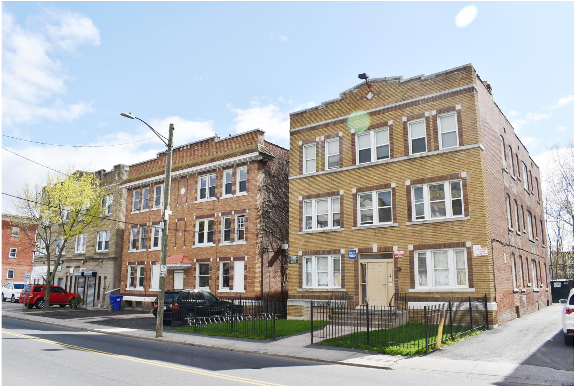
9. 179 Mather Street, 398–400 and 396–394 Garden Street, looking northwest (left to right)
