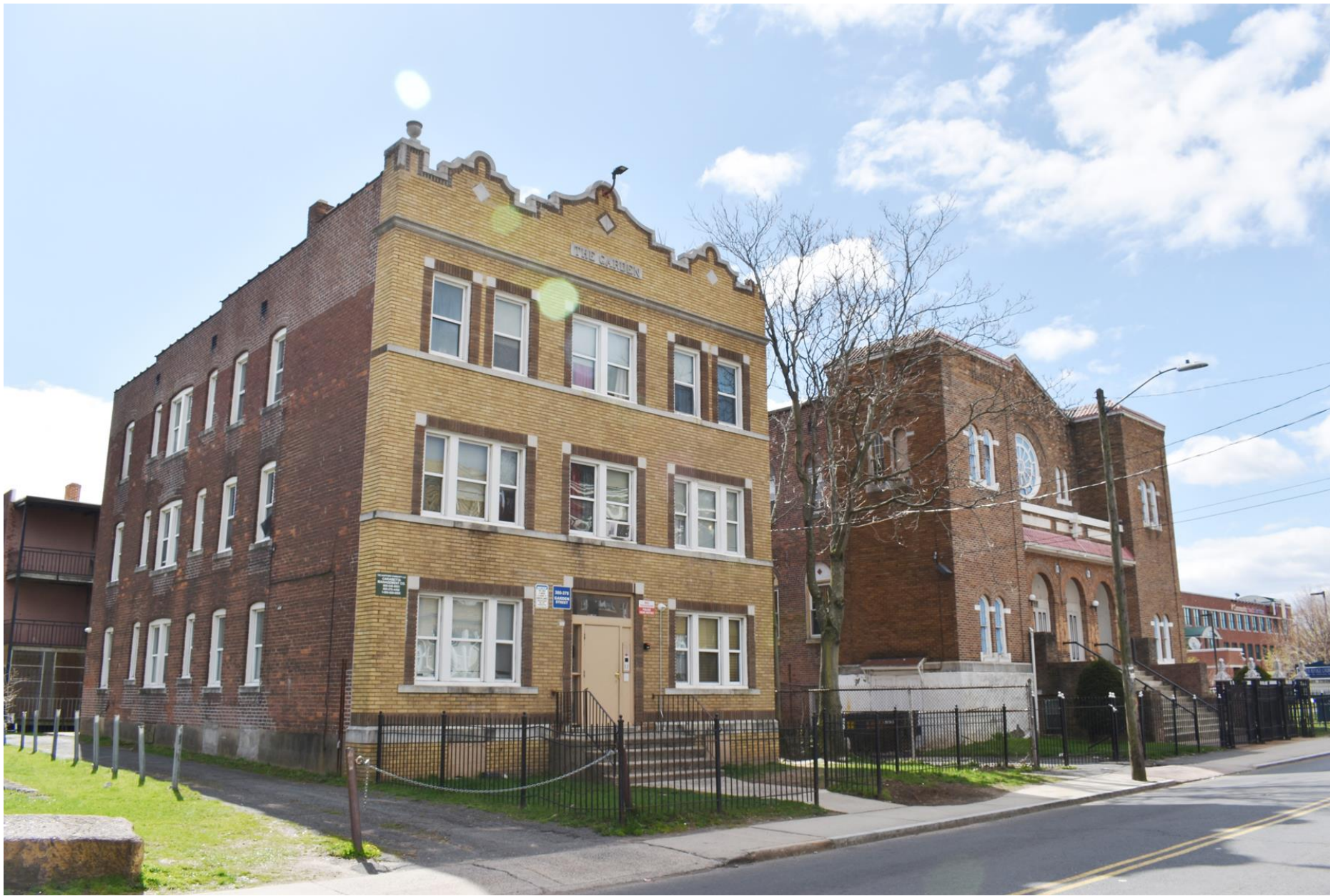
13. 378–380 & 370 Garden Street (former Beth Hamedrash Hagodol Synagogue), looking southeast (left to right)
