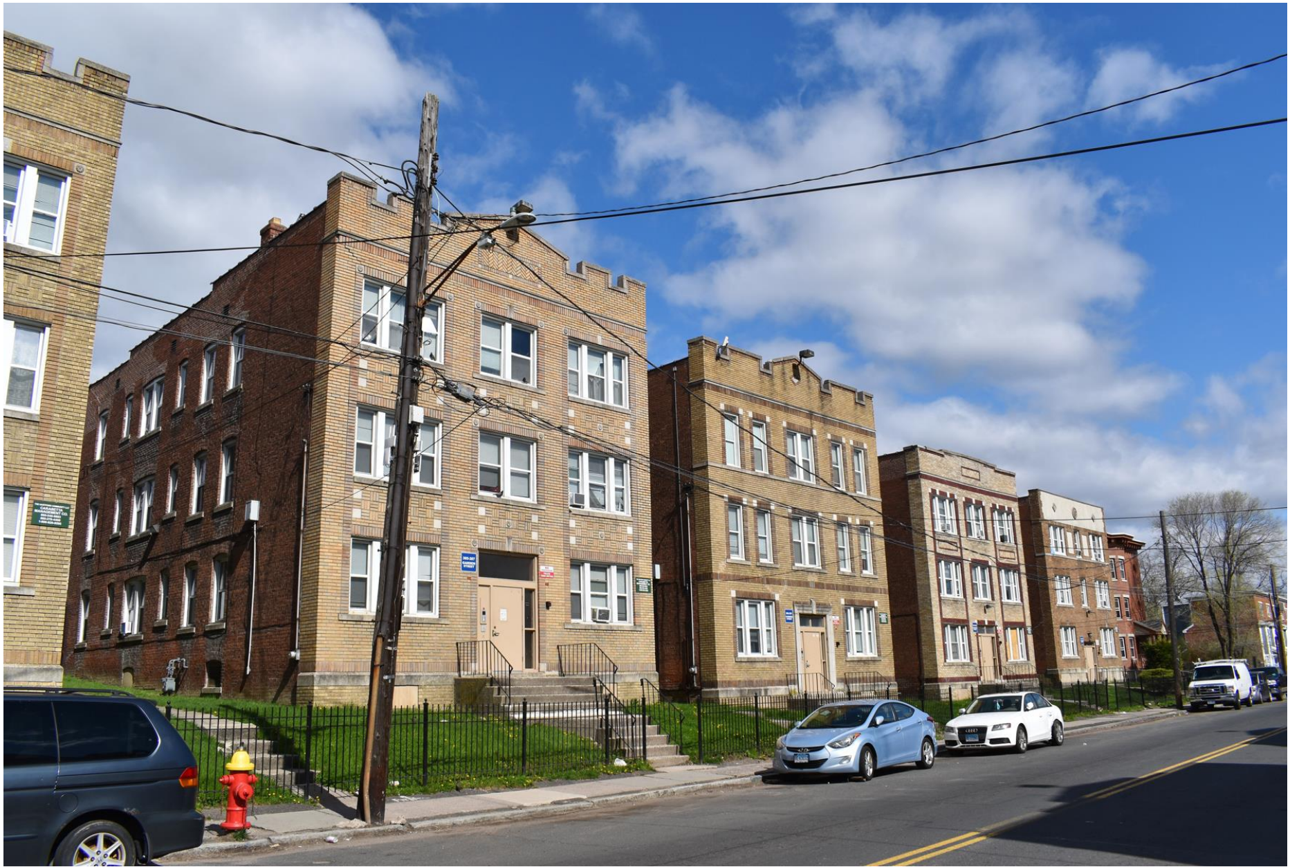
10. 387–399 Garden Street, looking northwest (left to right)
