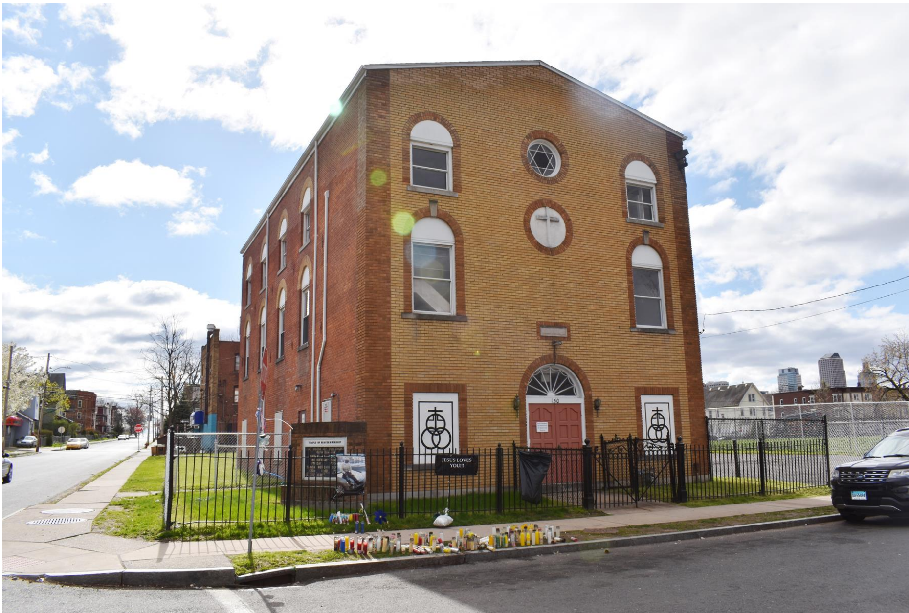
6. 148–150 Bedford Street (former Lomday Mishnays Synagogue), looking east
