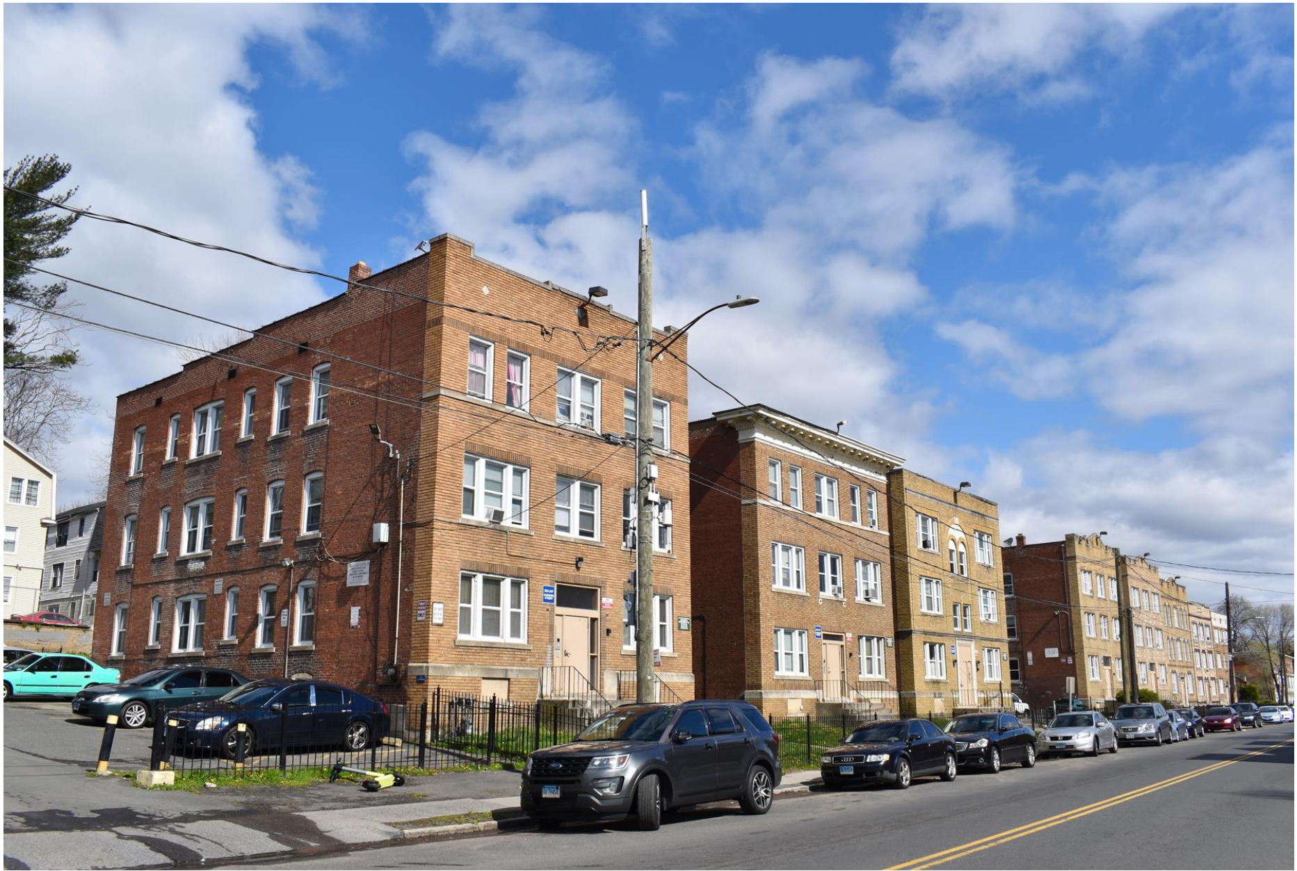
12. 377–399 Garden Street, looking northwest (left to right)
