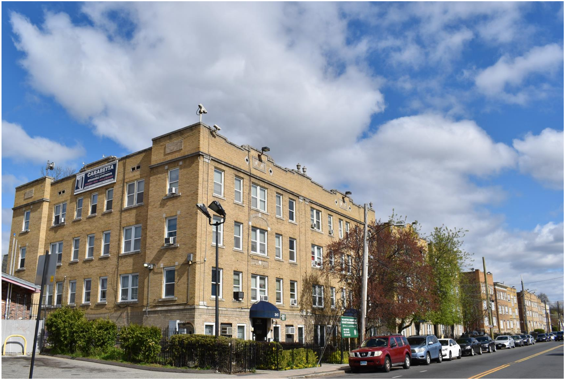
19. 343–387 Garden Street, looking northwest (left to right)
