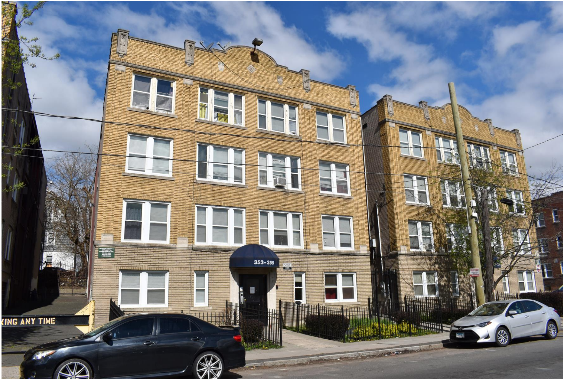
18. 353–359 Garden Street, looking northwest (left to right)
