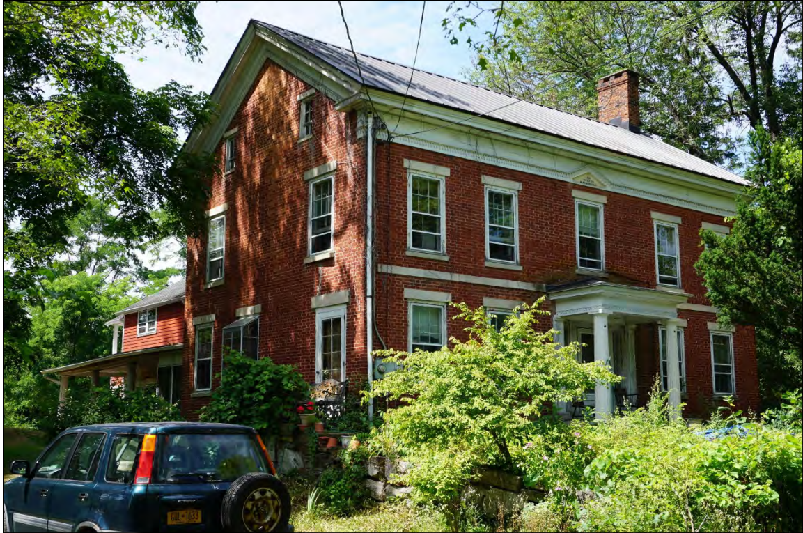
PHOTO 13: Henry Morehouse House, 257 Leedsville Rd., 1843.
