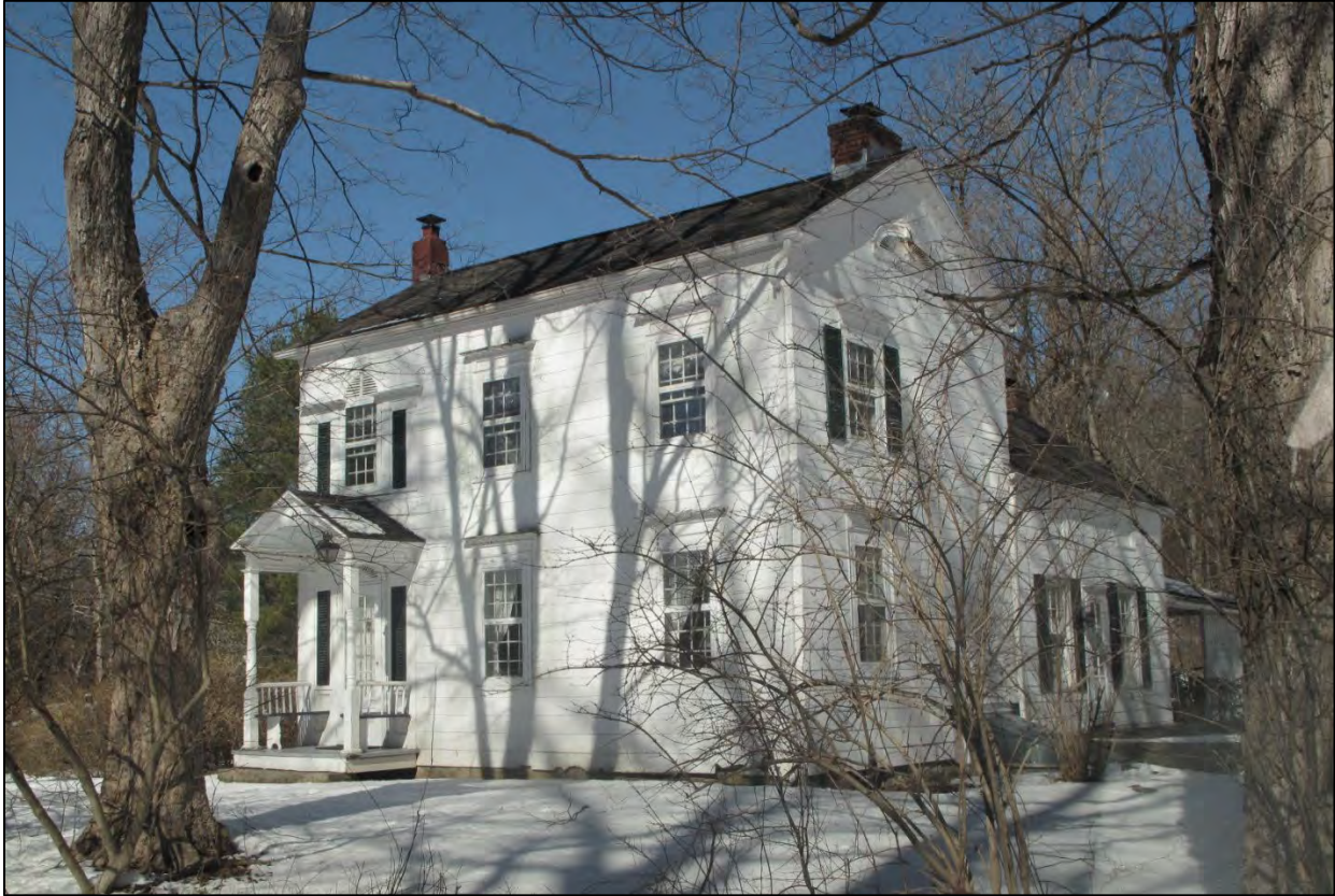
PHOTO 9: Hollister house at 442 Leedsville Rd.
