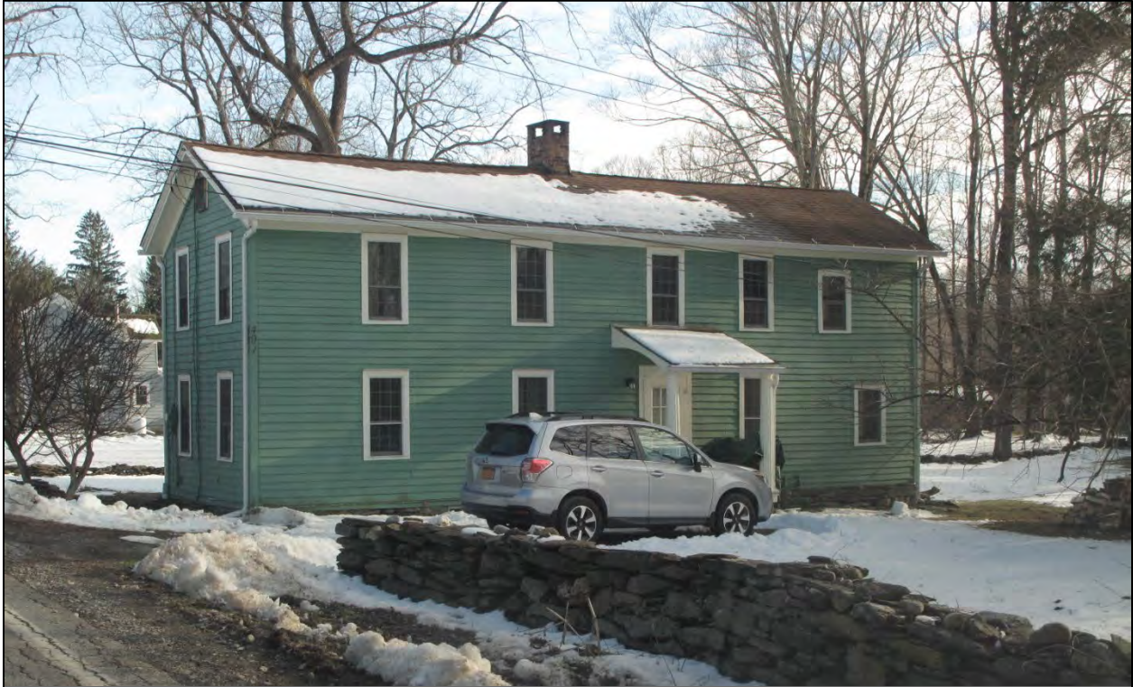
PHOTO 5: Dormitory building at 491 Leedsville Rd., ca. 1810.
