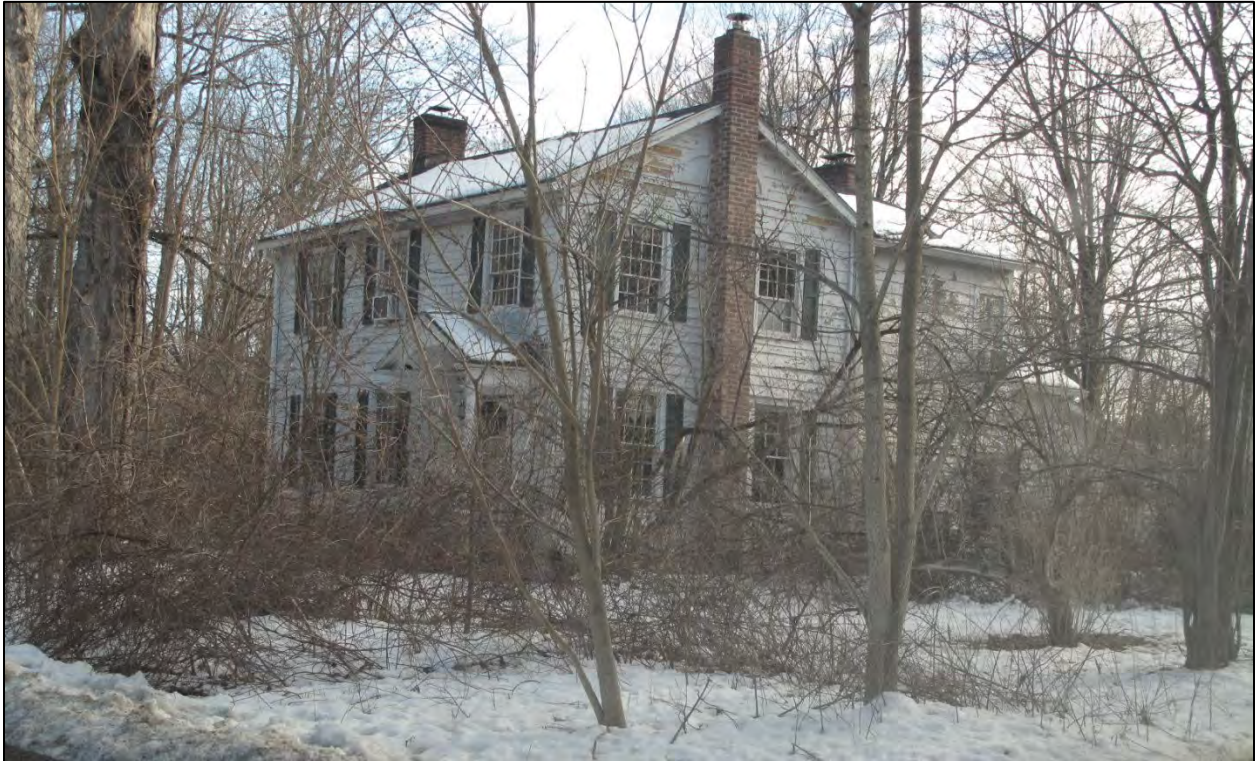
PHOTO 8: House at 441 Leedsville Rd.
