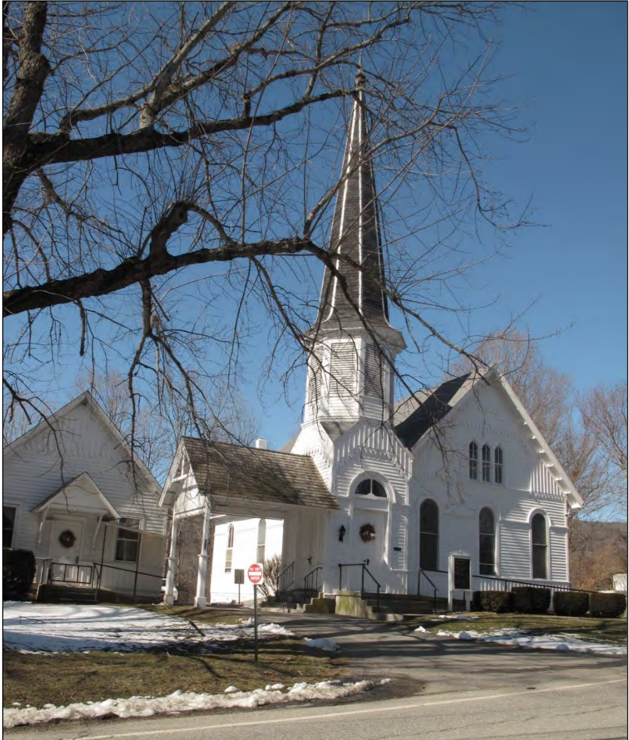
PHOTO 38: South Amenia Presbyterian Church, 229 S. Amenia Rd., 1880.
