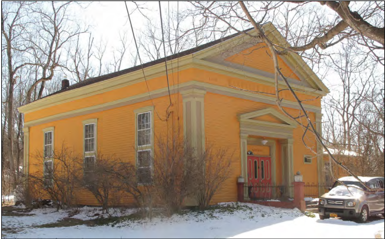
PHOTO 18: Amenia Union Methodist Church, 292 Amenia Union Rd., 1859.
