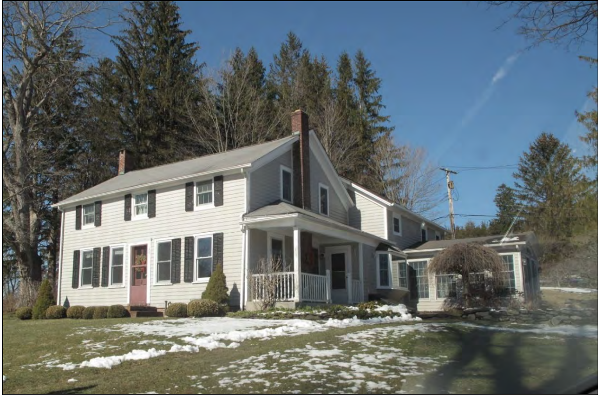
PHOTO 14: Delamater-Sherman House, 176 Leedsville Rd.
