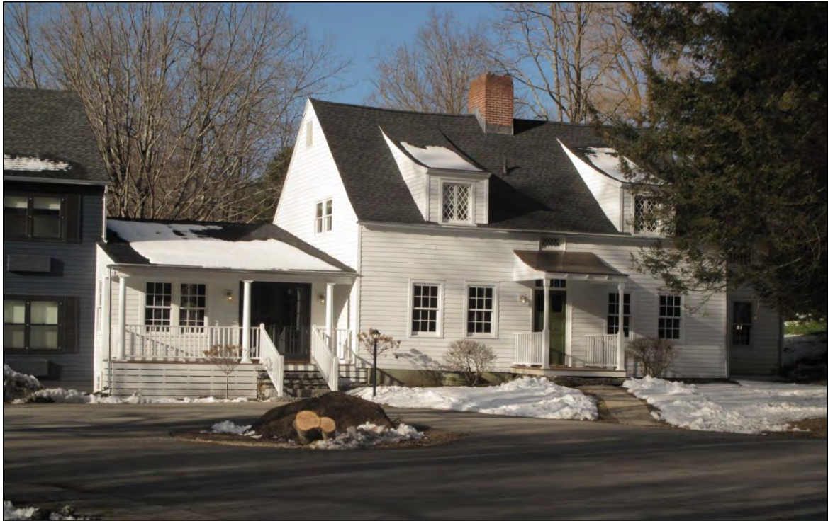
PHOTO 2: Joel Benton House, 12-26 Troutbeck Ln., ca. 1795.
