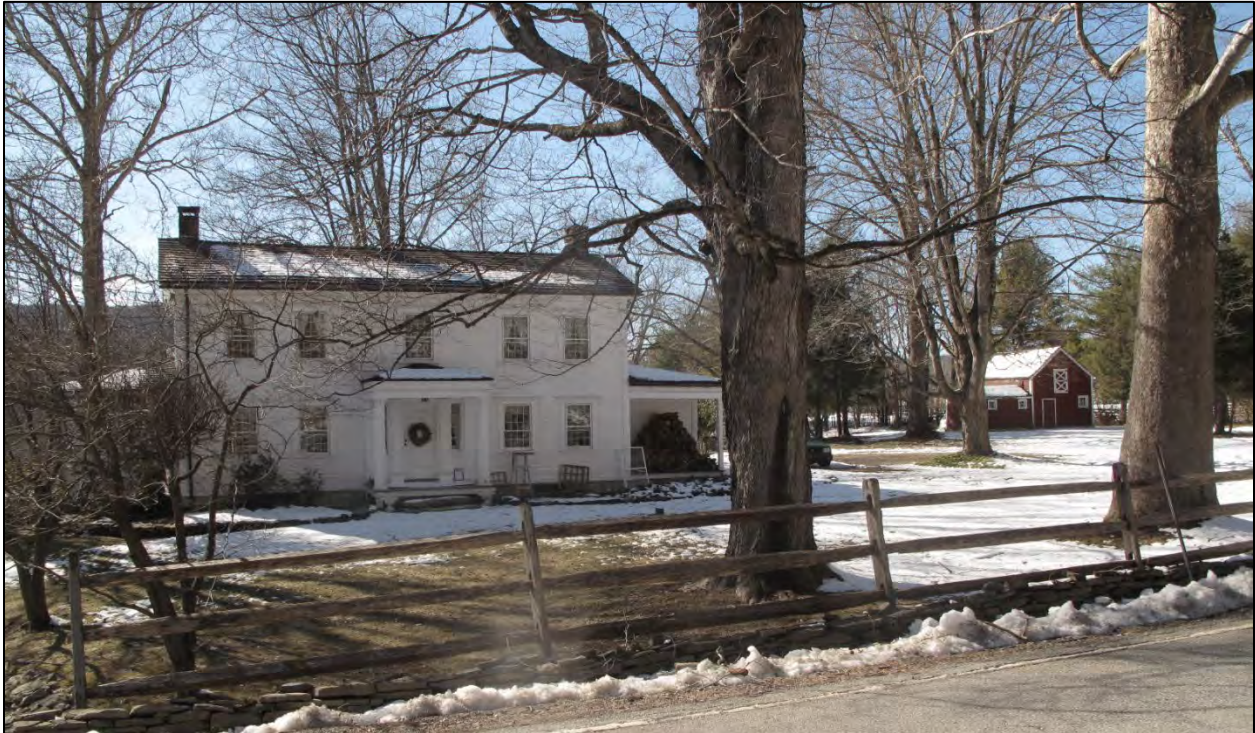
PHOTO 10: Hollister Farmhouse, 413 Leedsville Rd., ca. 1835.
