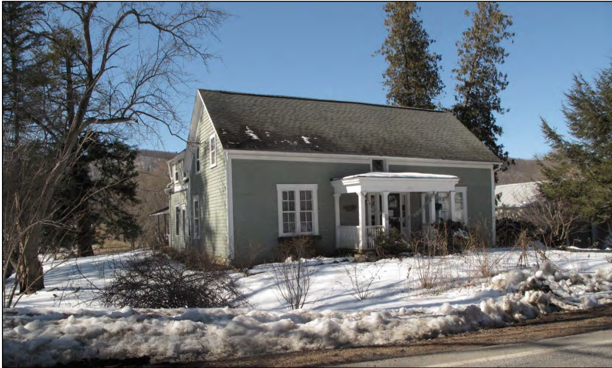
Photo 27: Delamater-Reed House, 103 Amenia Union Rd., contains house dating from ca. 1740.
