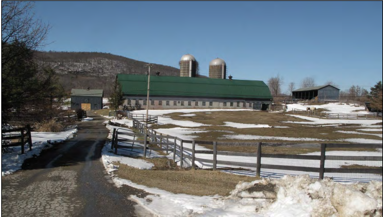
PHOTO 31B: Dairy Barn at 17 Amenia Union Rd.
