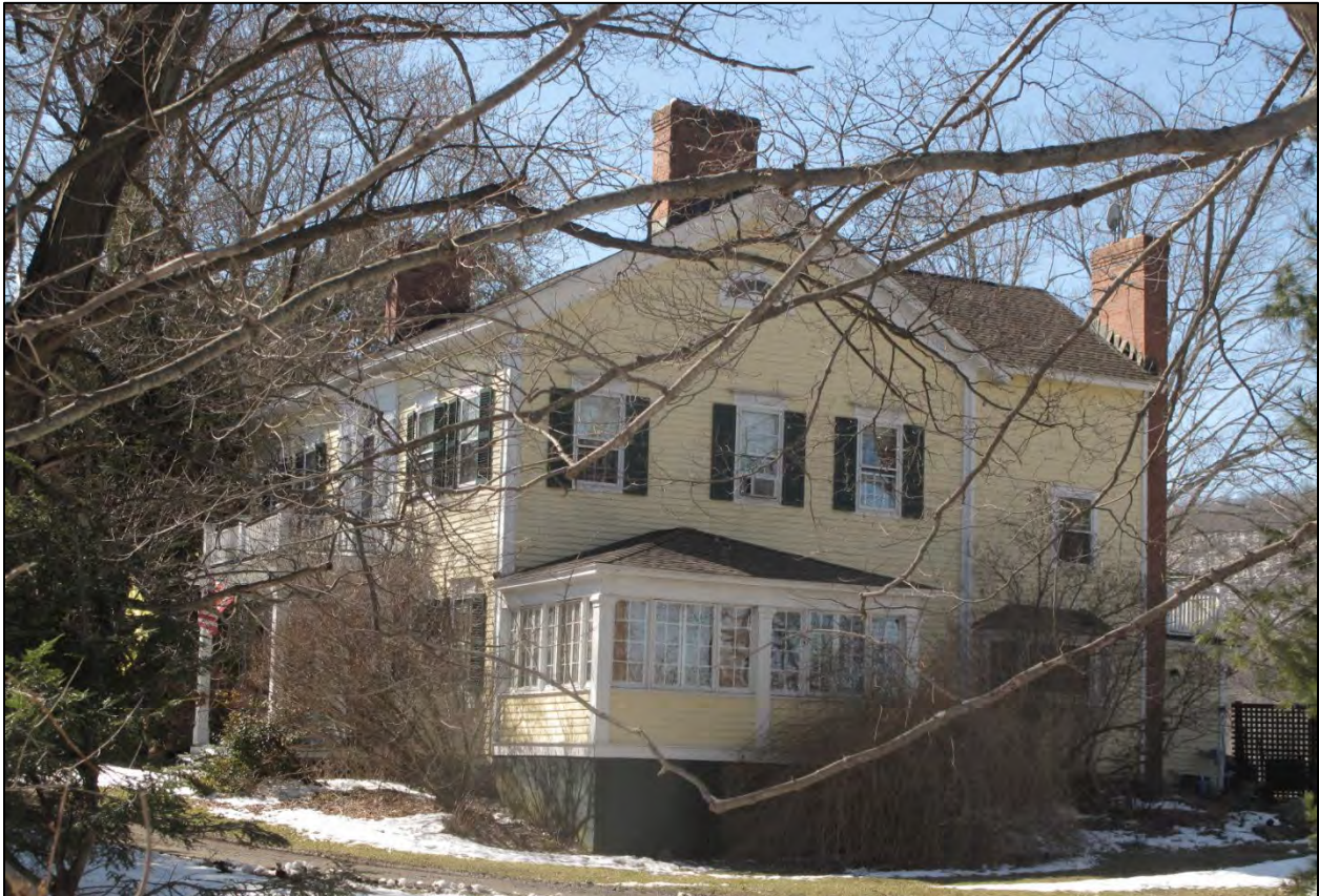
PHOTO 30: Swift-Cline House, 17 Amenia Union Rd., 1815.
