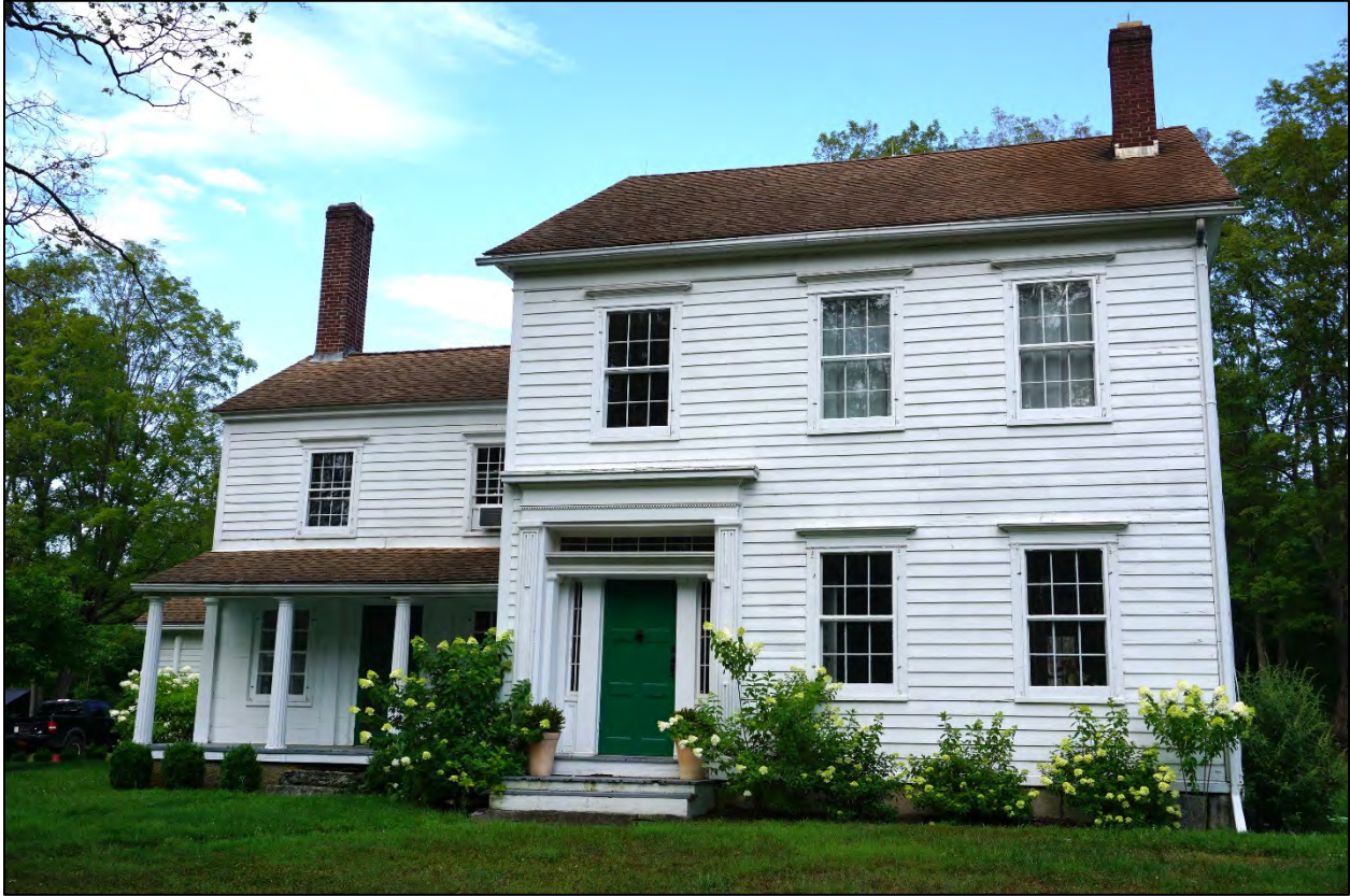
PHOTO 7: House at 496 Leedsville Rd.
