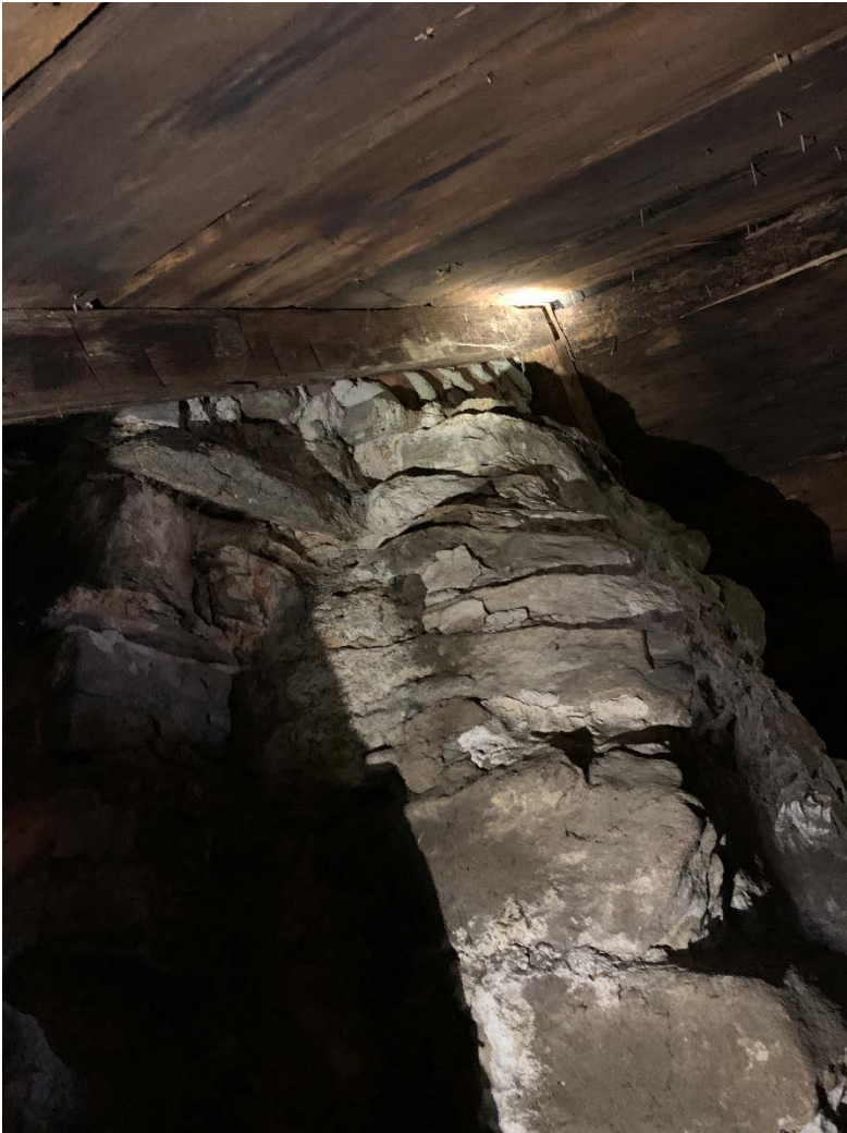
23 of 25. Attic, chimney, looking north.
