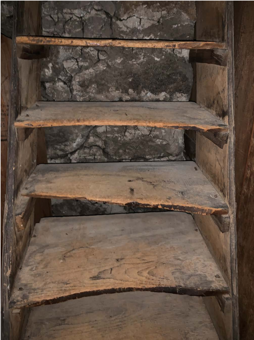
22 of 25. Attic ladder, looking northeast.
