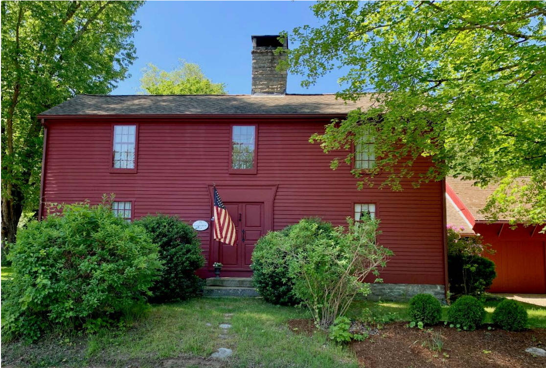
1 of 25. Caleb Pratt House, northeast elevation, looking southwest.
