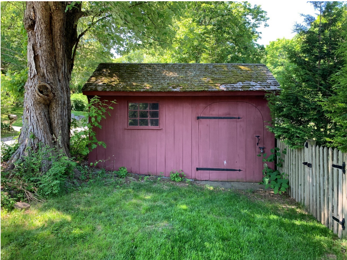
6 of 25. Tool shed, northeast elevation, looking southwest.
