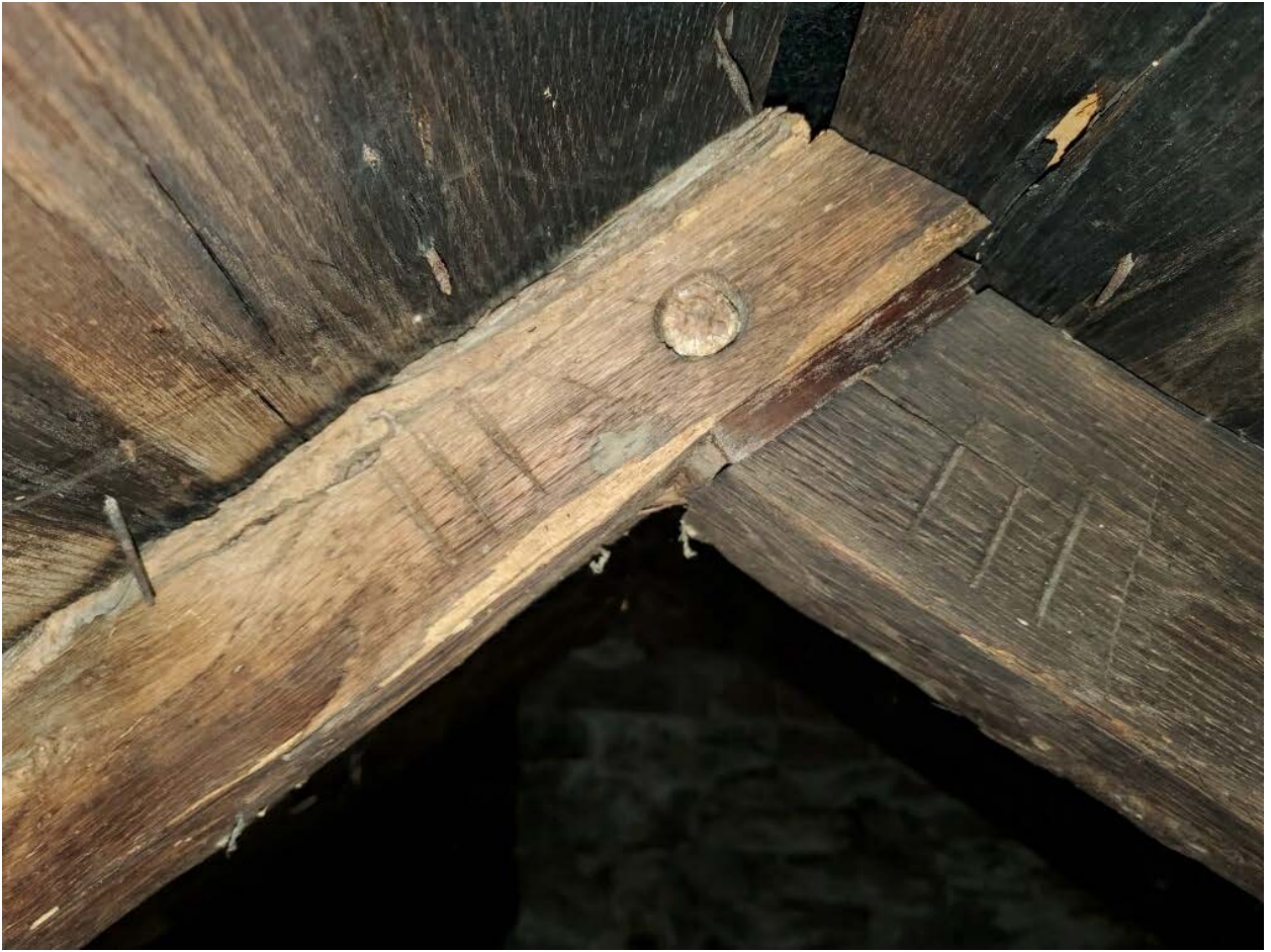
24 of 25. Attic, rafters, looking northwest.
