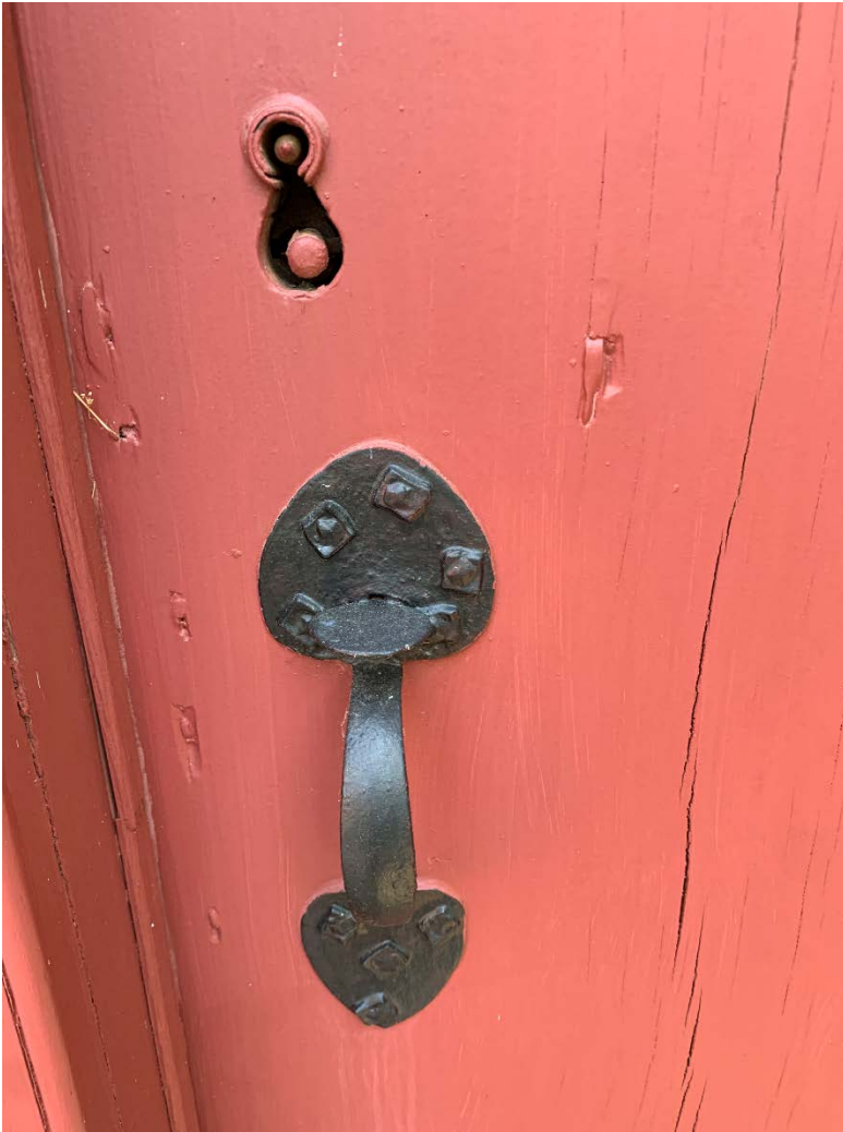
8 of 25. Latch and keyhole on rear (southwest) elevation of house.
