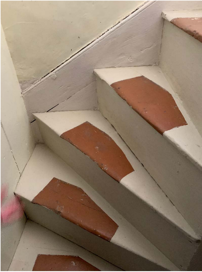
10 of 25. Front entry stair, looking southwest.
