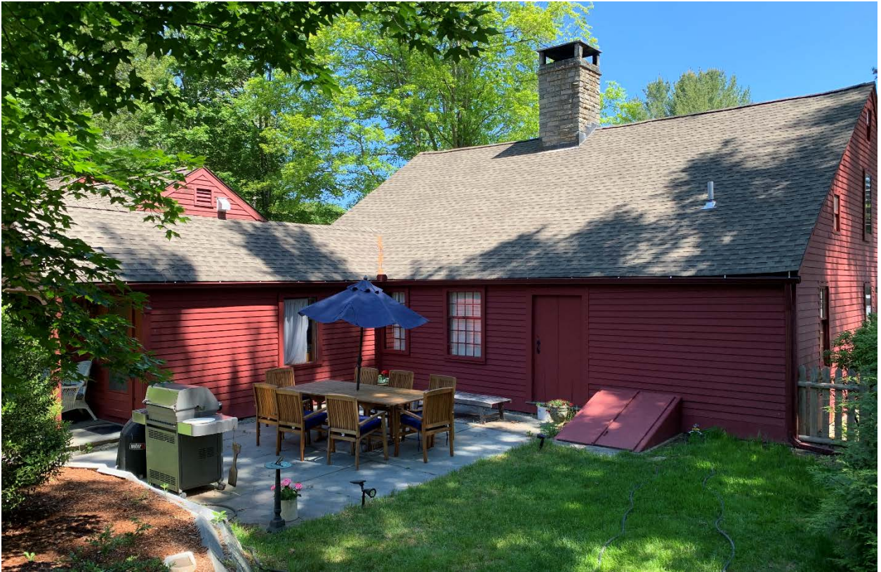
3 of 25. Rear elevation and ell, looking north.
