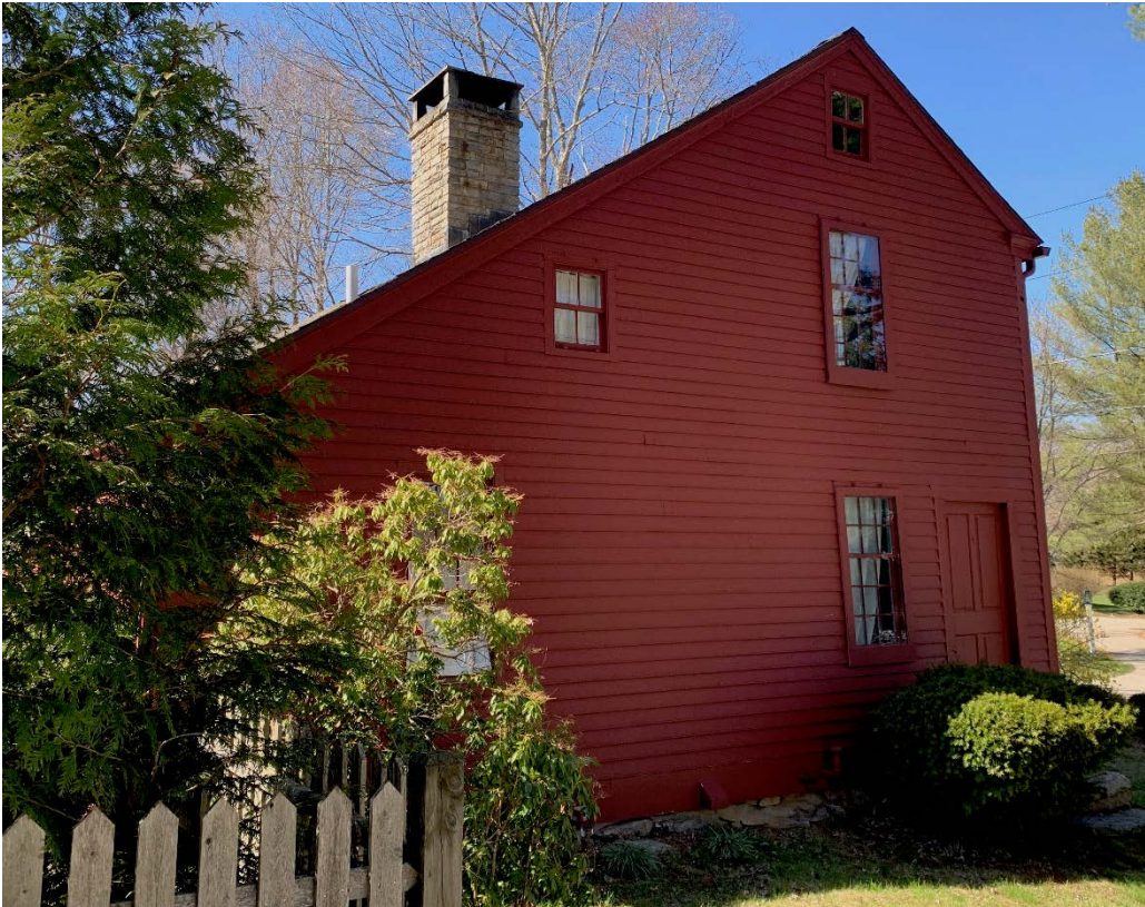
2 of 25. Southeast gable end, looking northeast.
