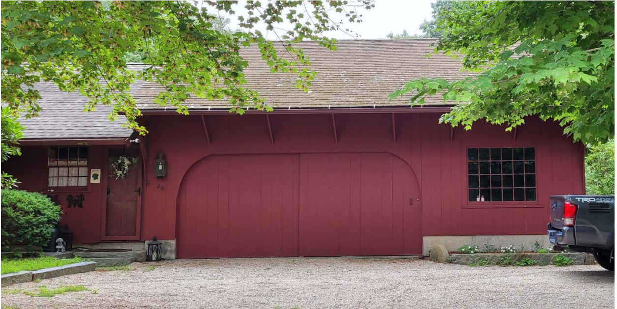
4 of 25. Attached garage/carriage house, northeast elevation, looking southwest.
