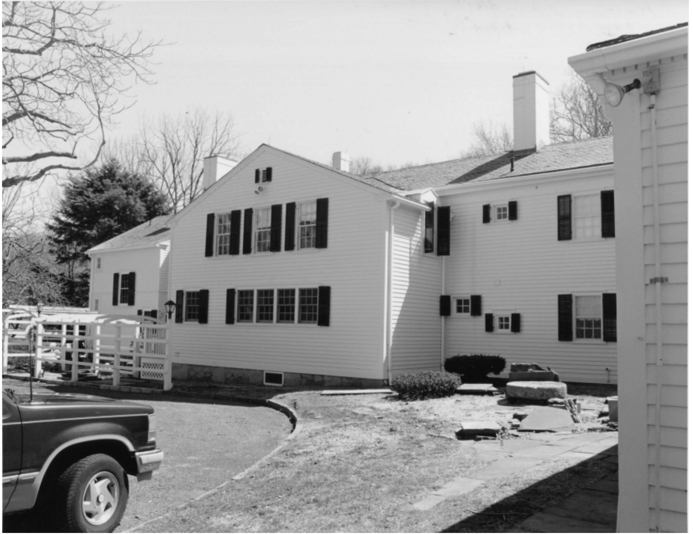
National Register photo of 80 Shore Road, rear wing, camera facing southeast.
