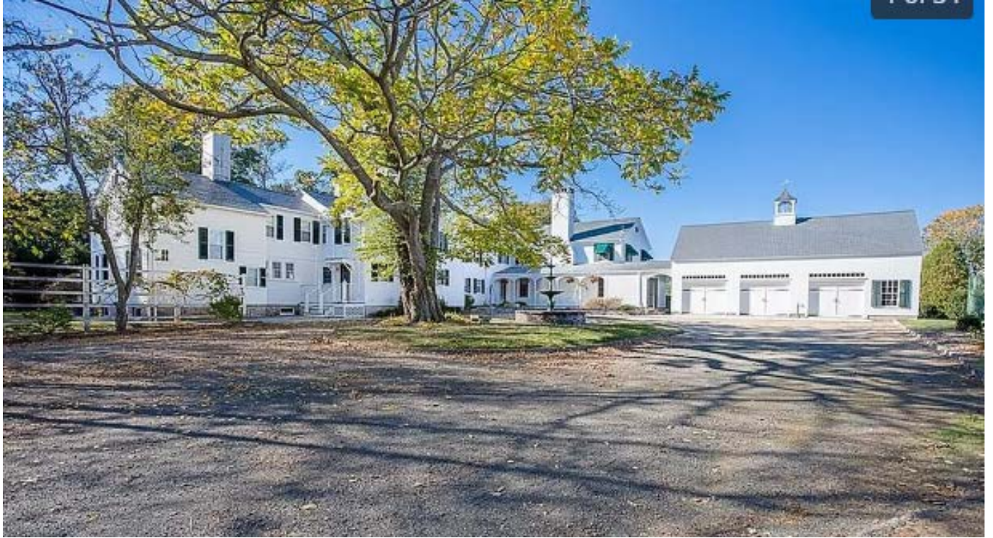
Photo of 80 Shore Road, Waterford, Preservation Connecticut Track Demolitions, October 11, 2023.
