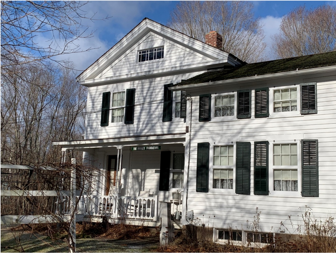
7 of 17. South Elevation, Nathan C. Dudley House, side porch (looking northwest).
