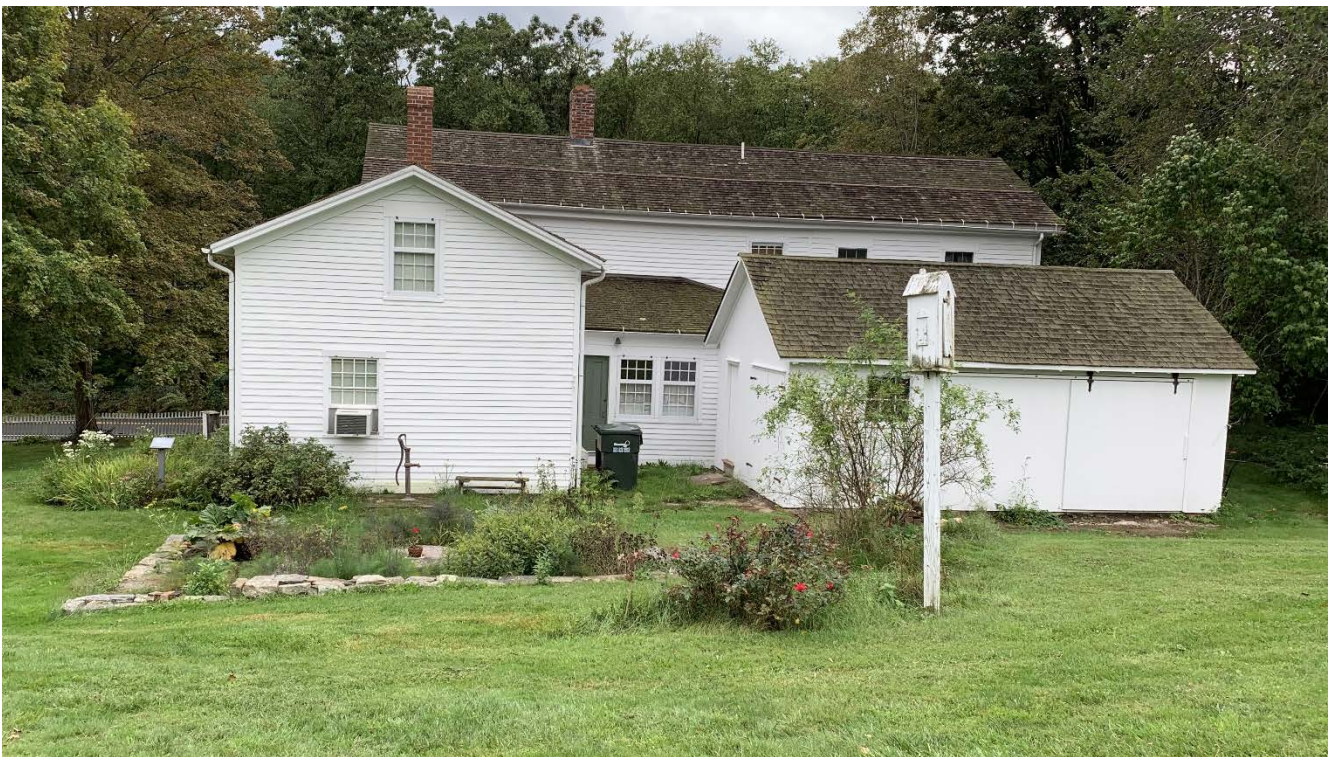
2 of 17. East Elevation, Nathan C. Dudley House and Woodshed, right (looking west).
