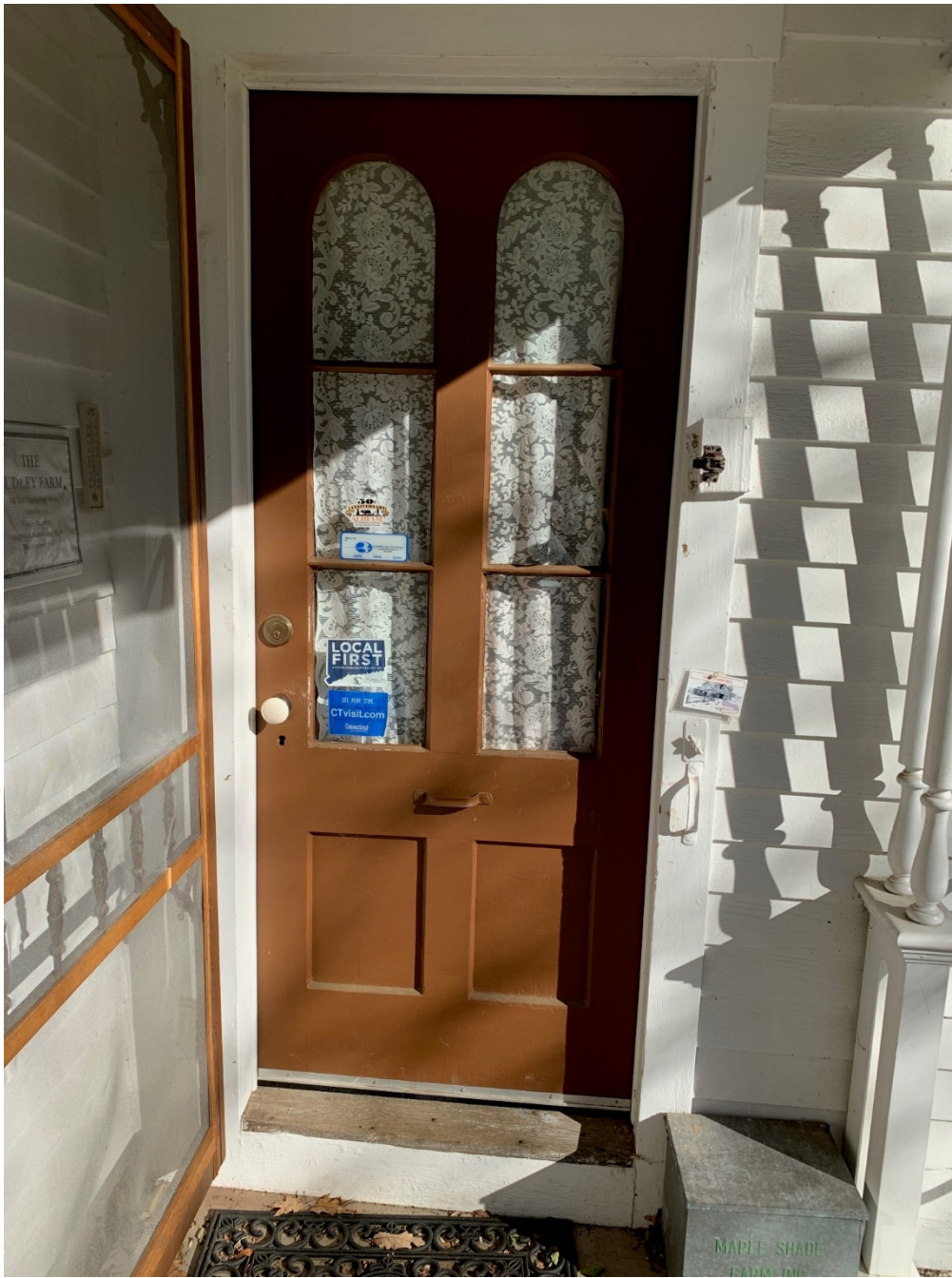
8 of 17. West Elevation, Nathan C. Dudley House, Southeast Wing, Side Door (looking east).
