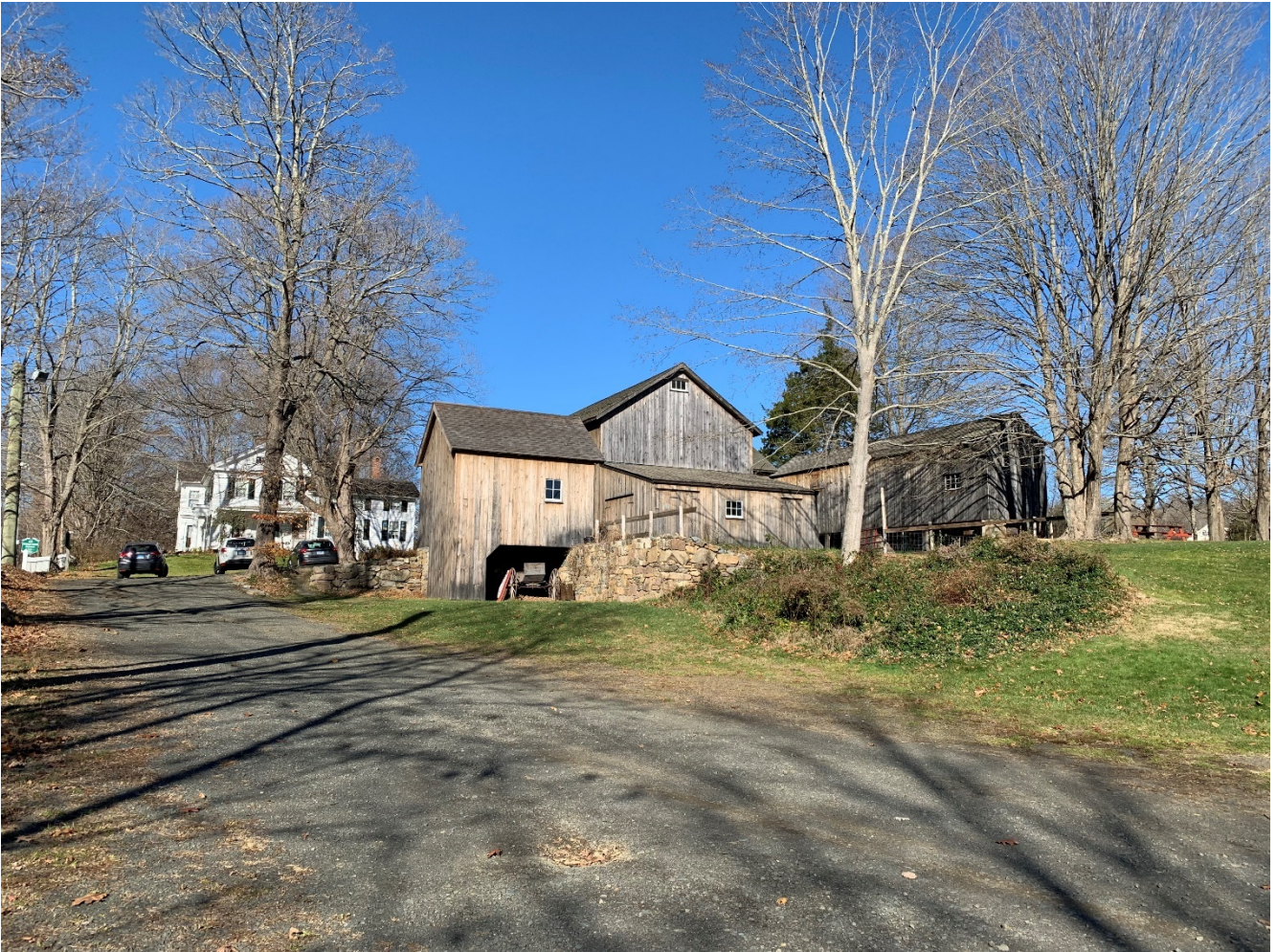
4 of 17. South View, Milk House and Main Barn Complex (looking north).
