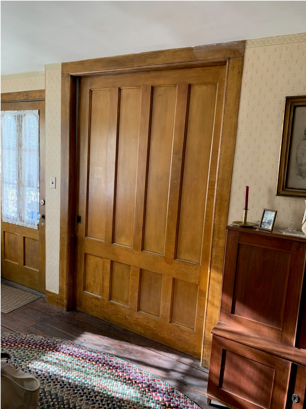
10 of 17. Nathan C. Dudley House, Dining Room, Pocket Door (looking west).
