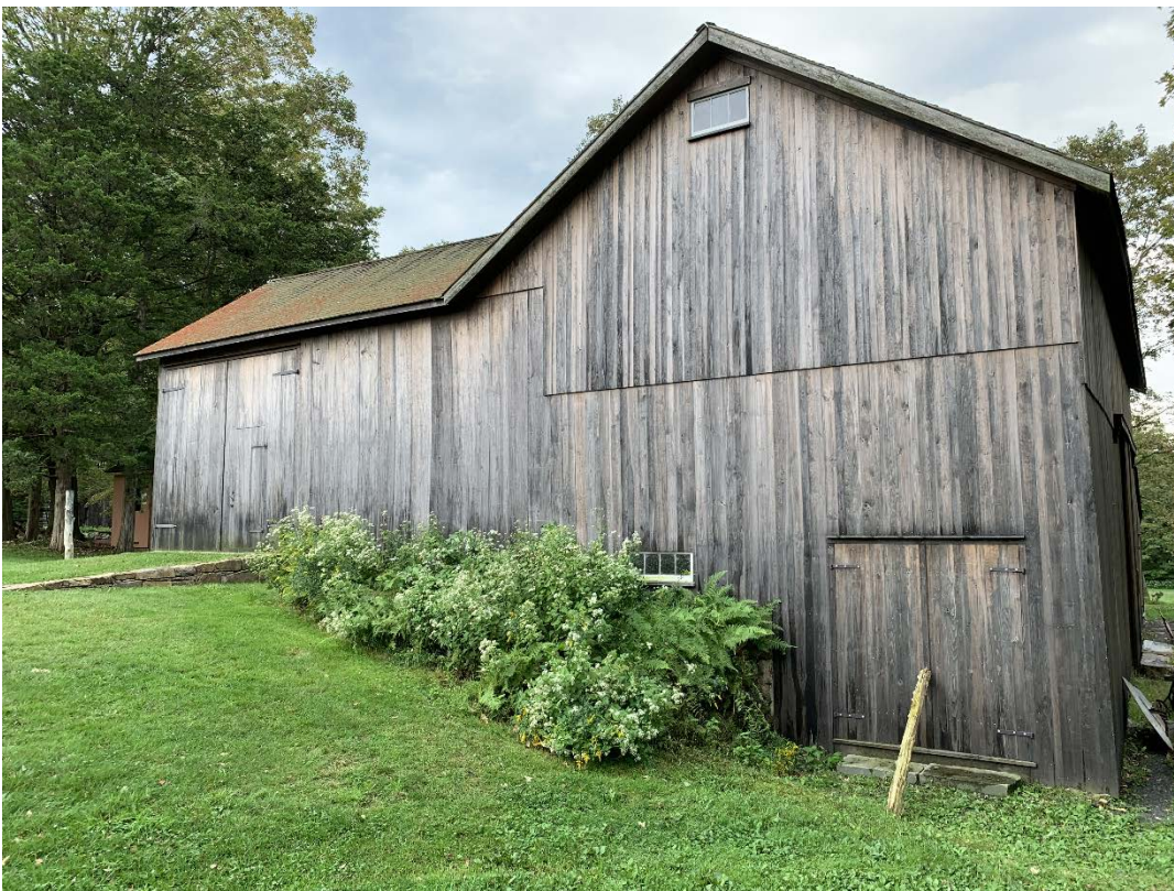
14 of 17. Main Barn Complex, North Elevation, West Barn (looking south).
