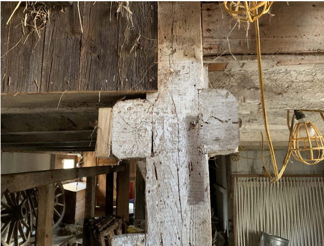
15 of 17. West Barn, Front Section, Square Rule Joint (looking south).
