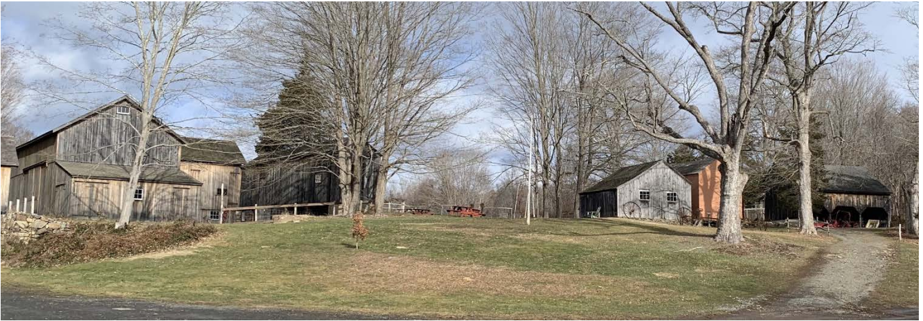
3 of 17. Southwest View, Main Barn Complex, Garage, Ice House/Restroom, Storage Shed (looking northeast).
