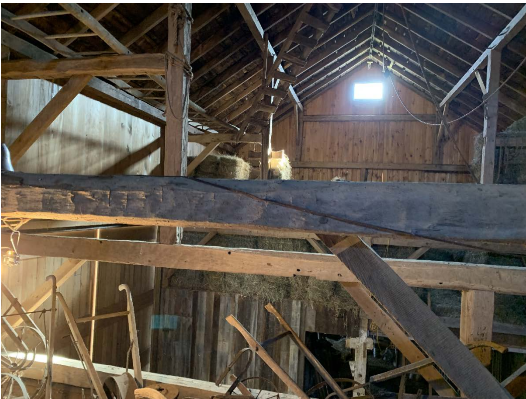
16 of 17. West Barn, Front Section, Loft (looking south).
