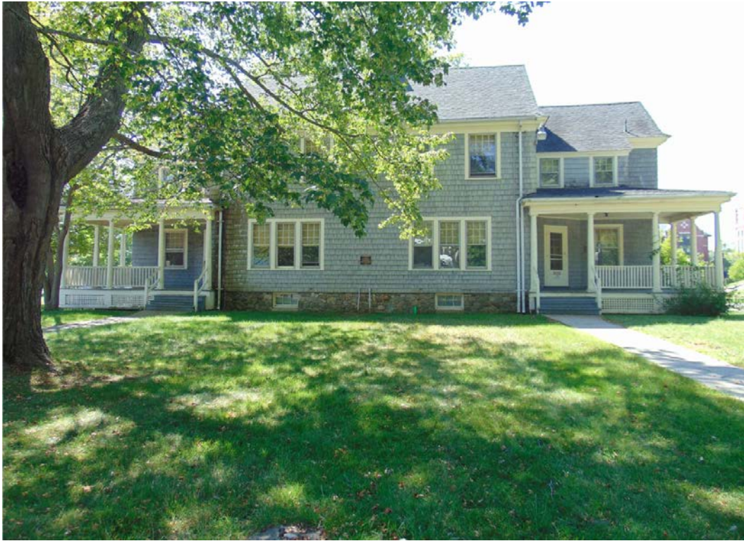
Front of 4 Gilbert Road (View Looking South at Façade/North Elevation)
