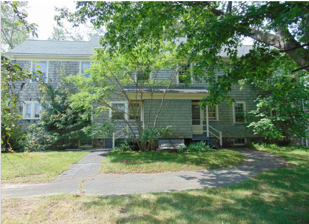
Rear of 4 Gilbert Road (View Looking North at South Elevation)
