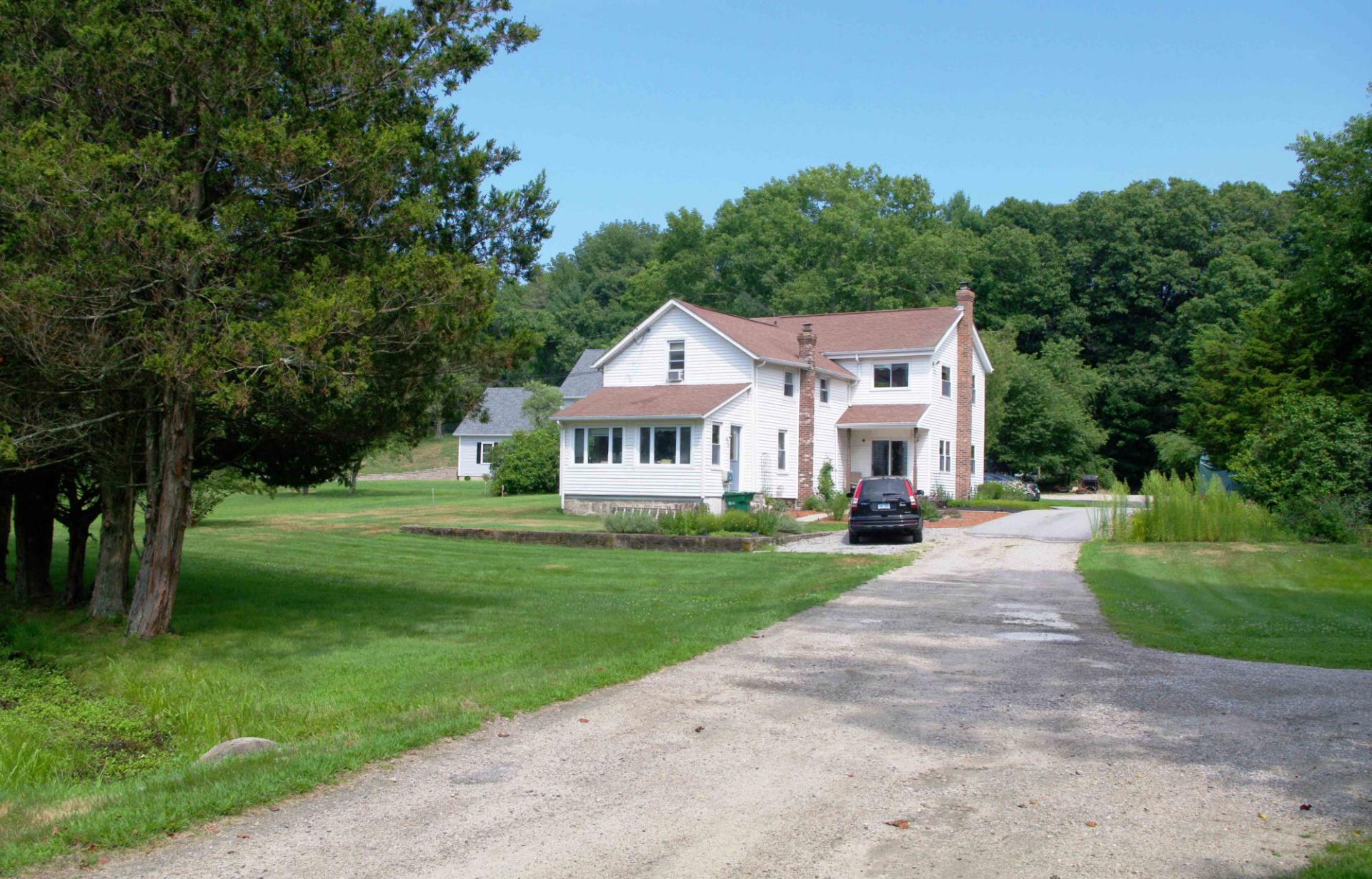
Thomas Ames House at 25 Oil Mill Road, camera facing east. Oil Mill Historic District New London County, Connecticut
