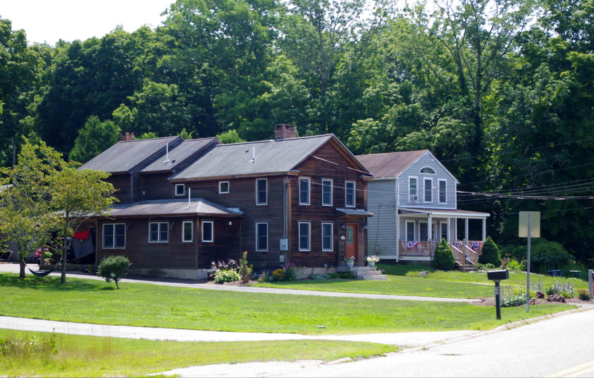
Winthrop Beebe House at 15 Oil Mill Road and George Brown House at 13 Oil Mill Road, camera facing southeast. Oil Mill Historic District New London County, Connecticut
