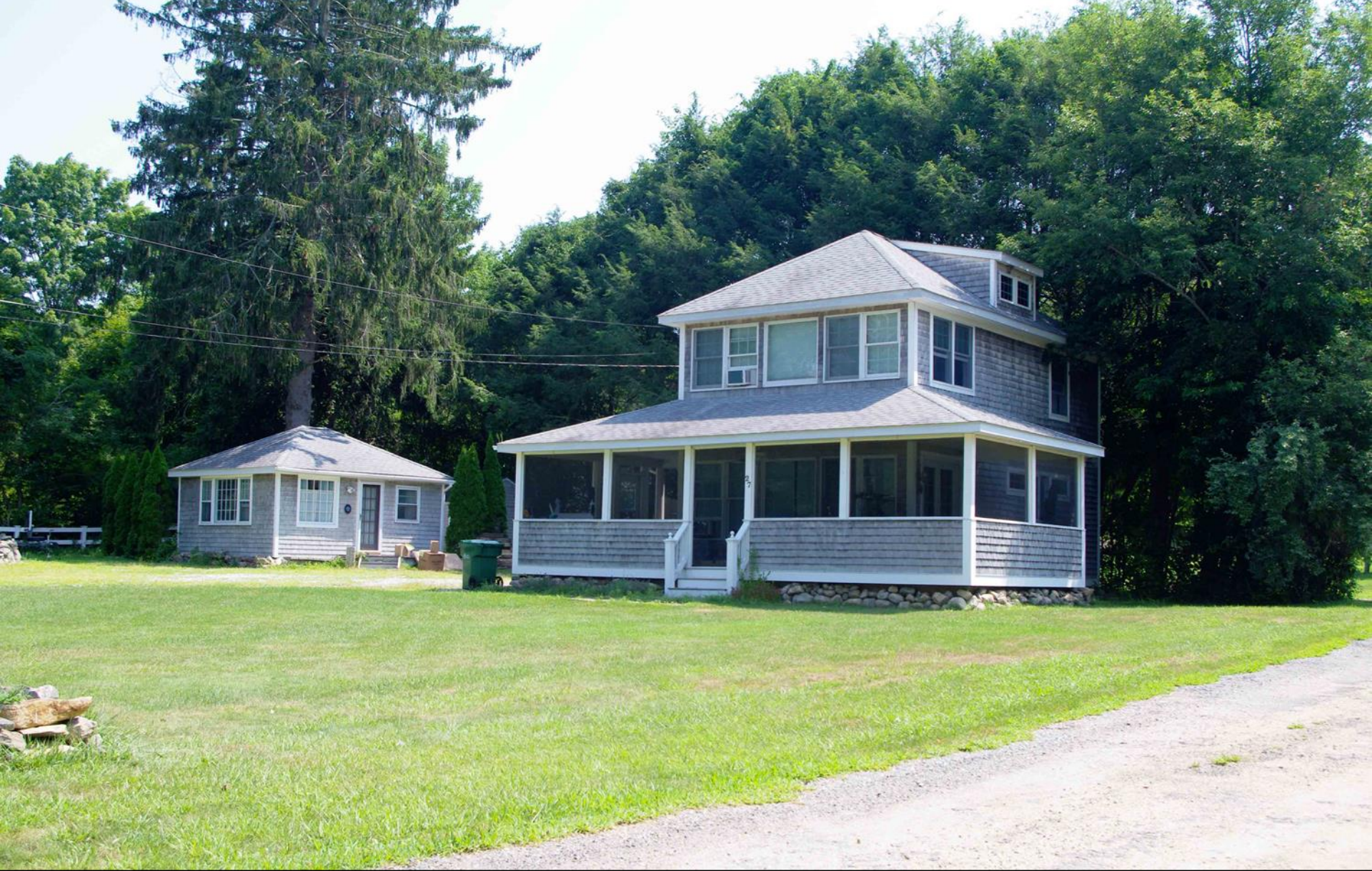
House and cottage at 27 Oil Mill Road, camera facing northeast. Oil Mill Historic District New London County, Connecticut
