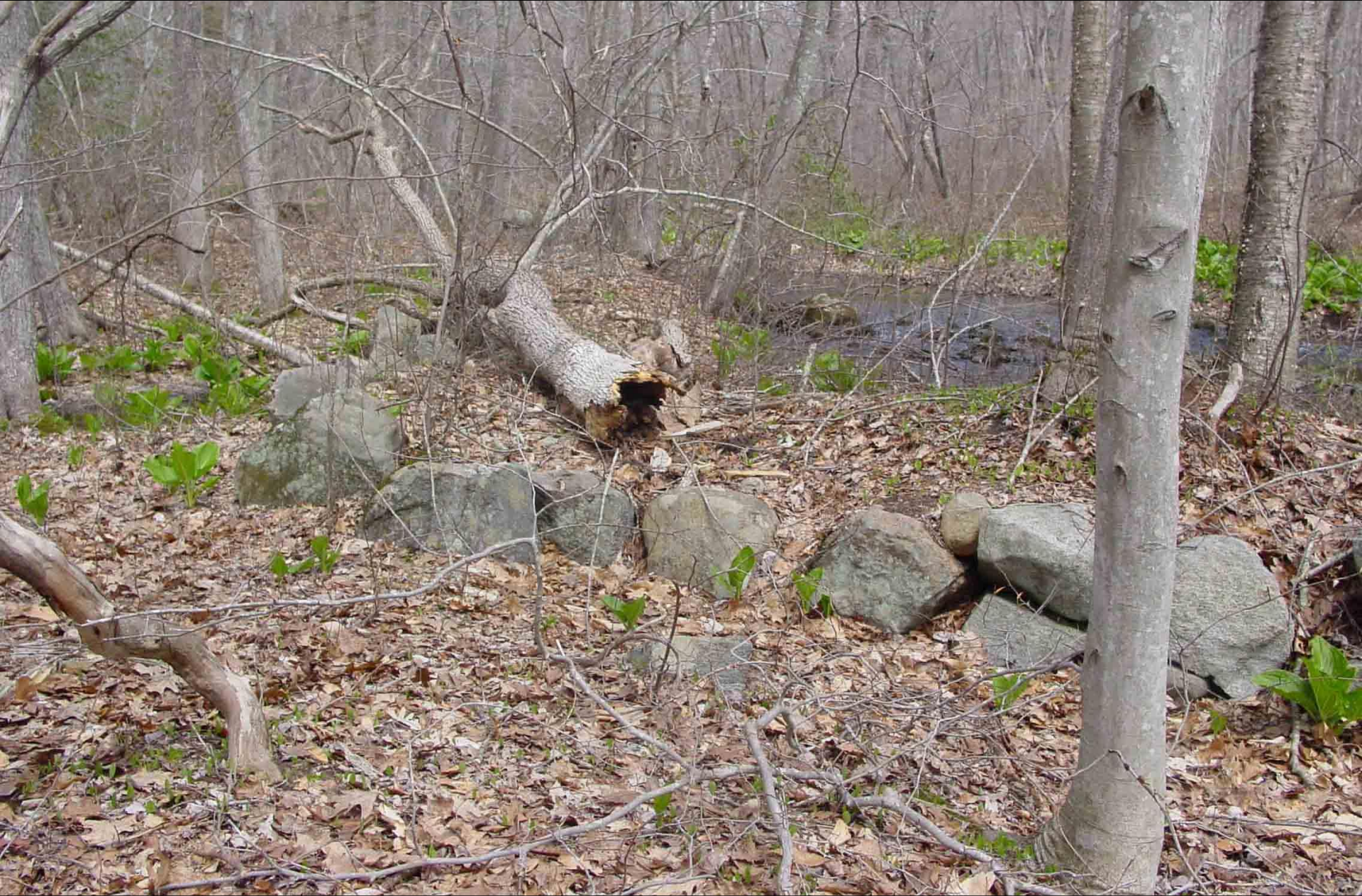
Southwest corner of dam at 54 Oil Mill Road, camera facing north (April 2015). Oil Mill Historic District New London County, Connecticut
