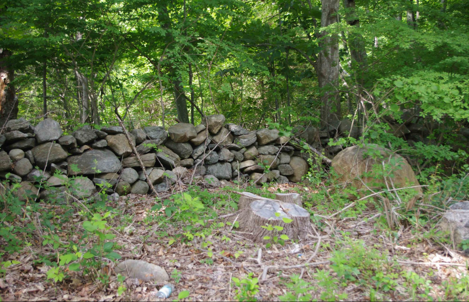
Stone wall at 21 Gurley Road, camera facing northeast. Oil Mill Historic District New London County, Connecticut
