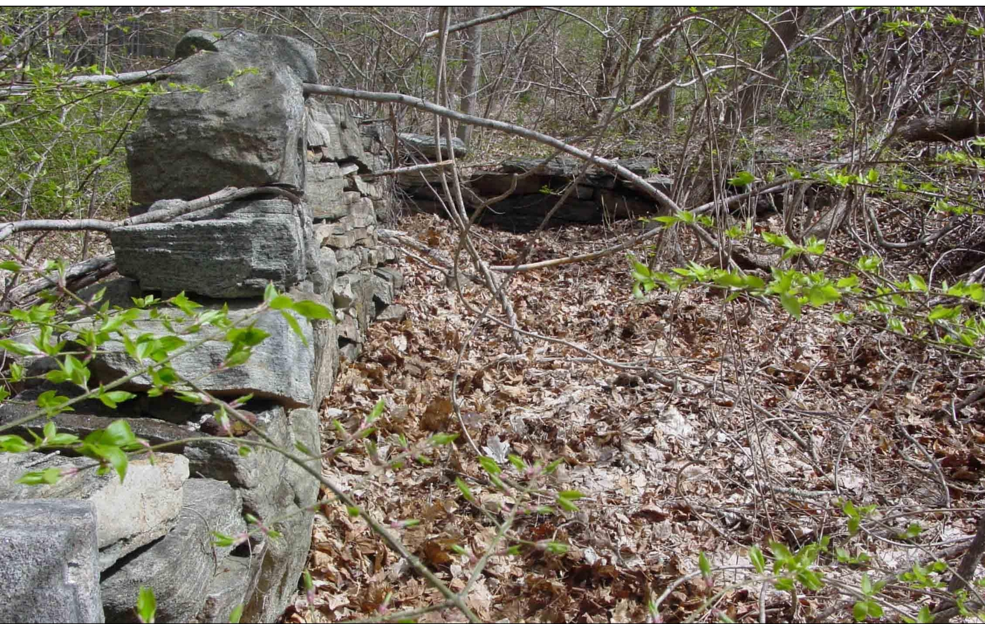
Foundation at 59 Gurley Road, camera facing north (April 2015). Oil Mill Historic District New London County, Connecticut
