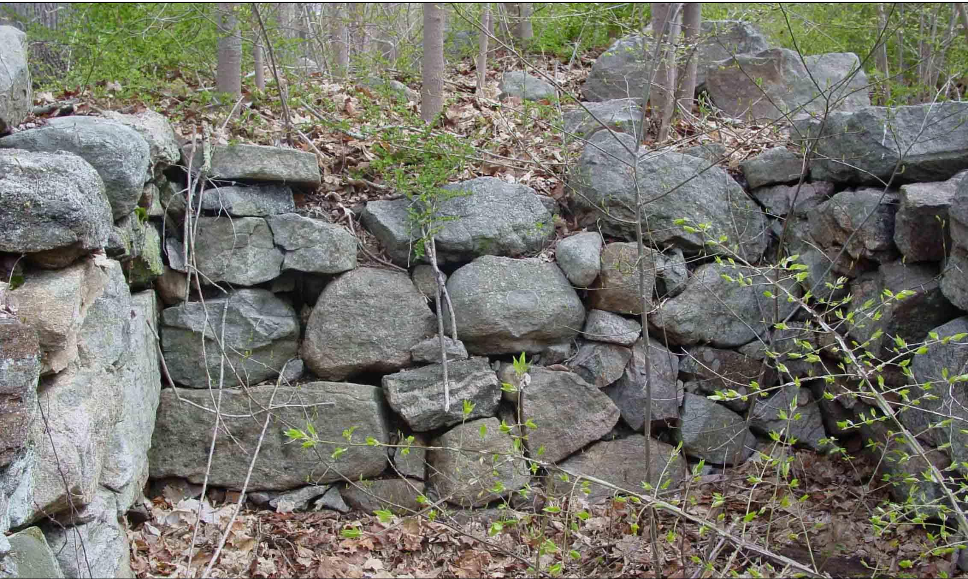
Wheel pit at 59 Gurley Road, camera facing north (April 2015). Oil Mill Historic District New London County, Connecticut
