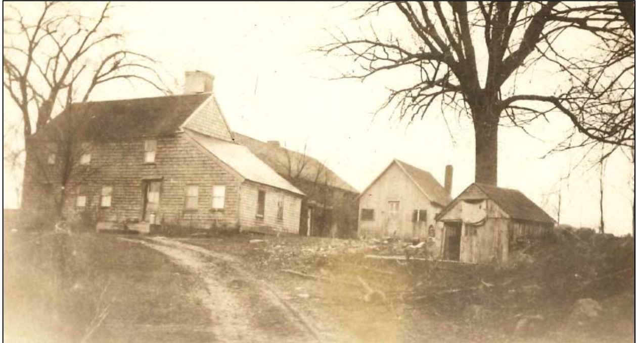
Figure 6. Former almshouse (built as the Abel Moore house), December 15, 1935, camera facing northwest (photographer Margaret Stacy, from Waterford Historical Society).
