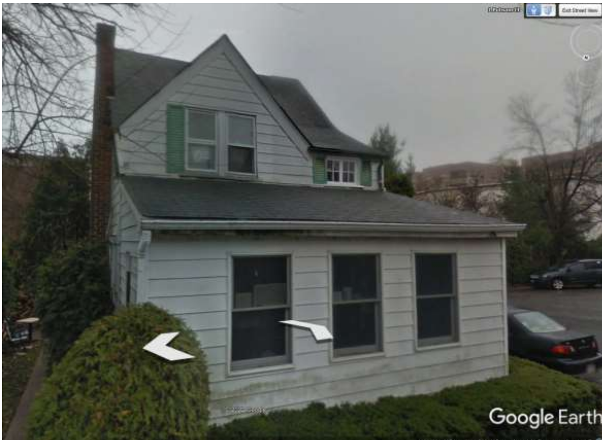
2 Putnam Court, facing southwest, (google earth, 12/2015).
