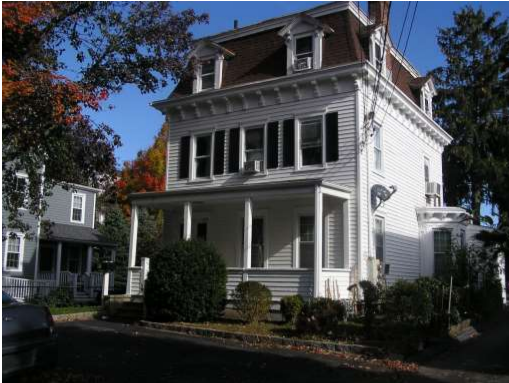
Façade (west elevation) of 47 Church Street, camera facing northeast (November 2021).
