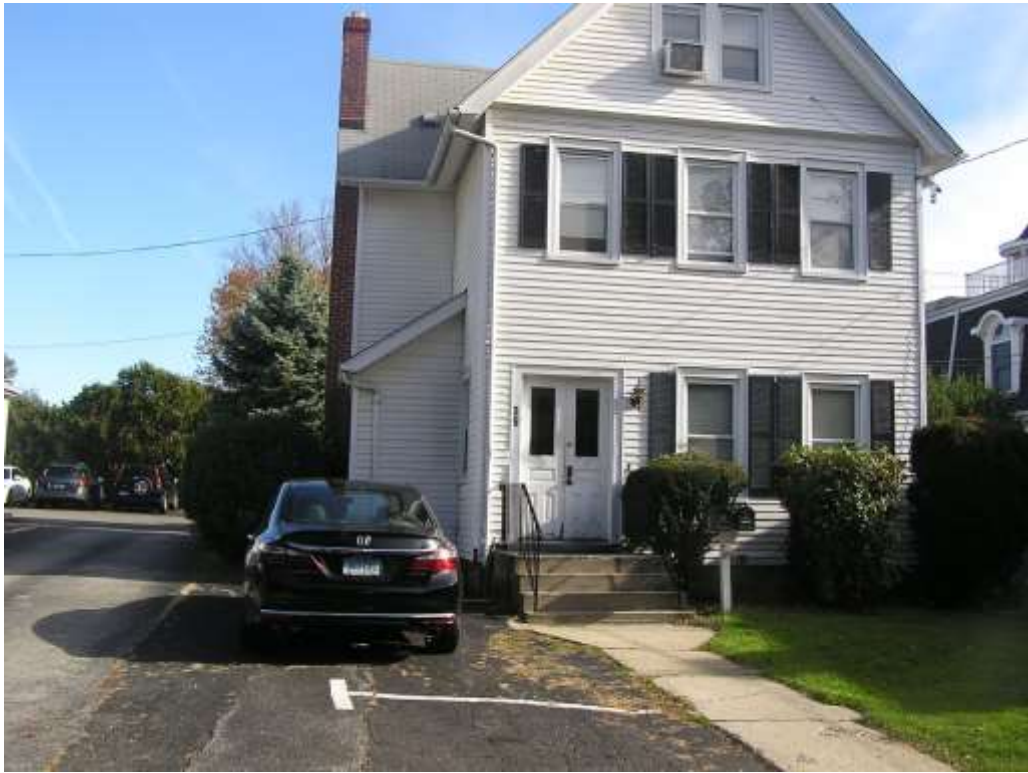
Façade (west elevation) of 39 Church Street, camera facing east (November 2021).
