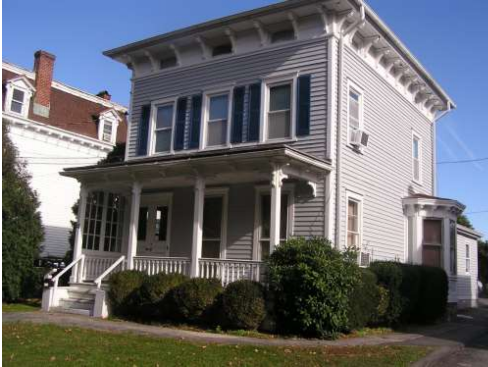
Façade (west elevation) of 43 Church Street, camera facing northeast (November 2021).
