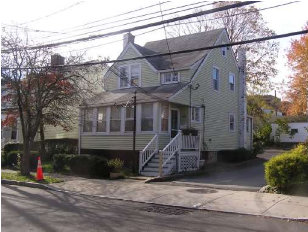
Façade (east elevation) of 32 Sherwood Place, camera facing southwest (November 2021).
