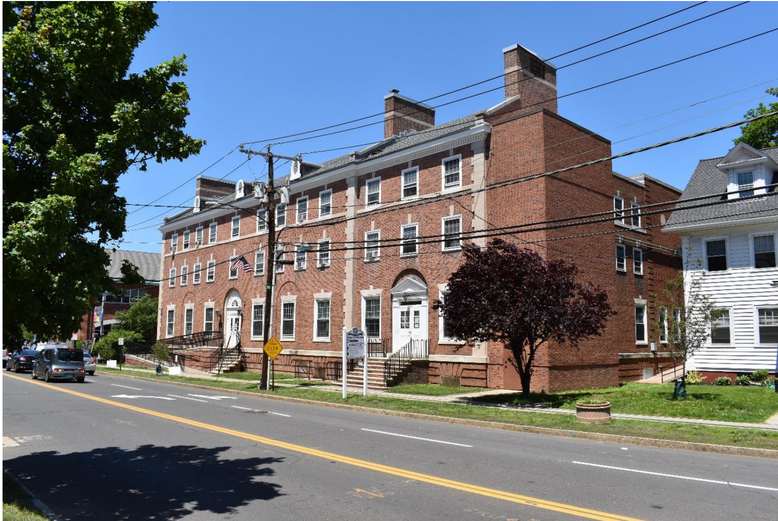
Photograph 1 of 42. West elevation. Camera facing northeast.
