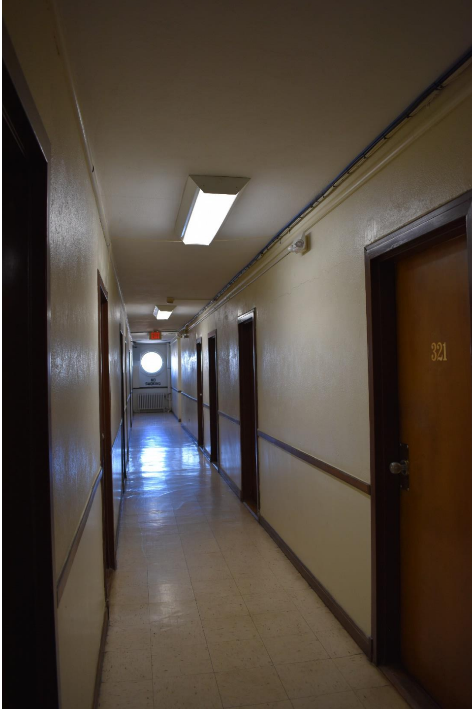
Photograph 36 of 42. Hallway of third floor dormitories. Camera facing north.
