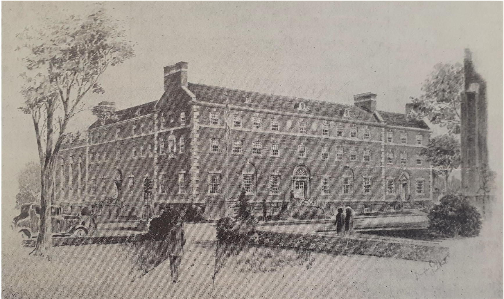
Figure 10. Drawing of the 99 Union Street building. Source: "Our Y" 2, no. 2 (October 18, 1928), archives of the YMCA of Northern Middlesex County.
