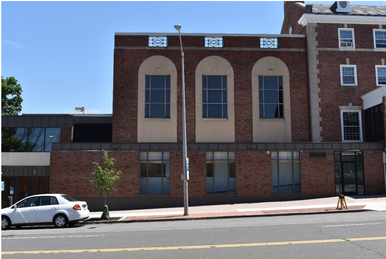
Photograph 5 of 42. Central portion of north elevation. Camera facing south.
