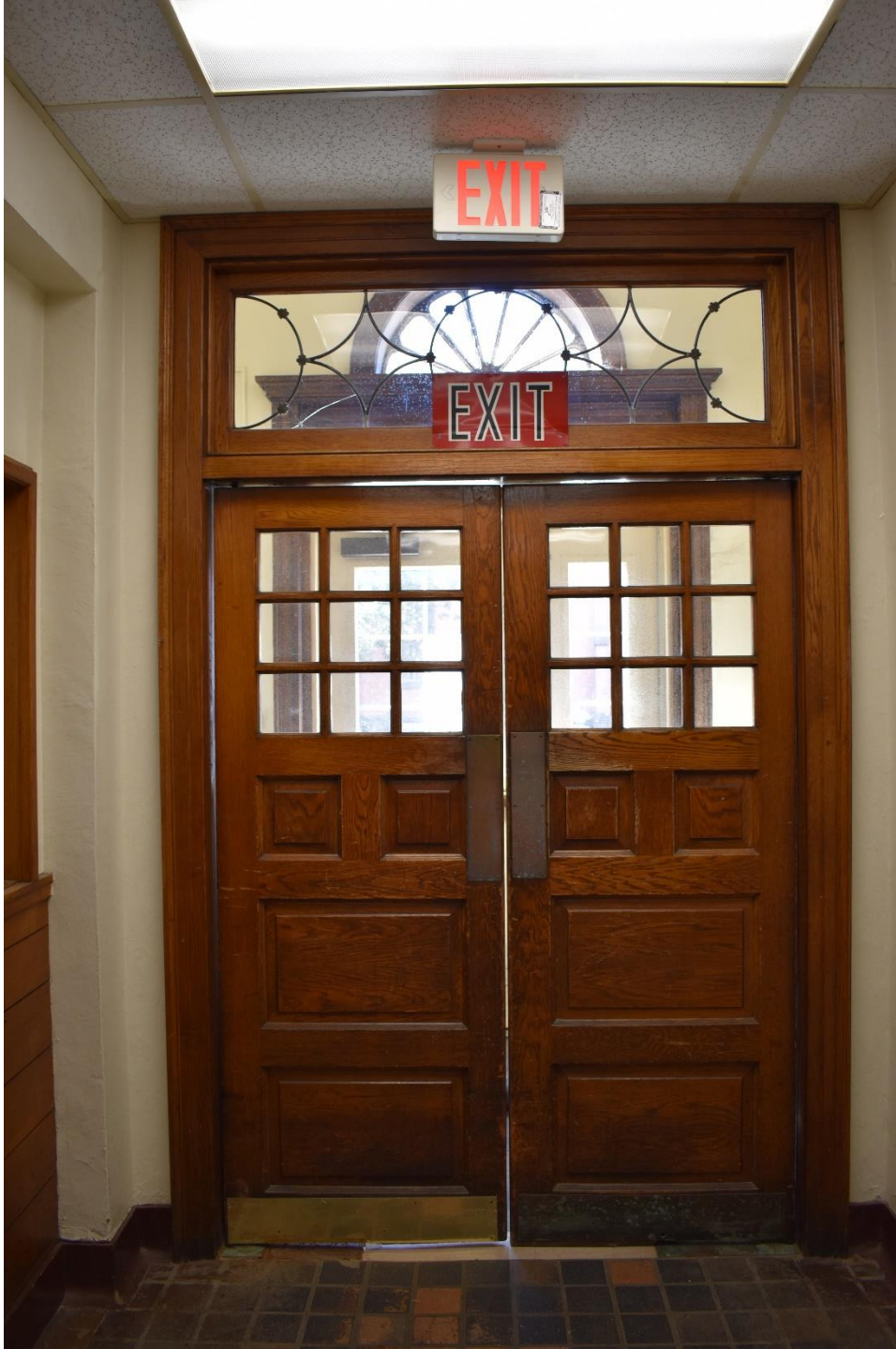
Photograph 14 of 42. Detail of the door and vestibule accessed via the entrance on the west elevation, originally the main entrance to the building.
