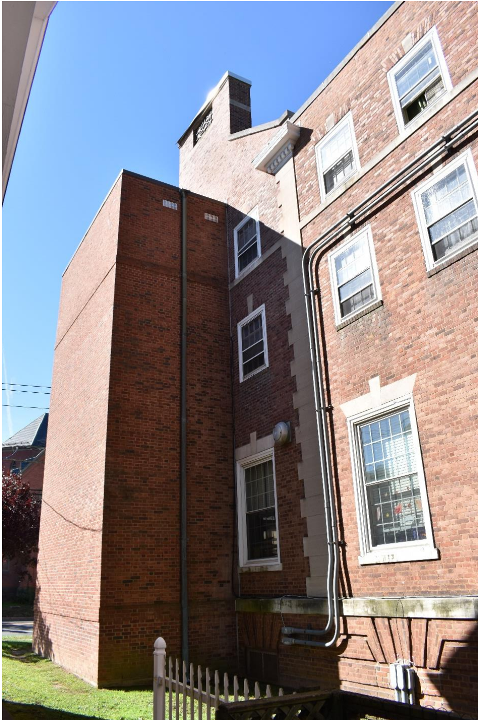
Photograph 9 of 42. South elevation. Camera facing northwest.
