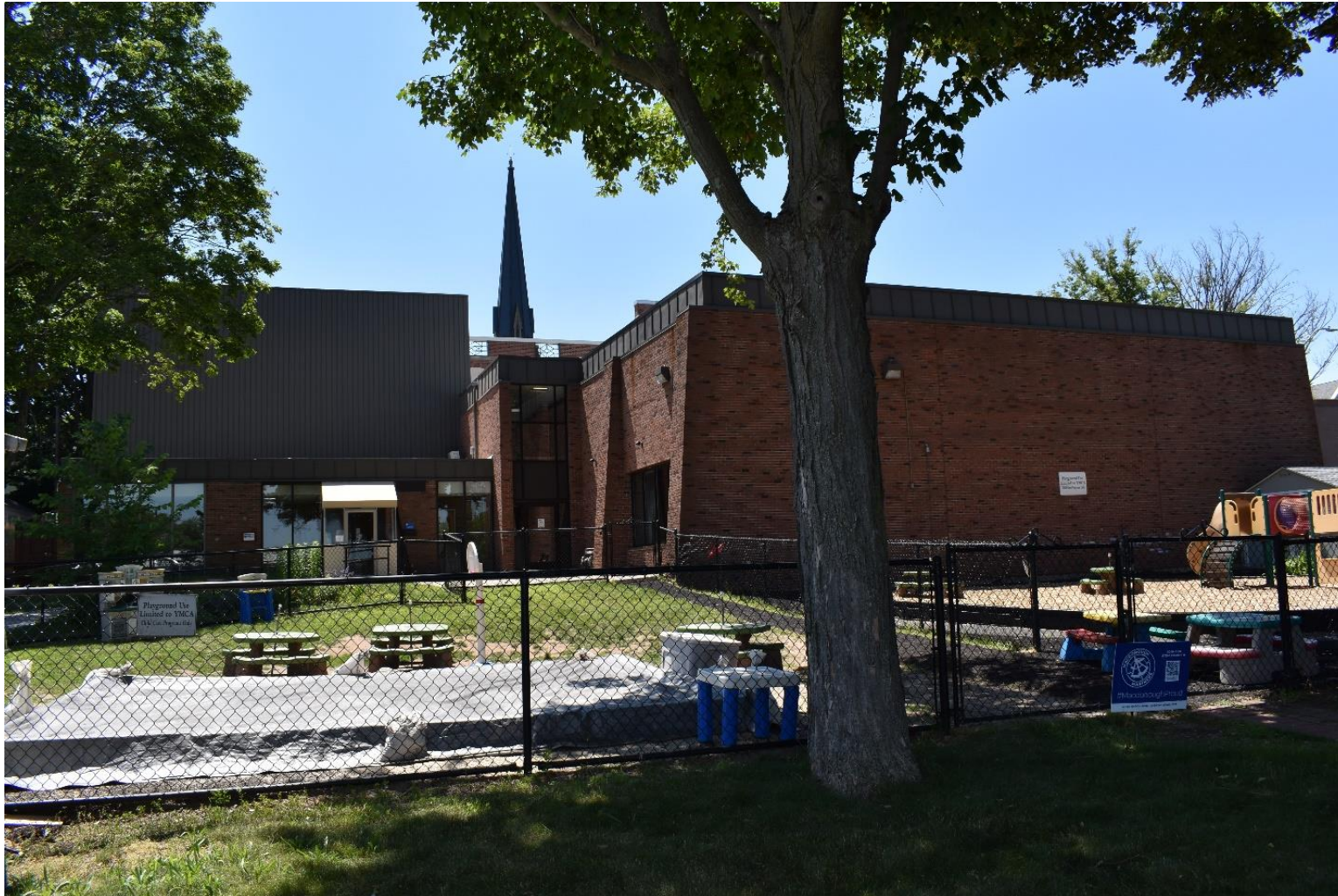
Photograph 10 of 42. East elevation. Camera facing west.
