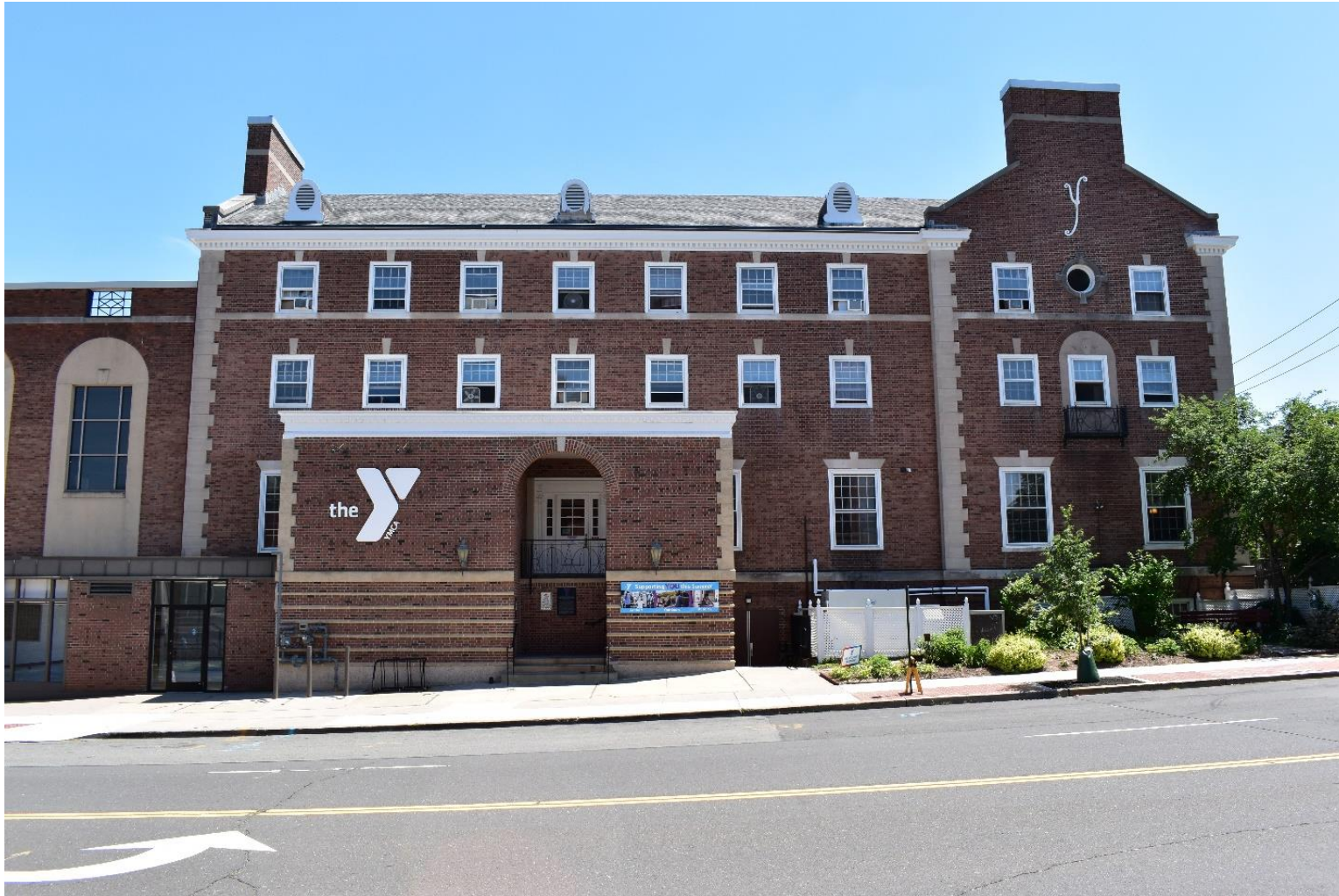
Photograph 4 of 42. Western portion of north elevation. Camera facing south.
