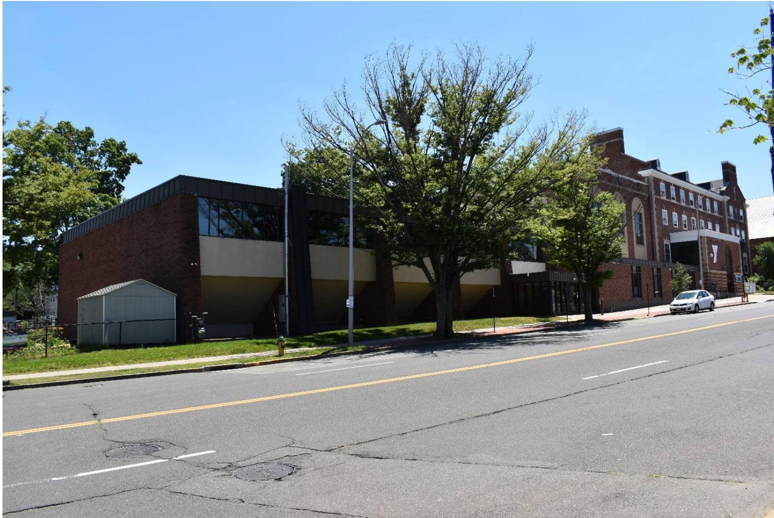
Photograph 7 of 42. North elevation. Camera facing southwest.
