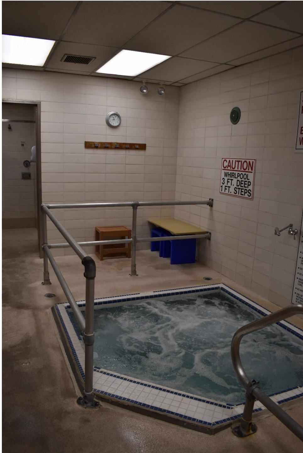
Photograph 29 of 42. Whirlpool room. Camera facing west.
