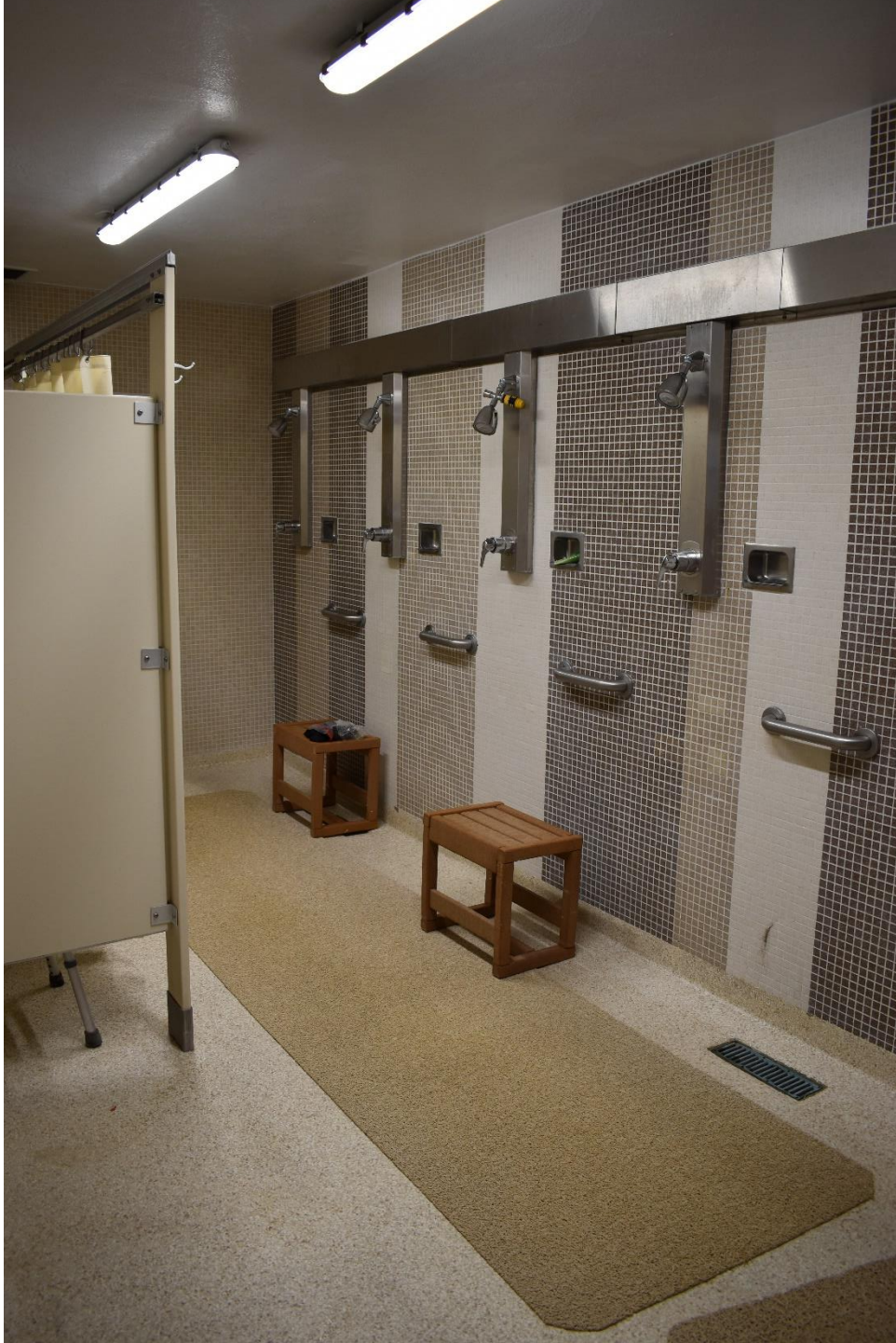
Photograph 27 of 42. Typical renovated shower room. Camera facing southwest.
