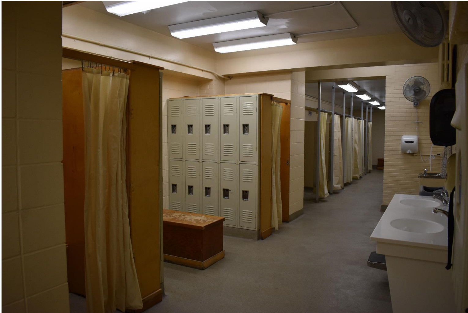
Photograph 24 of 42. Typical renovated locker room. Camera facing north.
