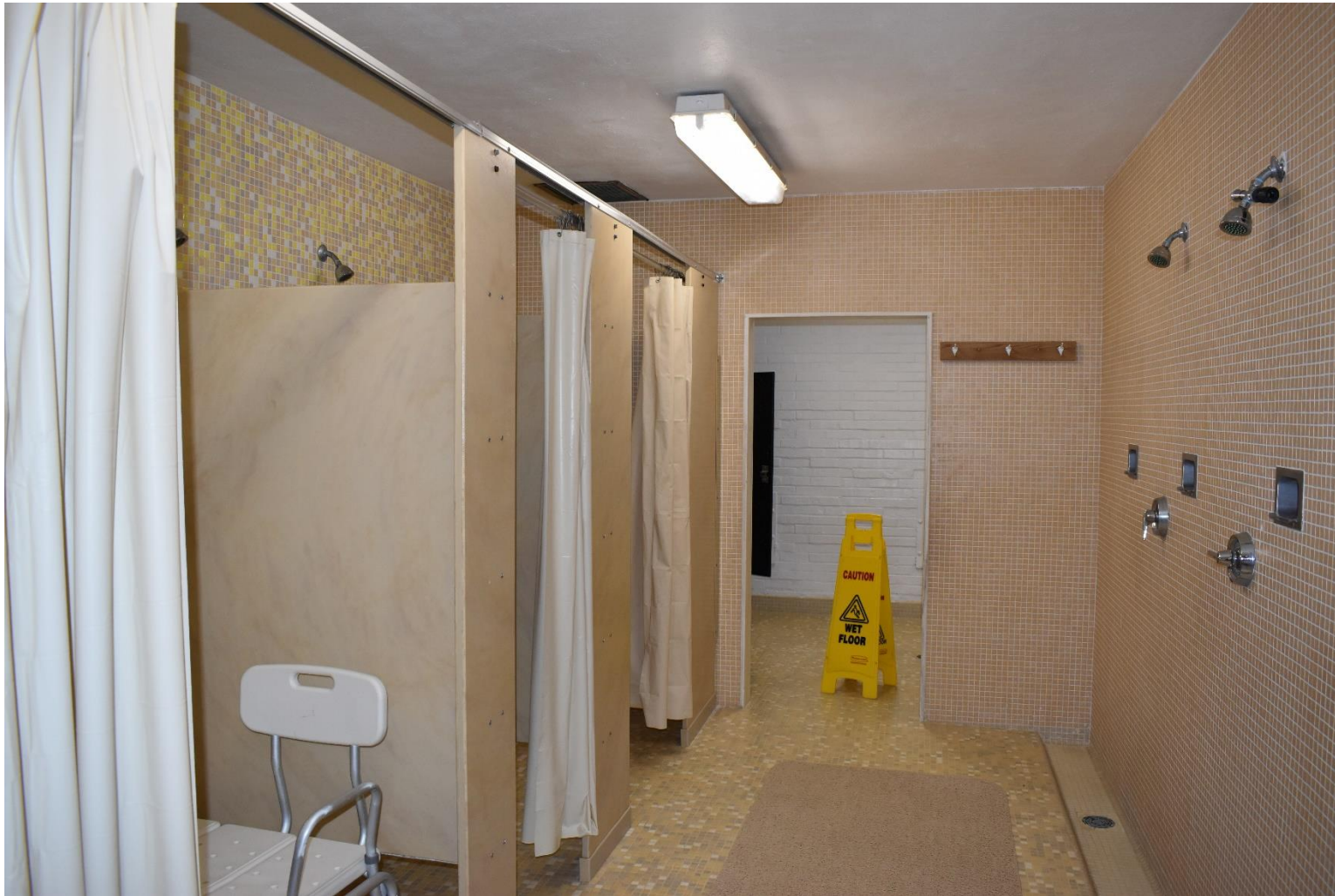
Photograph 26 of 42. Typical shower room with original materials. Camera facing southeast.
