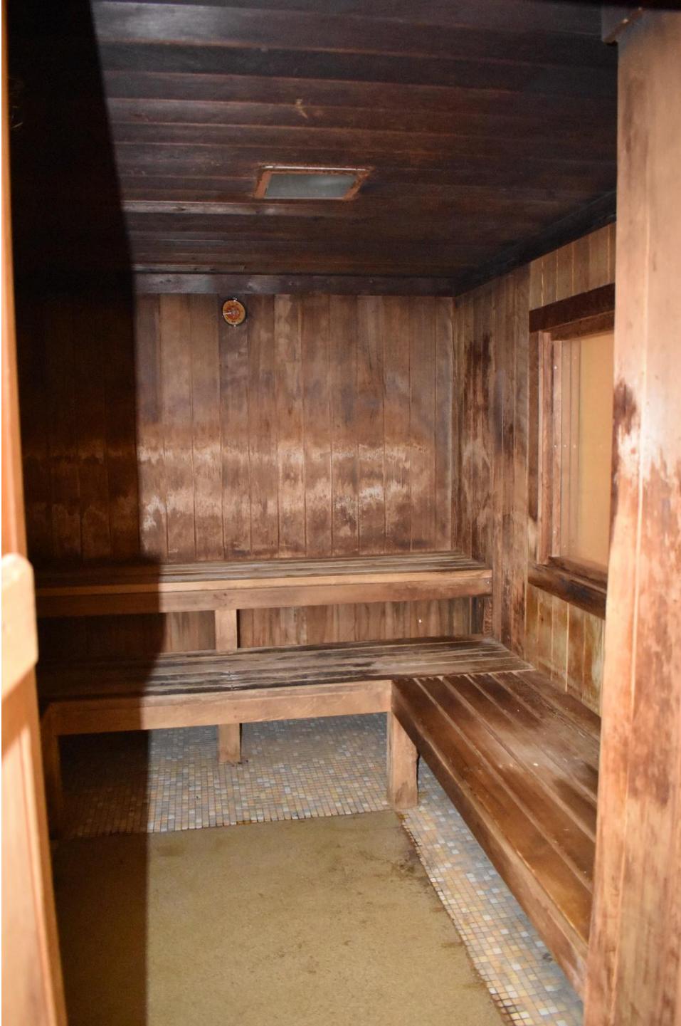
Photograph 30 of 42. Steam room interior. Camera facing south.
