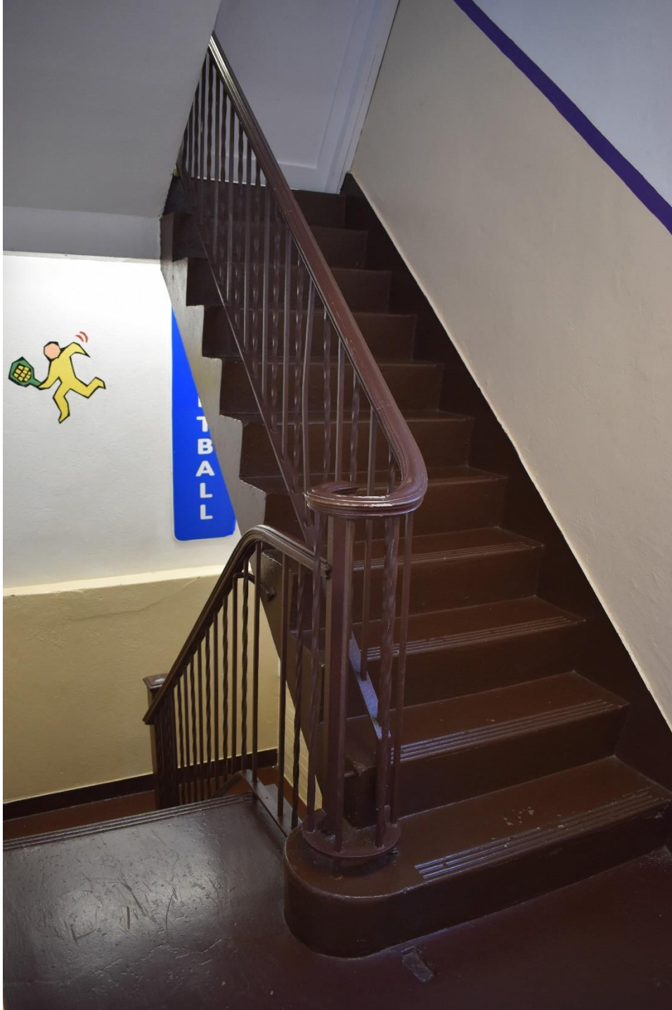
Photograph 40 of 42. Detail of stairwell in the center of the 1928 section of the building. Camera facing northwest.
