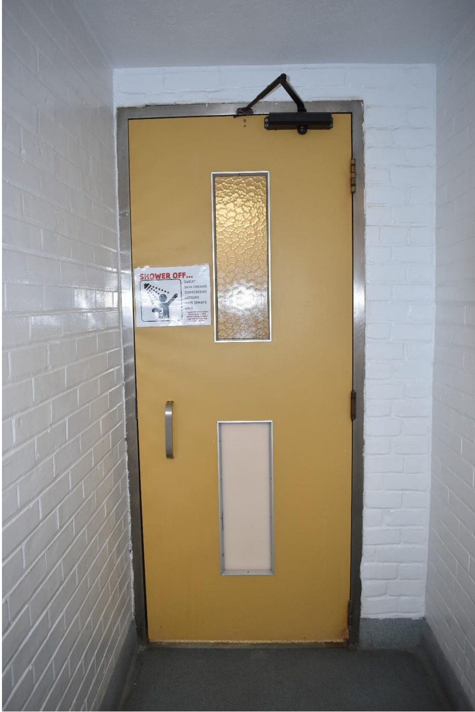
Photograph 28 of 42. Typical locker room door. Camera facing east.
