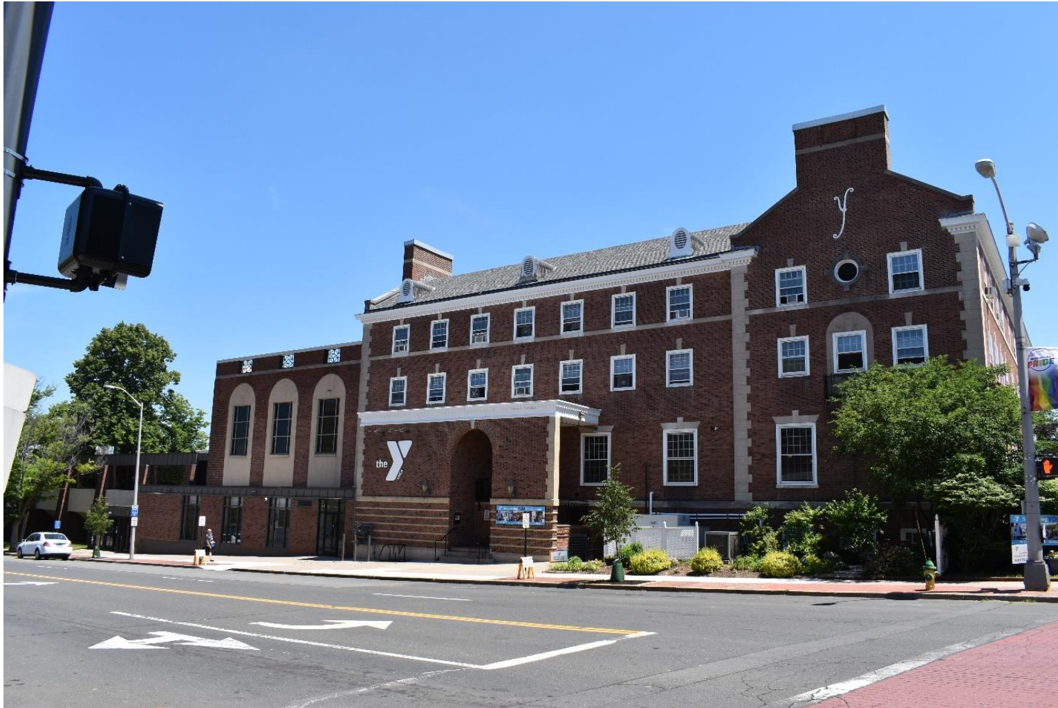
Photograph 3 of 42. North elevation. Camera facing southeast.
