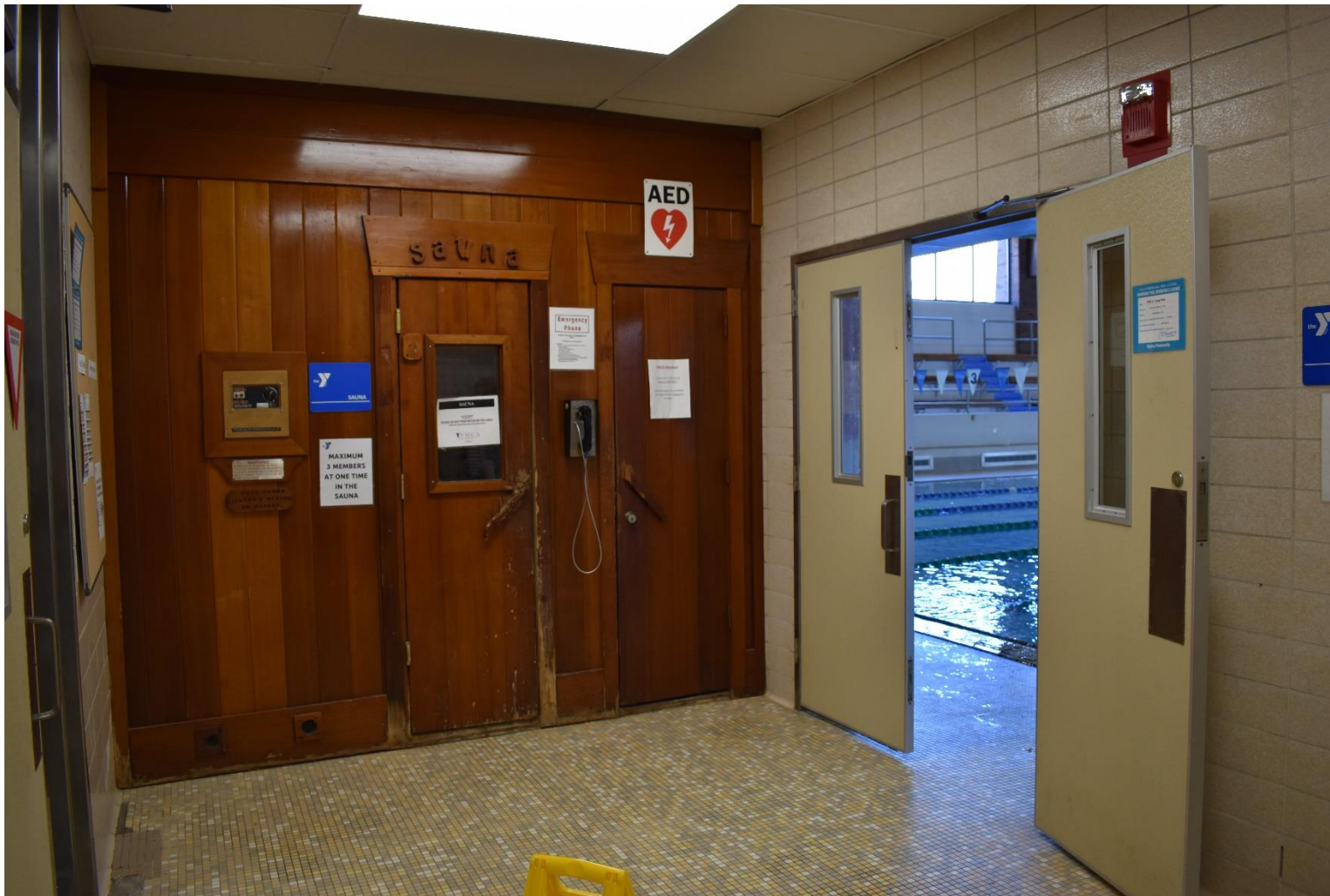
Photograph 31 of 42. Sauna entrance. Camera facing north.
