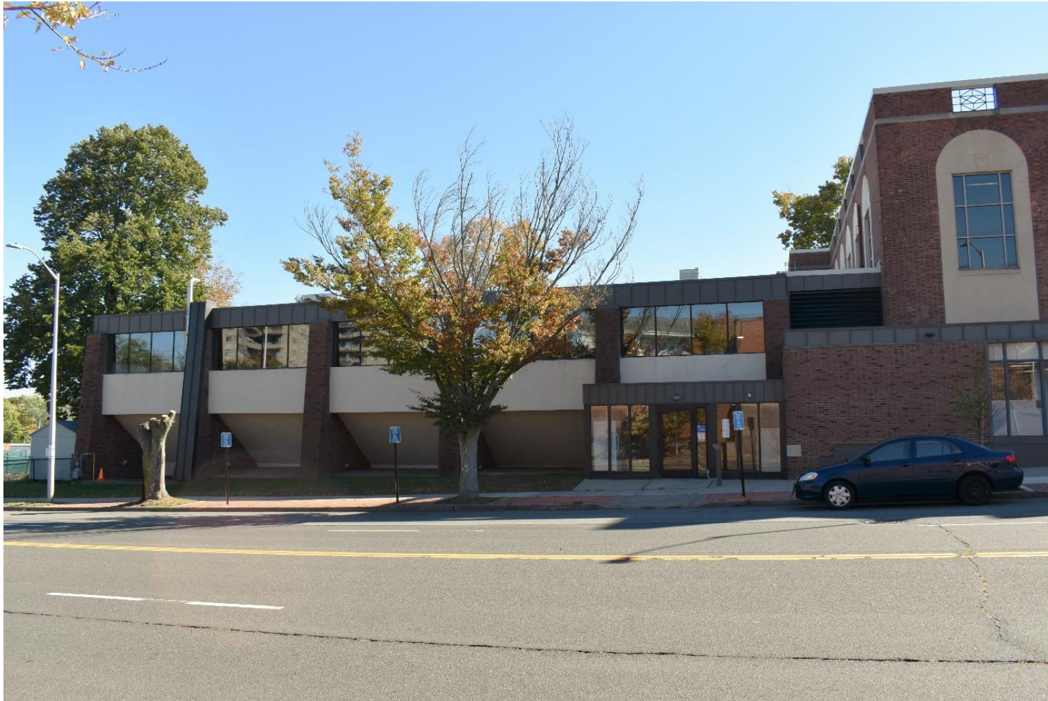
Photograph 6 of 42. Eastern portion of north elevation. Camera facing south.
