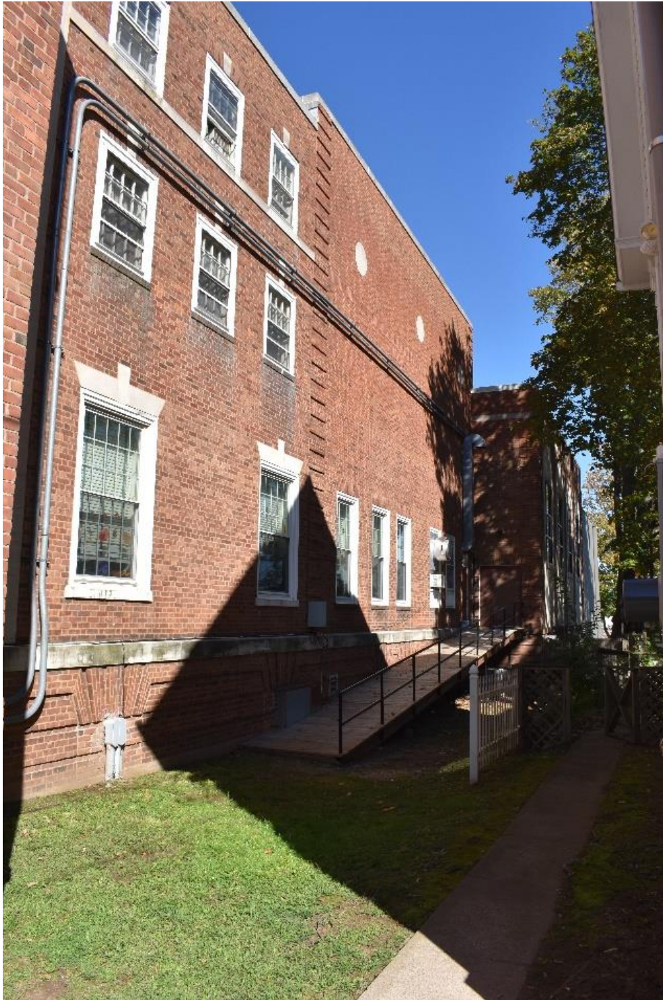
Photograph 8 of 42. South elevation. Camera facing northeast.
