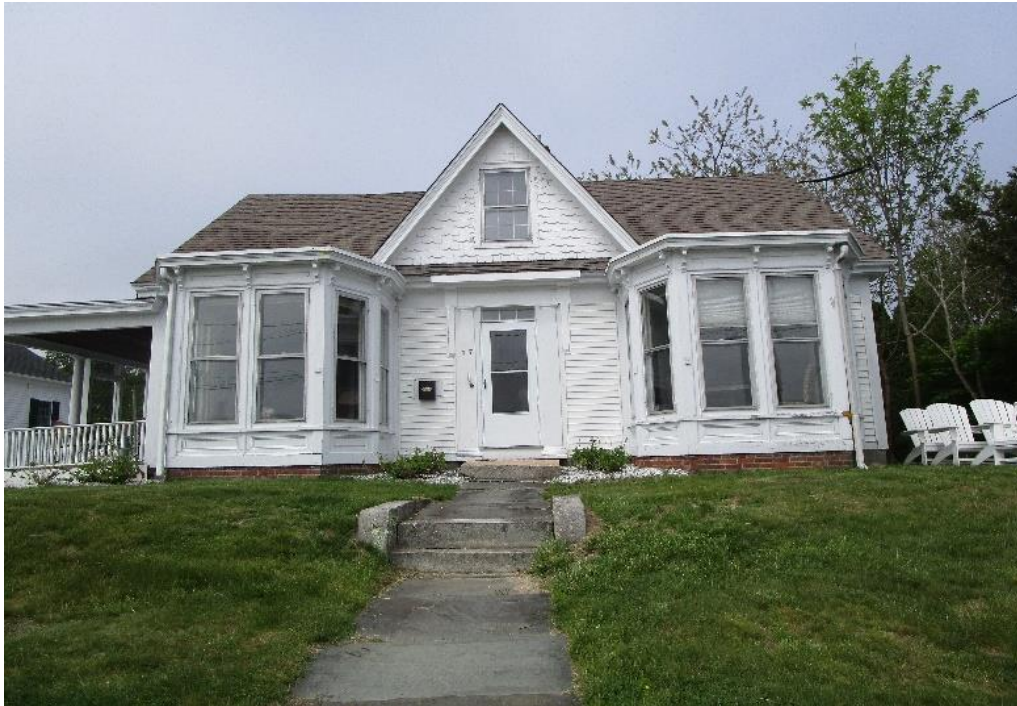
17 Gravel Street, Mystic (Groton), camera looking west. May 2022. Note: Overhang over entry door has been removed.
