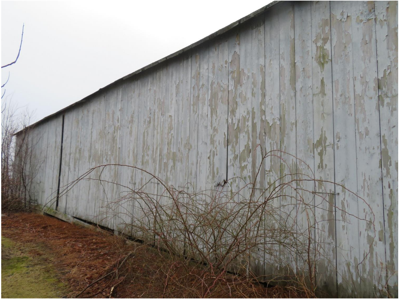
North elevation of shed, camera facing southeast, March 2022.
