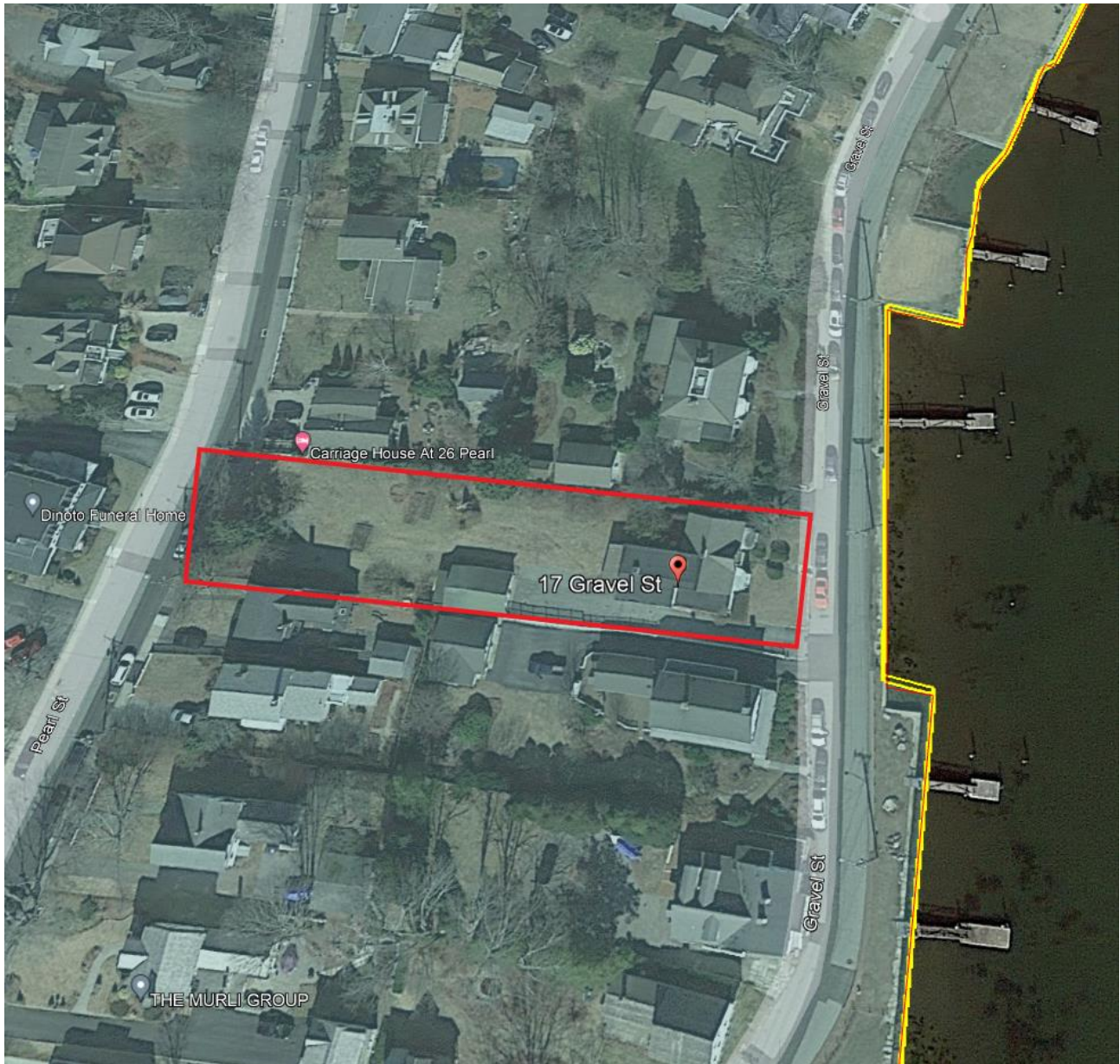
Location of 17 Gravel Street, outlined in red (google earth, 2/22/2020).
