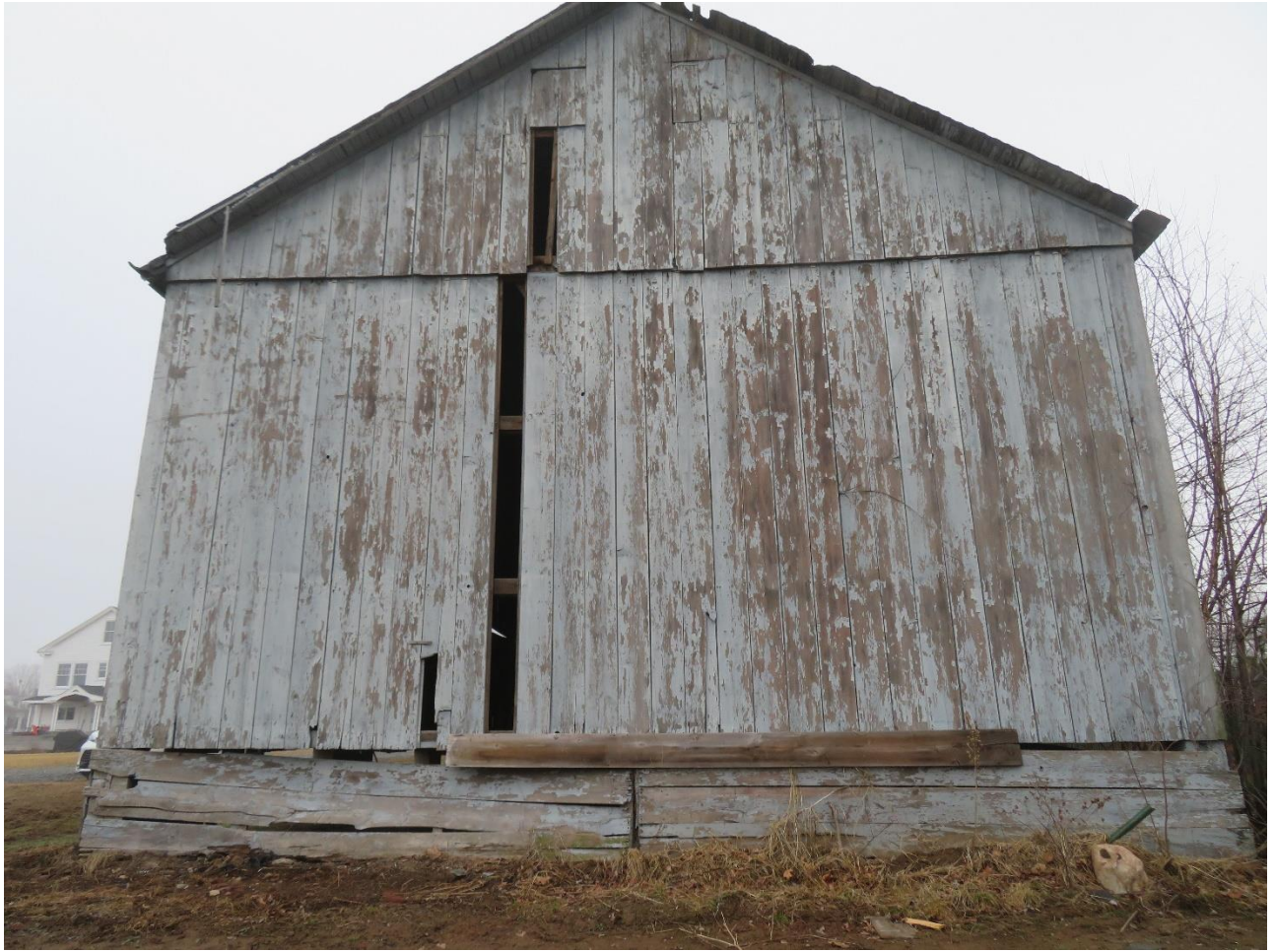
East elevation of shed, camera facing west, March 2022.
