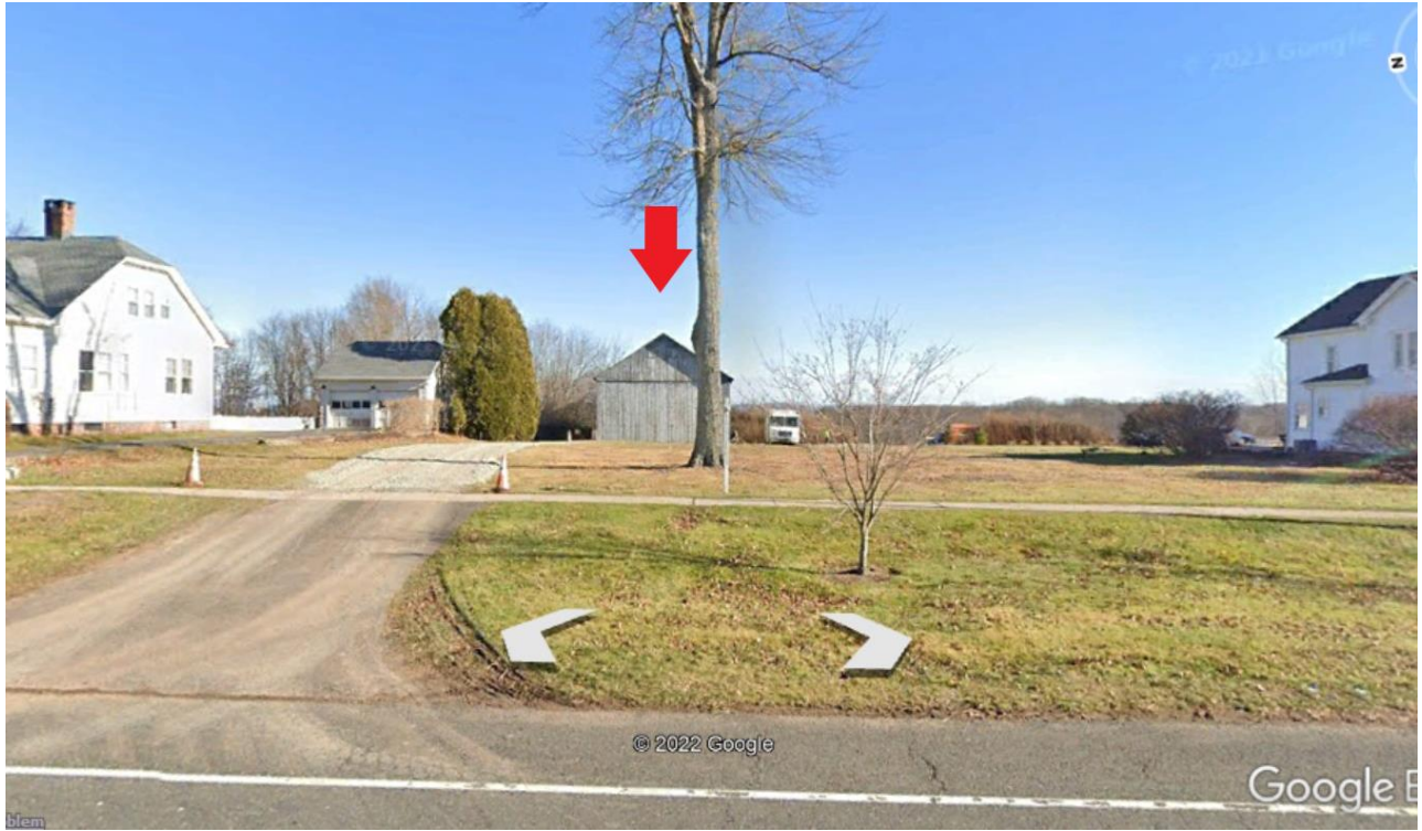
510 North Main Street, Suffield, camera facing east, tobacco shed in center, Google Earth , December 2021.
