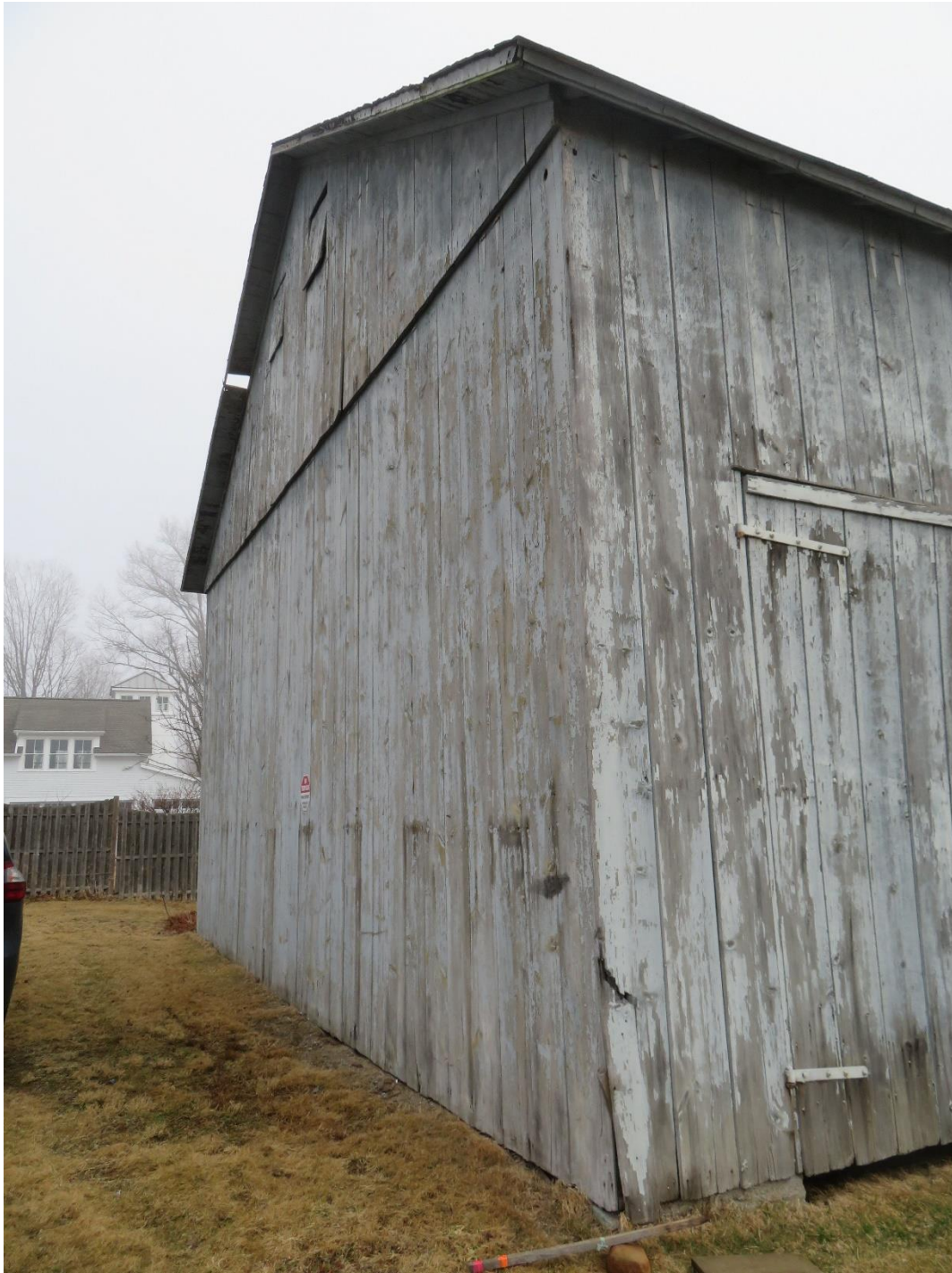
West Elevation of shed, camera facing north, March 2022.
