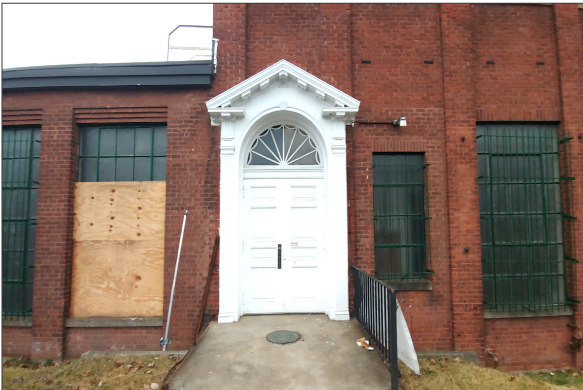
2. HSM Factory, entry detail, 1915 Block, camera facing south.
