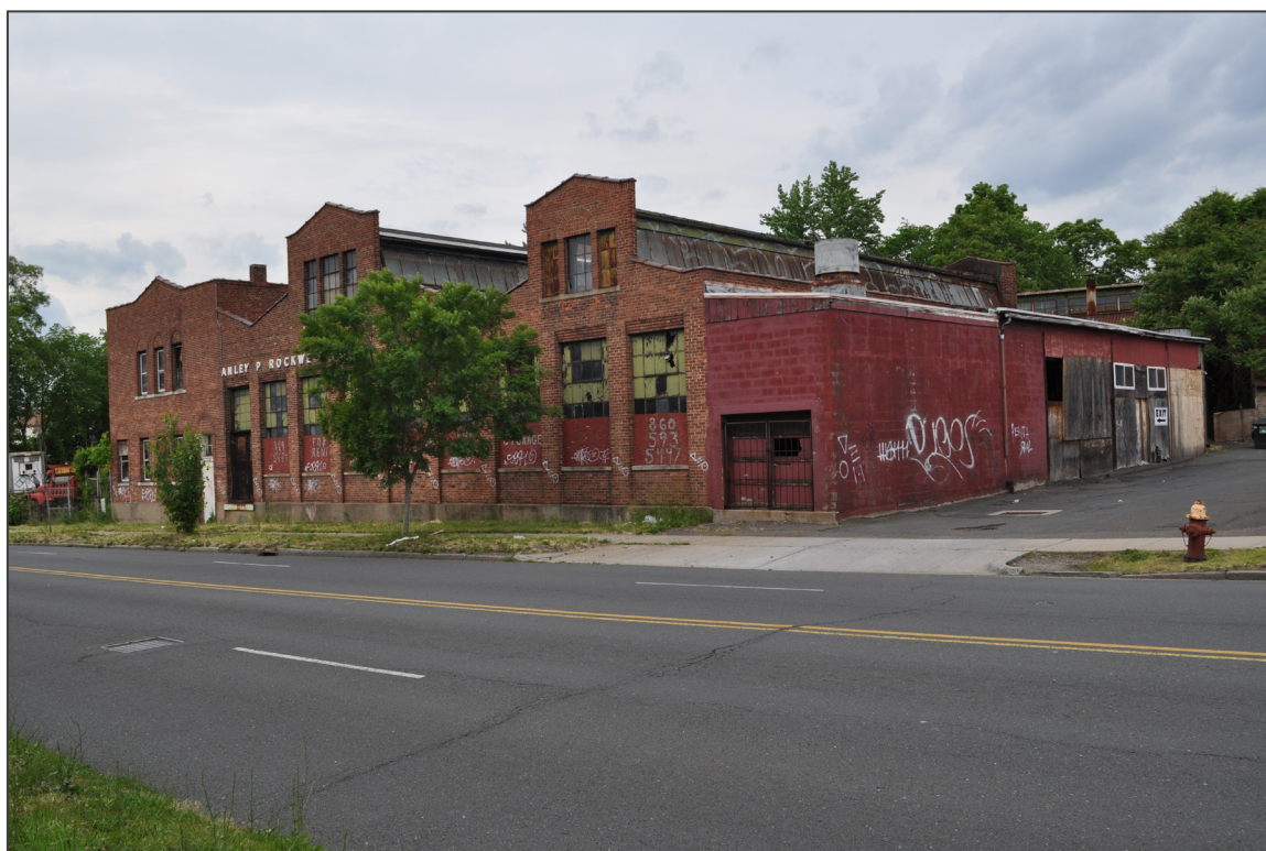
28. Stanley Rockwell Company Factory, south and east elevations, 1929, 1943, and ca. 1970 additions (left), camera facing northwest.
