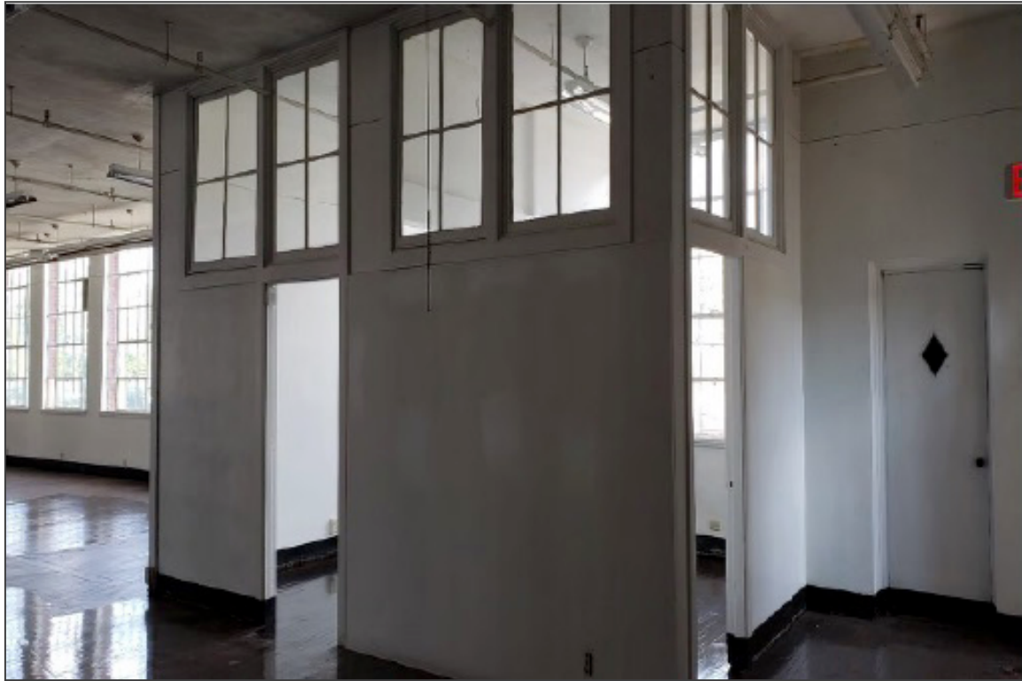
19. HSM Factory, 1915 Block, (1938 second floor addition), camera facing northwest.
