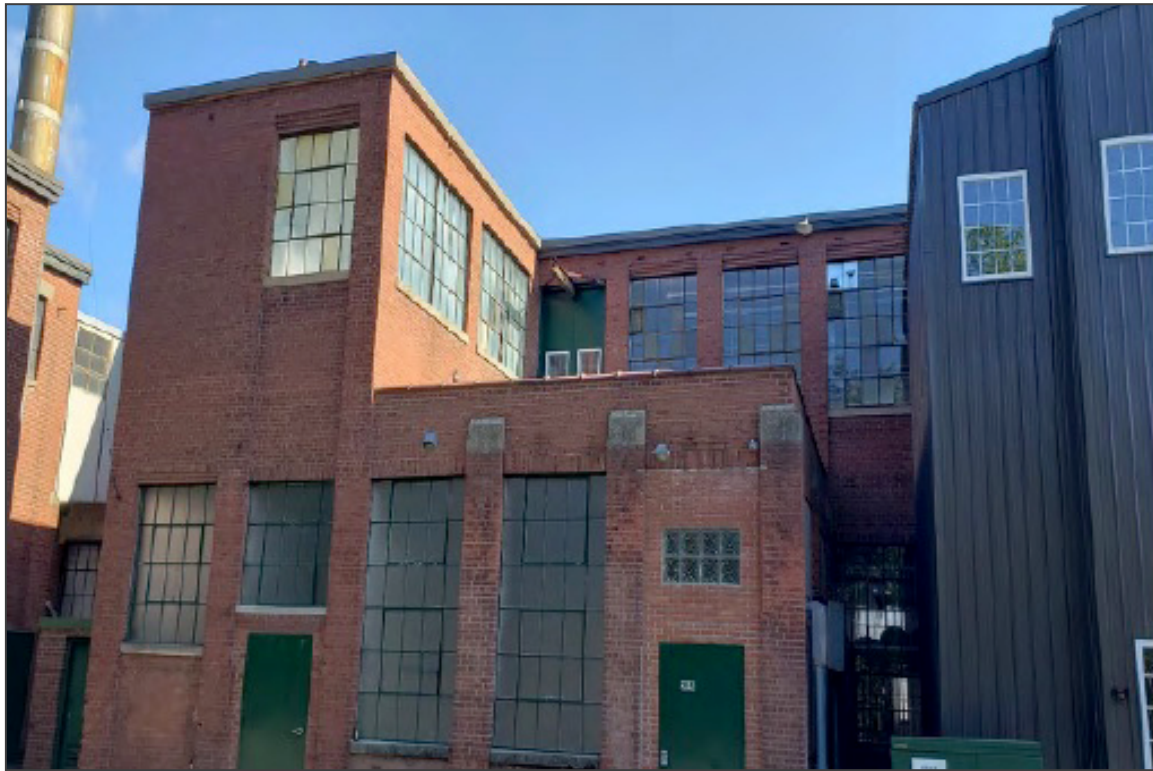
11. HSM Factory, south elevation, 1915 Block, camera facing north.
