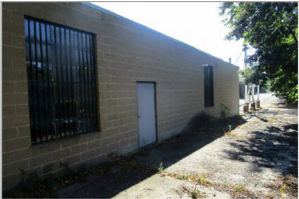
14. HSM Factory, south elevation, 1920 Block (ca.1945 addition), camera facing northeast.
