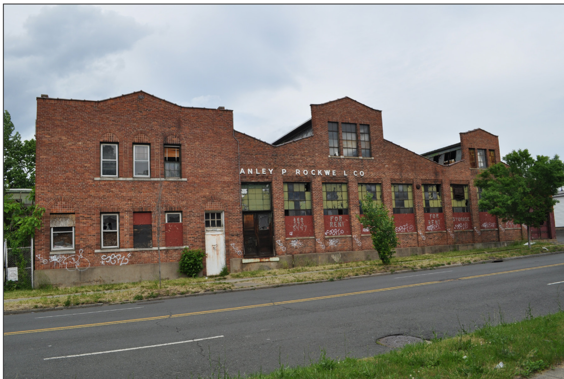
27. Stanley Rockwell Company Factory, South elevation, 1929 office and manufacturing blocks (left and center) and 1943 addition (right), camera facing northeast.
