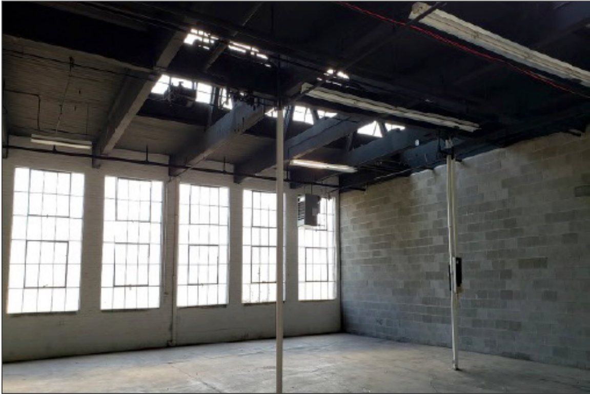
25. HSM Factory, 1942 Block, first floor, camera facing northeast.
