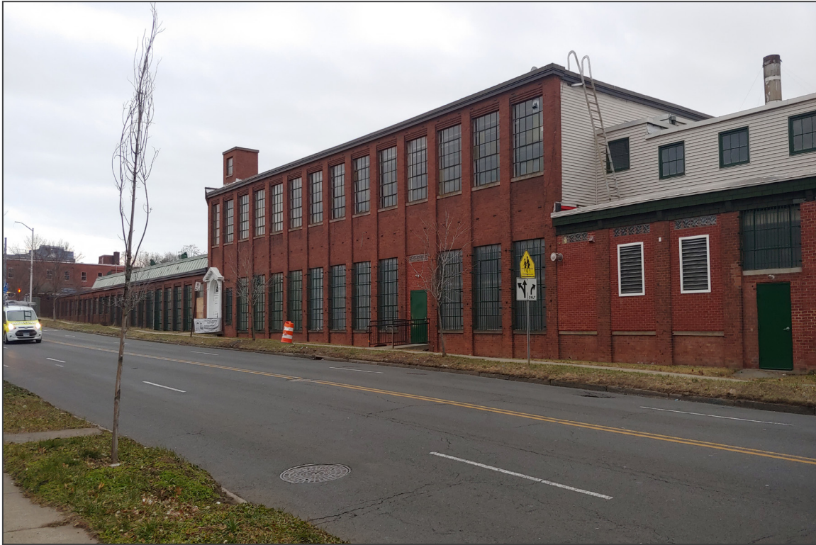
1. HSM Factory, north elevation, 1942 Block (left), and 1915 Block (right), camera facing southeast.
