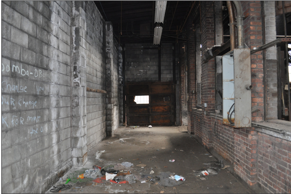
39. Stanley Rockwell Company Factory, 1929/1970 addition, camera facing south.
