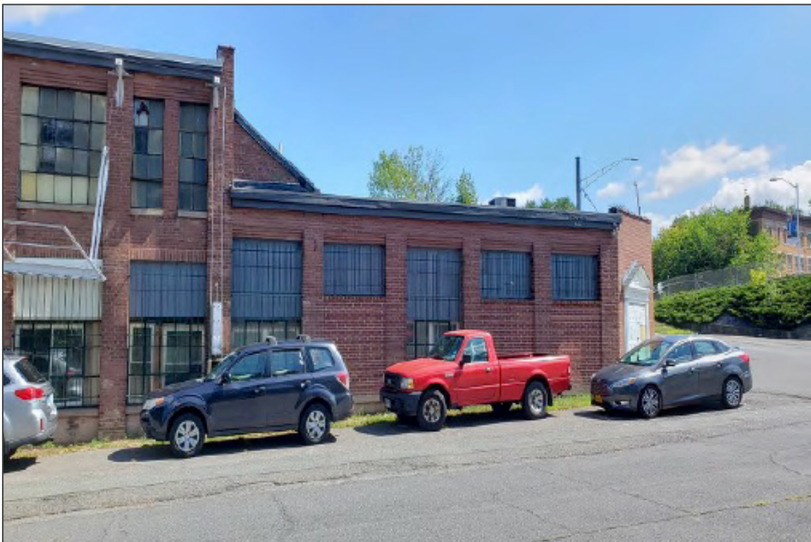
8. HSM Factory, south elevation, 1942 Block, camera facing northeast.
