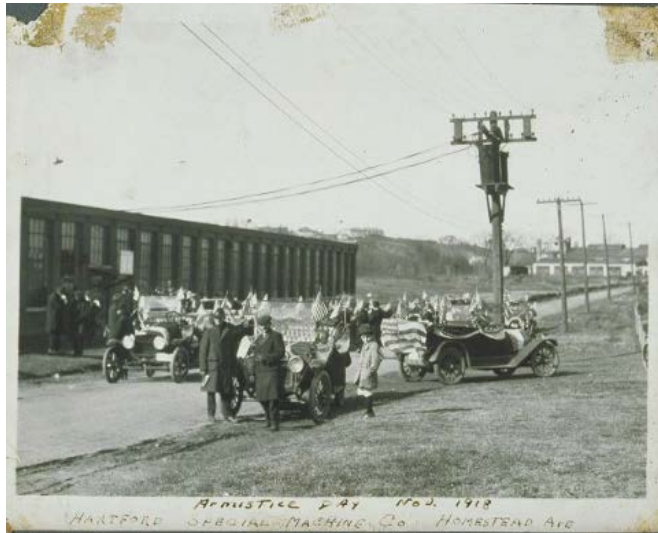
Figure 22: The northern elevation of the Hartford Special Machinery Company building taken on Armistice Day, November 1918, showing the western end of the building prior to its 1920 addition.
