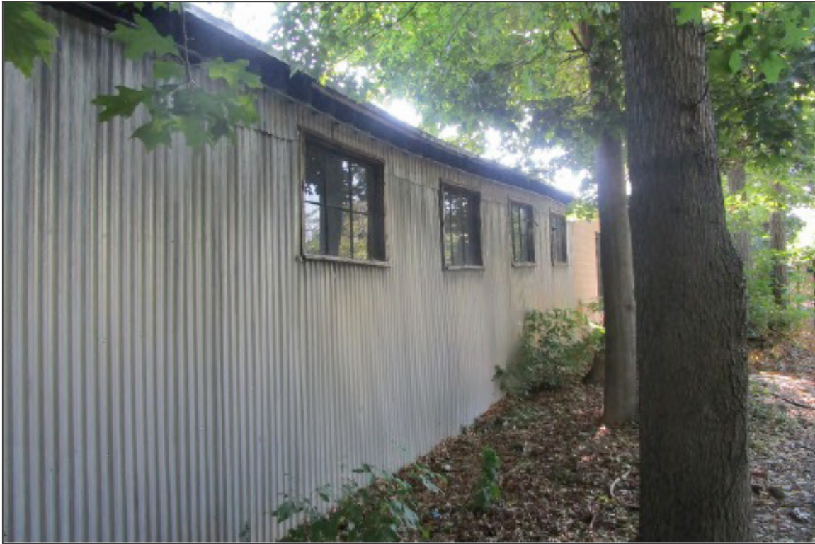
15. HSM Factory, south elevation, 1920 Block (ca. 1945 addition), camera facing northeast.
