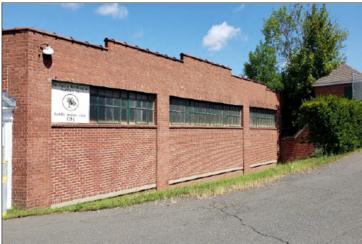
6. HSM Factory, east Elevation 1942 Block (left) and south elevation Guard House (right), camera facing northwest.
