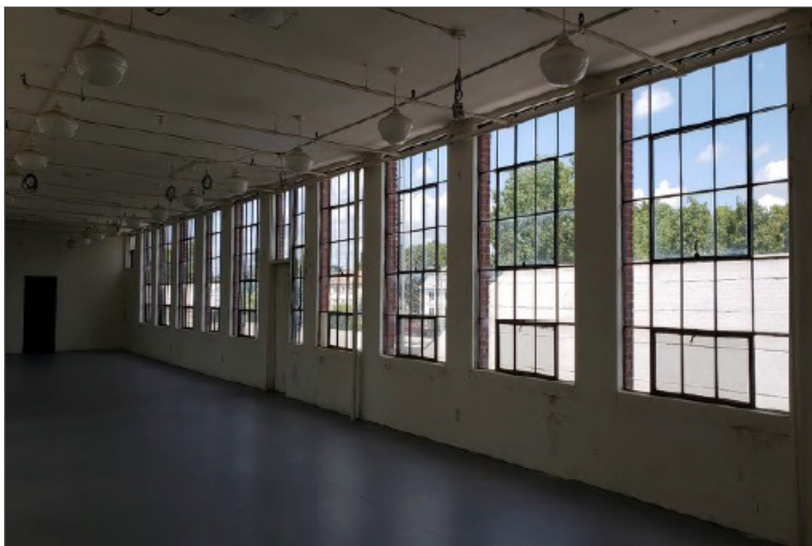
18. HSM Factory, 1915 Block, (1938 second floor addition), camera facing northwest.
