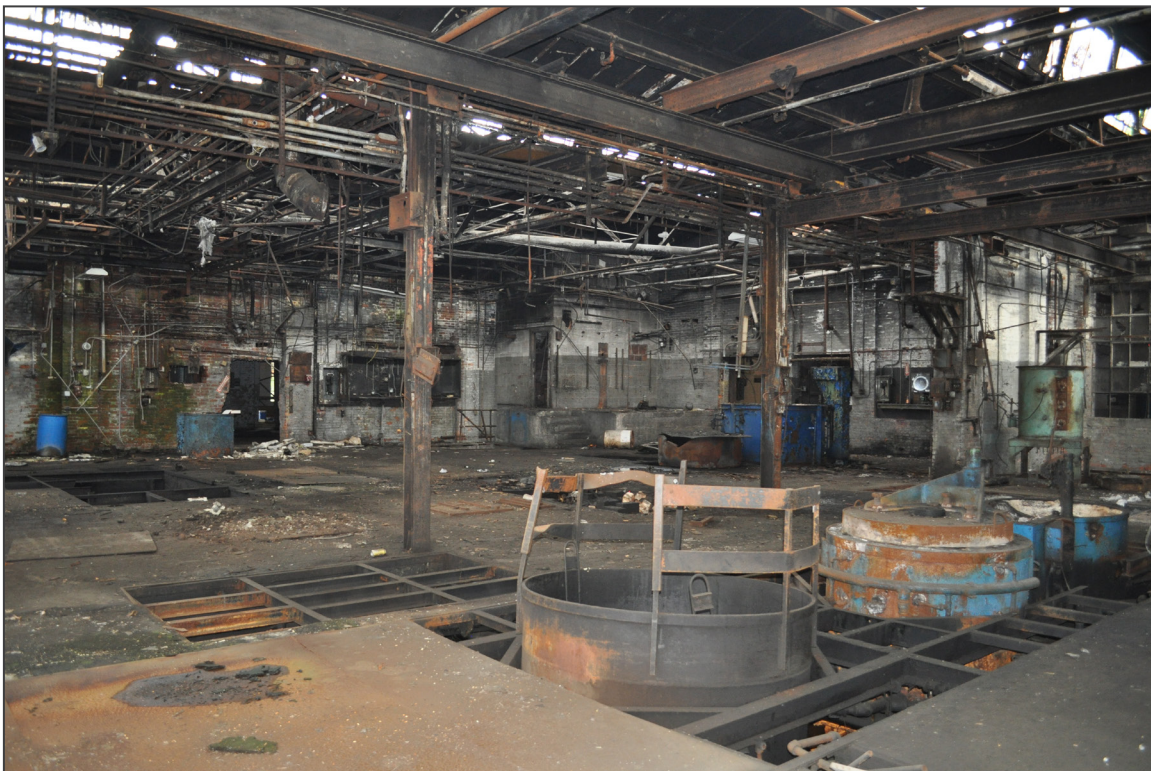
38. Stanley Rockwell Company Factory, 1929 and 1943 manufacturing blocks, camera facing northwest.
