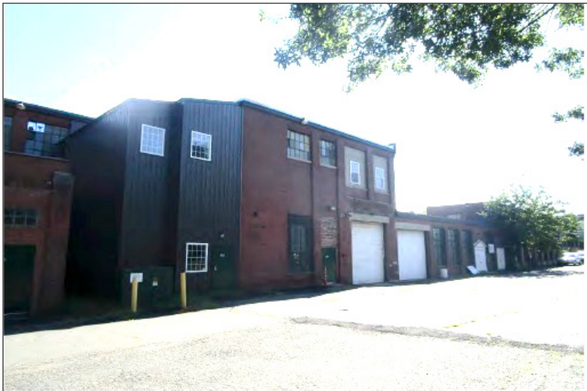
10. HSM Factory, south elevation, 1915 Block and 1942 Block, camera facing northeast.
