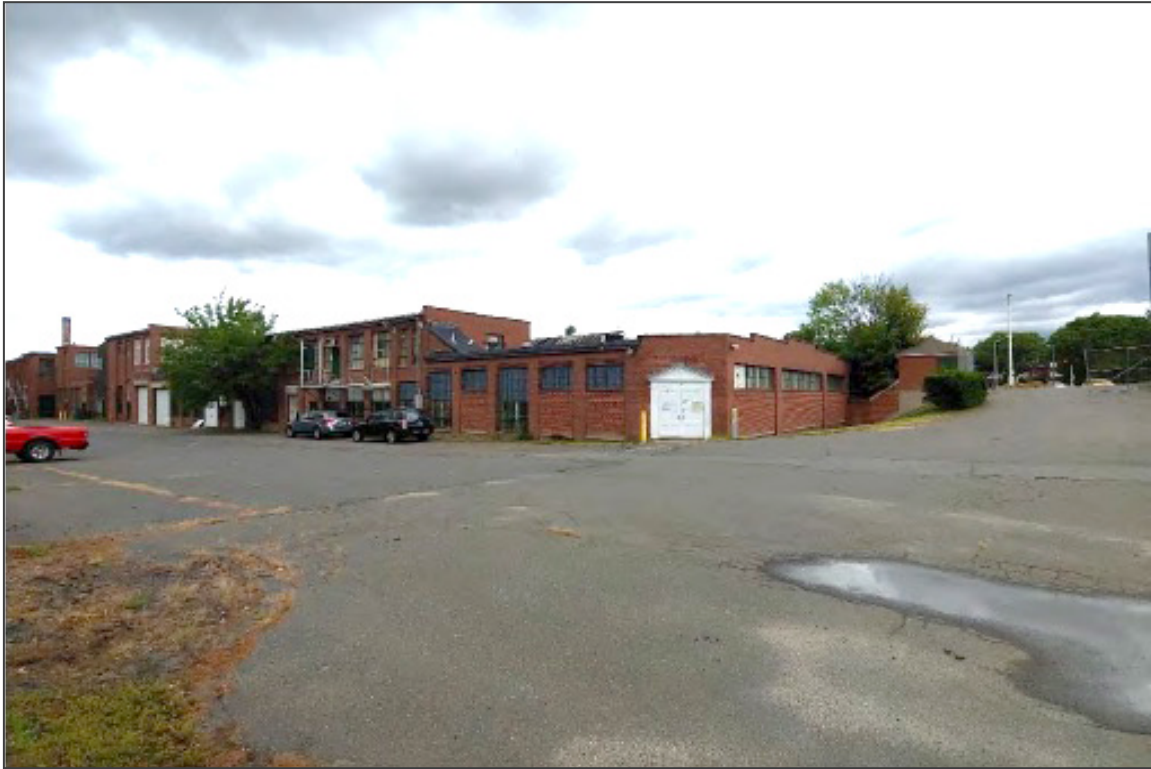
7. HSM Factory, east and south elevations, 1942 Block, camera facing northwest.
