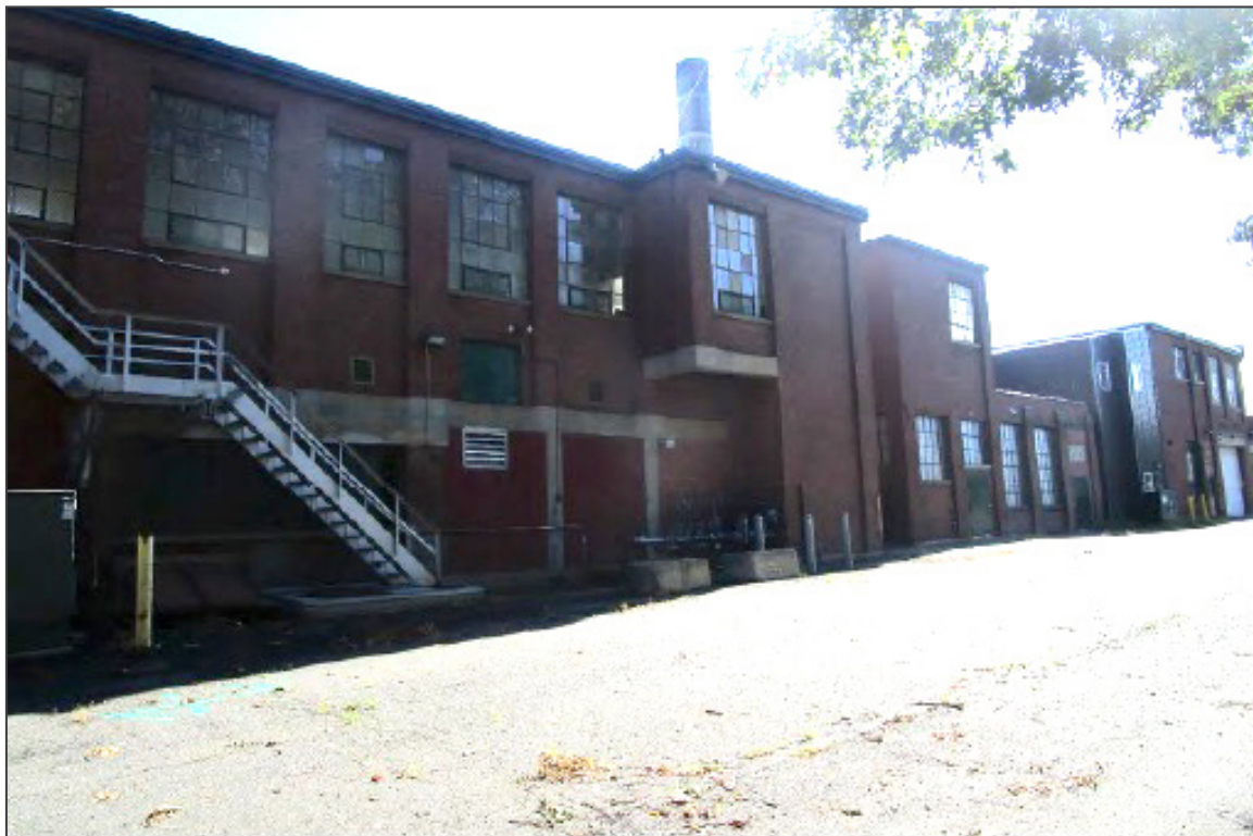
12. HSM Factory, south elevation, 1915 Block, camera facing northeast.
