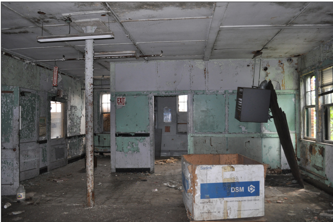
36. Stanley Rockwell Company Factory, 1929 second floor office, camera facing southeast.
