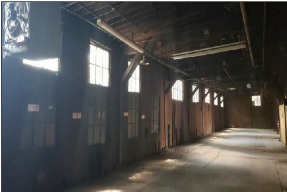
24. HSM Factory, 1920 Block (ca.1945 addition), camera facing southwest.
