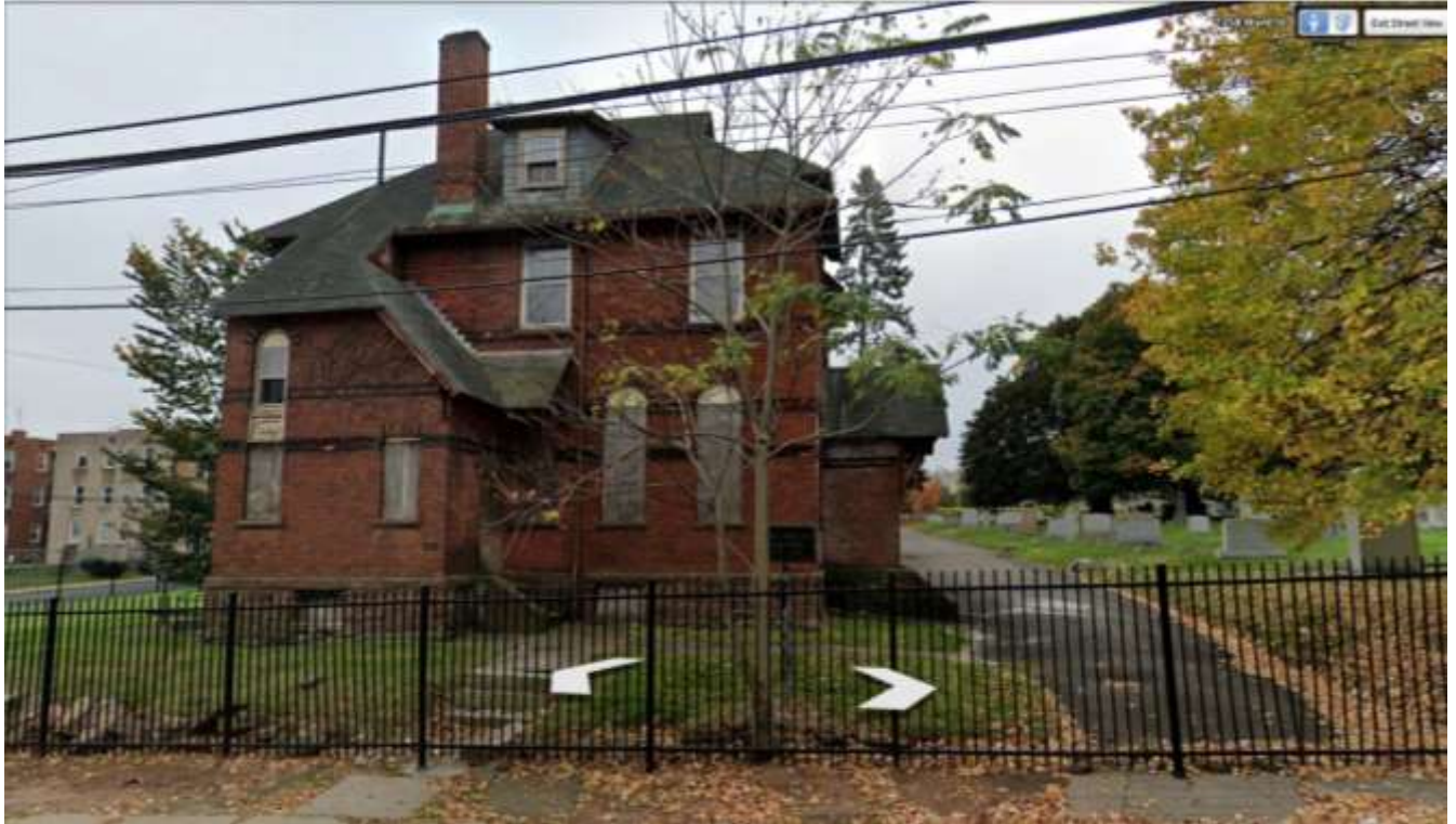
Deborah Chapel, north elevation. Main entrance is to the right, on the west elevation (google earth, 10/2020).
