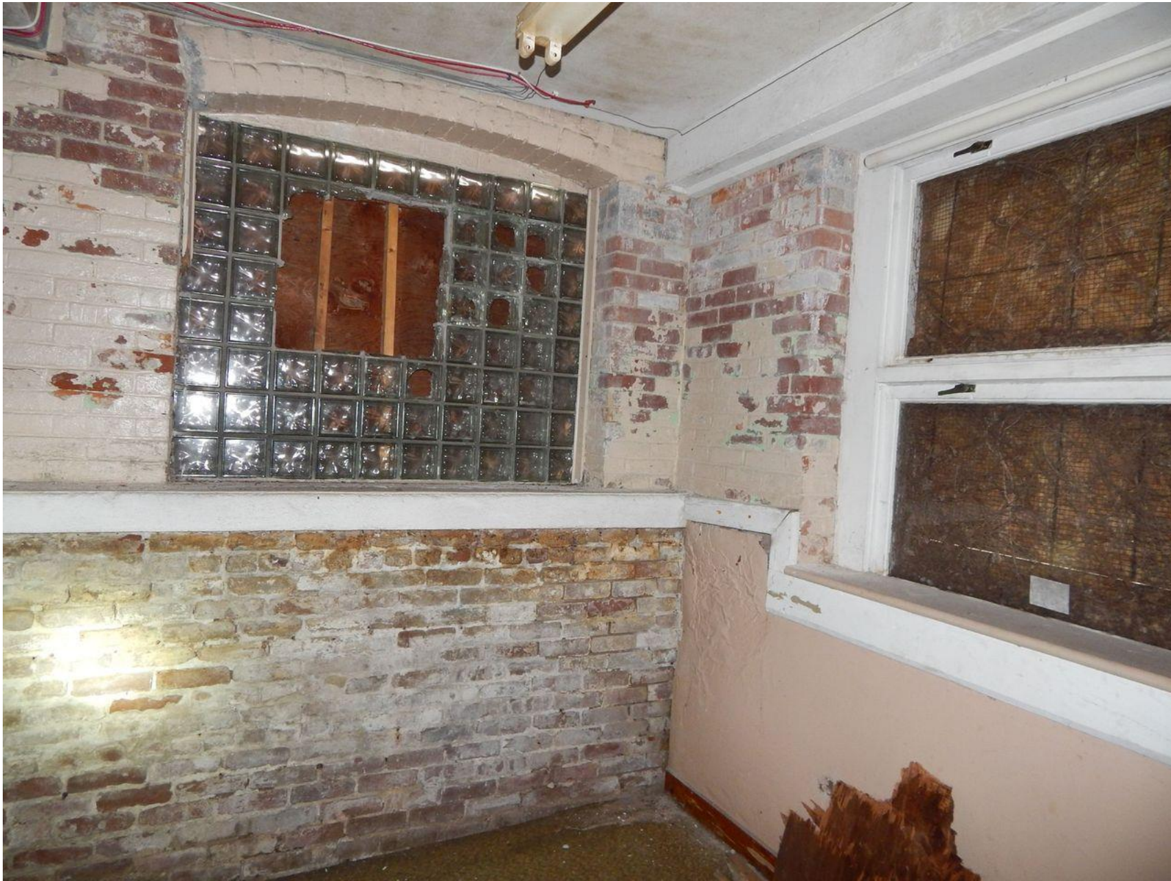
Interior first floor. Southeastern office. Camera facing southeast. Photograph 12 of 37
