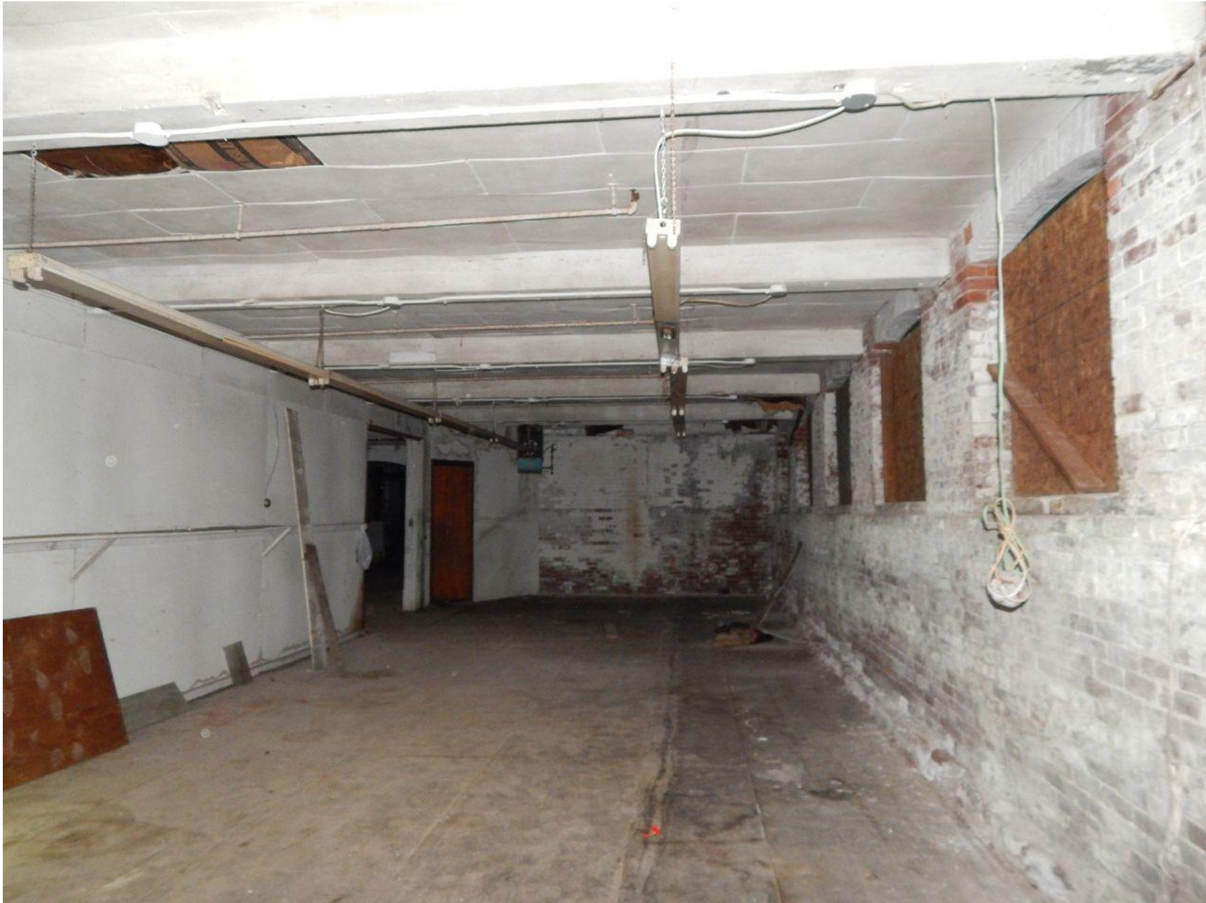
First floor interior space. Camera facing north. Photograph 15 of 37
