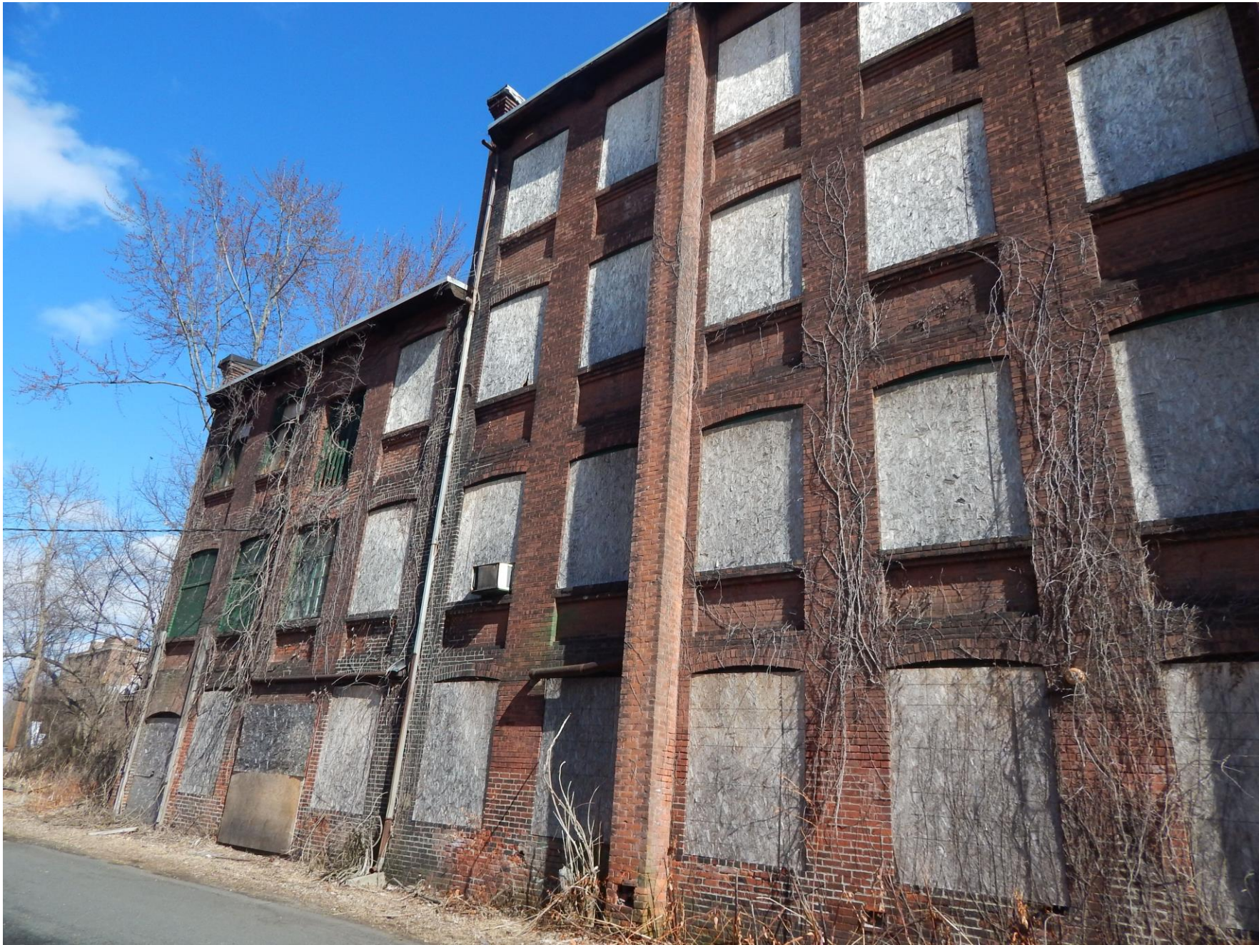
Detail of northern block western elevation. Camera facing northeast.
