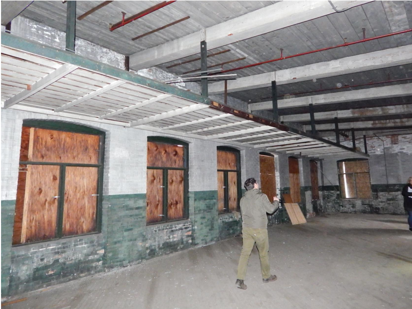
Fourth floor interior. Camera facing north. Photograph 35 of 37
