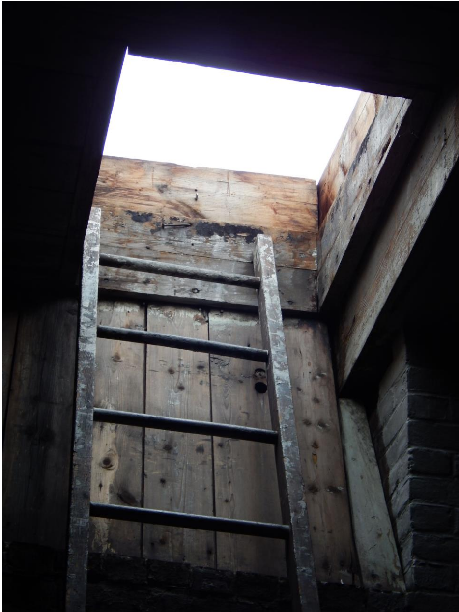
Fourth floor roof exit. Camera facing west. Photograph 37 of 37
