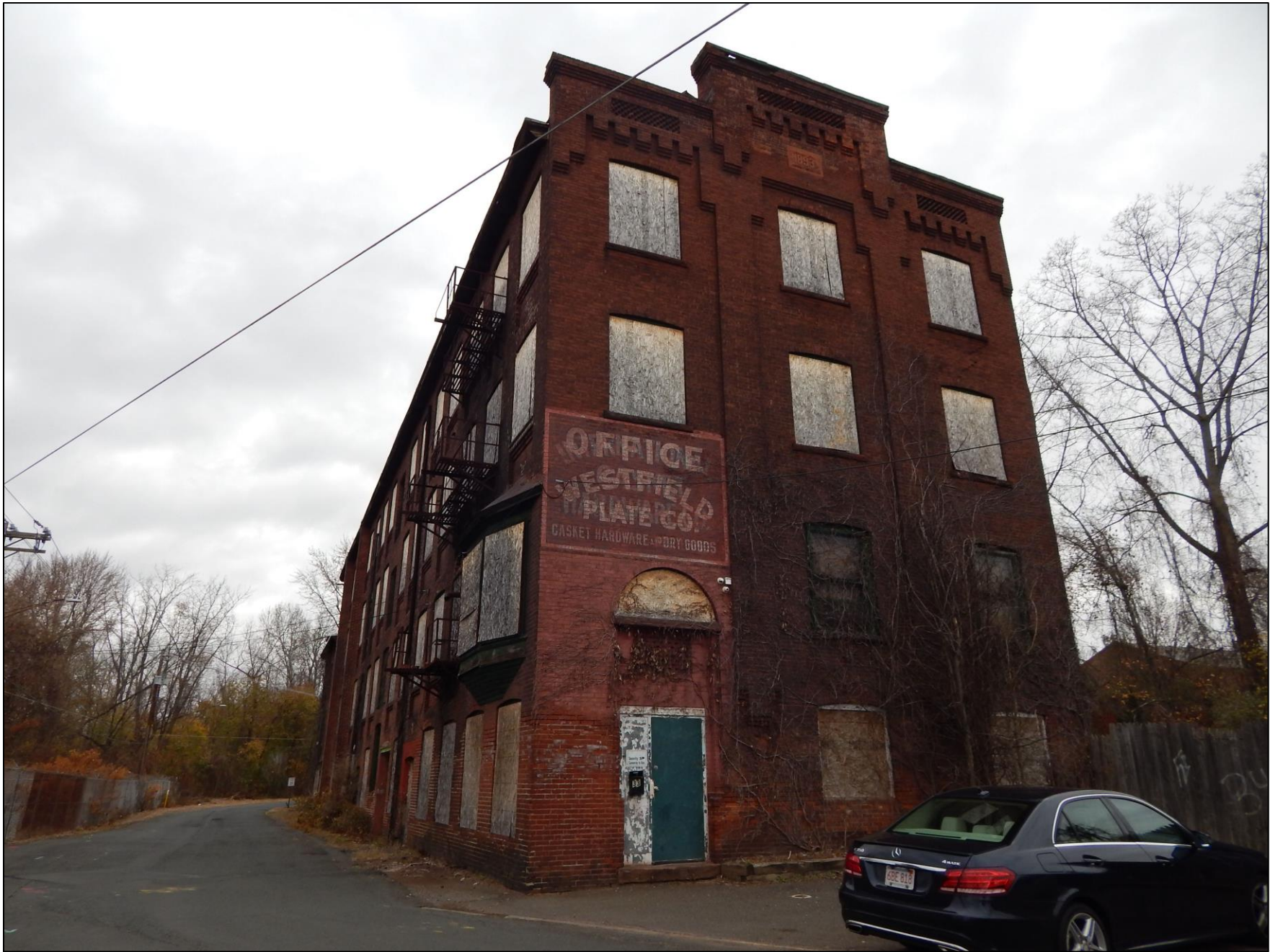
Southern elevation (façade) and western elevation (side). Camera facing northeast. Photograph 1 of 37
