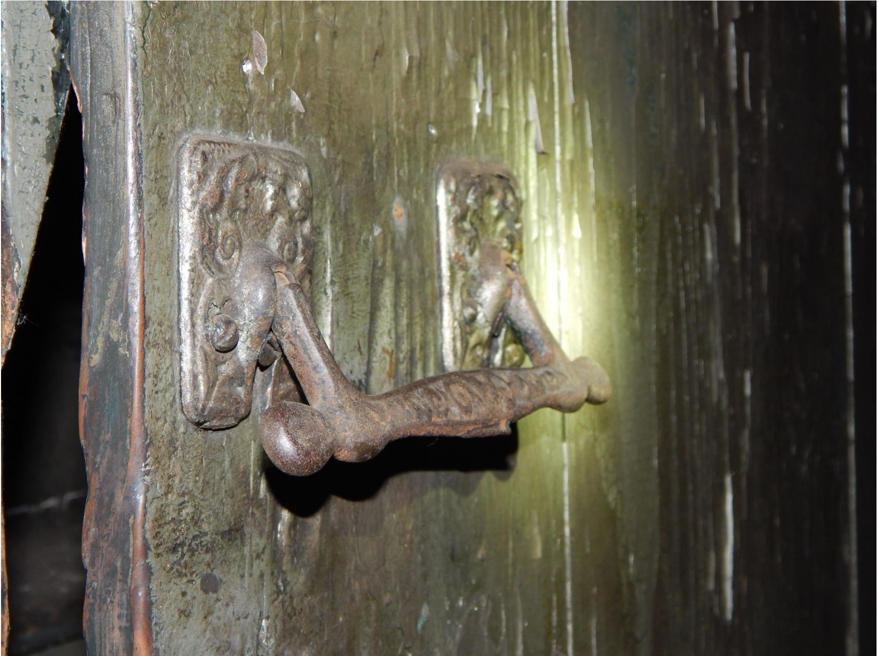
Second floor. Detail of casket handle repurposed for door. Photograph 31 of 37
