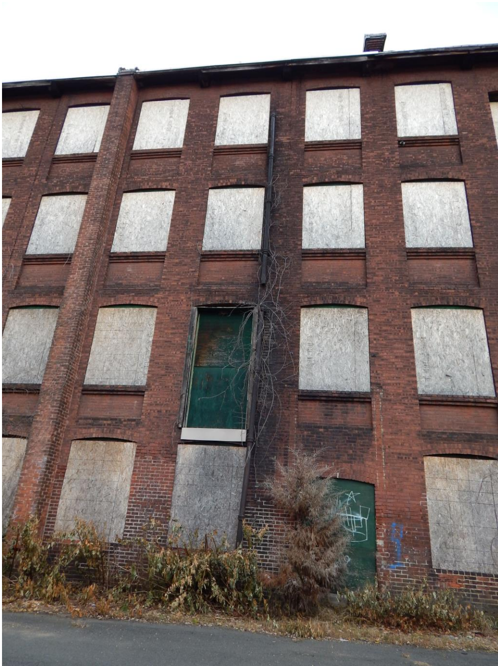
Detail of western elevation of southern block. Camera facing east.
