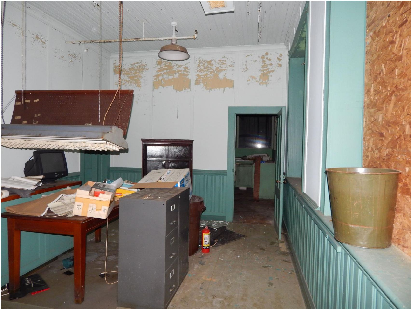
Second floor interior office space. Camera facing north. Photograph 20 of 37
