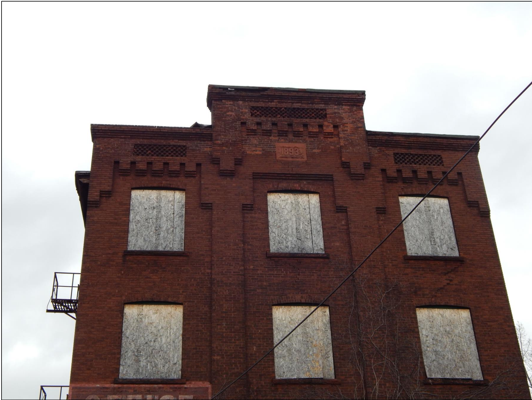
Southern Elevation (façade) brickwork detail. Camera facing north.
