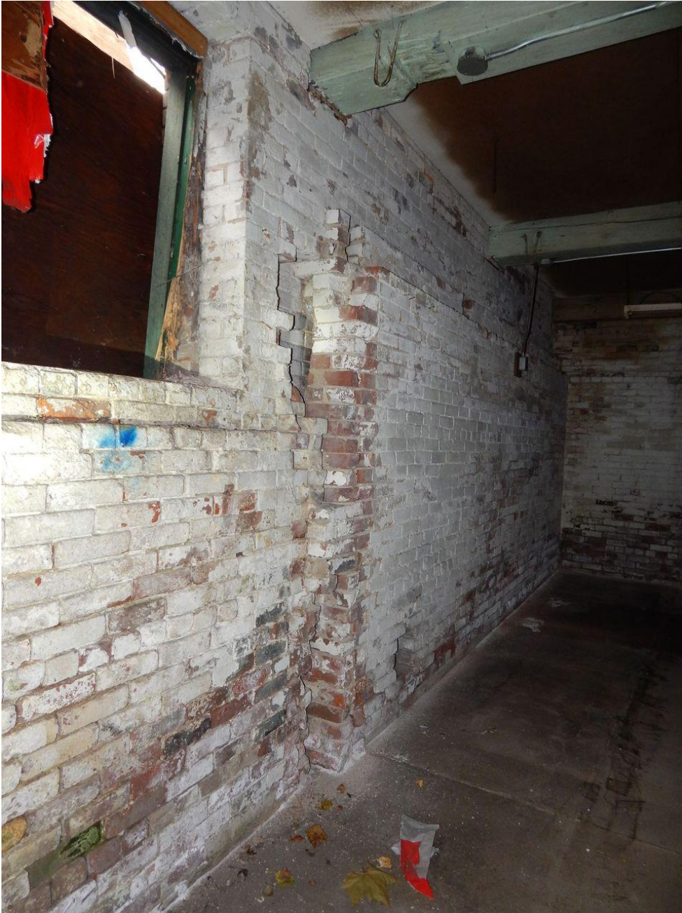
First floor remnants of casting operation. Camera facing south. Photograph 17 of 37
