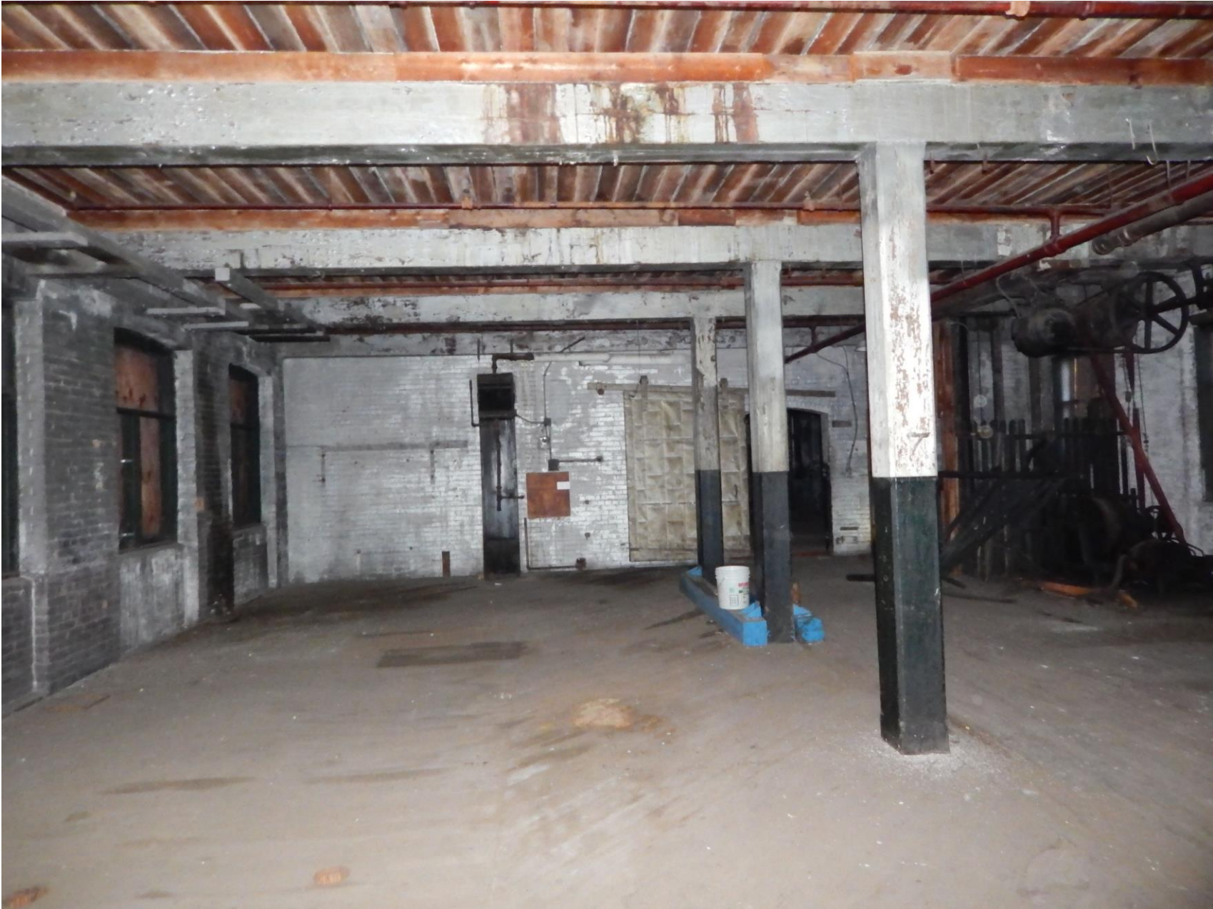
Third floor interior space. Camera facing south. Photograph 33 of 37
