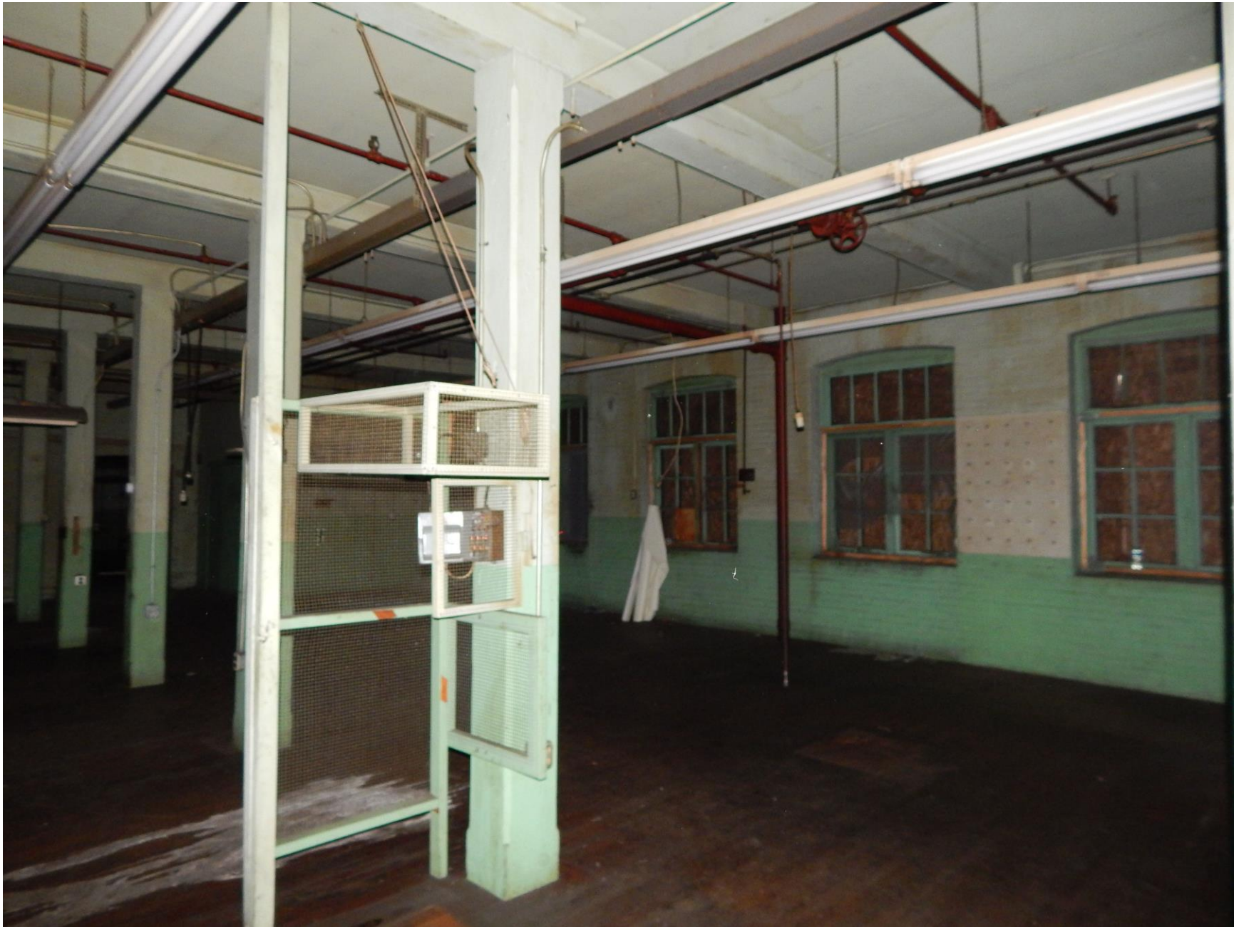
Second floor. Open manufacturing space. Camera facing northeast.
