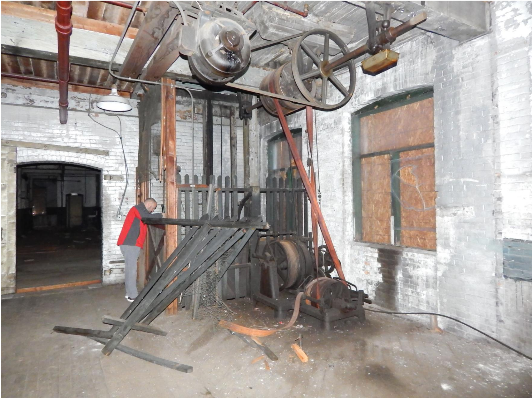
Third floor interior elevator. Camera facing southwest. Camera facing 34 of 37
