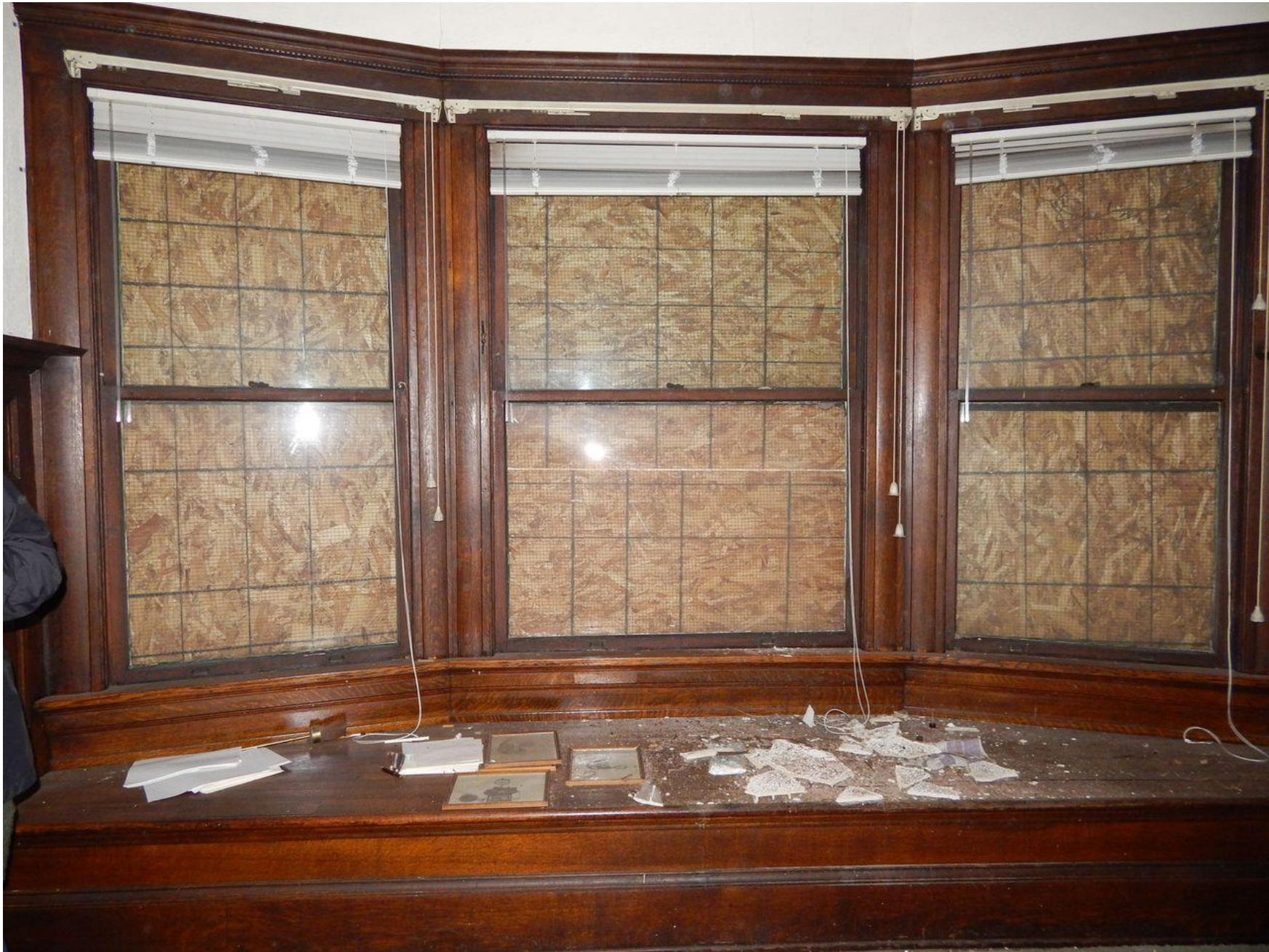
Interior detail of bay window. Camera facing west. Photograph 24 of 37
