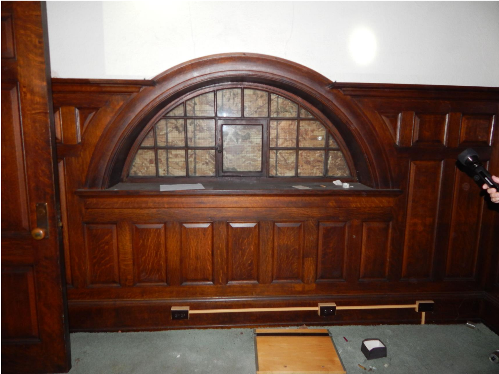
Interior shot of boarded transom window. Camera facing south. Photograph 25 of 37
