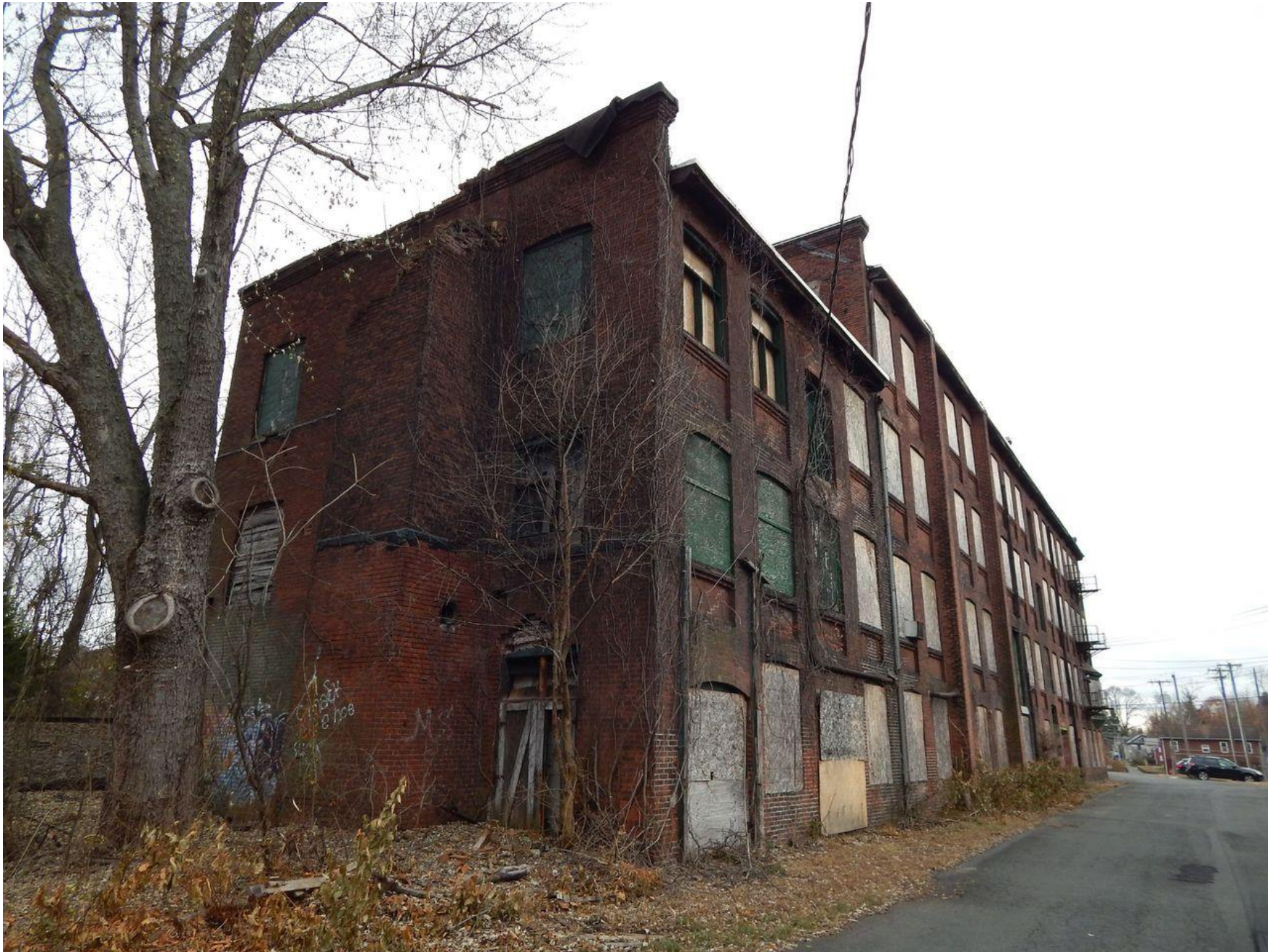
Northern elevation of northern block and western elevation. Camera facing southwest.
