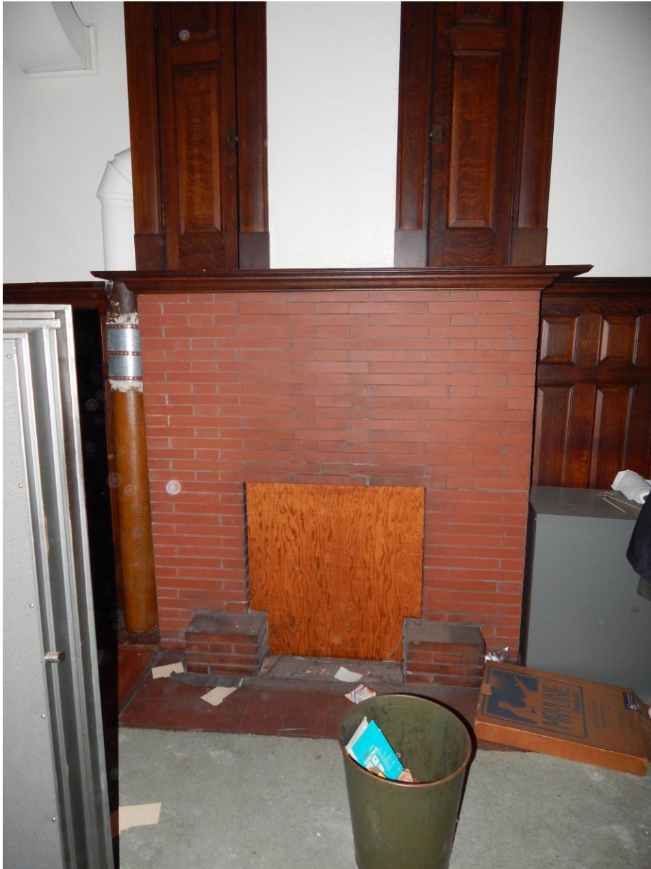
Second floor interior. Manager's office fireplace. Camera facing east. Photograph 23 of 37
