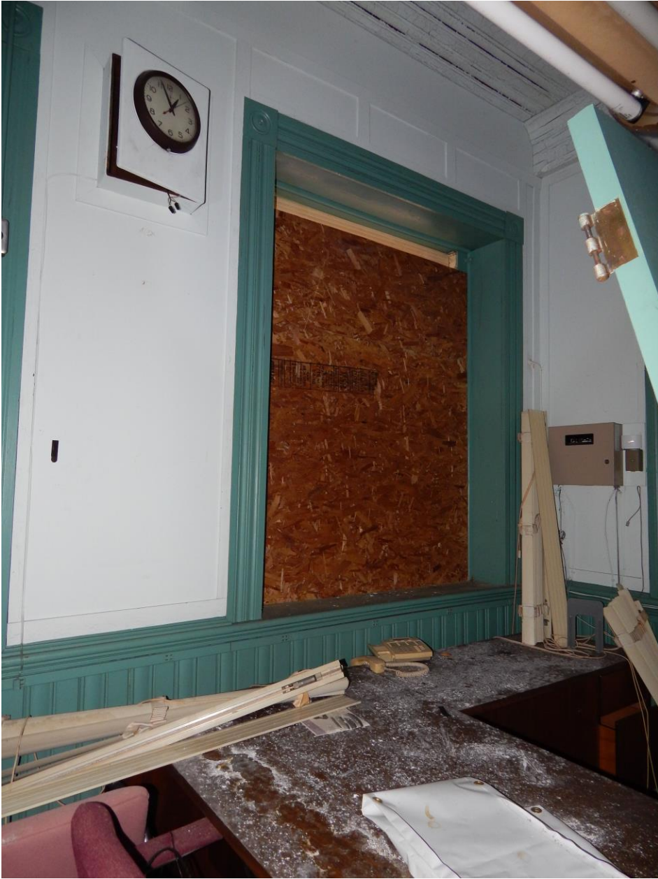
Second floor interior detail. Camera facing southeast. Photograph 21 of 37
