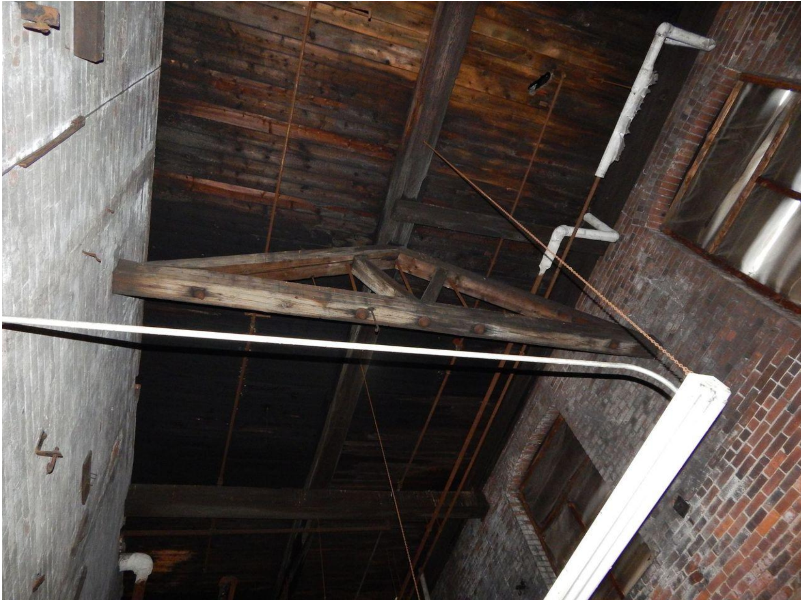
Interior of northern boiler room. Detail of support truss. Photograph 19 of 37
