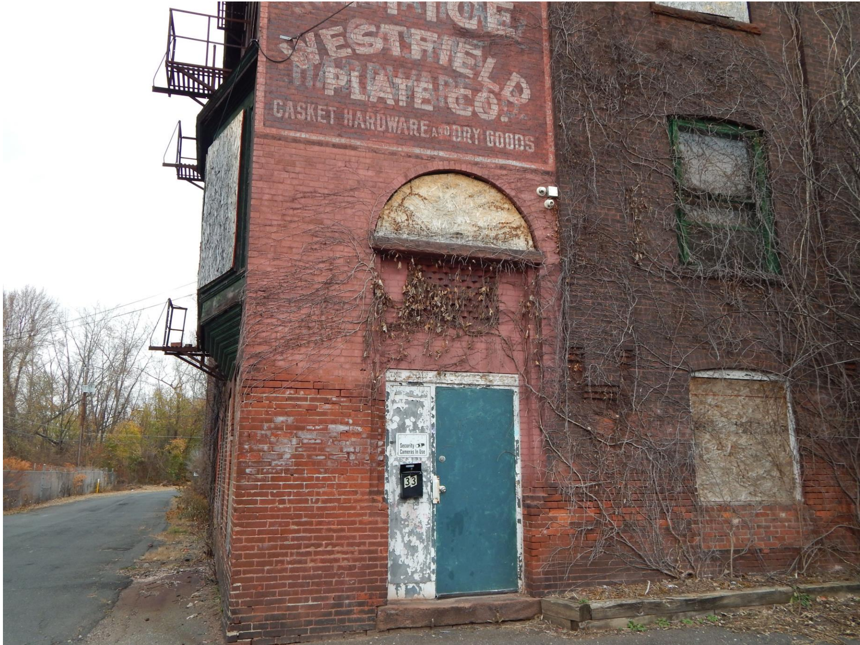
Southern elevation (façade) entryway detail. Camera facing north. Photograph 3 of 37
