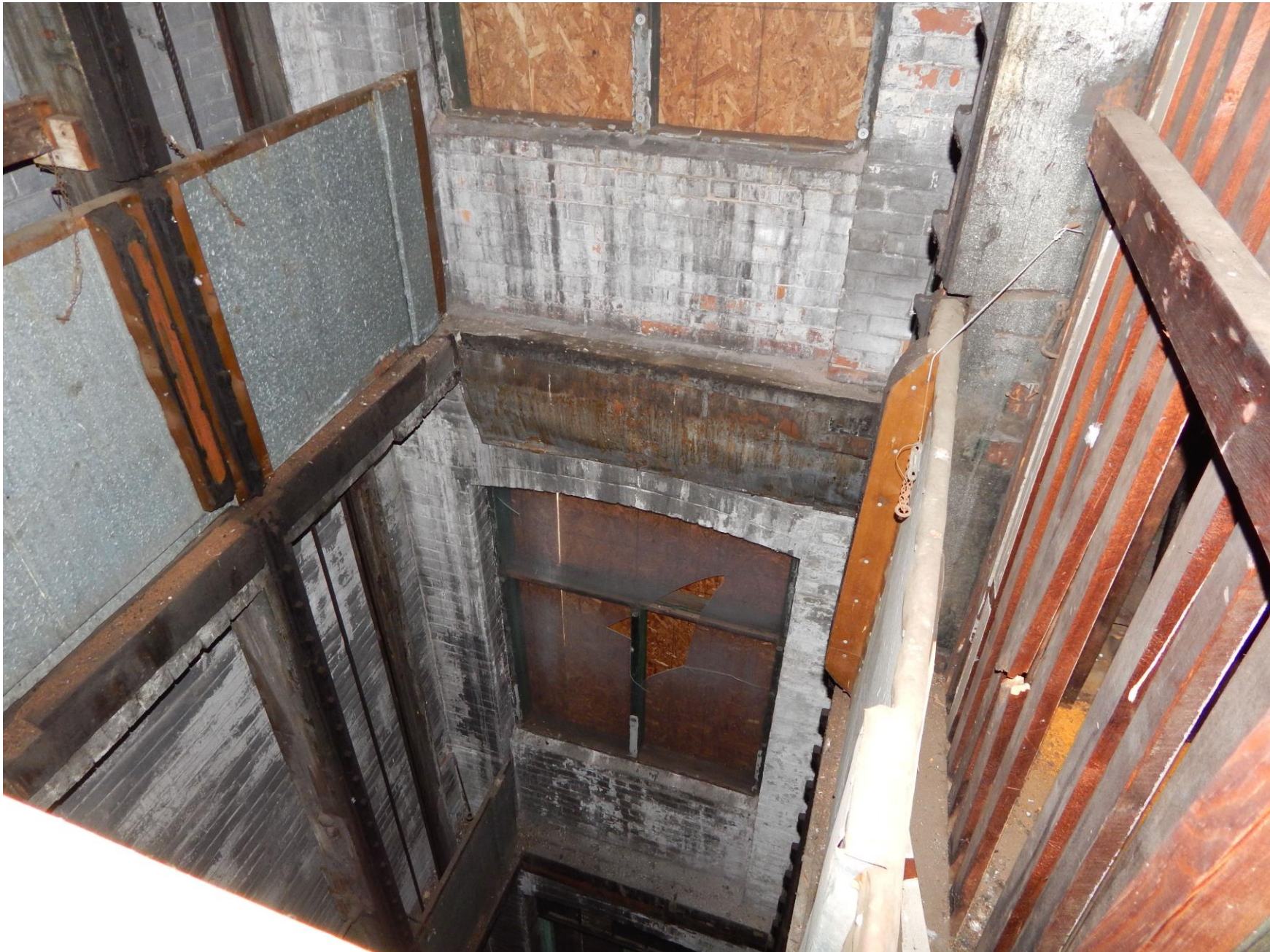
Fourth floor interior elevator shaft. Photograph 36 of 37
