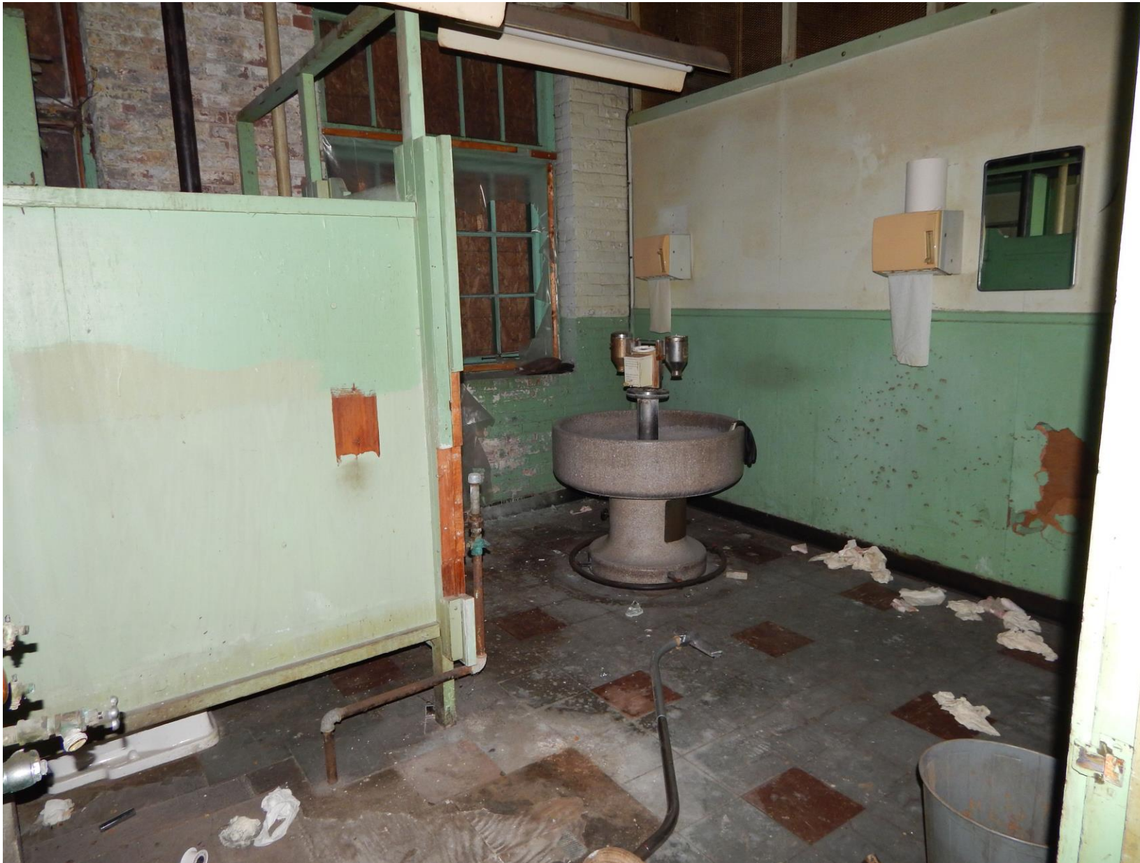
Second floor interior bathroom. Camera facing northwest. Photograph 26 of 37
