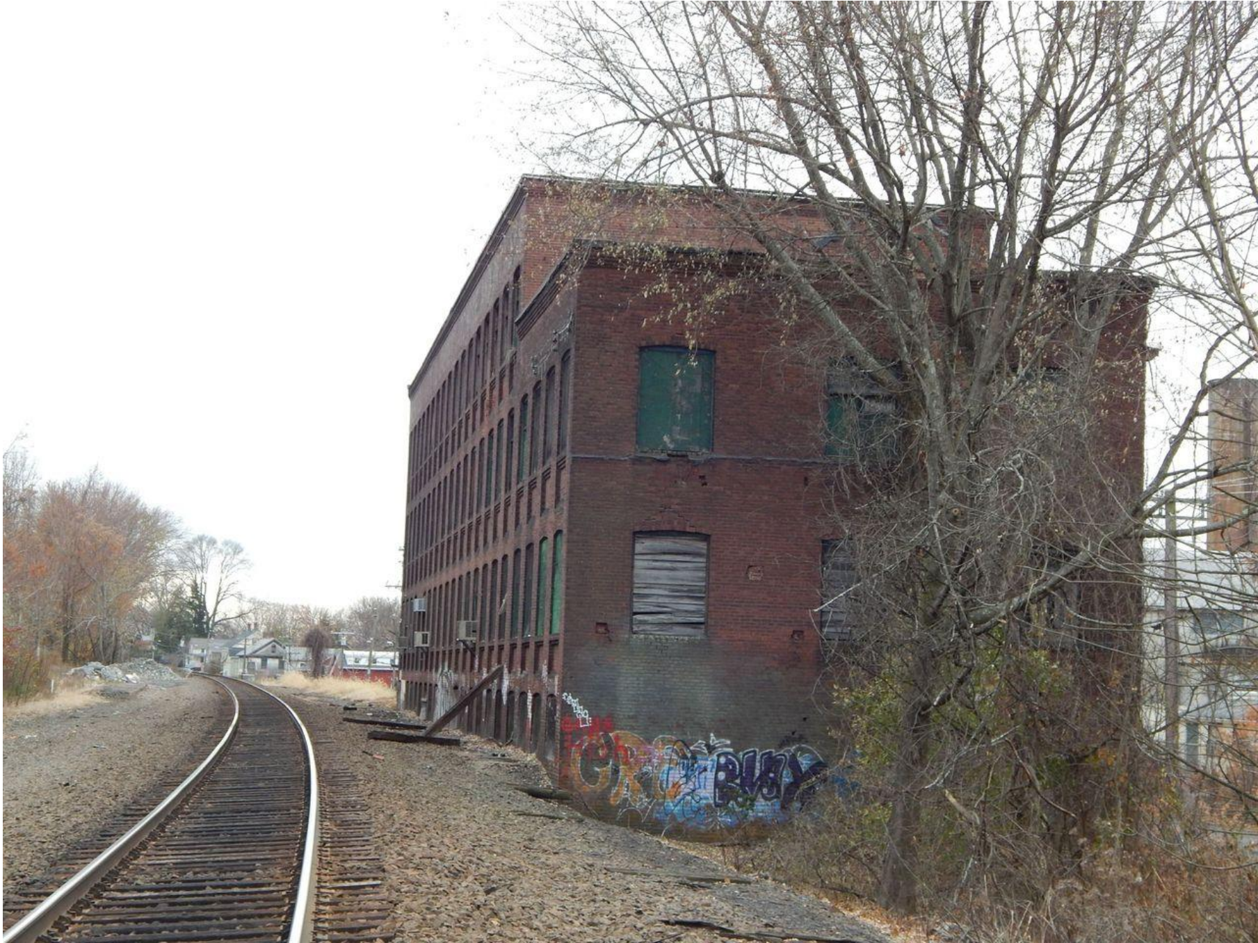
North and eastern elevations showing the “ghost sign” near the roofline of the eastern elevation. Camera facing south.
