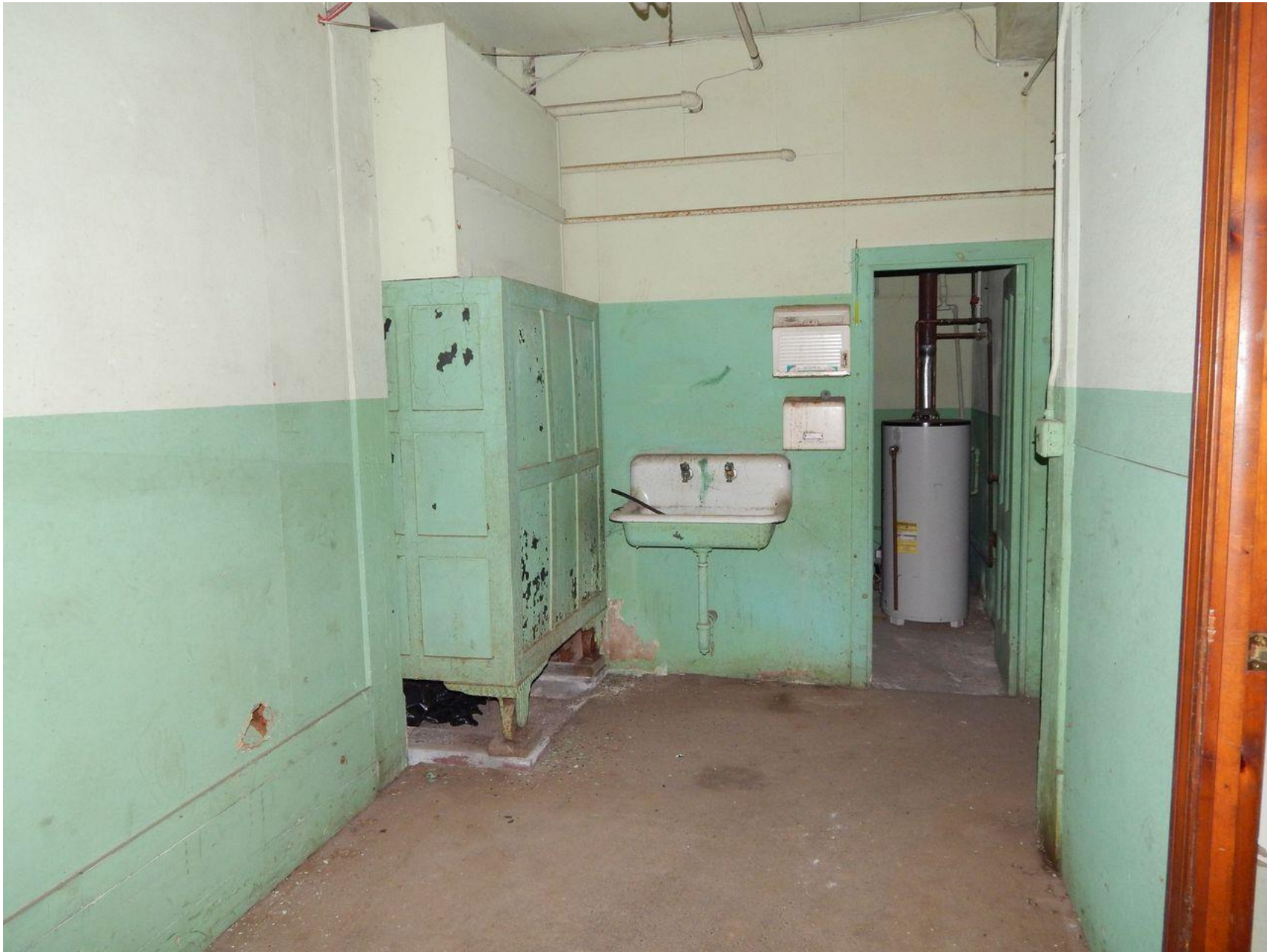
Interior first floor utility room. Camera facing north. Photograph 14 of 37
