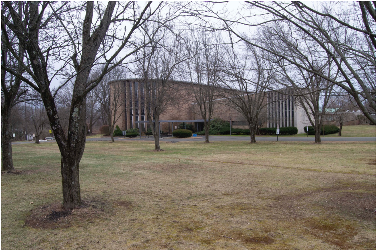
1 of 45 North elevation, setting. Camera facing Southeast.
