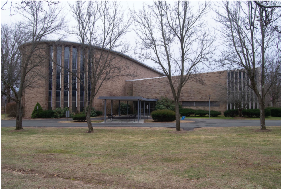
6 of 45. North Elevation, chapel. Camera facing South/Southeast
