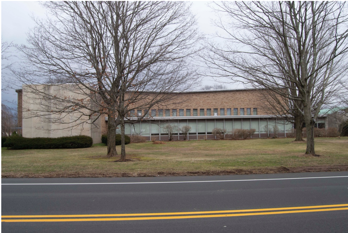
7 of 45. West elevation. Camera facing East.
