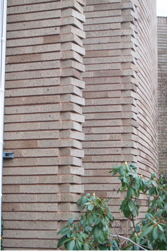
4 of 45. North Elevation, detail of an exterior wall of the sanctuary. Camera facing South.
