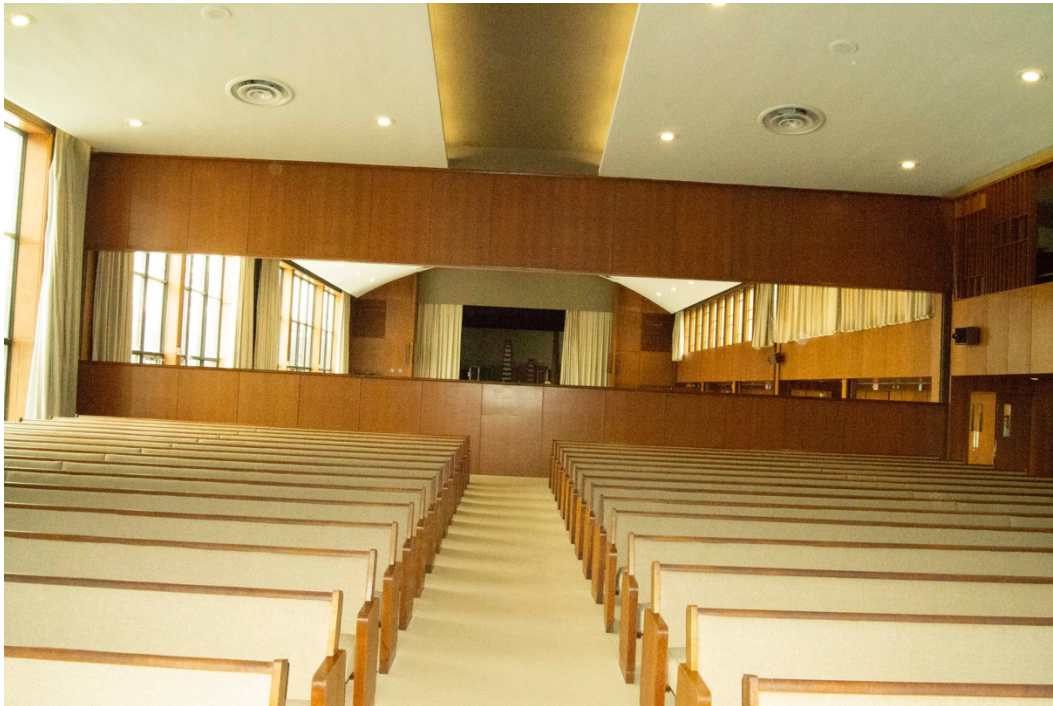
25 of 45. Interior, social hall, rear wall, bi-parting, counterbalanced mechanical partitions.
