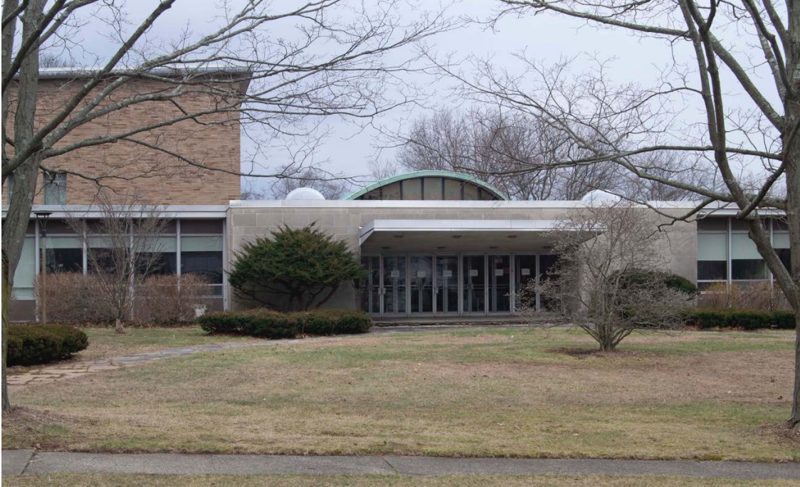
8 of 45. West Elevation, entrance. Camera Facing East.
