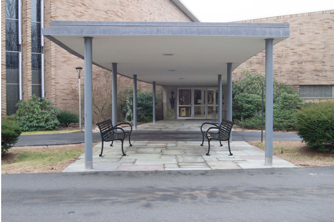
2 of 45 North elevation, entrance. Camera facing South.
