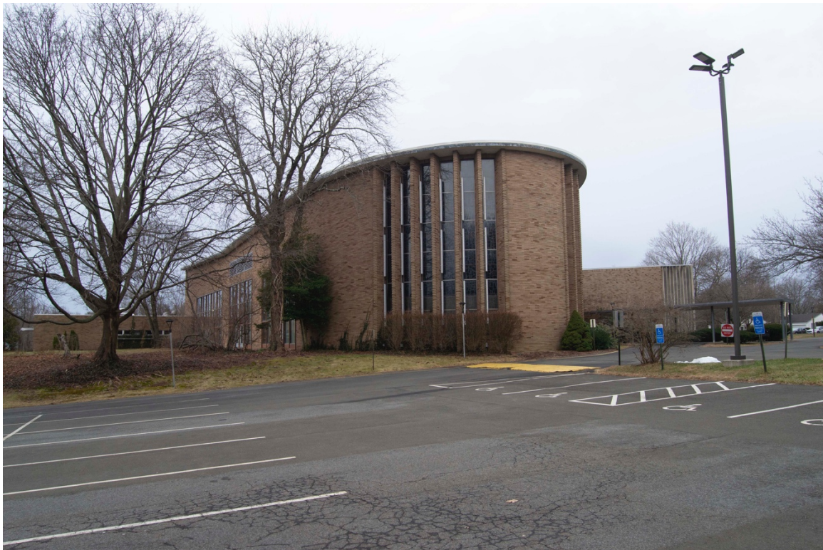
3 of 45. North Elevation. Camera facing Southwest.
