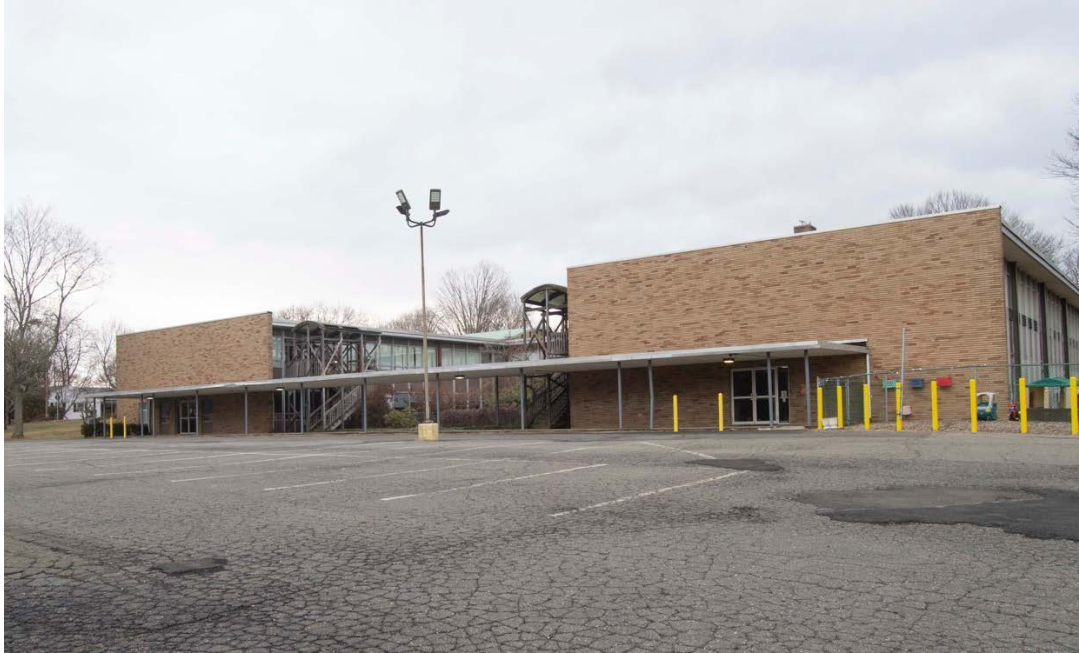
10 of 45. South elevation. Camera facing Northwest.
