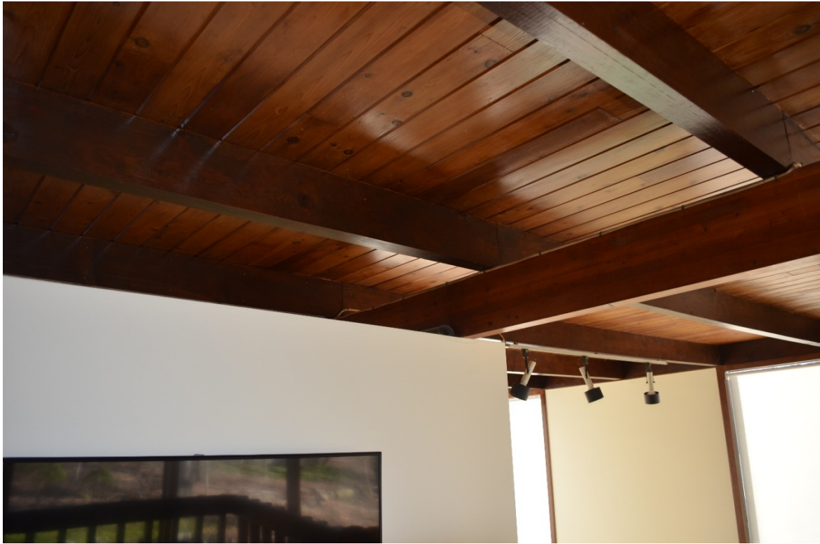
Photograph 18 of 18. The center cross beam atop the western stairwell wall.
