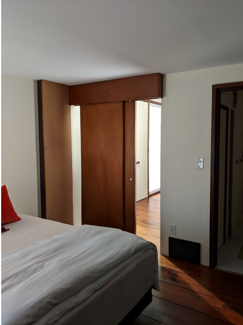
Photograph 15 of 18. Hanging sliding door between master bedroom and front entry.
