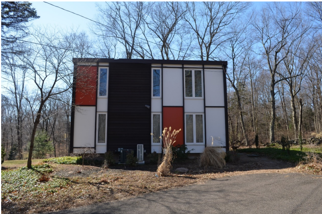
Photograph 6 of 18. North elevation of bedrooms and study; camera facing south.
