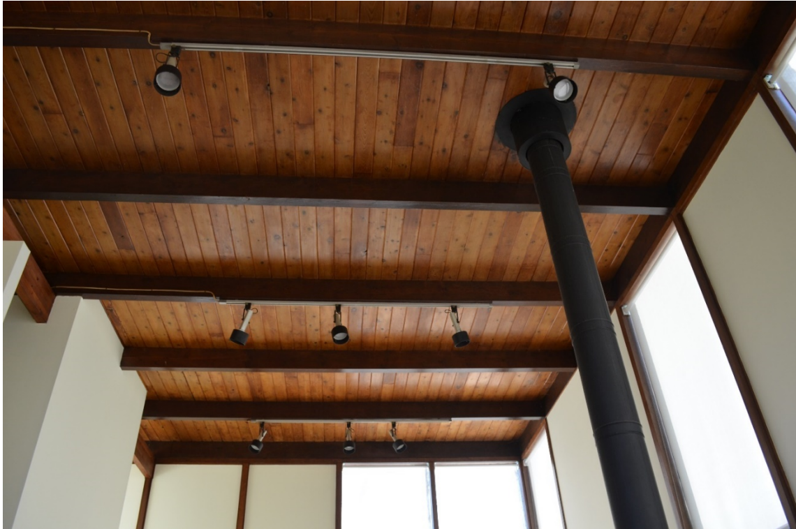
Photograph 9 of 18. Detail of exposed ceiling joists and deck over living area.
