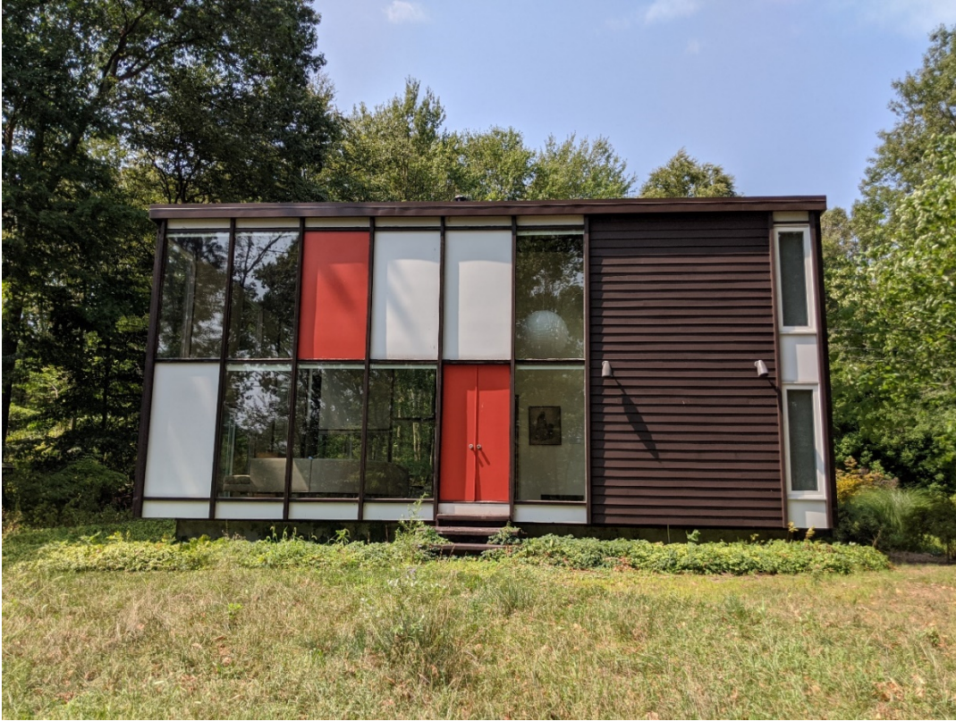
Photograph 3 of 18. Front/east elevation, camera facing west.
