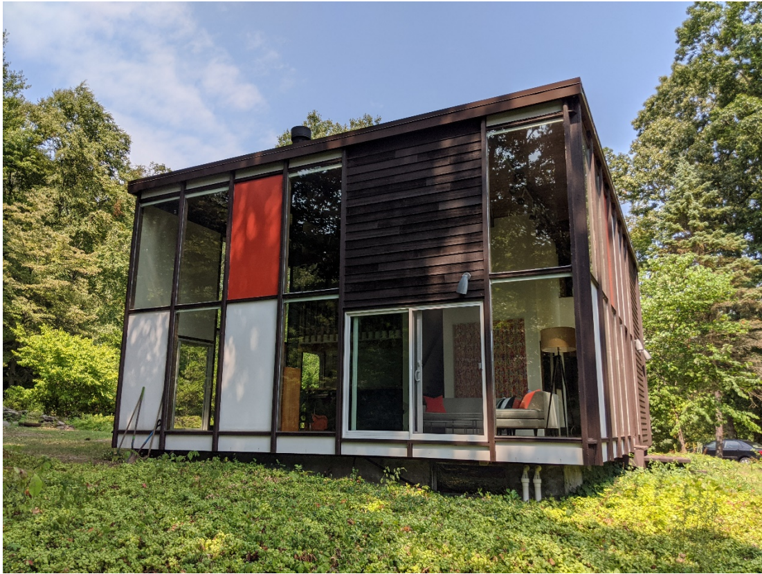
Photograph 5 of 18. South elevation, camera facing north.
