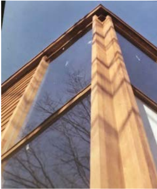
Figures 5a and 5b. Corner “L” construction details: (L) photo taken by owner during 1964 construction, courtesy Laurie Meyst; (R) 3/2020.
