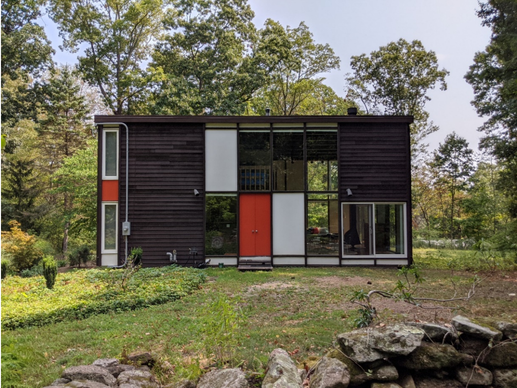
Photograph 4 of 18. West elevation, camera facing east.
