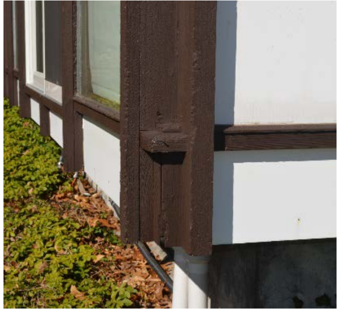
Figures 5a and 5b. Corner “L” construction details: (L) photo taken by owner during 1964 construction, courtesy Laurie Meyst; (R) 3/2020.
