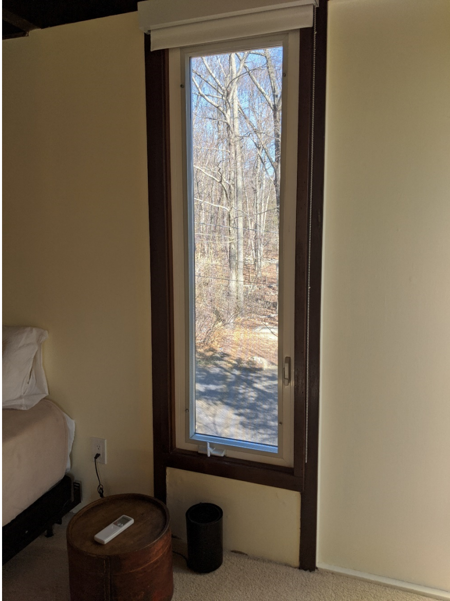
Photograph 13 of 18. Example of interior casement window framing in private spaces.
