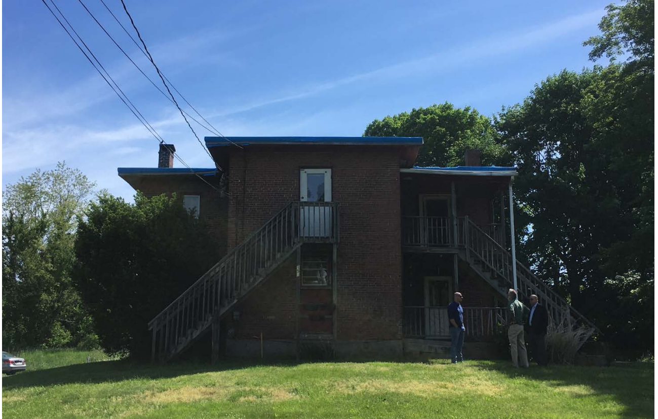
Photo of façade, camera facing east (May 2021).
