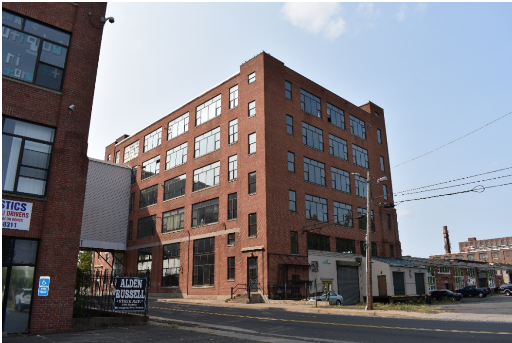
Photo 14. Landers, Frary & Clark; Building Nos. 822–824, 826, Ellis Street Bridge, and 831; looking northwest.
