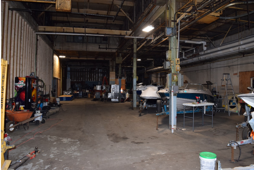
Photo 33. Landers, Frary & Clark, Building No. 822 interior, looking north.
