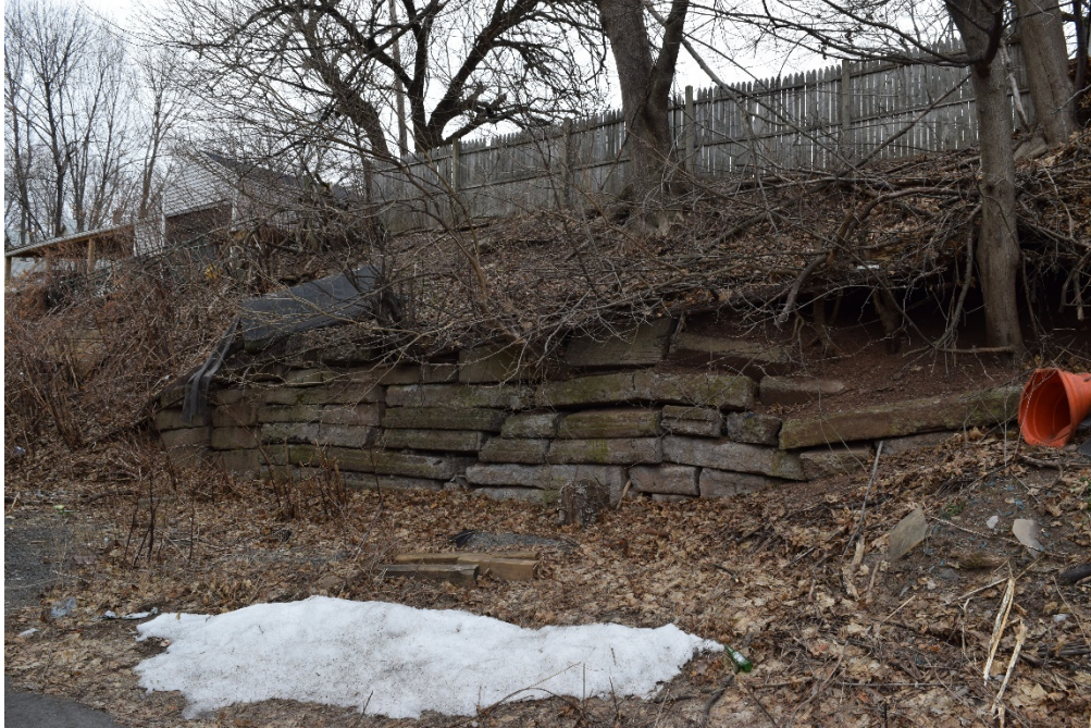
Photo 15. Landers, Frary & Clark, concrete retaining wall, looking east.
