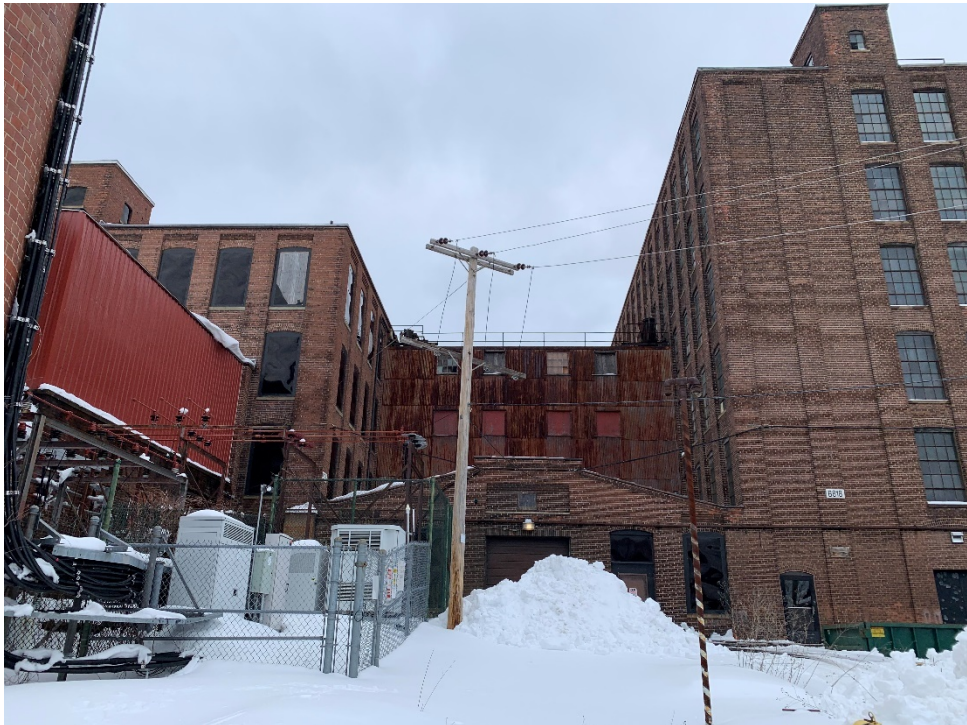
Photo 6. Landers, Frary & Clark; (left to right) Building Nos. 816, 817, 818; looking east.
