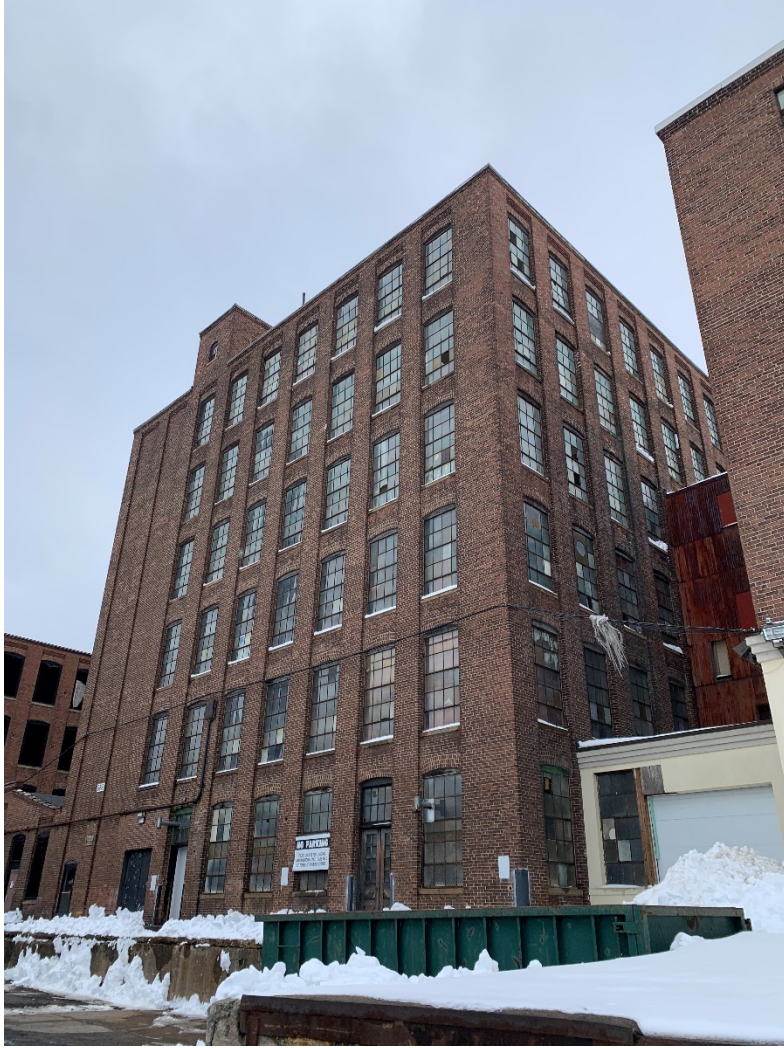
Photo 8. Landers, Frary & Clark, Building Nos. 818 and 819, looking northeast.
