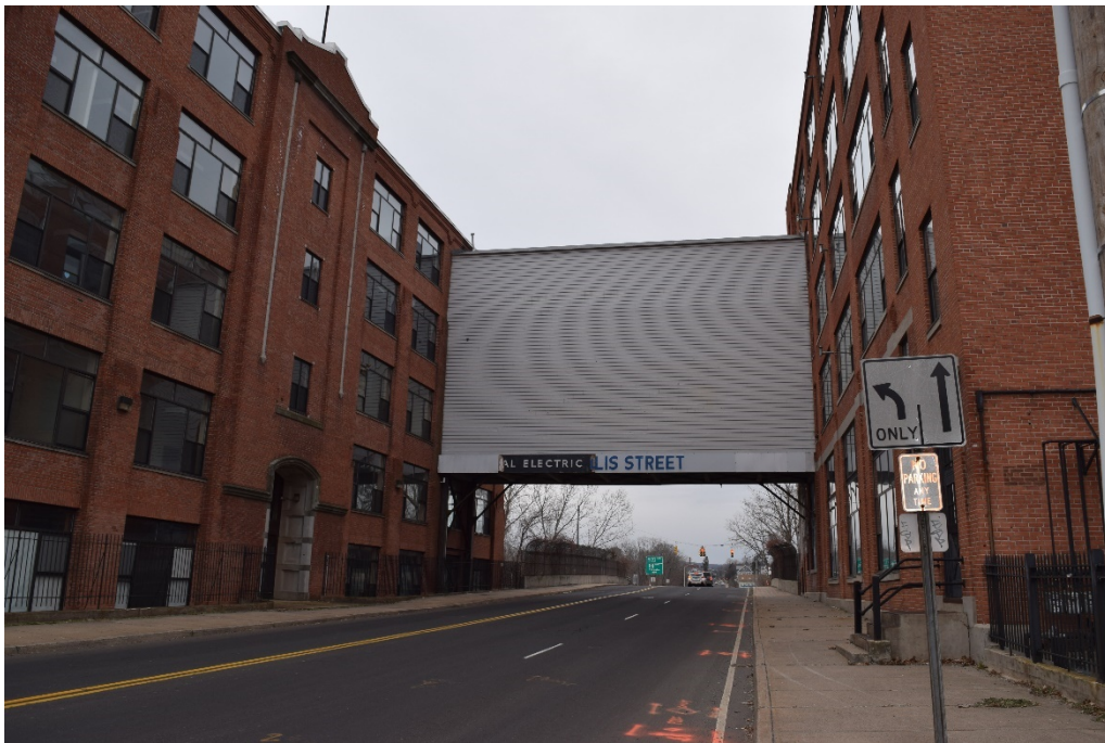
Photo 16. Landers, Frary & Clark; Building Nos. 826 and 831, and Ellis Street Bridge; looking west.
