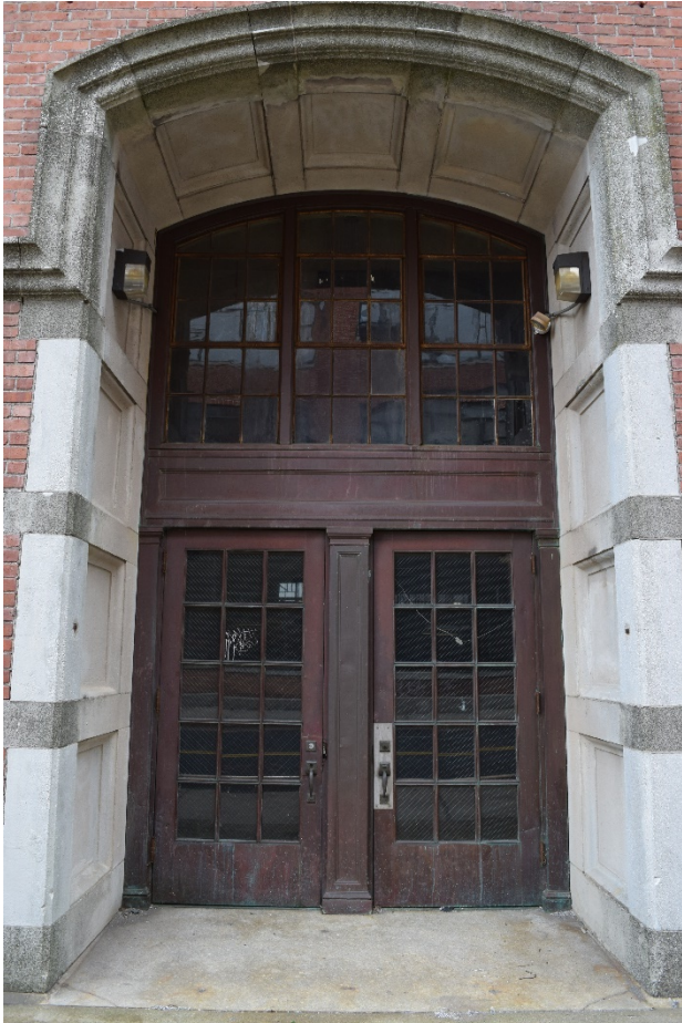
Photo 18. Landers, Frary & Clark, Building No. 831 main entrance, looking south.
