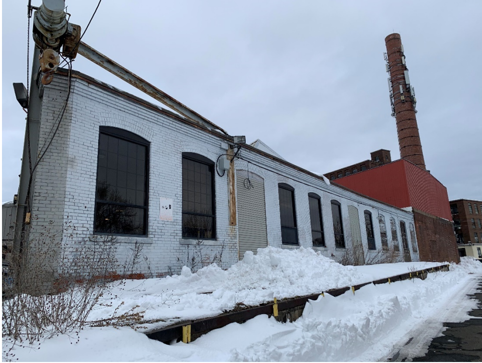
Photo 5. Landers, Frary & Clark, Building Nos. 806 and 805, looking southeast.
