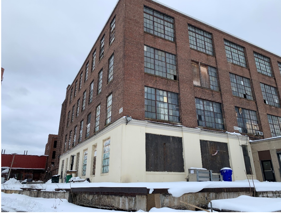
Photo 9. Landers, Frary & Clark, Building No. 820, looking northeast.
