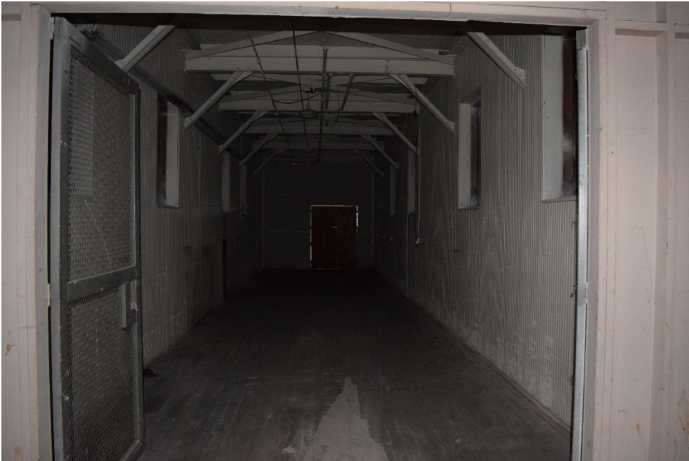
Photo 36. Landers, Frary & Clark, Ellis Street Bridge interior, looking south.
