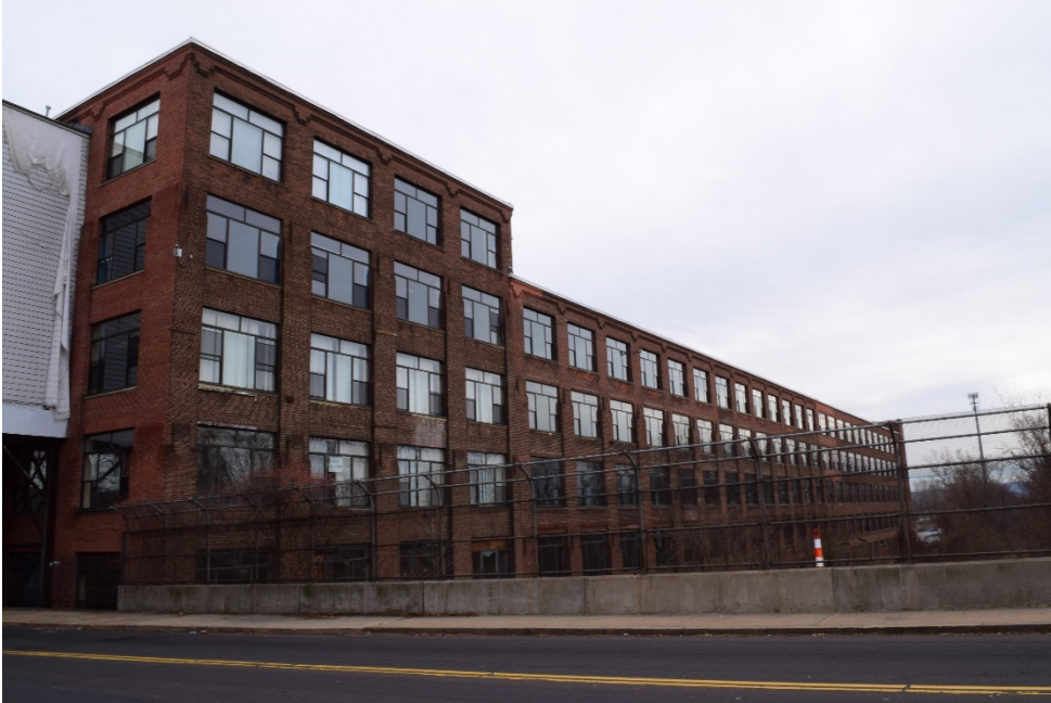
Photo 17. Landers, Frary & Clark; Building Nos. 831, 835, and 836; looking southeast.
