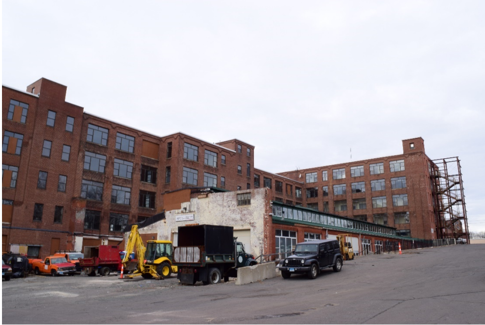
Photo 19. Landers, Frary & Clark; Building Nos. 831, 832, 835, and 836, looking northwest.
