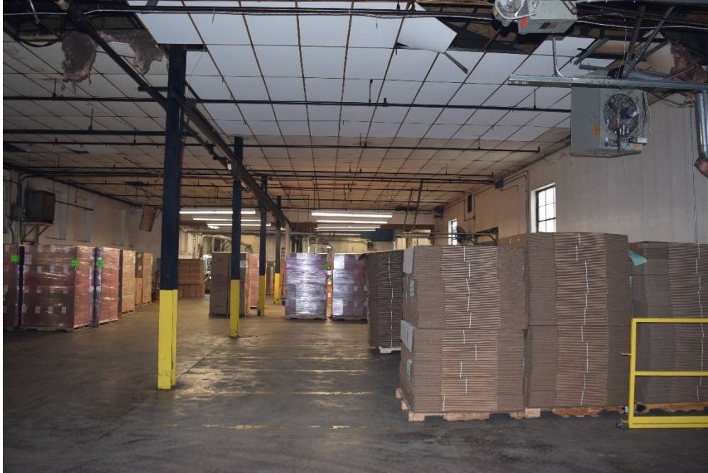
Photo 23. Landers, Frary & Clark, Building No. 804 interior, looking south.
