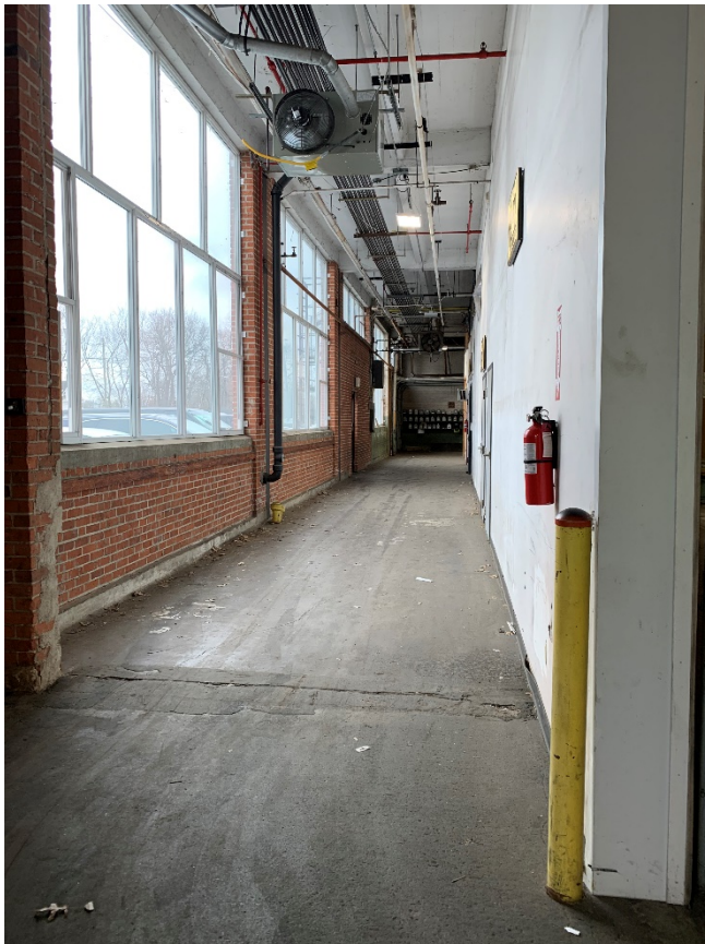
Photo 34. Landers, Frary & Clark, Building No. 823–824 interior, looking south.
