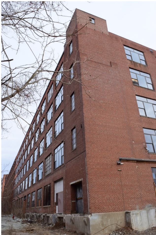
Photo 22. Landers, Frary & Clark, Building Nos. 835, and 836, looking northeast.
