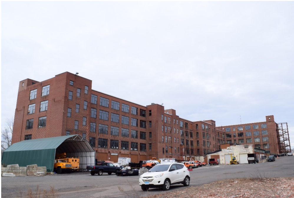
Photo 20. Landers, Frary & Clark; Building Nos. 831, 832, 835, and 836, looking northwest.
