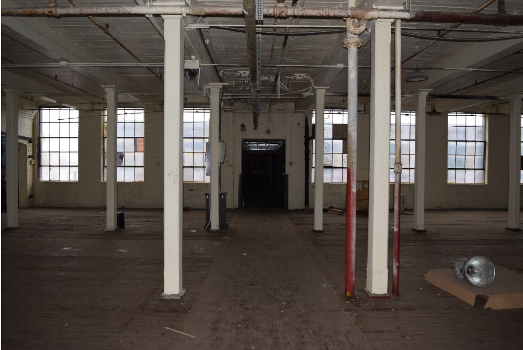
Photo 29. Landers, Frary & Clark, Building No. 818 interior, third floor, looking north.
