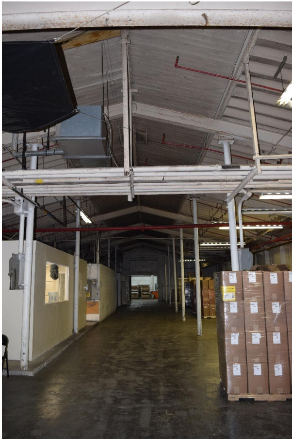
Photo 28. Landers, Frary & Clark, Building No. 817 interior, looking east.
