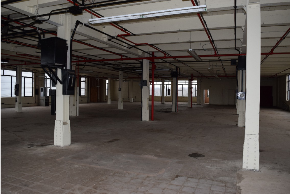
Photo 35. Landers, Frary & Clark, Building No. 825 interior, second floor, looking southwest.
