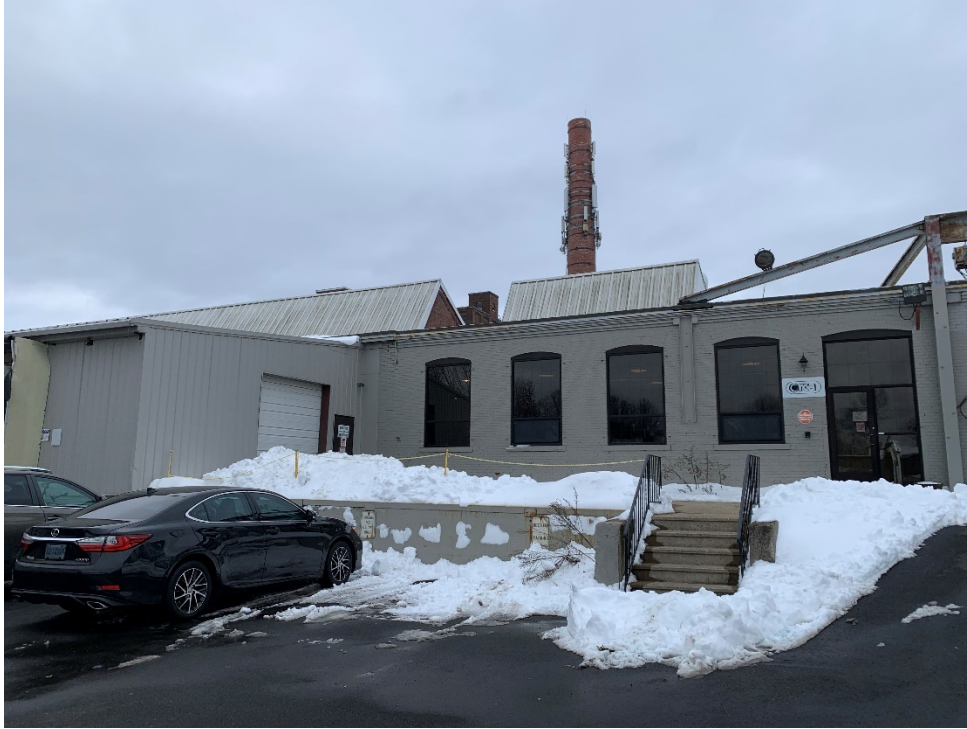
Photo 3. Landers, Frary & Clark, Building No. 806, looking southeast.
