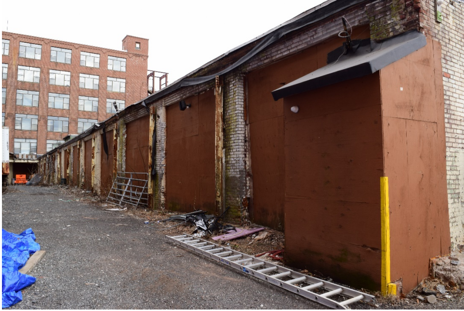
Photo 21. Landers, Frary & Clark, Building Nos. 831 and 832, looking northeast.
