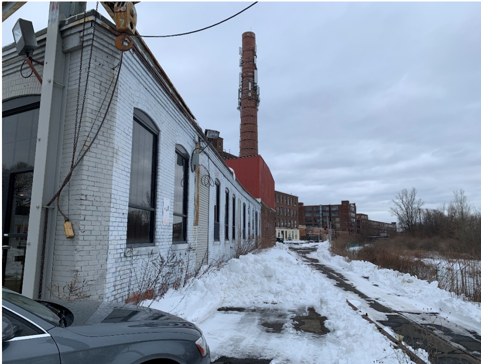
Photo 4. Landers, Frary & Clark; Building Nos. 806, 805, 820, and complex; looking southeast.
