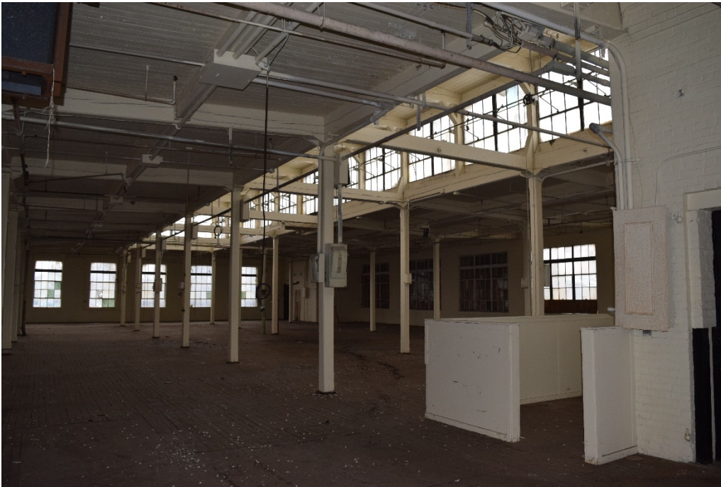
Photo 30. Landers, Frary & Clark, Building No. 820 interior, third floor, looking southeast.
