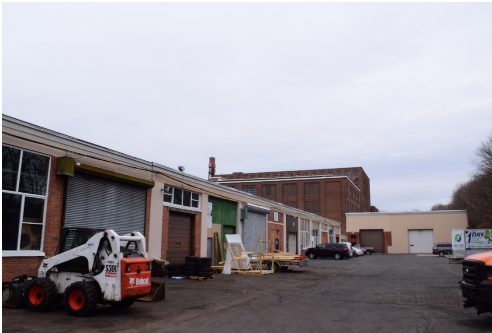
Photo 10. Landers, Frary & Clark; Building Nos. 822-824, 820, and 815; looking northwest.
