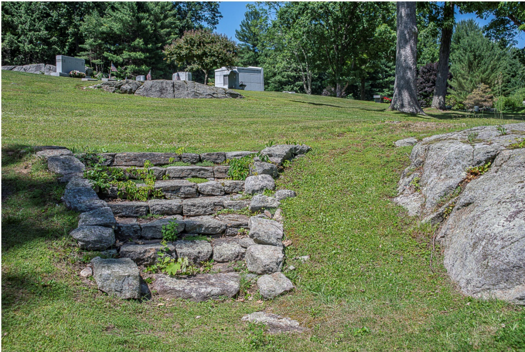
Photograph 14. View east toward Section E showing stone stairs, plantings, rock outcroppings and monuments. June 27, 2019.
