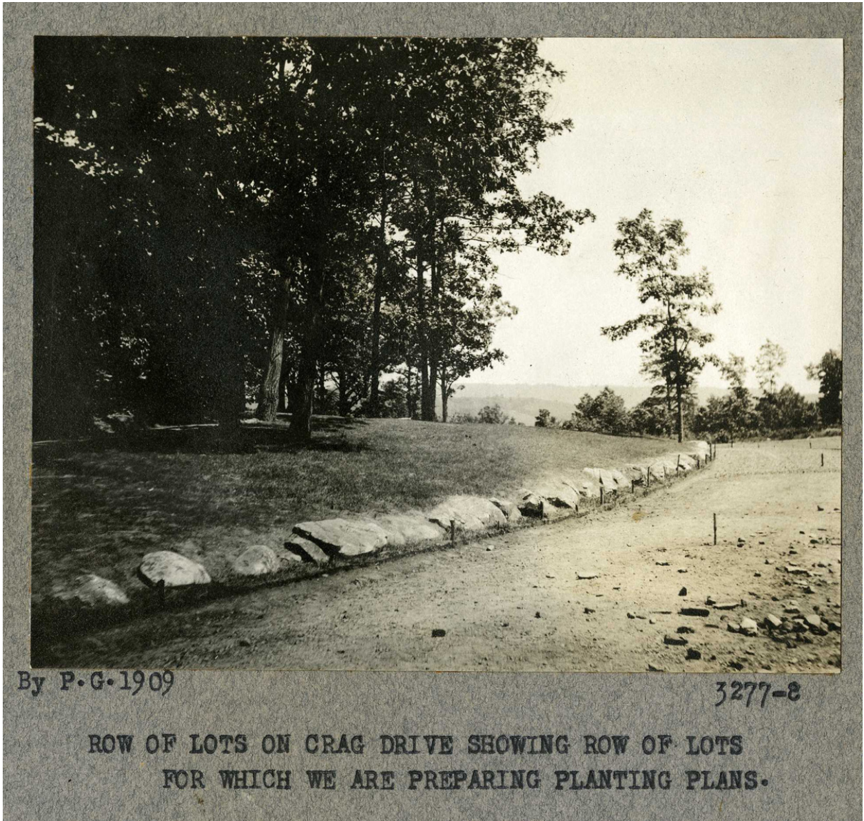
Figure 9. Shown during preliminary grading work, large stones lie along the edge of the drive to provide a naturalistic border and address the grade change of Crag Drive. The Naugatuck Valley is seen in the distance. (Torrington Historical Society, David Hosford Collection)
