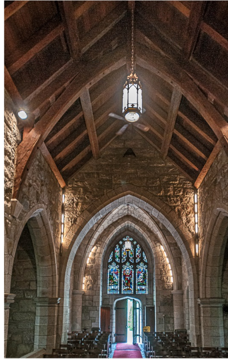
Photograph 29. Interior view north showing narthex and stained-glass window. June 6, 2014..
