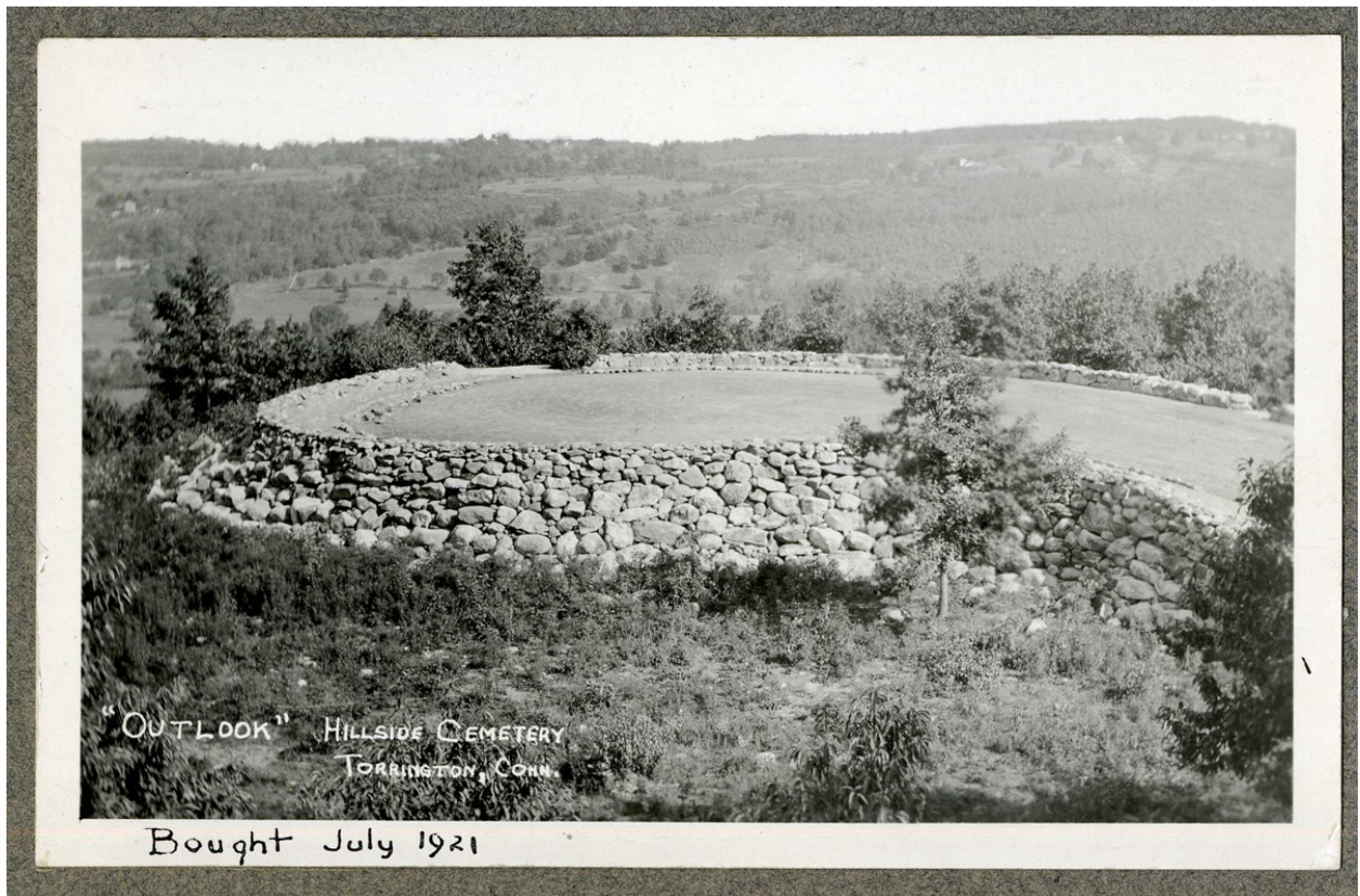
Figure 11. View east of the “Outlook” located at the terminus of Overlook Drive along the eastern ridge of the developed cemetery grounds, Hillside Overlook offers panoramic views of Torrington center and Naugatuck Valley. The overlook is constructed of compacted earth and gravel with a large stone laid back retaining wall but is now overgrown. (Torrington Historical Society, David Hosford Collection)
