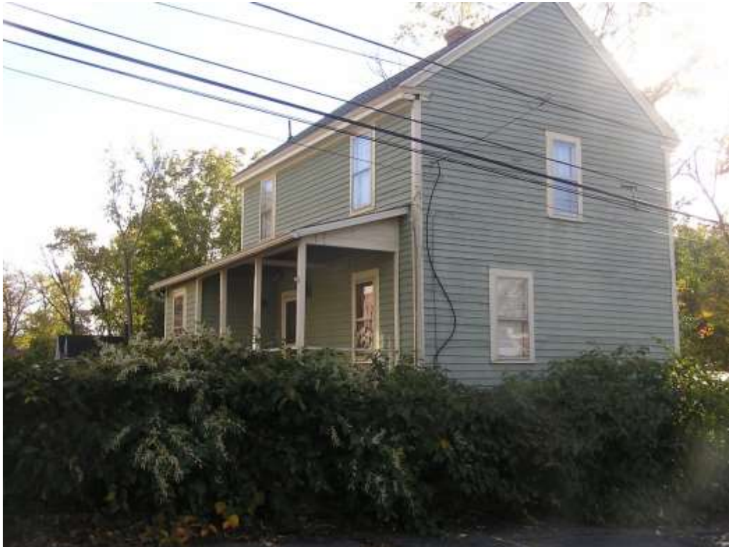
2283-2289 Main Street Rear, camera facing southwest (October 2021).
