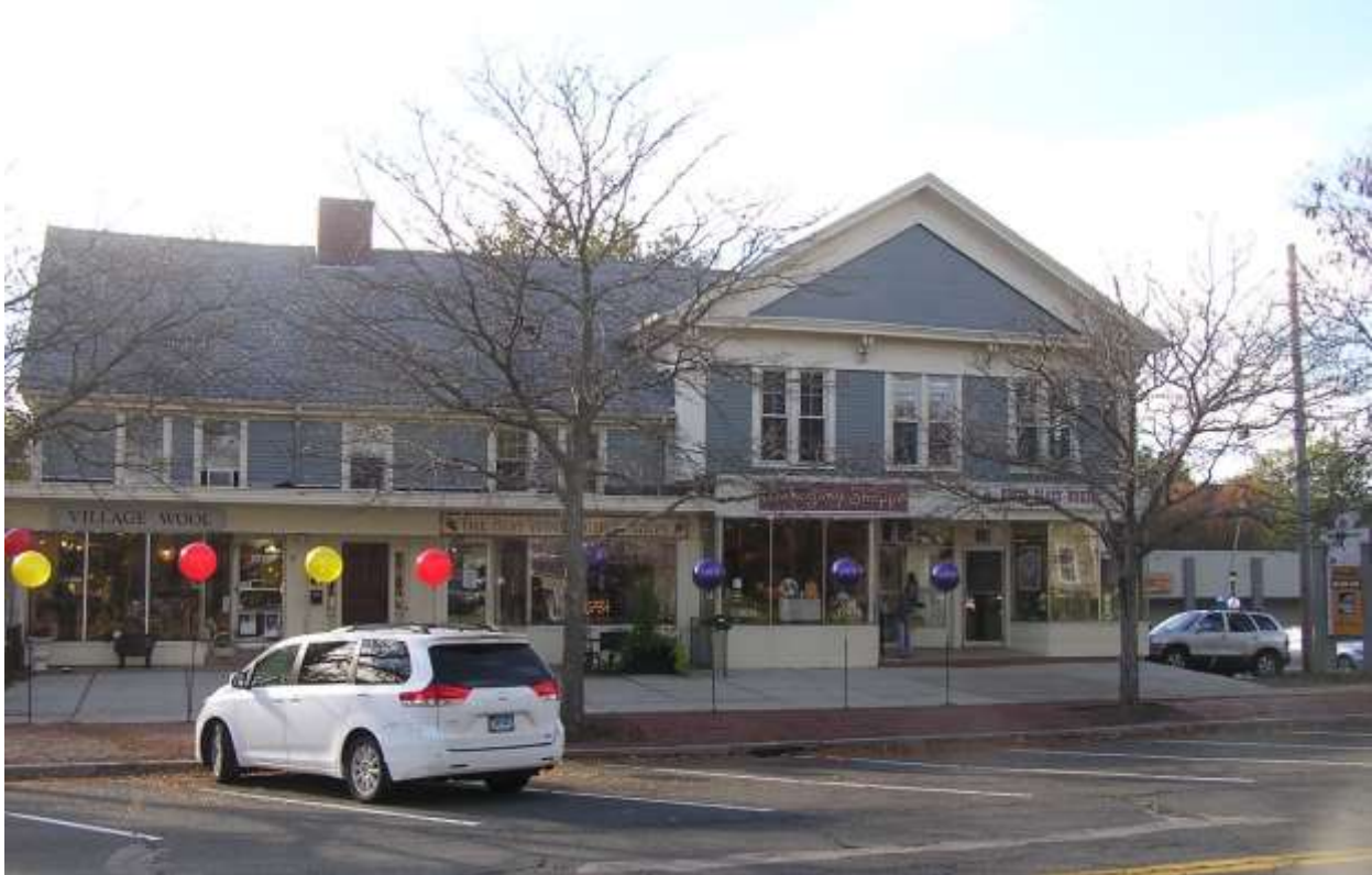
2283-2289 Main Street, facing west (October 2021).
