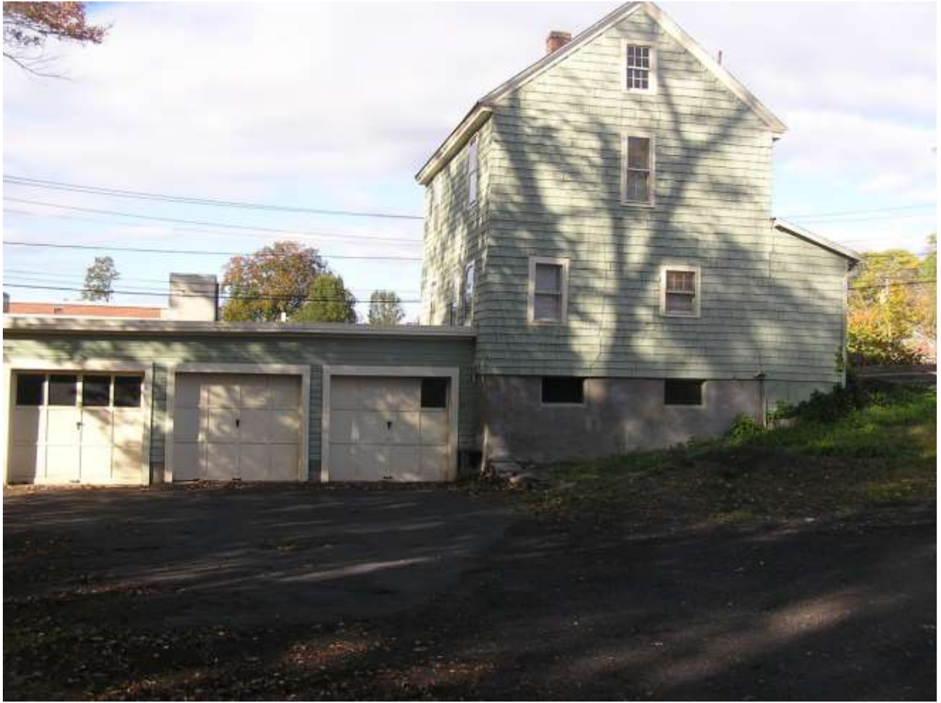
South elevation of 2283-2289 Main Street Rear, camera facing north (October 2021).
