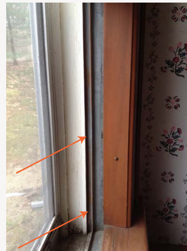
The red arrows indicate metal weather stripping that fits into a routed channel along the sides and bottom of the sash.
