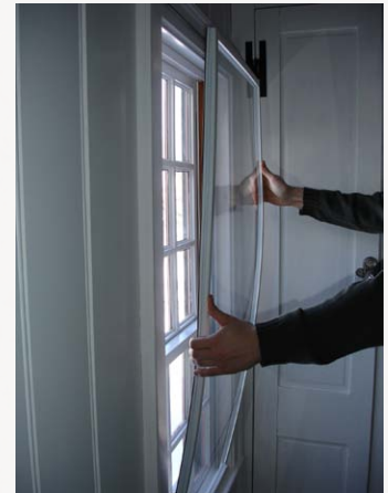
Interior storm panel.
