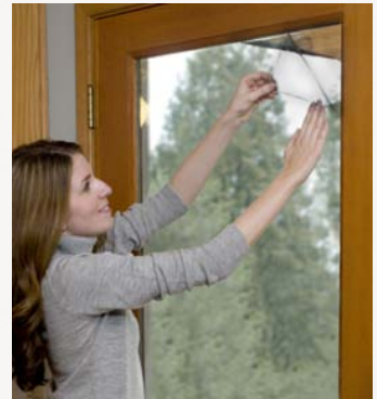
Homeowner installation of low-e interior surface film.
