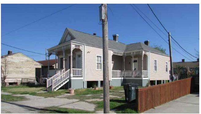
The same dwelling after being elevated 3.5 feet on both a solid and open pier concrete foundation. New stairs and a safety railing to match the original railing were added. This was a project completed for Rebuild Together New Orleans.
