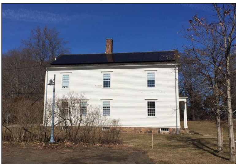
Solar panels on the south-facing roof of the Whitney Boarding House.
