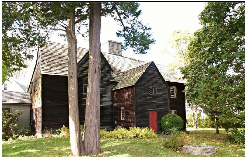
Steeply pitched roof on the Joshua Hempstead House in New London.
