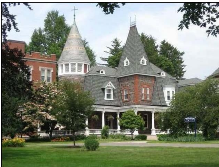
Character defining features on Lauralton Hall in Milford, CT: its asymmetrical roof, masonry walls, and porches. Source: NPS Archives.
