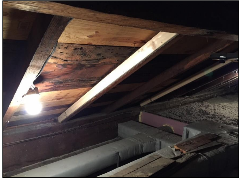
Structural reinforcements added to support the weight of solar panels.
