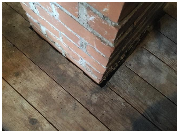
Chimney before and after air sealing with mineral wool. Photos: Marguerite Carnell.
