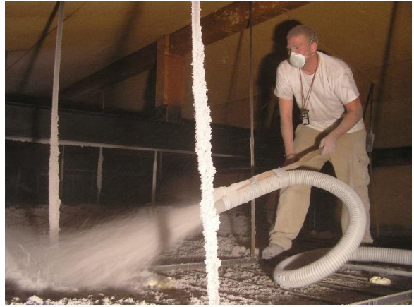
Installation of loose-pack cellulose insulation in an attic. Source: Greenbuildingadvisor.com .
