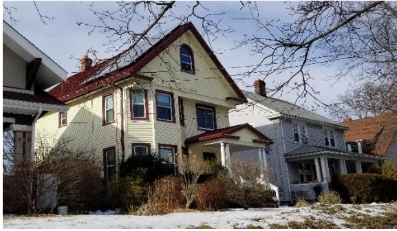
Do: Place panels on a nonpublic facing slope
