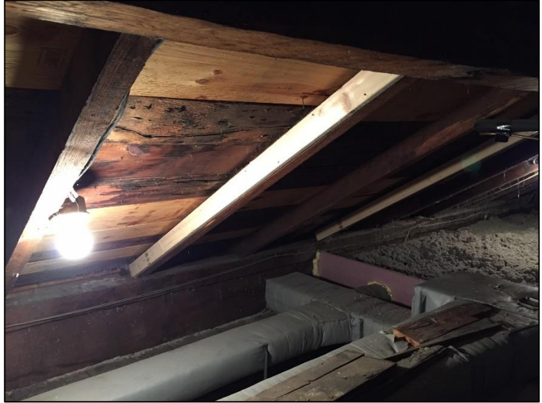
Structural reinforcements added to support the weight of solar panels. Photo: Stacey Vairo.
