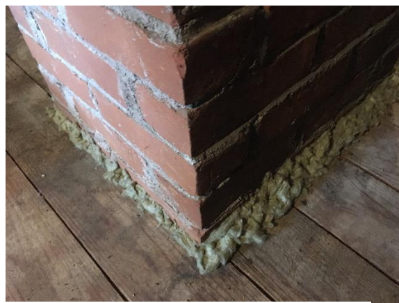
Chimney before and after air sealing with mineral wool. Photos: Marguerite Carnell.
