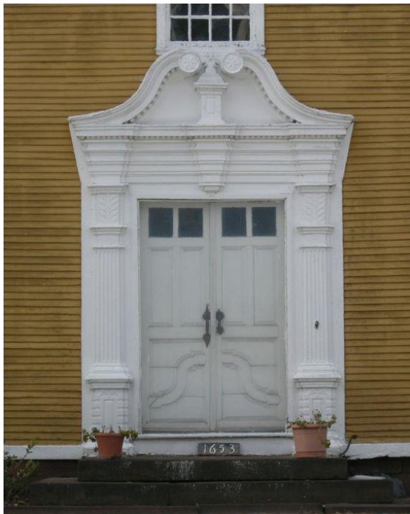
A typical Connecticut River Valley Doorway, South Windsor. Source: SHPO Archives.
