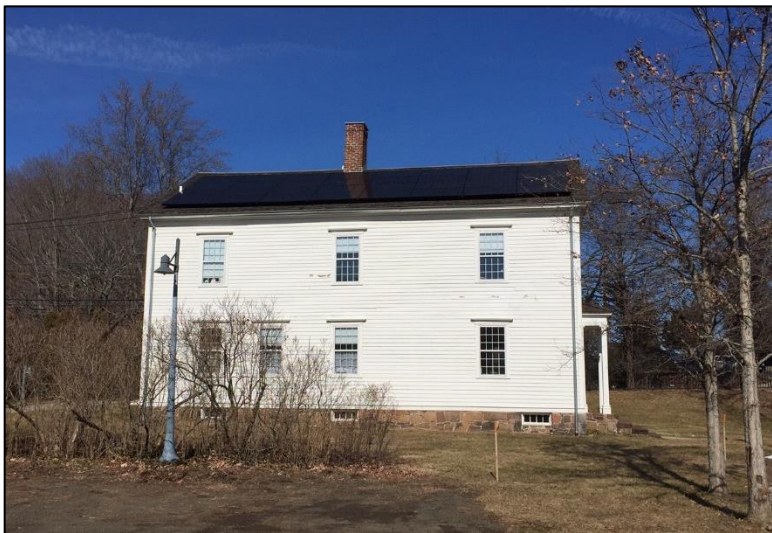
Solar panels on the south-facing roof of the Whitney Boarding House. Photo: Stacey Vairo.
