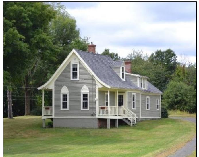
Double-hung windows on a Gothic Revival cottage, Suffield. Photo: Lucas Karmazinas
