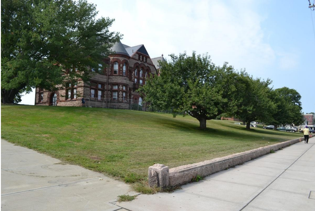
View southwest toward the Williams Memorial Institute building from the sidewalk along Broad Street with the stone curbing that may date to the Olmsted design.
