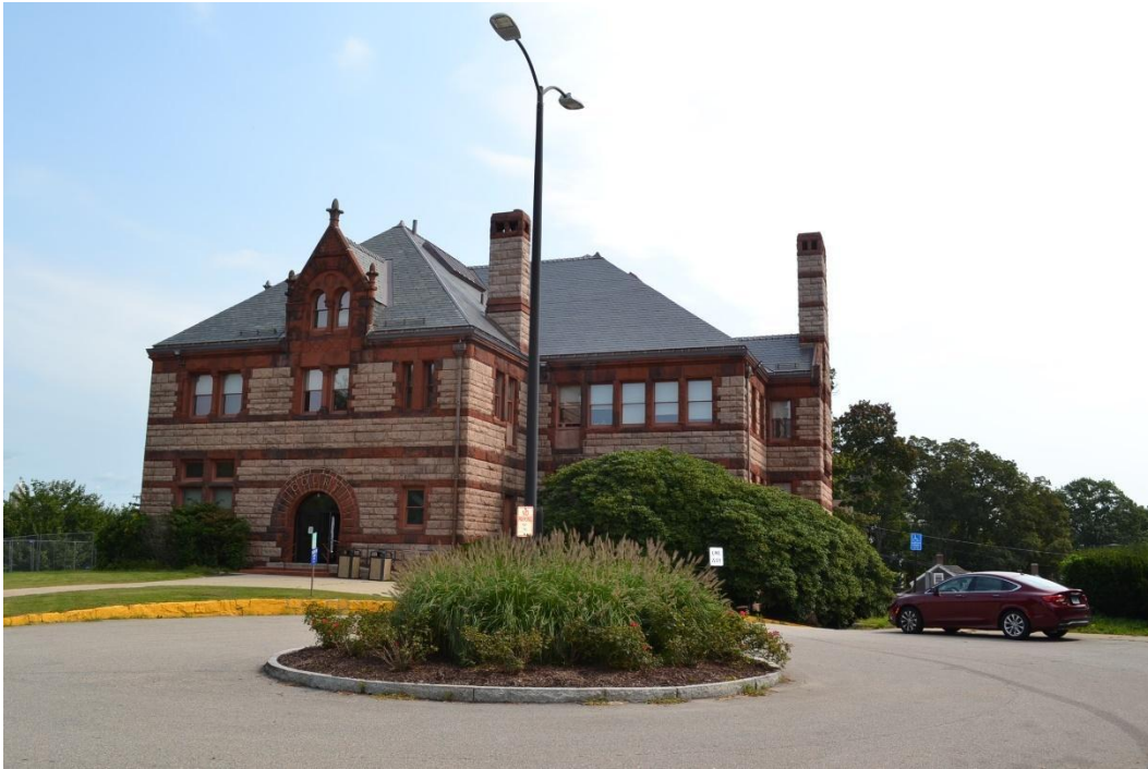
View east toward the present-day principal entrance into the building from the internal access road.
