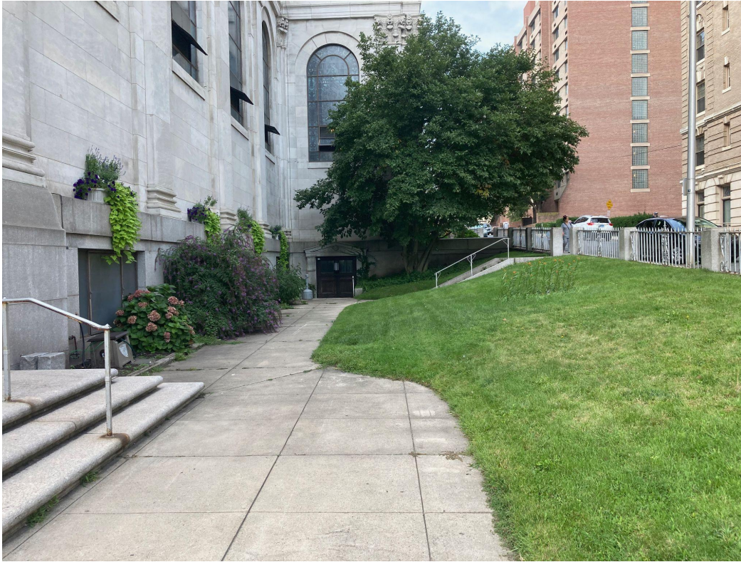
View north along eastern side of basilica.
