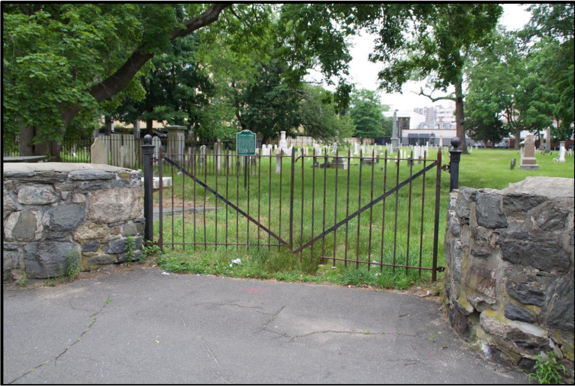
Photograph 11 of 25: Western entrance at Franklin Street, curved masonry wall, and cast and wrought iron gate, facing east
