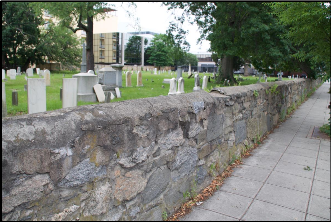
Photograph 9 of 25: Stone masonry wall along North Street, facing northeast
