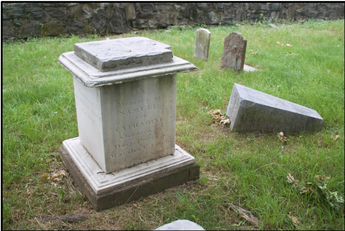
Photograph 25 of 25: Obelisk monument separated from pedestal, facing west
