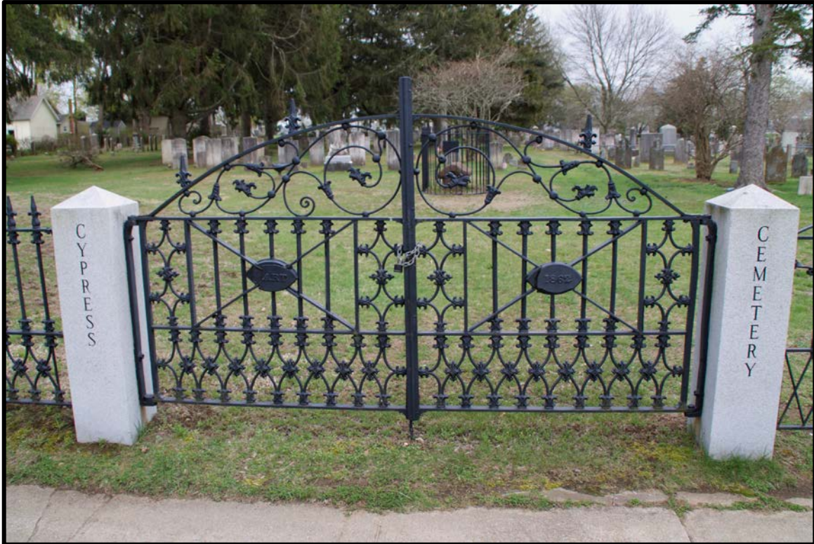
Photograph 5 of 36: Cast-iron gate at the pedestrian entrance on College Street (C. Harris)
