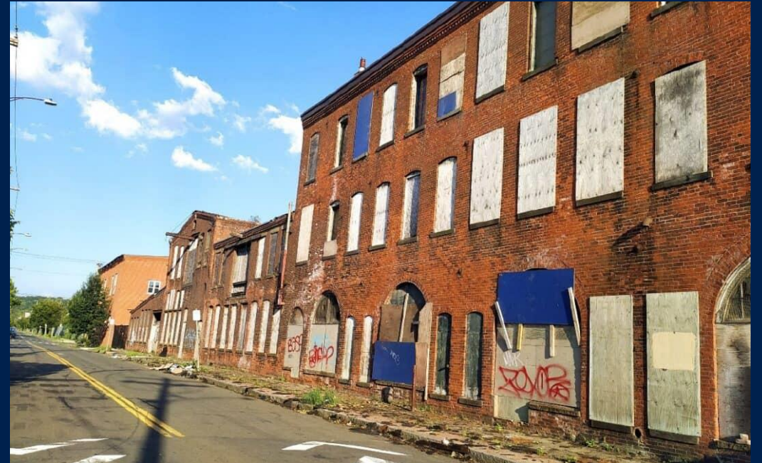
Bigelow Boiler Complex, New Haven, CT.
