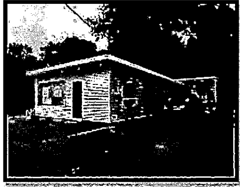
2. VACANT COMMERCIAL PROPERTY
