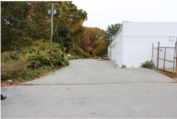
Photo #6: Rear of building overview west corner.
