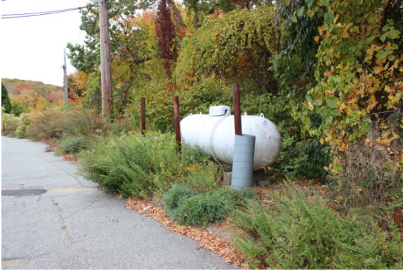
Photo #9: Rear of building unsecured gas tank.
