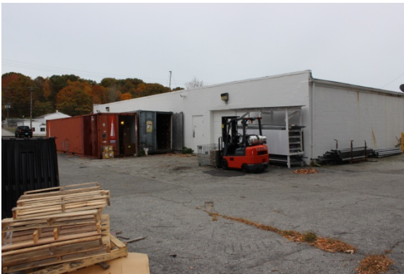
Photo #10: Overview north corner of building.
