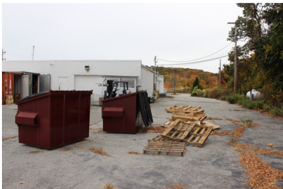
Photo #8: North corner of building overview.
