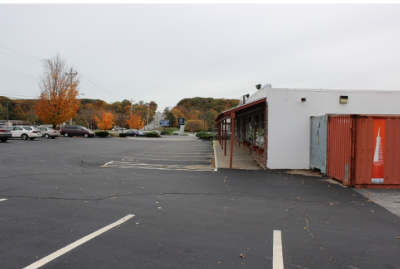
Photo #11: East corner of building.
