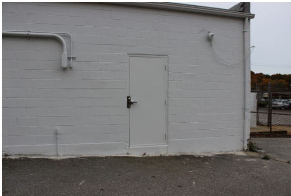
Photo #7: Rear entrance door west corner of building.
