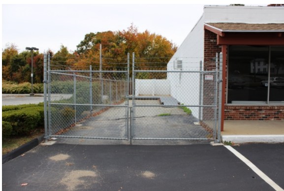
Photo #4: South corner of building fenced loading/unloading area.
