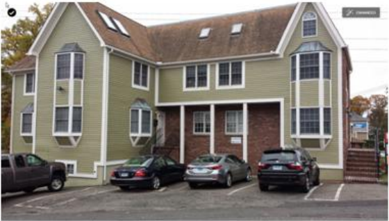
North Side of Building
