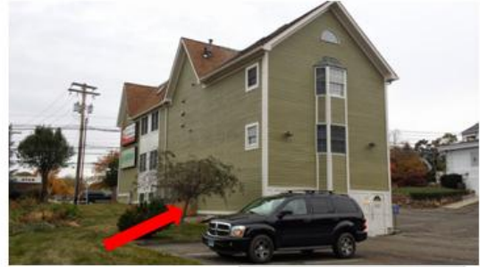
East Side of Building
