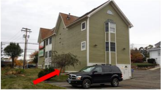
East Side of Building
