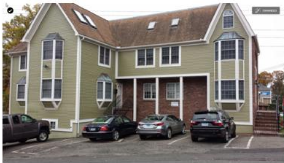
North Side of Building
