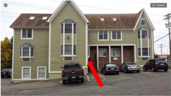
North Side of Building
