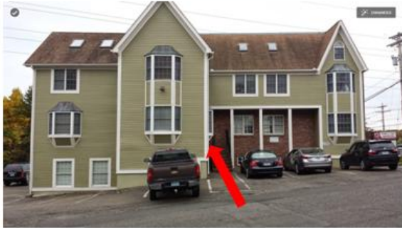
North Side of Building
