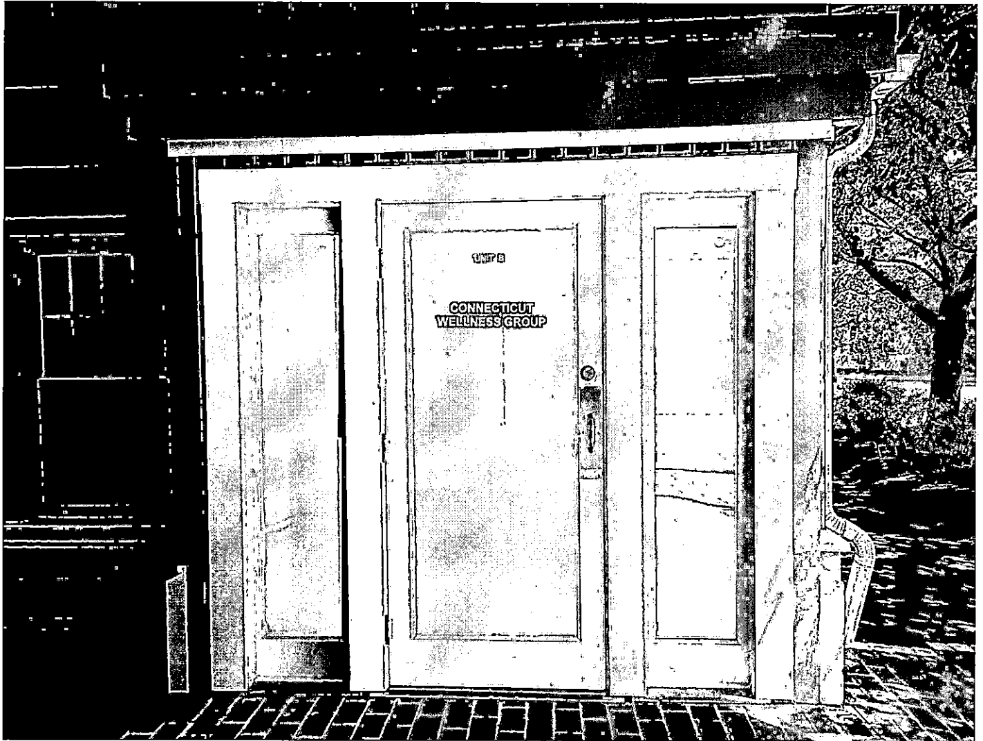
Front Entrance with Actual Signage FRONT ENTRANCE (All glass will be frosted for privacy)
